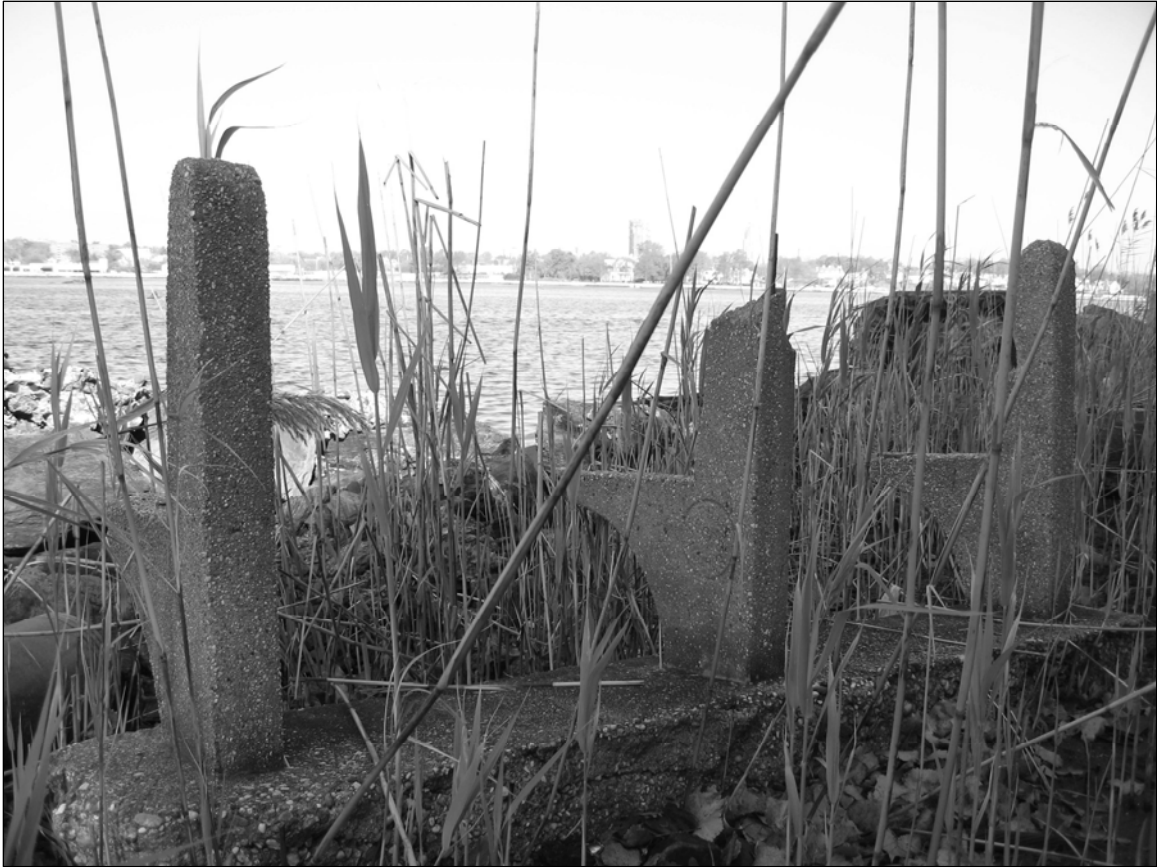
Photo 8. Concrete bench frame, vicinity of Building 11, facing northwest.
