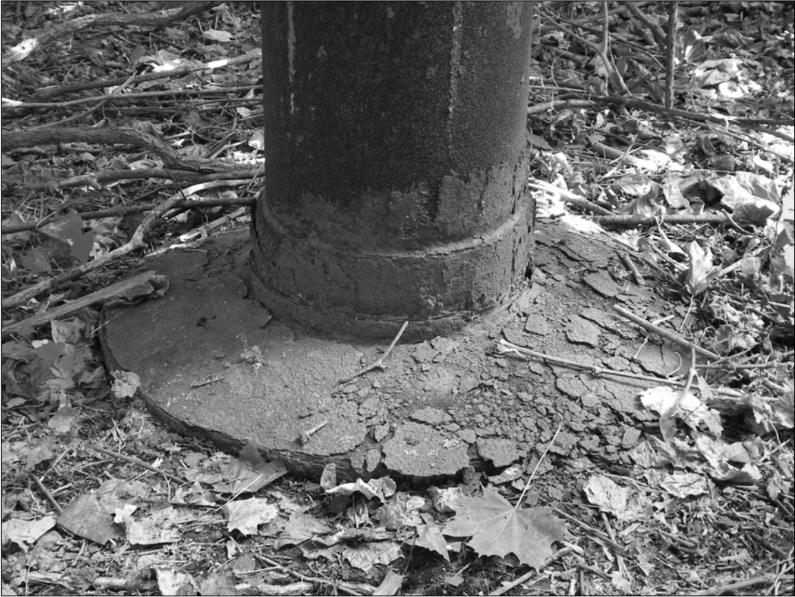
Photo 4. Flagpole base, detail, facing southeast.
