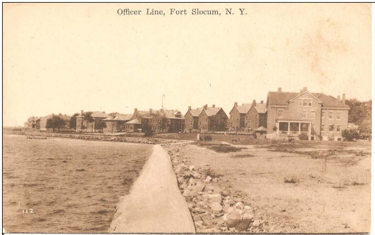
Figure 6. "Officer Line, Fort Slocum, N.Y.," circa 1917, facing north-northeast. Divided back postcard published by Italia Art Co. Italia Art Co., New York. No copyright date or postmark. Photograph shows Segment C of the seawall on the western shore of Davids Island. Note that the top of the wall has been covered with a layer of concrete. Officers' Quarters (Building 35) is at right. In the background are (right to left) Buildings 9, 10, 11 (with flagpole [erected 1914] behind it), 12, 13, 42, and 43. The Officers' Bathing Pier (built 1920) is absent from this scene. Collection of Christopher L. Borstel, Tetra Tech EC, Inc., Morris Plains, NJ.
