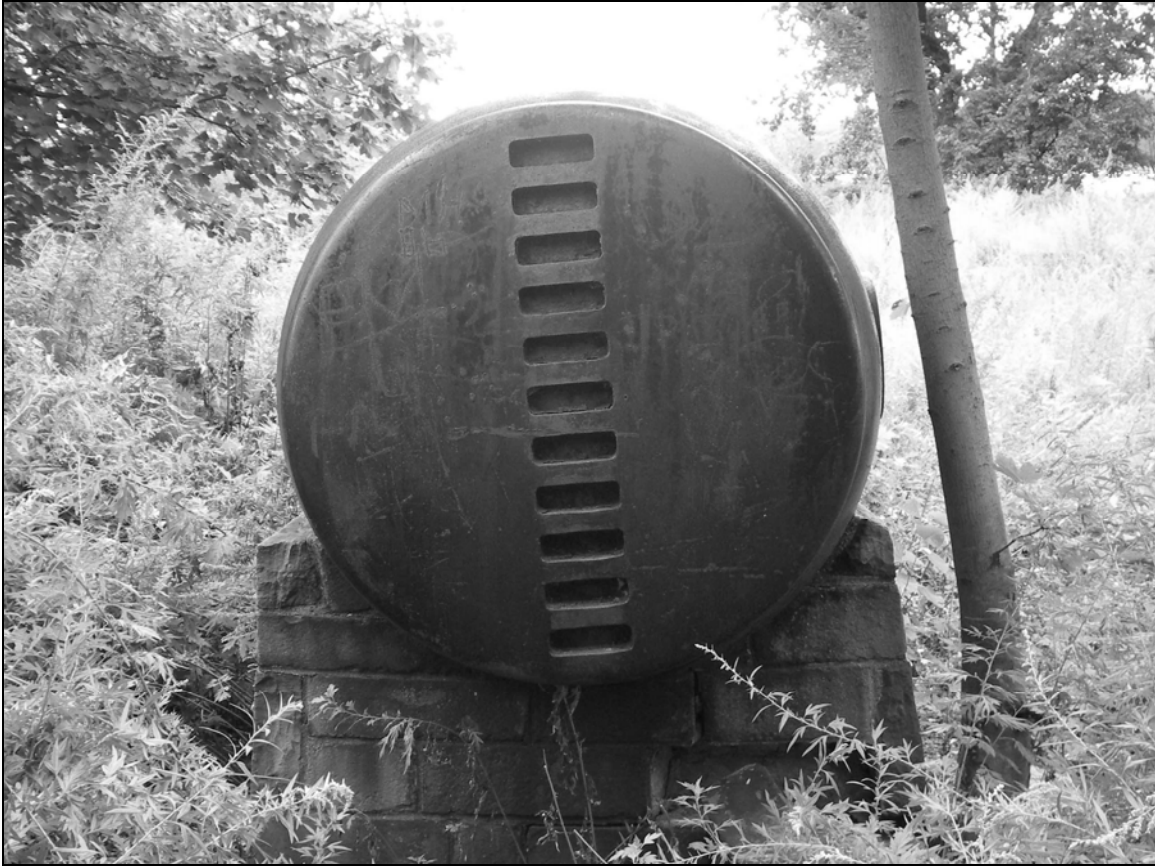
Photo 4. Rodman Gun Monument, rear knob and lifting notches detail, facing southwest.
