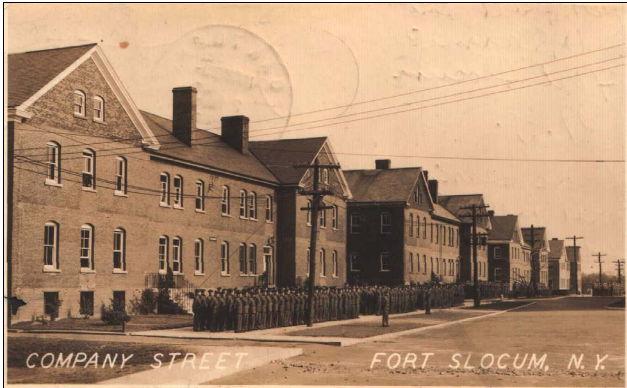
Figure 14. "Company Street, Fort Slocum, N.Y.," circa 1940, facing southeast. Real-photo postcard by unidentified publisher. No copyright date; illegible postmark, circa 1940. This view of Bomford Road shows a wide thoroughfare that saw much use for parading and daily inspections. The company barracks at left are Buildings 64-61. Collection of Christopher L. Borstel, Tetra Tech EC, Inc., Morris Plains, NJ.
