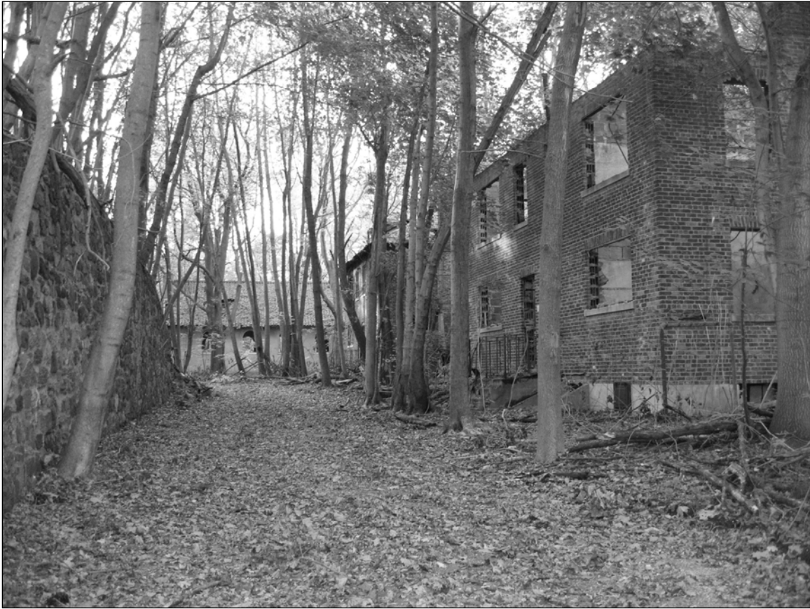
Photo 12. Hartshorn Road, facing west. The road and the retaining wall at left were constructed in 1939-1940. The Post Chapel (Building 108) is at center, Buildings 107 and 106 at right.
