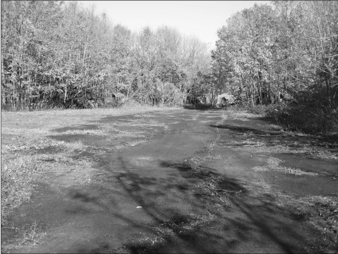
Photo 9. Bomford Road, vicinity of Building 64, facing north.
