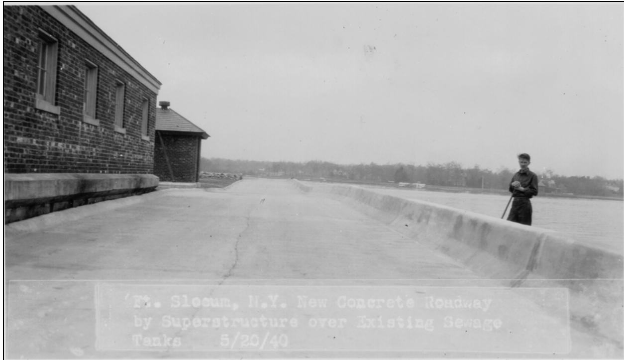
Figure 16. Recently-constructed section of Parker Road beside Sewage Tank House (present-day Building 52), May 1940, facing northwest. Contrast this image with the collapsed roadway and seawall in Photo 7 of current conditions. Record Group 77, National Archives, College Park, MD.
