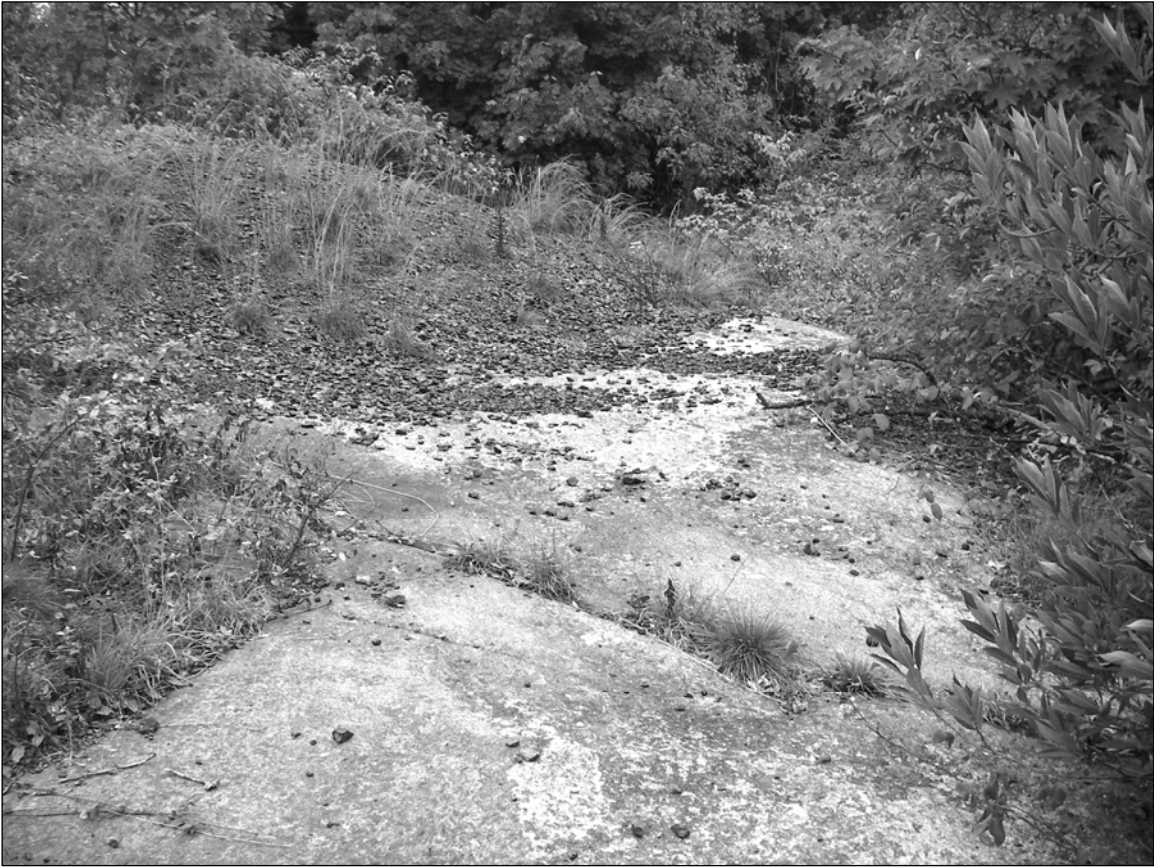
Photo 3. Battery Practice, abandoned coal pile in the southeastern interior corner of the concrete revetment and vicinity, facing south.
