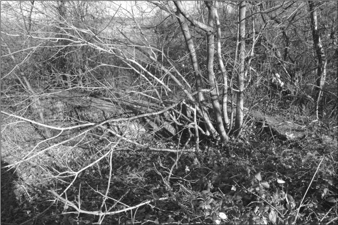
Photo 1. Battery Practice, south section of concrete revetment from interior showing bow in wall for Gun No. 1 emplacement (behind clump of small tree trunks at center), facing east.
