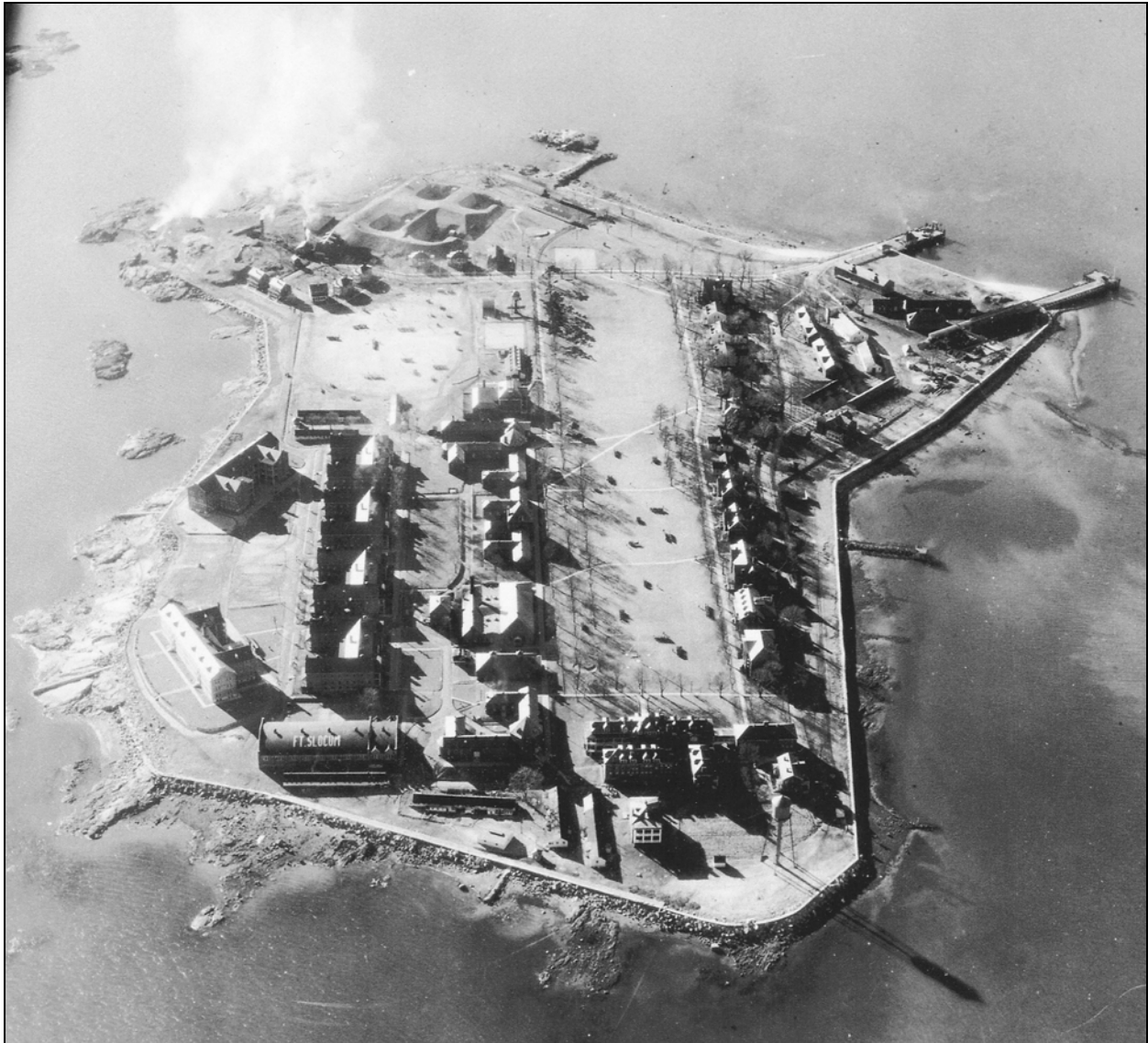
Figure 7. Oblique aerial view of Fort Slocum, January 1936, facing south. Showing Davids Island at low tide, this photograph illustrates the extent of the seawall around the northern three-quarters of the island. Original in National Archives, College Park, MD; digital copy from Fort Slocum Alumni and Friends Collection, Michael A. Cavanaugh, Los Angeles, CA, custodian.
