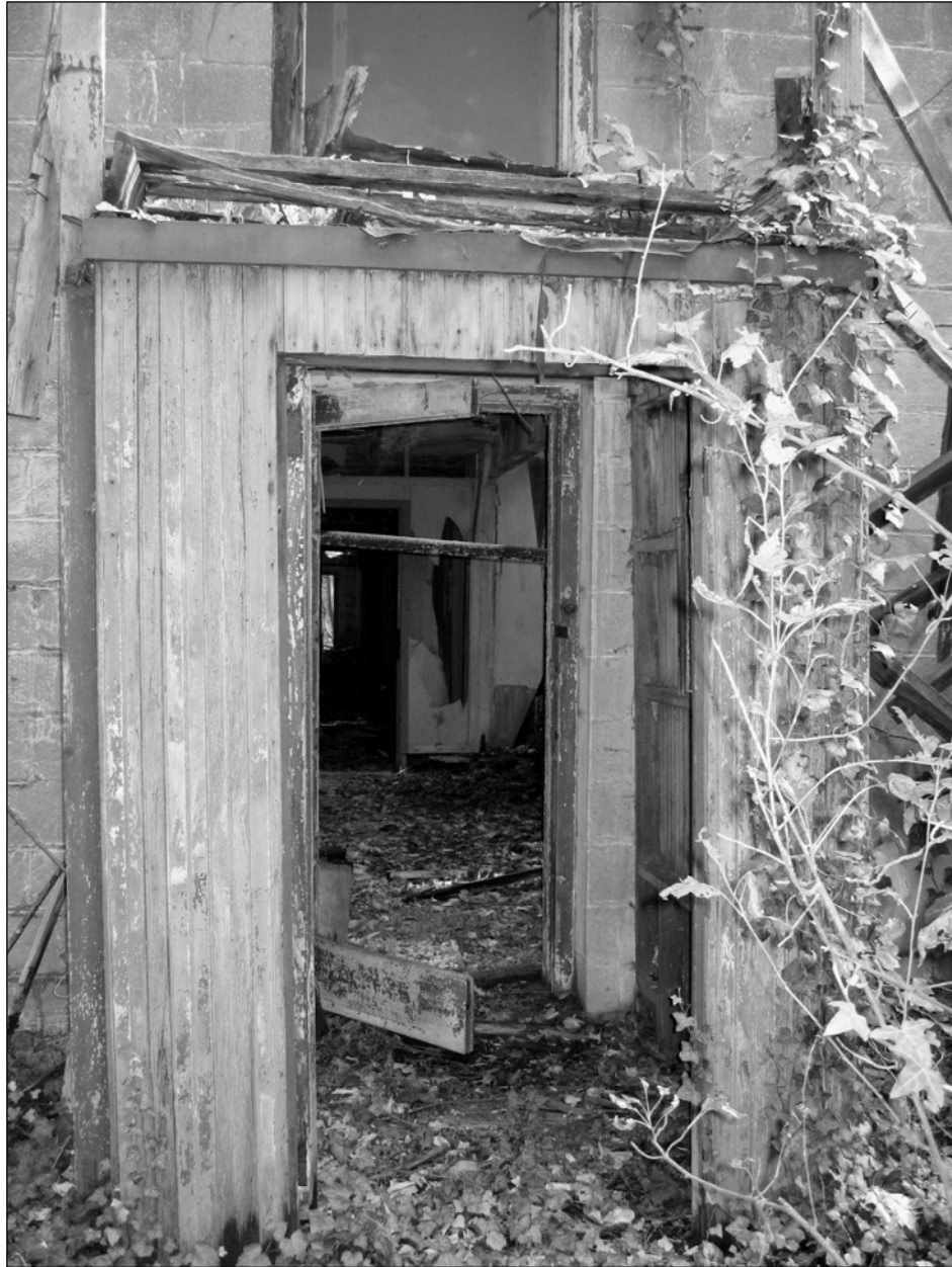
Photo 7. Northwestern façade, detail: first-floor vestibule and second-floor porch, facing southeast.
