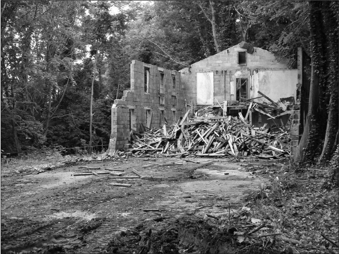
Photo 8. Building 134 during demolition, facing northwest.
