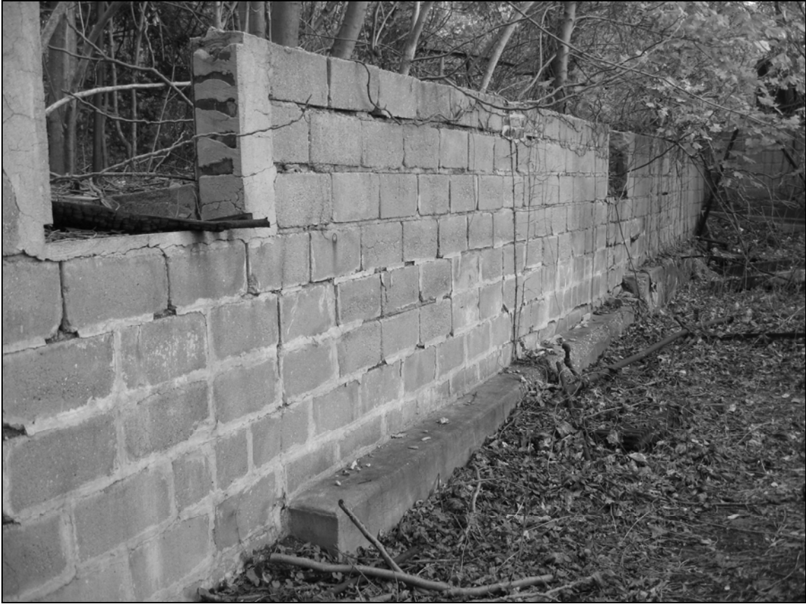
Photo 2. Foundation interior, northeastern wall near westerly end, facing southeast.
