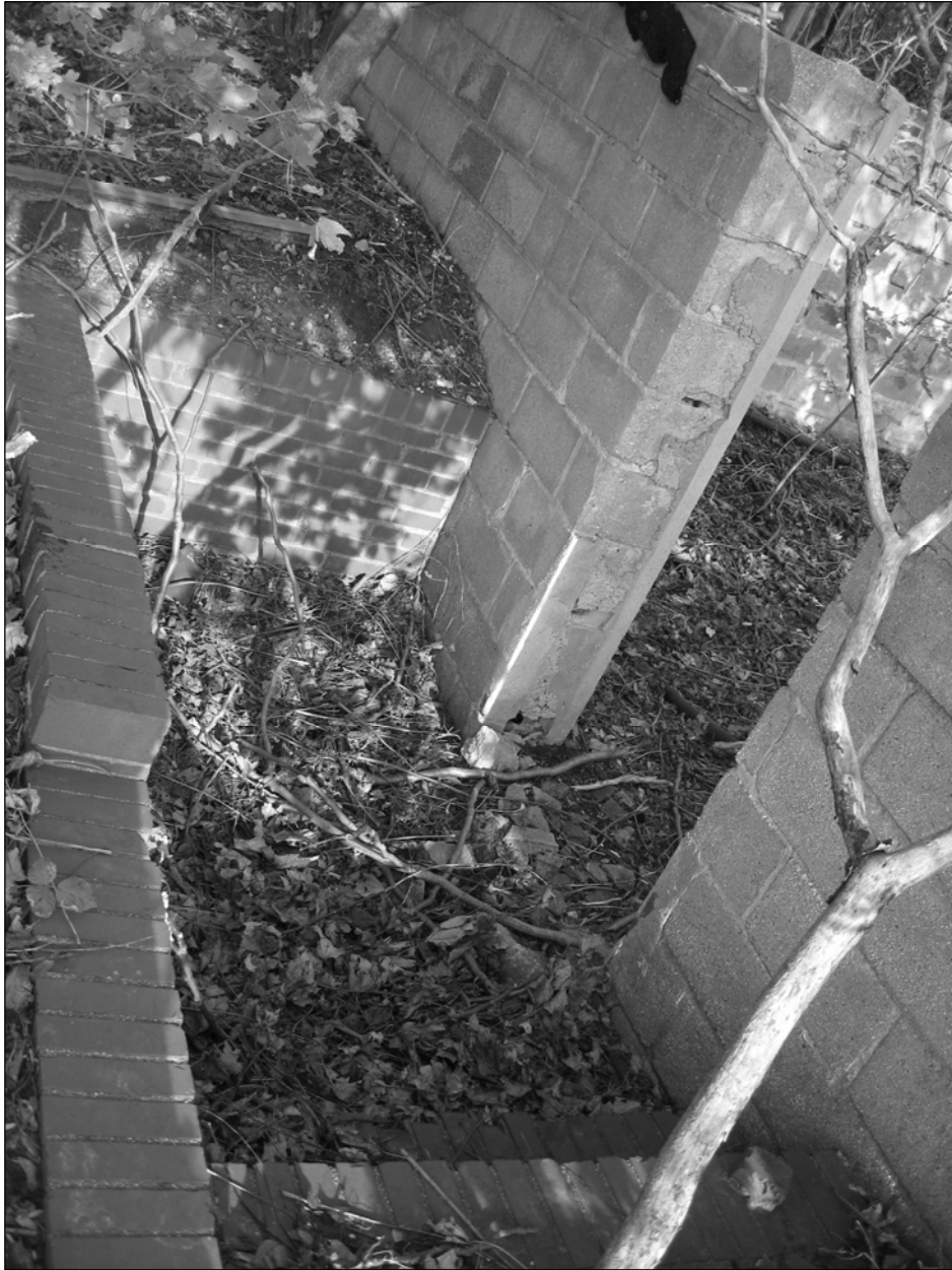
Photo 4. Northwestern end of foundation ruin at crawlspace entrance, facing northeast.
