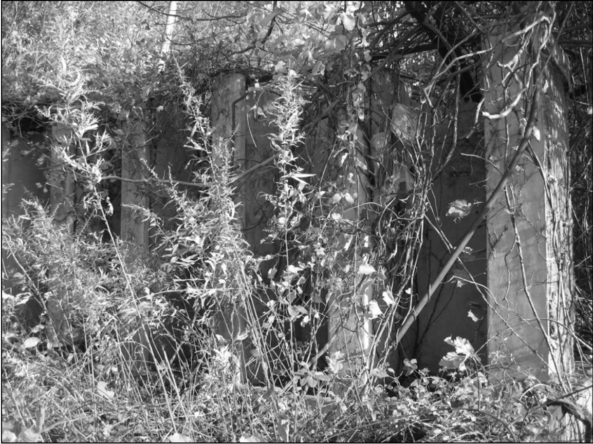
Photo 5. Cast concrete shower enclosures near center of foundation, facing southeast.
