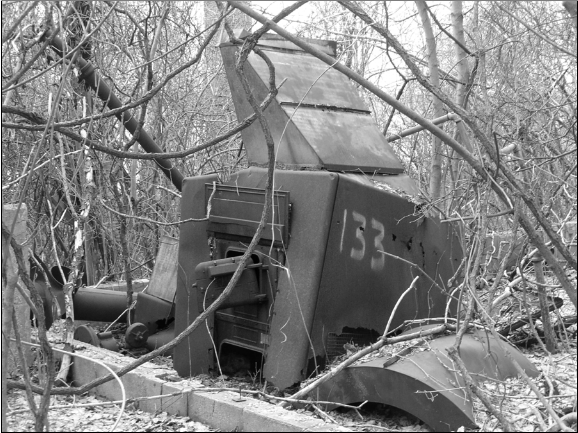
Photo 2. Boiler at southeastern end of ruin, facing west.
