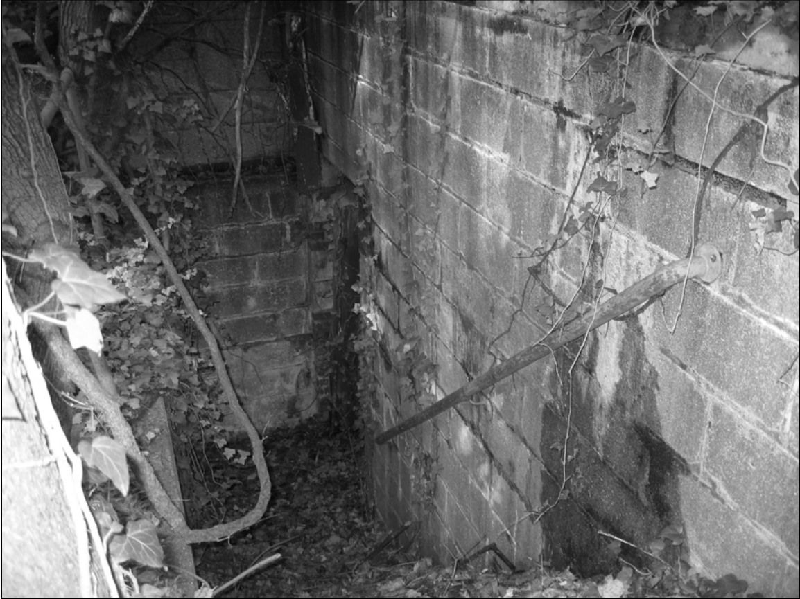
Photo 5. Stairwell to boiler room on southwestern side of dependency, facing northwest.
