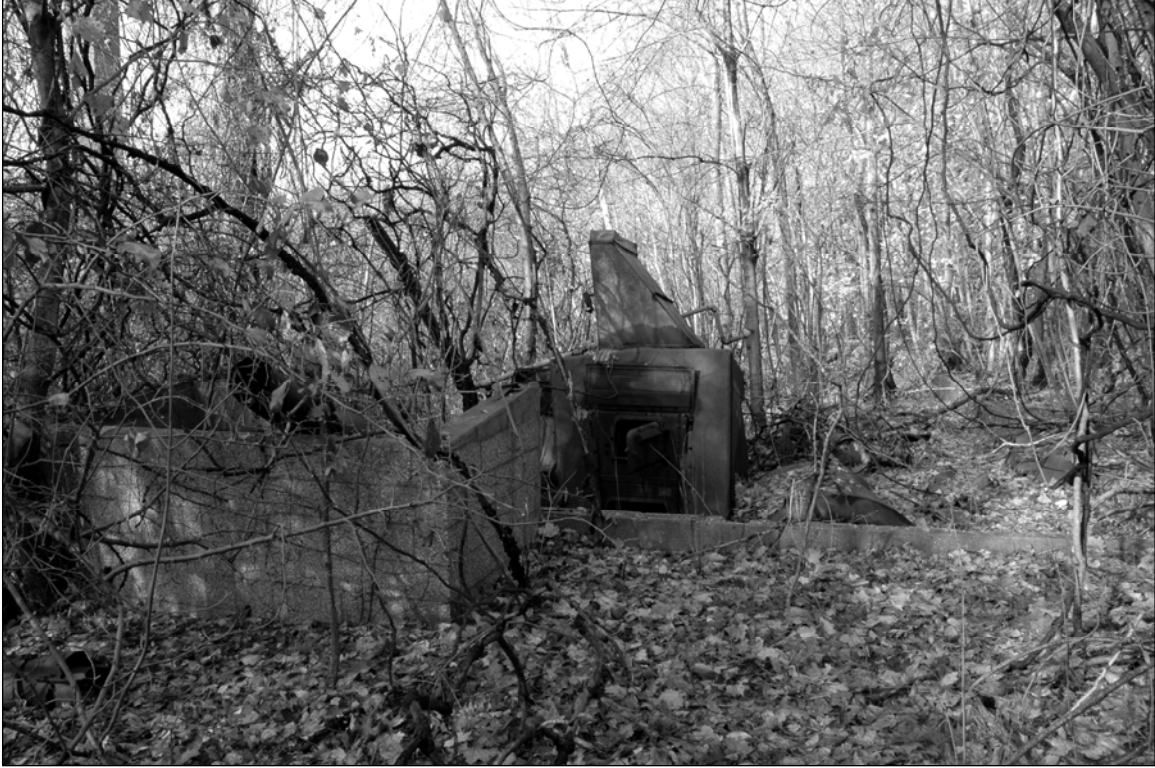
Figure 1. Foundation ruins of Building 133, facing northwest from southeastern end of former building.
