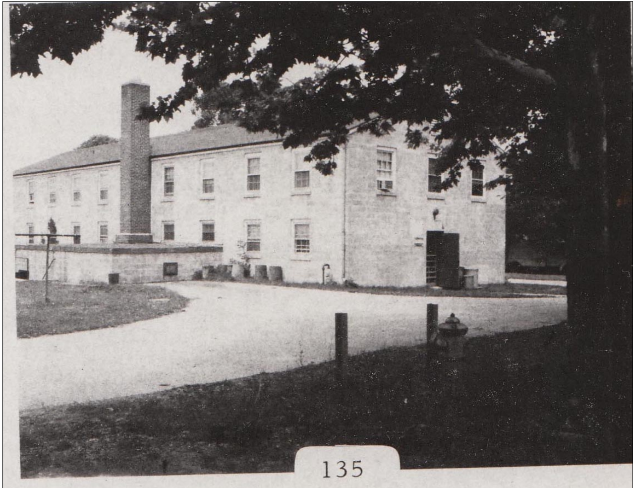
Figure 3. Building 135 in the 1950s. View northwest. Note boiler room on southwestern side of building. Fort Slocum Alumni and Friends Collection, Michael A.Cavanaugh, Los Angeles, CA, custodian.
