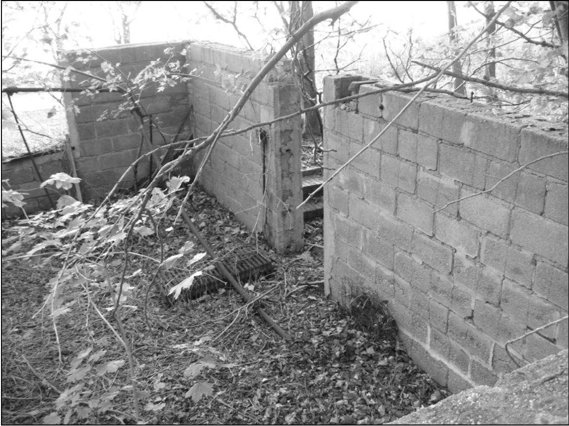
Photo 3. Interior of northwestern end of foundation, facing west.
