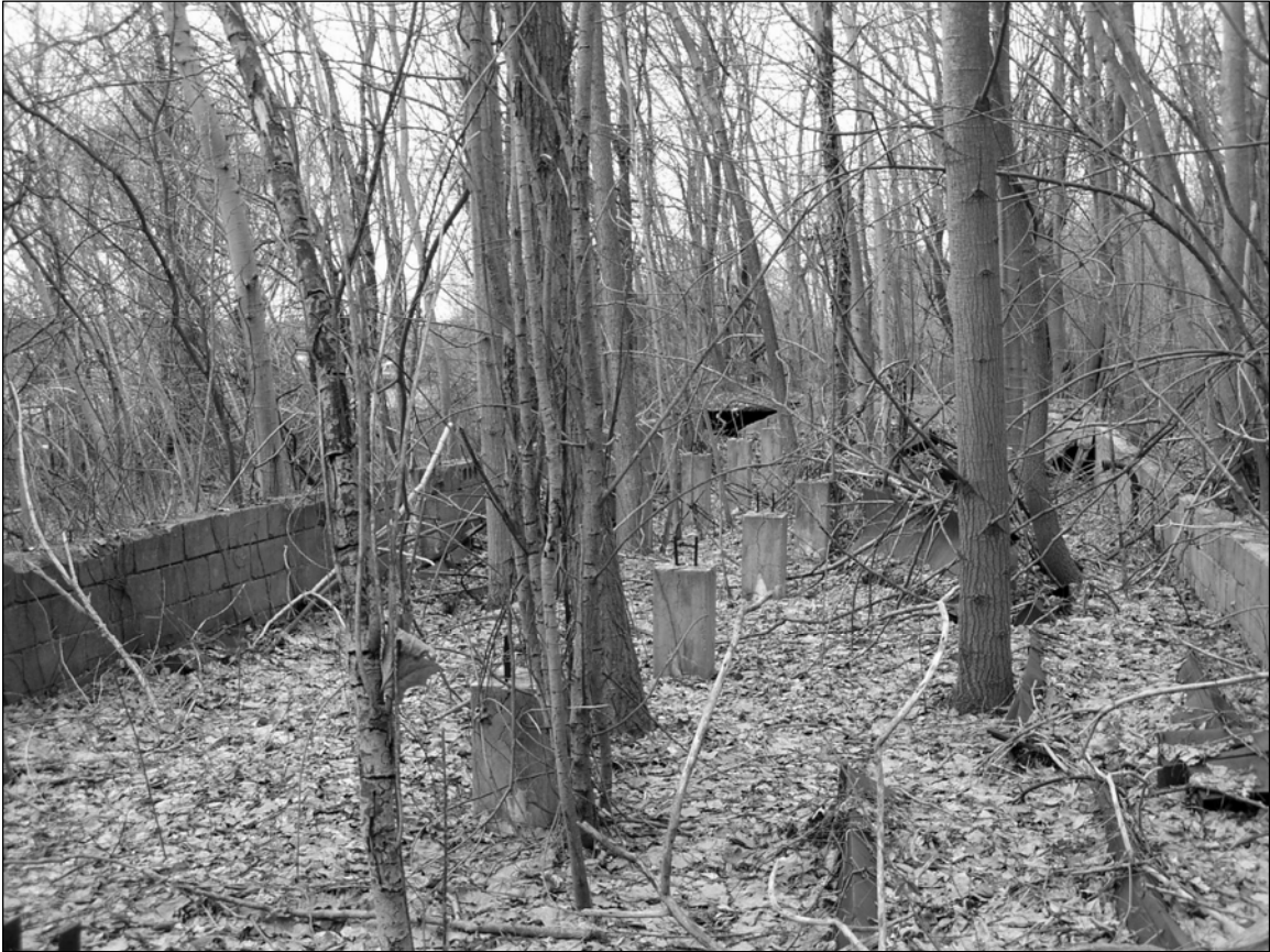
Photo 3. Foundation interior with floor joist supports, facing northwest.
