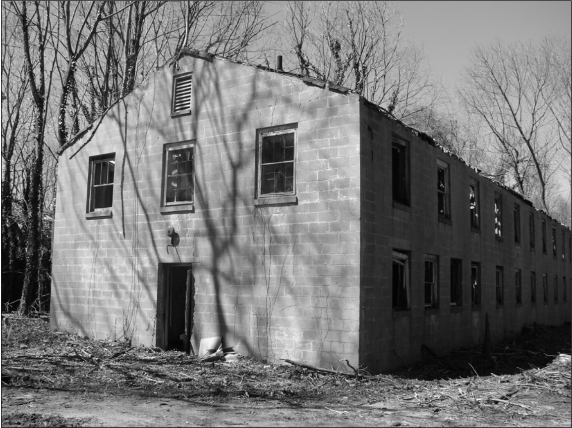
Photo 1. Principal (southeastern) façade, facing west.
