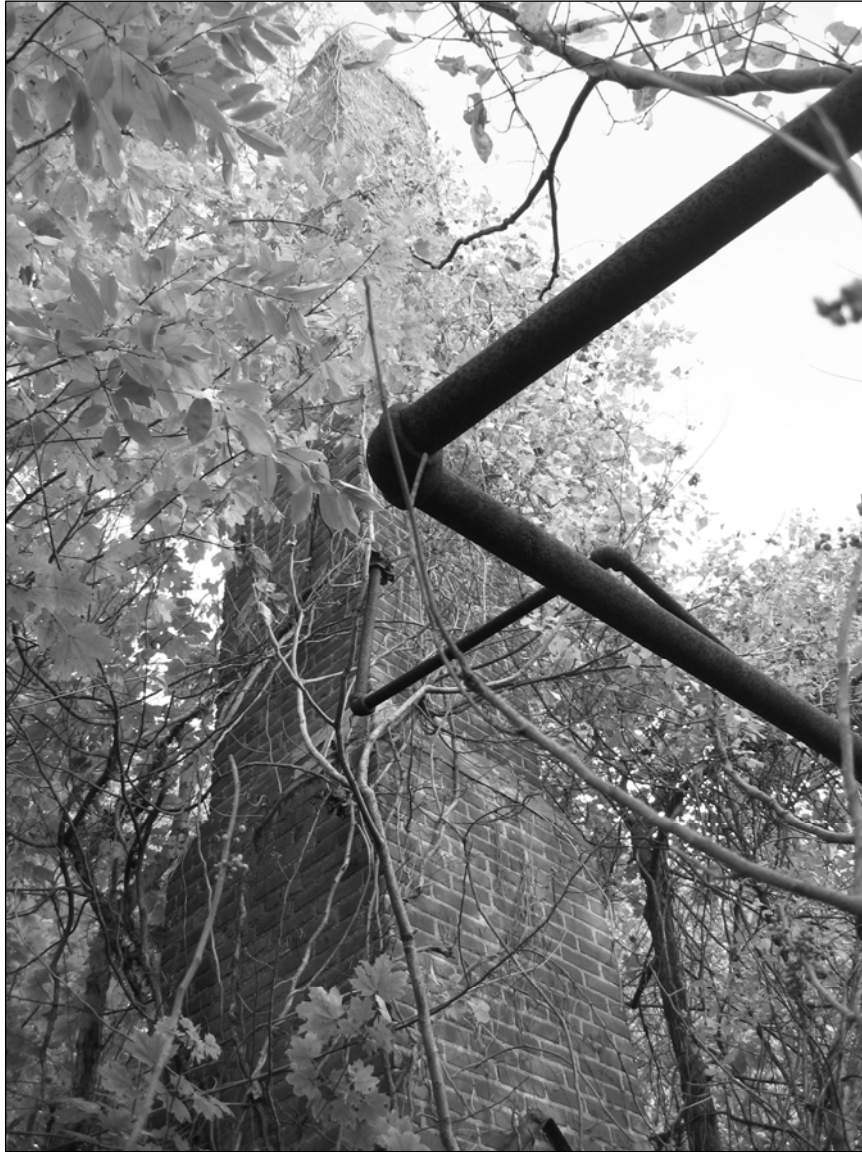
Photo 3. Chimney, facing northwest.
