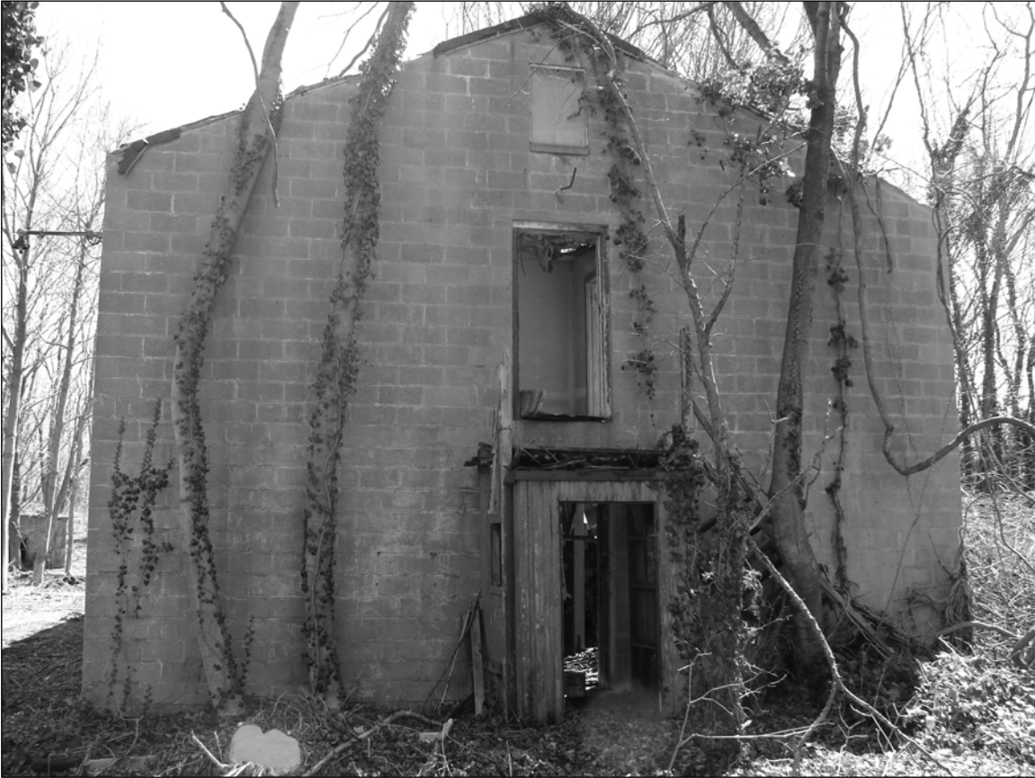
Photo 6. Northwestern façade, facing southeast.
