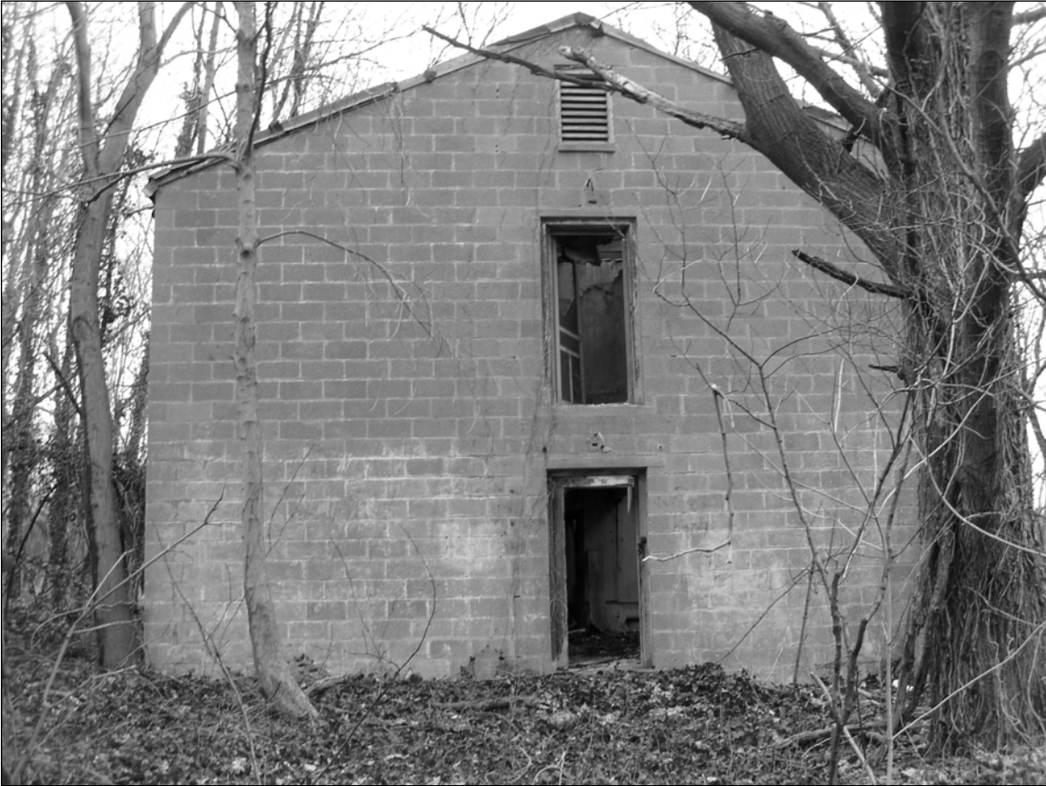
Photo 4. Northwestern façade, facing southeast.
