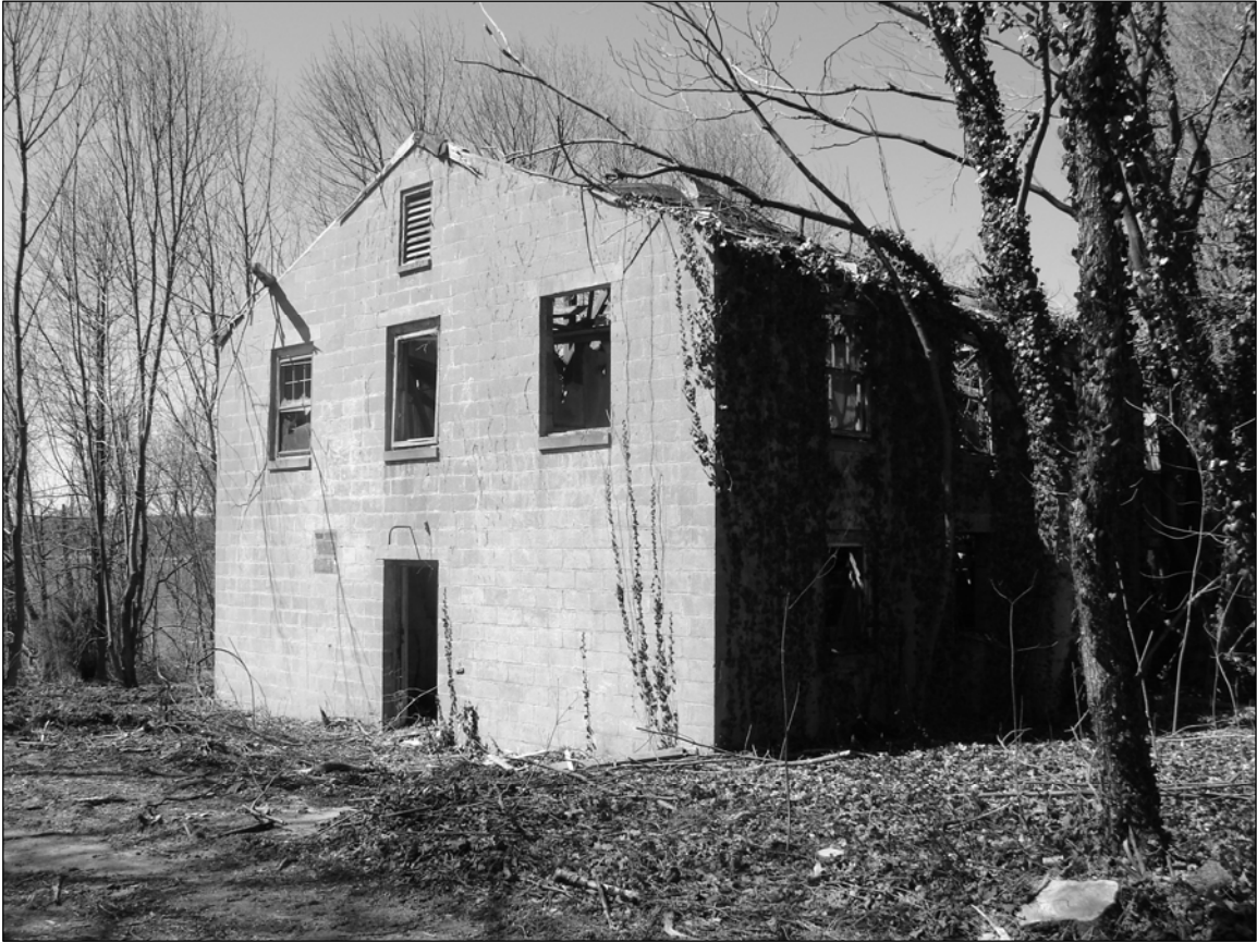
Photo 1. Principal (southeastern) façade, facing west.
