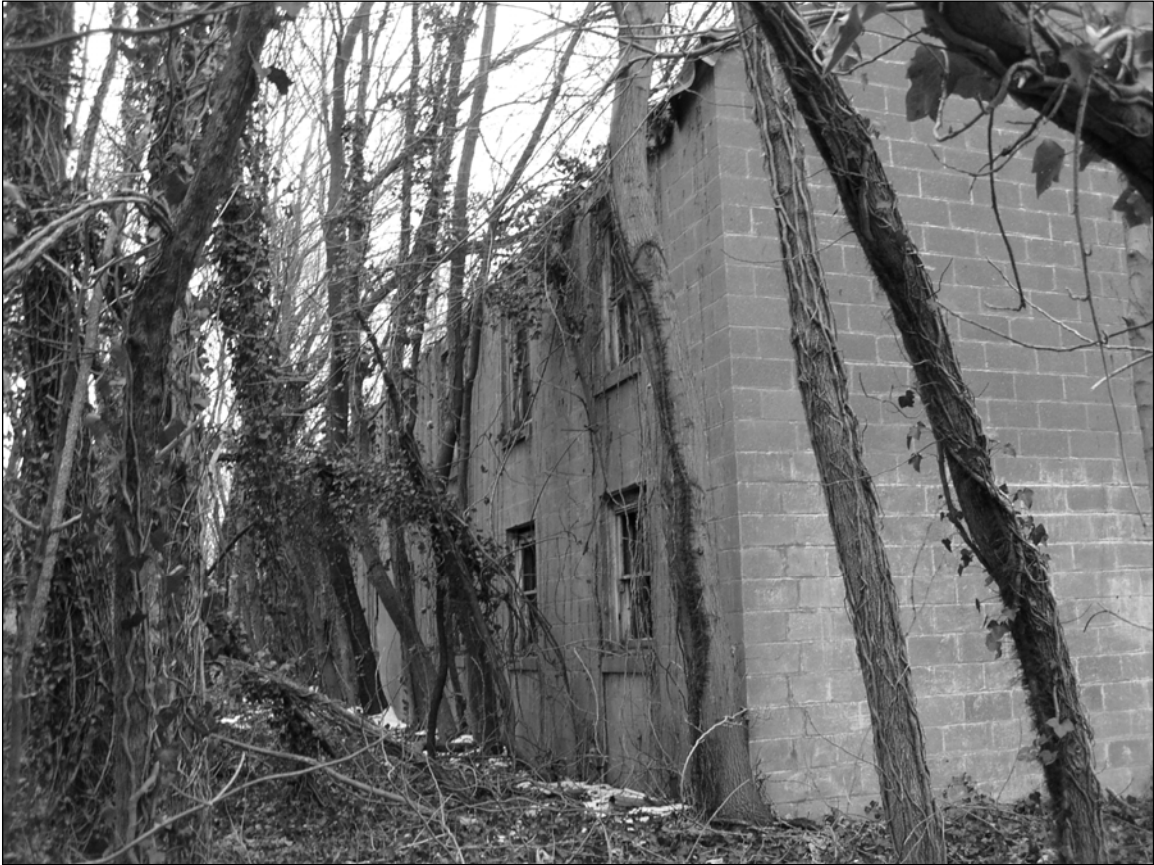
Photo 6. Portion of northwestern end (right) and northeastern side, facing south.
