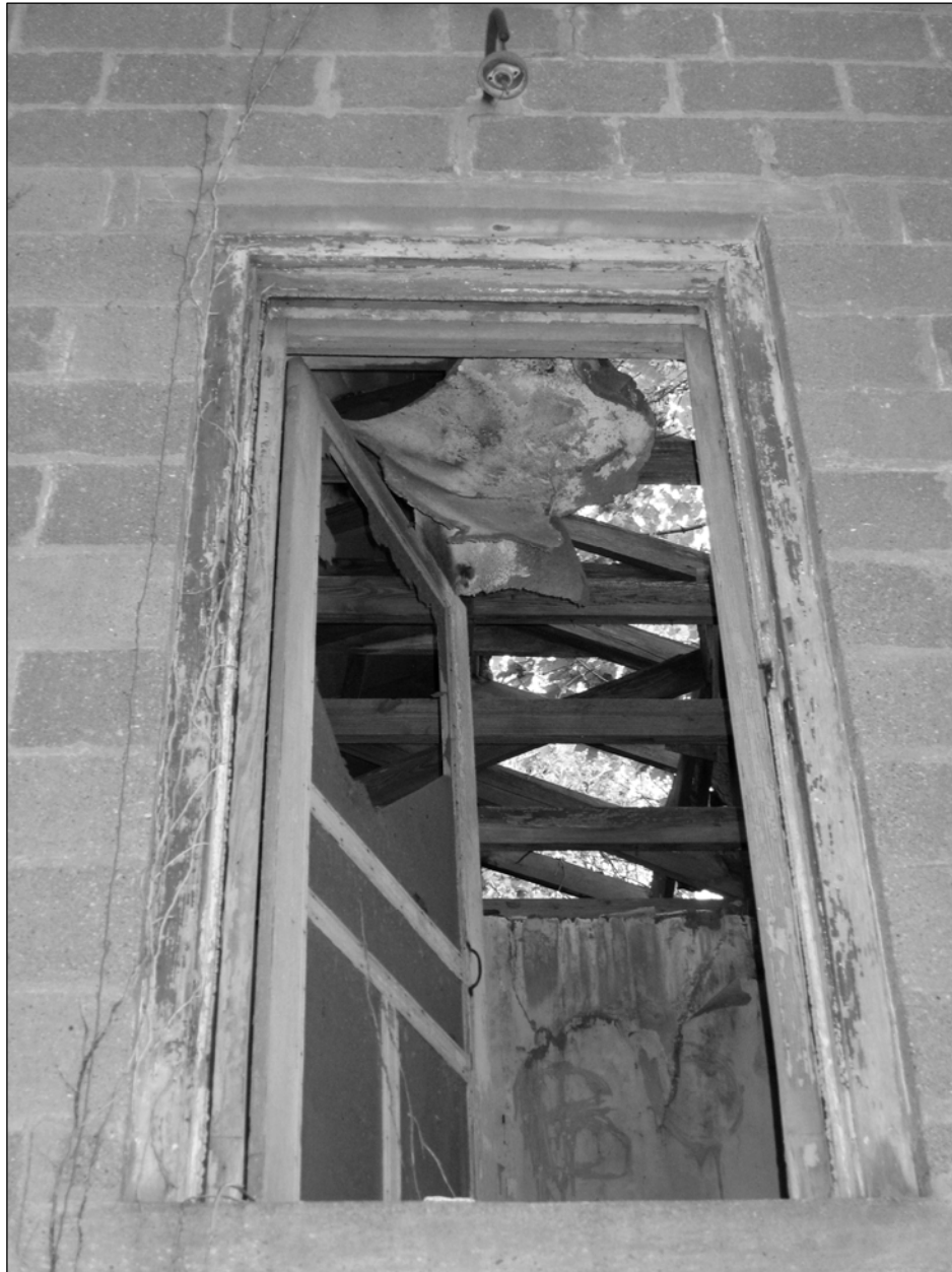
Photo 5. Northwestern façade, detail: second-story door. Facing southeast.
