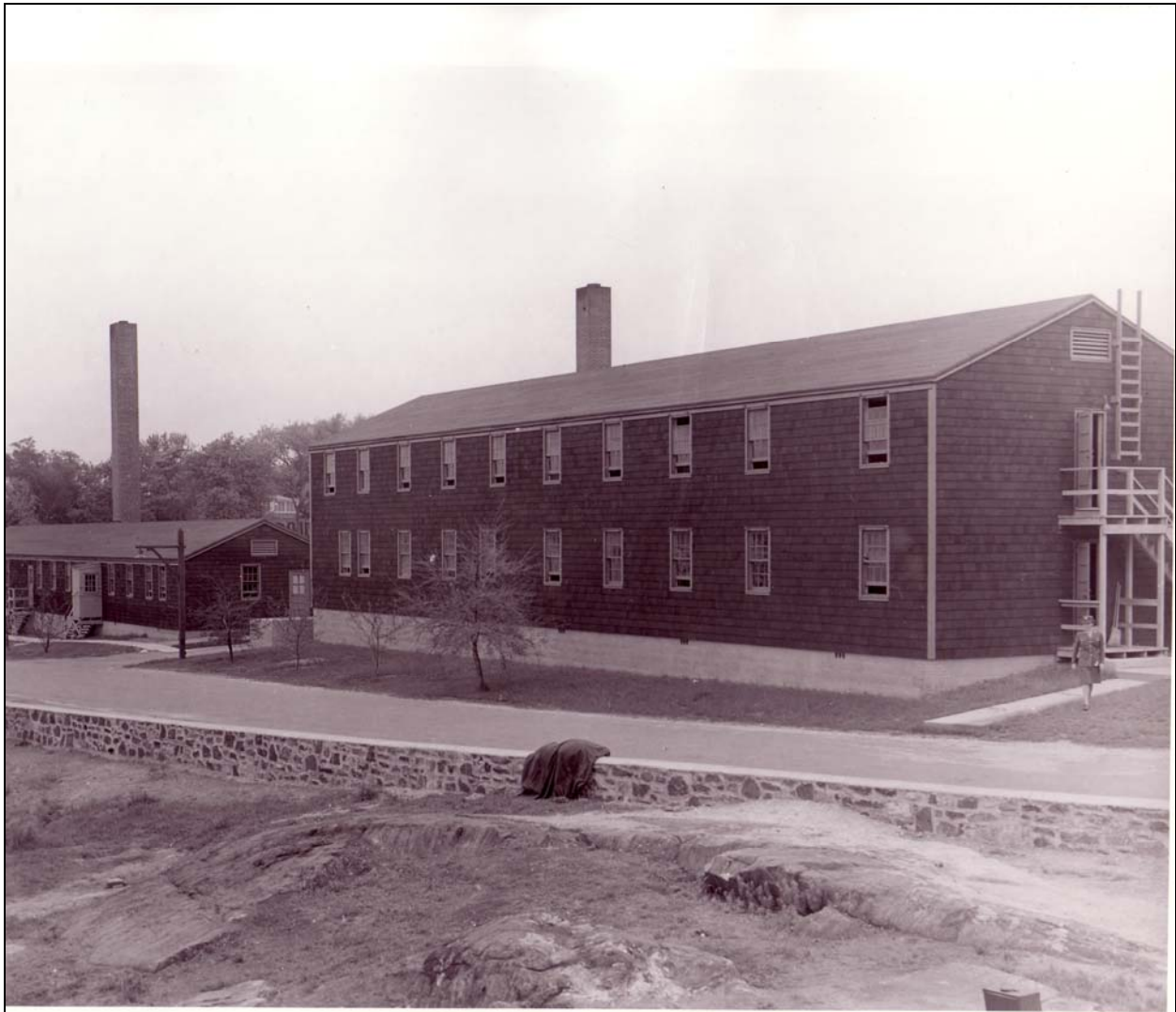
Figure 1. Southern end of WAC area from Parker Road, ca. 1944. View north. WAC Barracks (Building 130) is in the foreground at right. Shown are the back end and southwestern side of the building. Note the exterior wood fire escape stairs leading from the second story. The WAC Recreation and Administration Building (Building 131) is at left. Fort Slocum Collection, New Rochelle Public Library, New Rochelle, NY.
