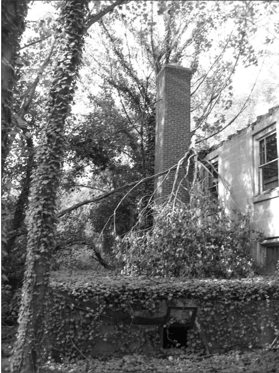
Photo 4. Dependency containing boiler room on southwestern side of building, facing northwest.
