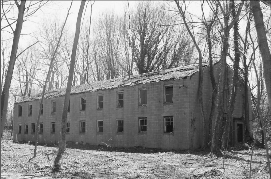
Photo 8. Northwestern and northeastern façades, facing south.
