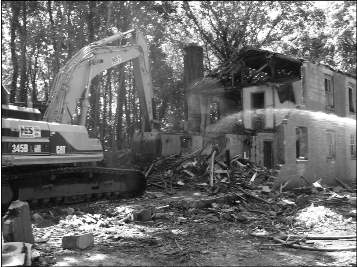
Photo 11. Demolition of Building 135, facing west.
