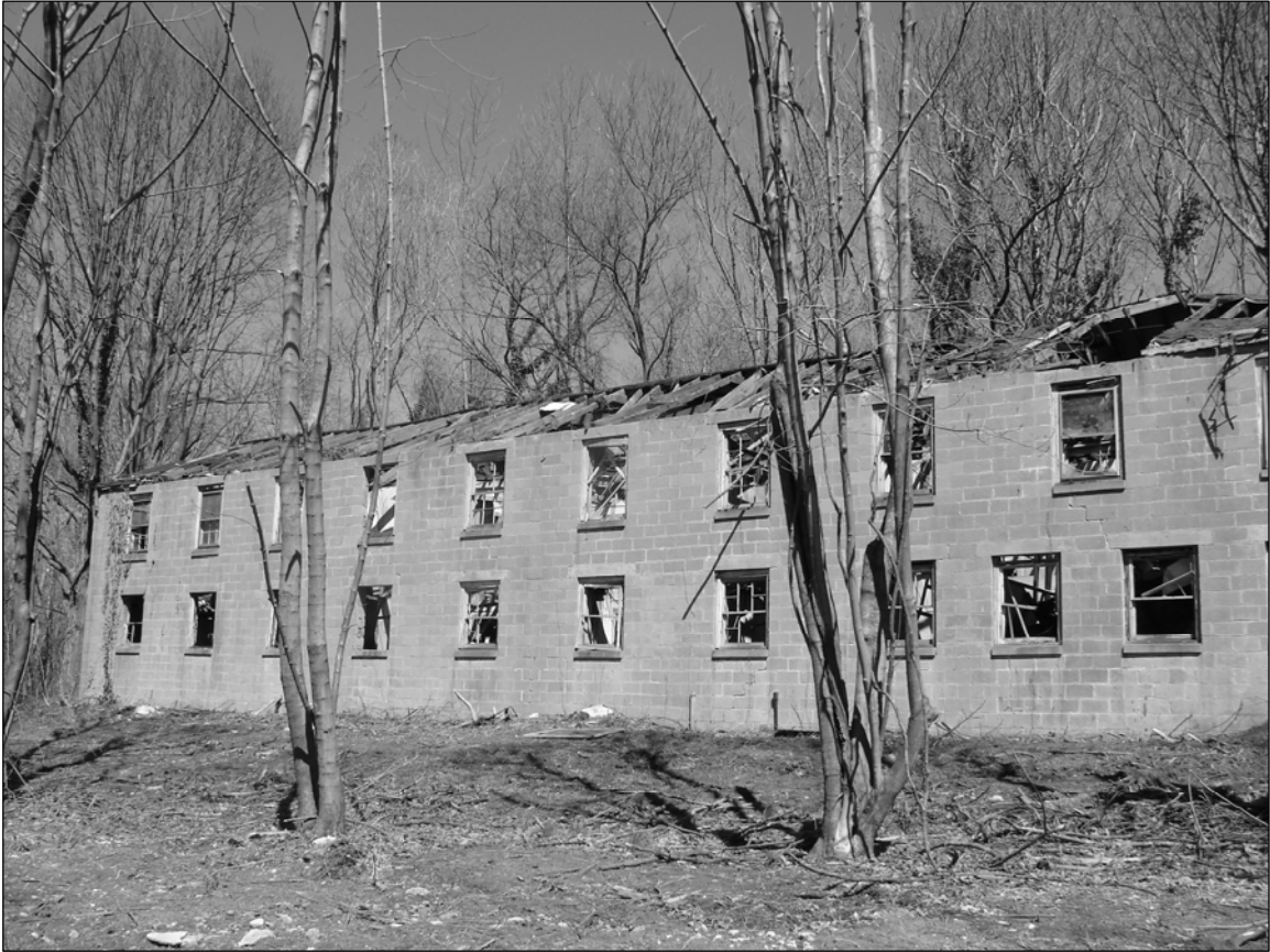
Photo 3. Southwestern side of building, facing north.
