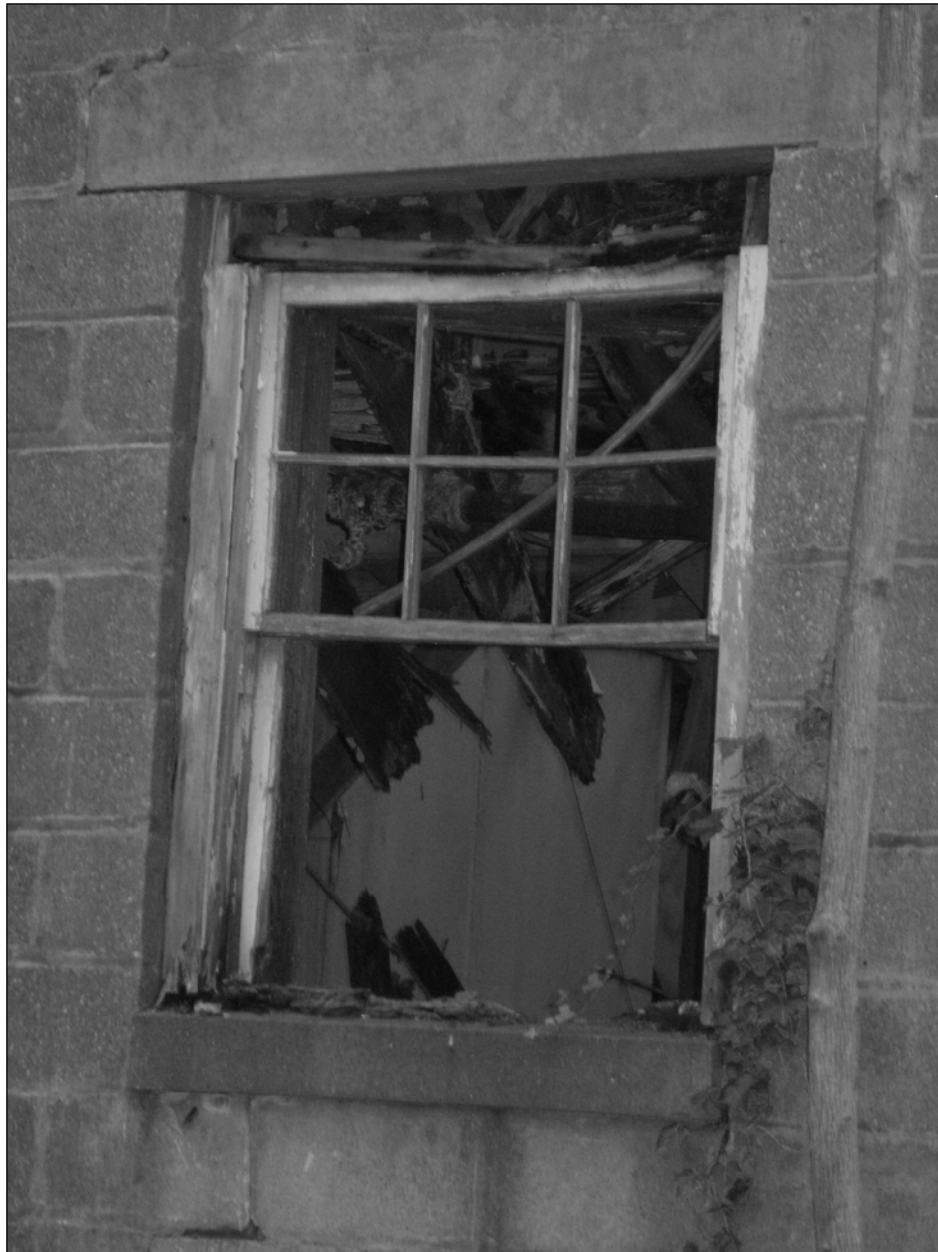
Photo 10. Northeastern façade, detail: partially intact typical six-over-six double-hung wood sash window.
