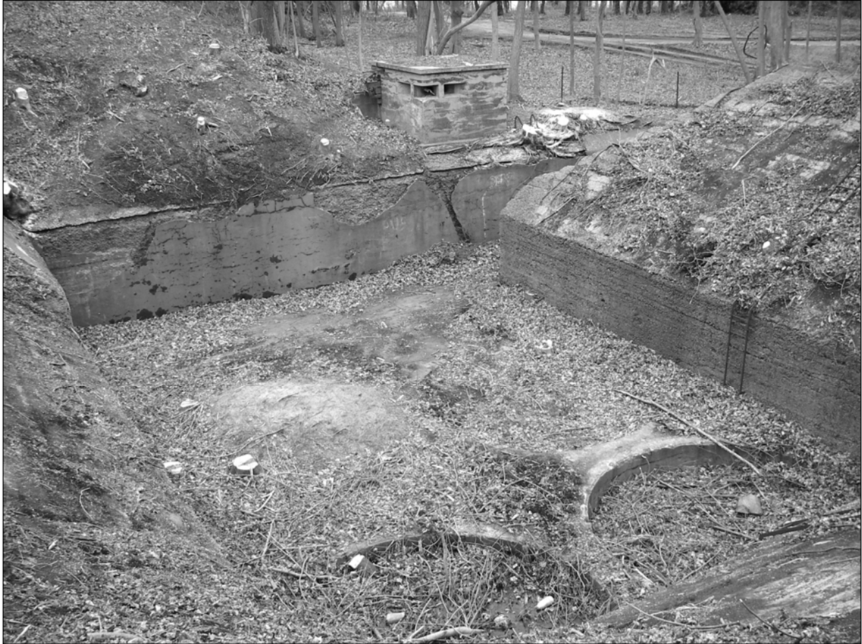
Photo 3. Battery Overton Pit B after removal of opportunistic growth of trees from walls and floor of pit in fall 2008, facing southwest. Mortar Battery Data Booth (Building 128A) at center of photograph. Mortar Battery Powerhouse, which formerly stood behind the data booth, had been removed by the time of the photograph.
