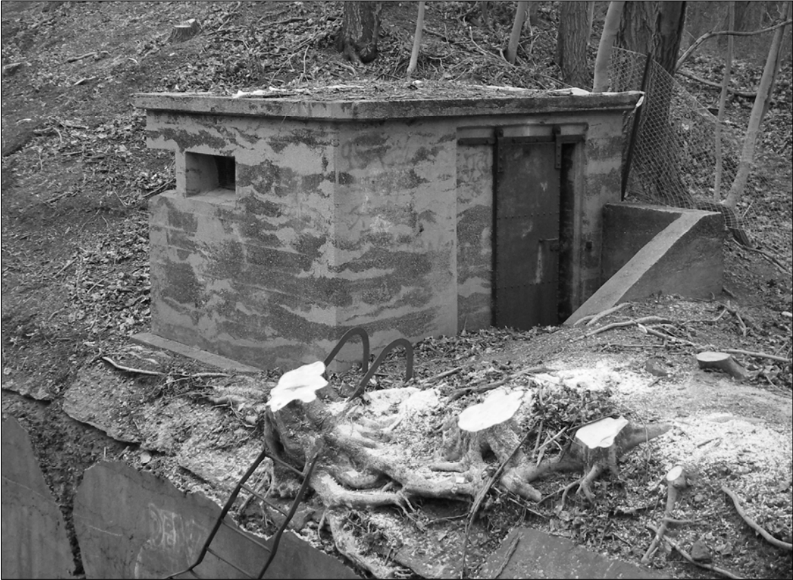
Photo 4. Northern and western façades, facing southeast.
