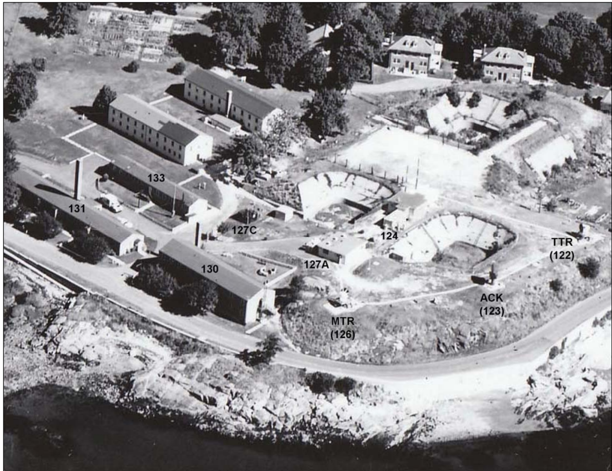
Figure 2. High angle oblique aerial photograph of Davids Island, ca. 1958, detail. View north. Labels have been added to this version of the image to indicate buildings and structures included in the Nike Battery NY-15 IFC Area. The battery's three radar sets are visible in this image and are labeled as follows: MTR—missile tracking radar; ACK—target acquisition radar; and TTR—target tracking radar. Building 127C is at center left. Original from Record Group 291, National Archives, New York, NY; digital copy from Fort Slocum Alumni and Friends Collection, Michael A. Cavanaugh, Los Angeles, CA, custodian.
