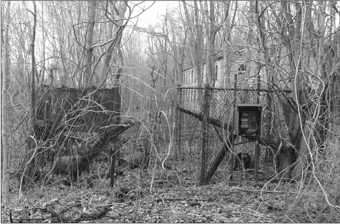
Photo 4. Southeastern side of transformer vault enclosure, with Building 134 in background, facing northwest.
