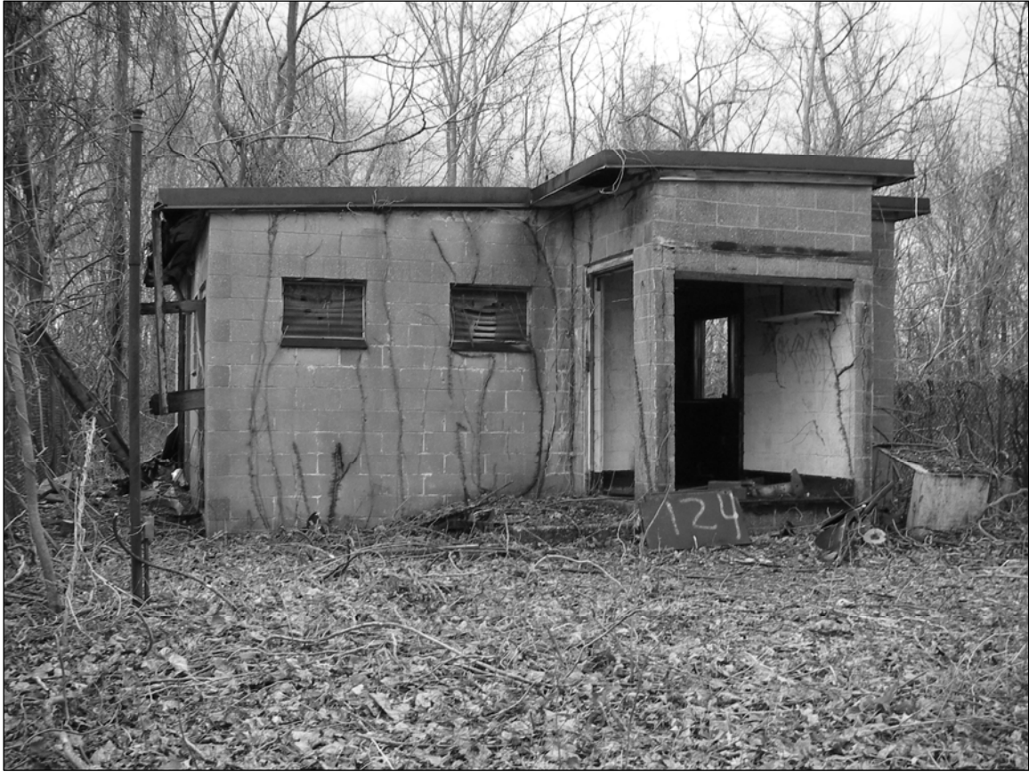
Photo 1. Southwestern façade, facing northeast.
