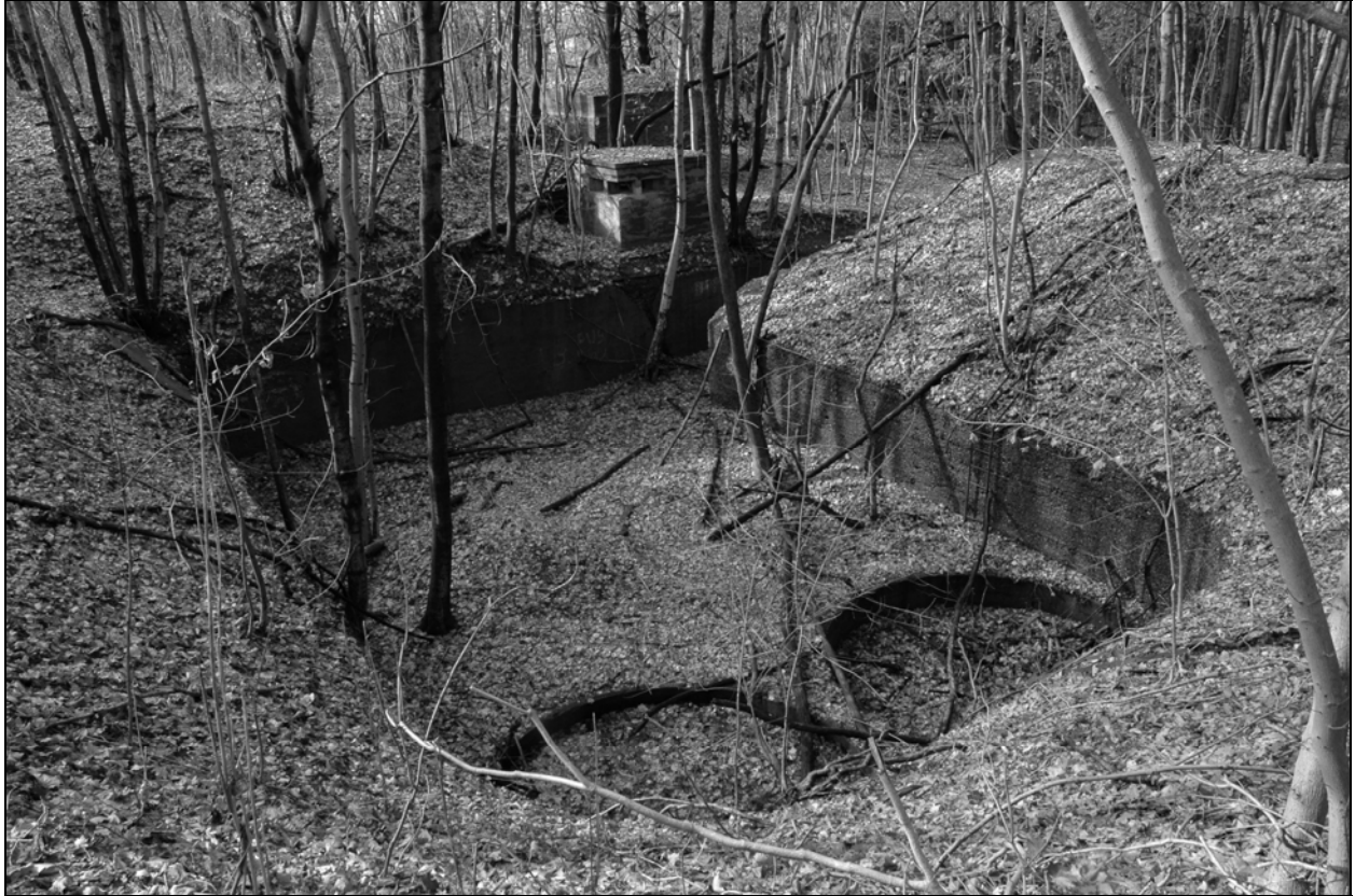
Photo 1. Battery Overton Pit B (Building 127), showing northeastern (left) and northwestern (right) gun emplacements, facing southwest. The Mortar Battery Data Booth (Building 128A) and Mortar Battery Powerhouse (Building 128) are at center rear. The walls and floor of the pit are covered by leaf litter and trees that began growing on the feature opportunistically after maintenance of it ceased.
