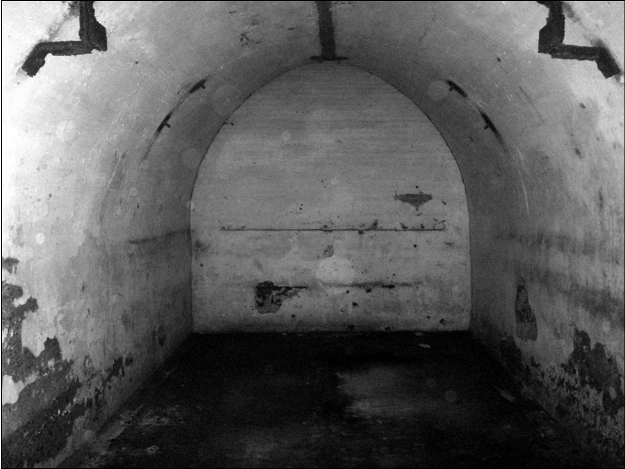
Photo 11. Storage Bay at north end of Main Tunnel, facing north-northeast.
