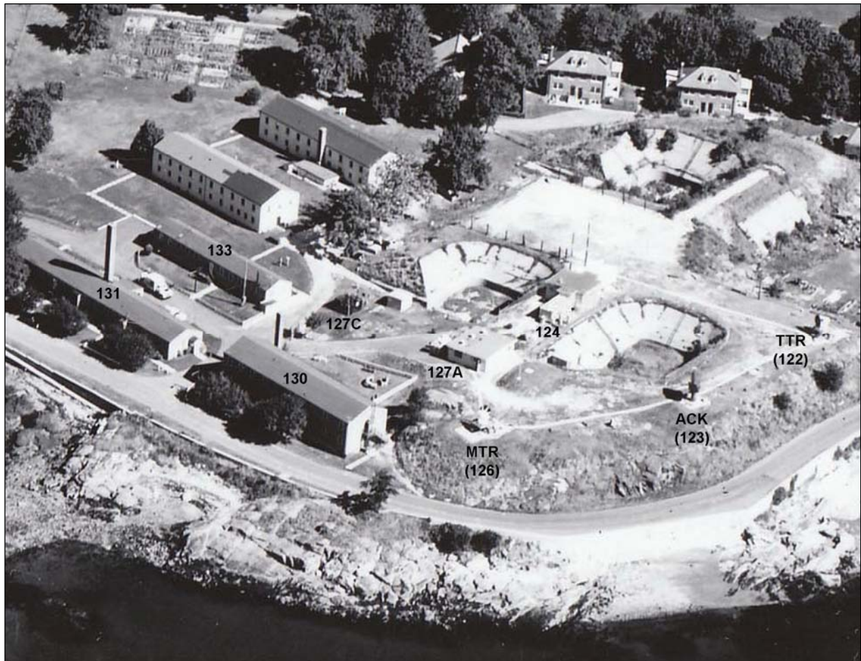
Figure 1. High angle oblique aerial photograph of Davids Island, ca. 1958, detail. View north. Labels have been added to this version of the image to indicate buildings and structures included in the Nike Battery NY-15 IFC Area. The battery's three radar sets are visible in this image and are labeled as follows: MTR—missile tracking radar; ACK—target acquisition radar; and TTR—target tracking radar. Building 127A is near the center of the image. Original from Record Group 291, National Archives, New York, NY; digital copy from Fort Slocum Alumni and Friends Collection, Michael A. Cavanaugh, Los Angeles, CA, custodian.
