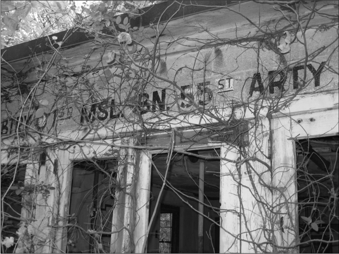
Photo 2. Southwestern façade, detail of sign showing unit assigned to battery, facing north.
