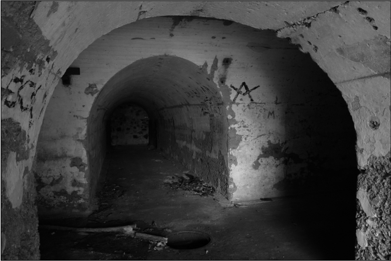
Photo 10. Overton Lateral Tunnel, at junction of Main Tunnel, facing east-southeast toward blocked-off entrance to the now-demolished Battery Overton Pit A.
