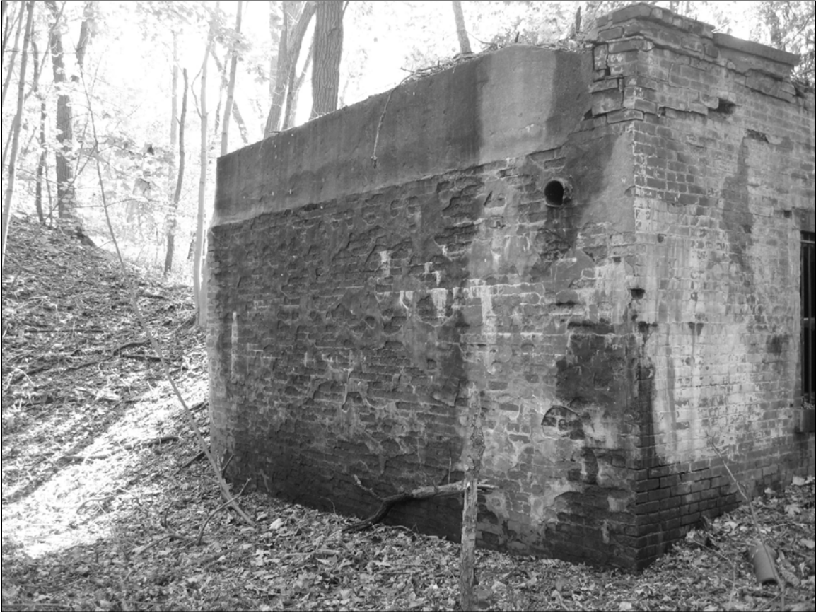
Photo 4. Northern façade, facing south.
