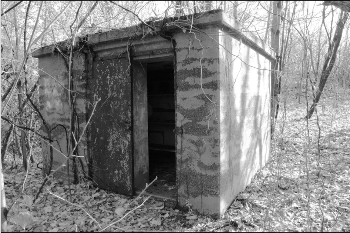
Photo 1. Western and southern façades, facing northeast.
