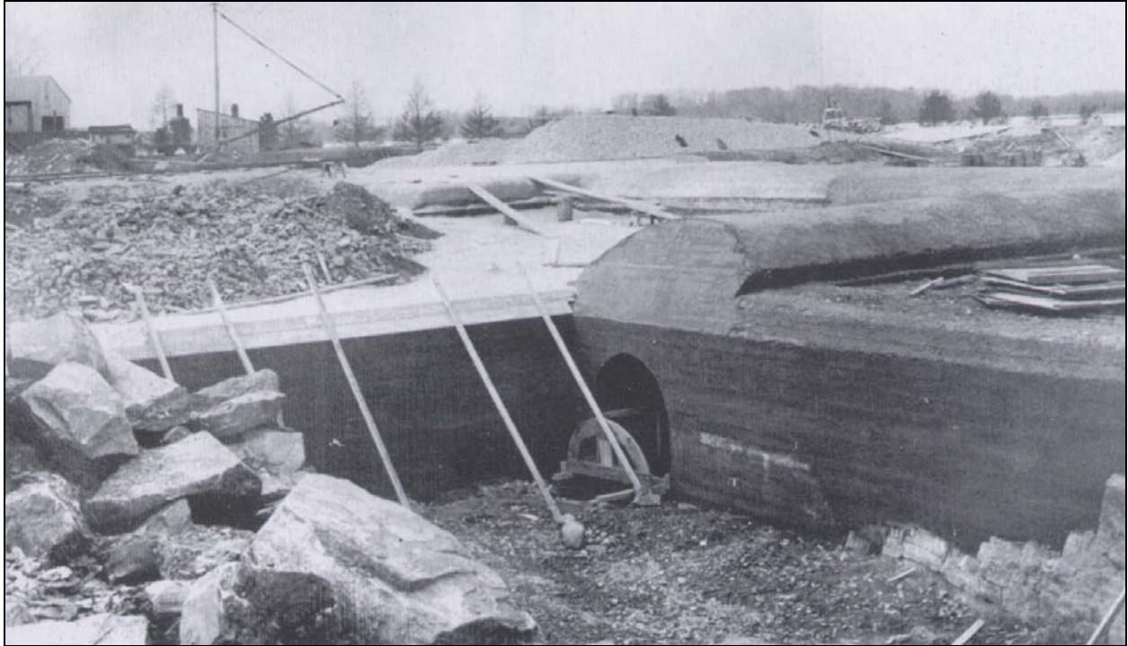
Figure 9. Typical cut-and-cover construction of a mortar battery in the 1890s, unknown location. From Polaski and Williford (2003: 87).
