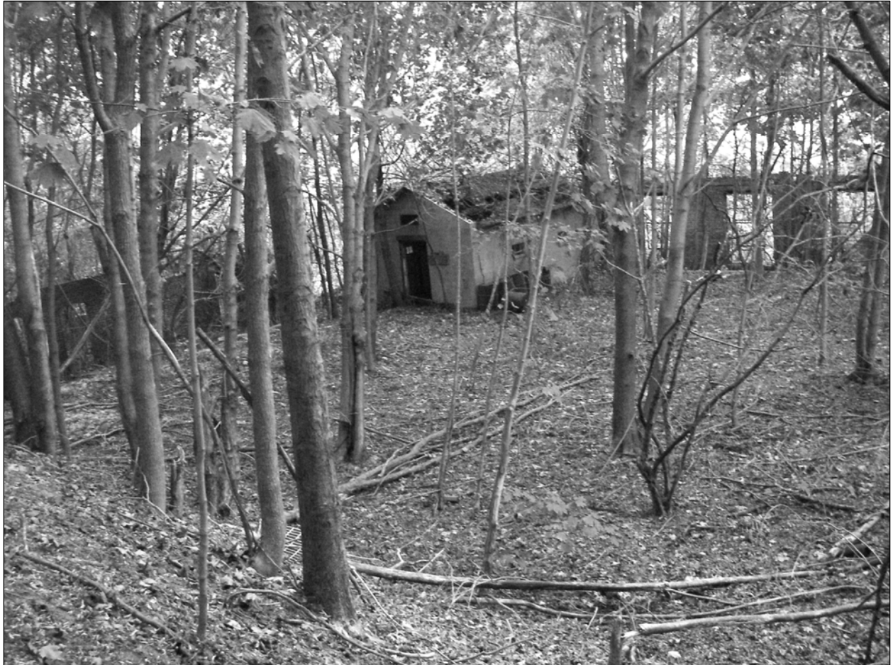
Figure 8. Northern end of Pistol Range constructed at the former location of Battery Overton Pit A, facing east-northeast from western wall of former mortar pit. Small structure in center is the Pistol Range Storehouse (Building T-111). Portions of the west (left) and south (right) wings of the Ordnance Storehouse/Laundry (Building 110) stand behind Building T-111 beyond the edge of the Pistol Range. The area is covered by trees that began growing on the feature opportunistically after maintenance of it ceased.
