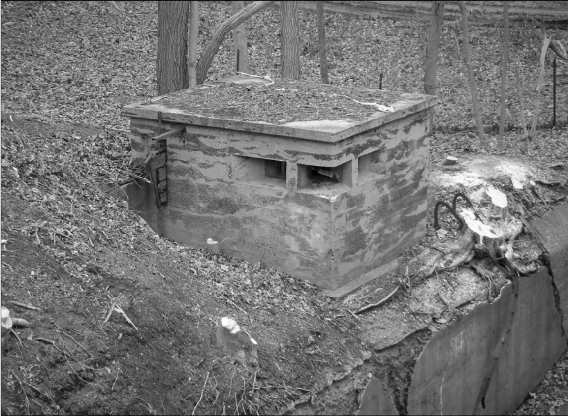
Photo 5. Northern and eastern façades, facing southwest.
