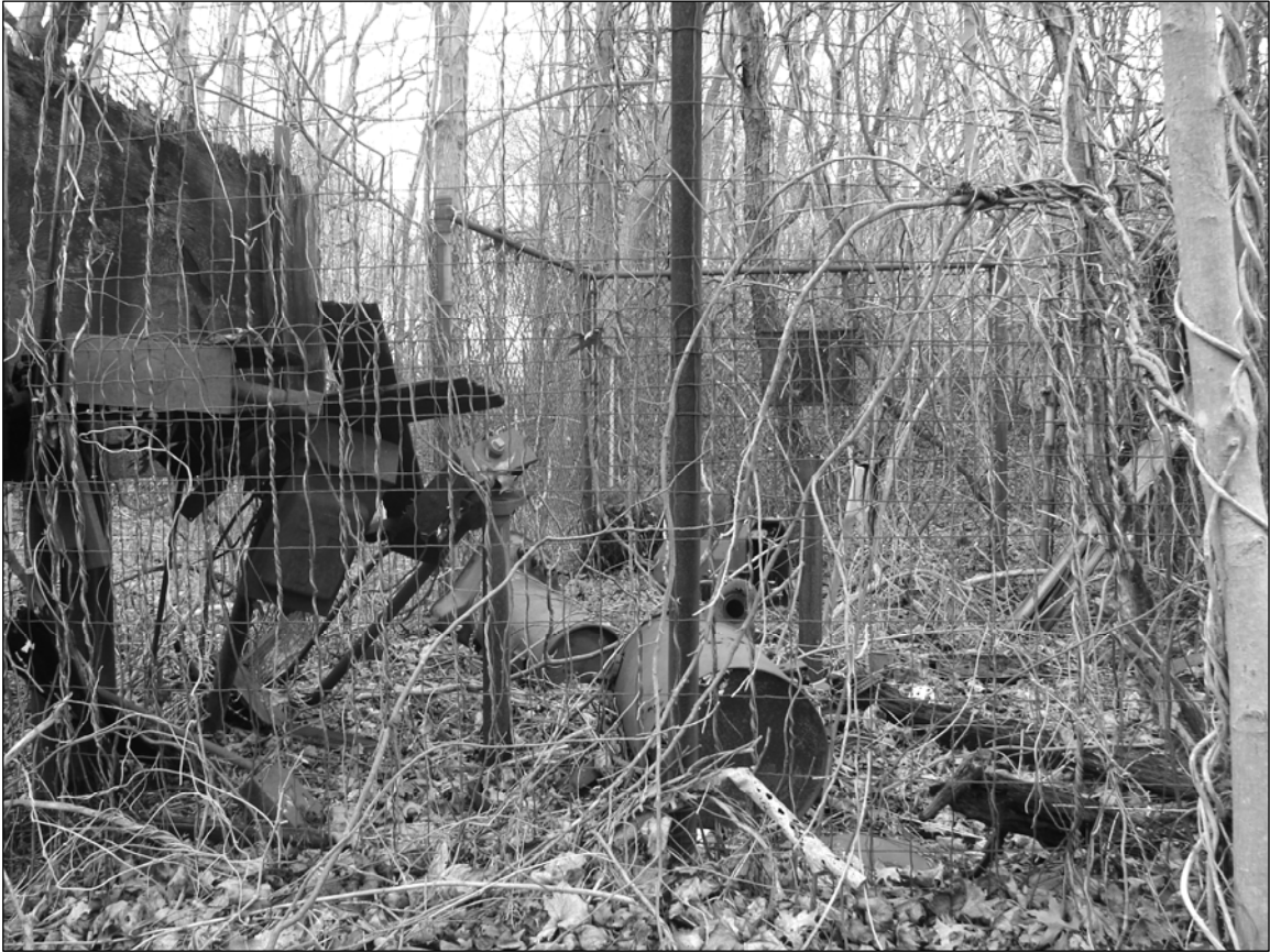
Photo 5. Interior of transformer enclosure, facing northeast.
