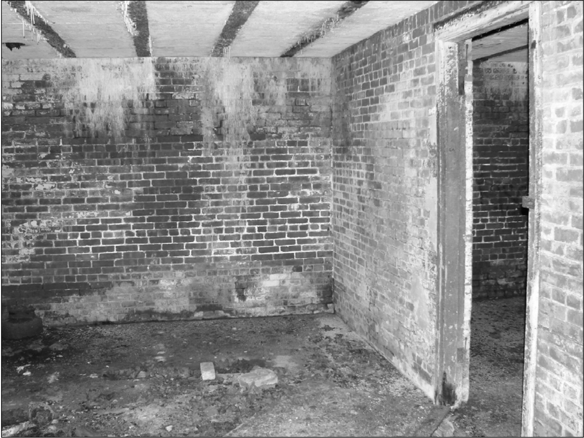
Photo 5. Interior, showing main room and room partition wall, facing southeast.
