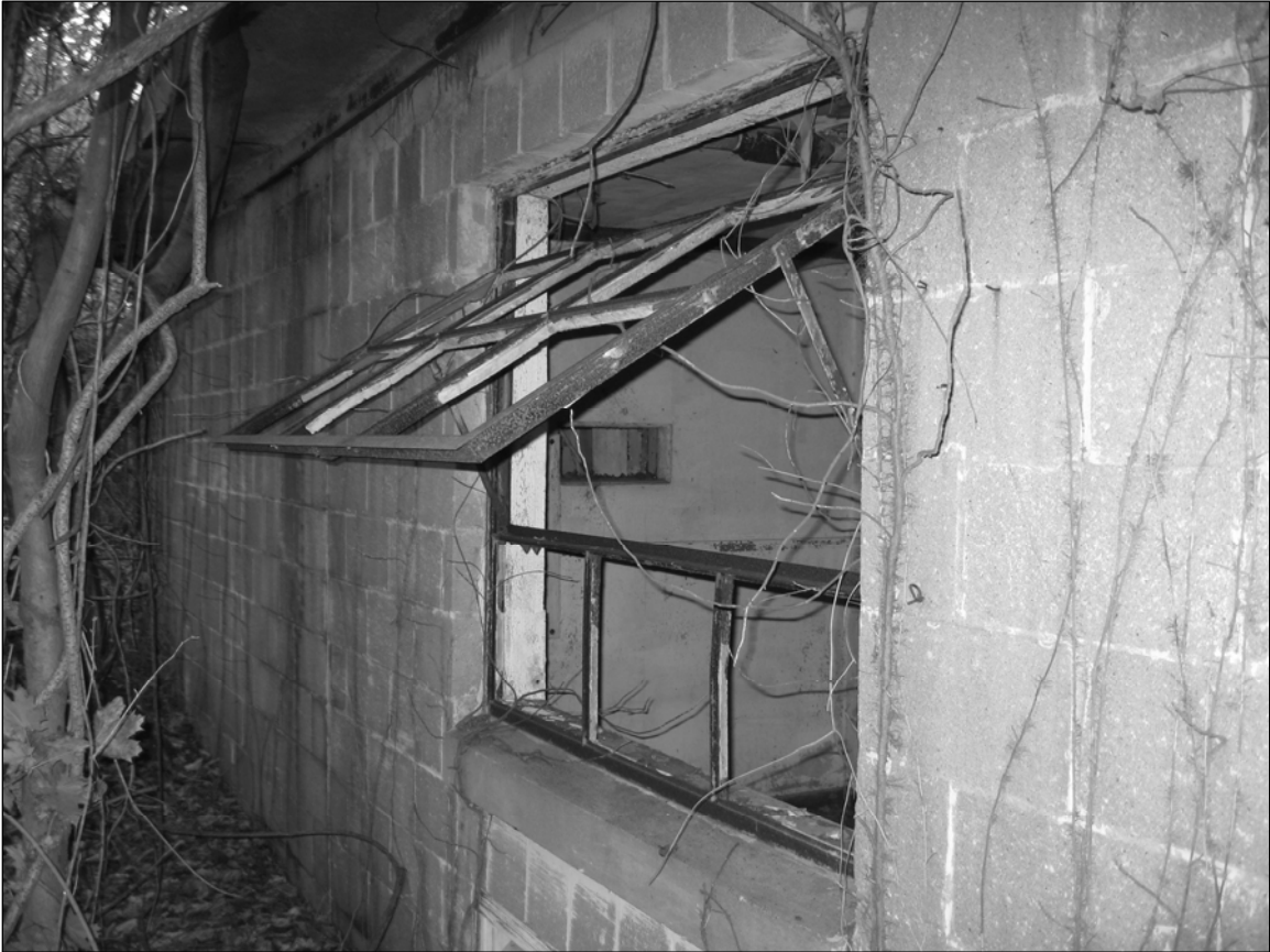
Photo 3. Northwestern façade, facing northeast.
