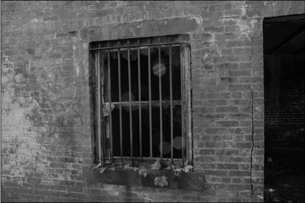
Photo 3. Western façade, detail: window to left of door, facing southeast.
