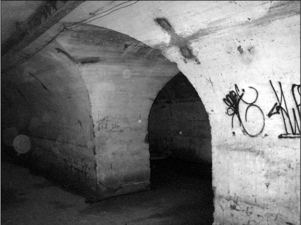
Photo 12. Junction of Main Tunnel and West Entrance Bay, facing southwest.
