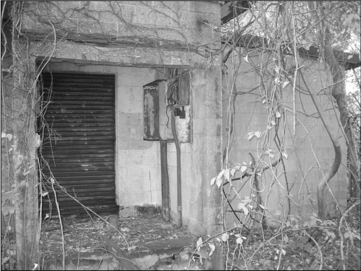
Photo 3. Western portion of northeastern façade, including docking bay or porch, facing southwest.
