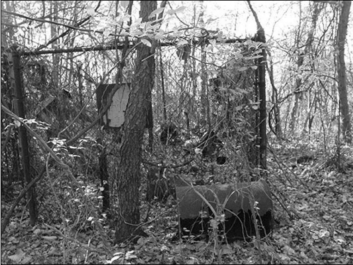
Photo 1. Northeastern side of transformer vault enclosure, facing southwest.
