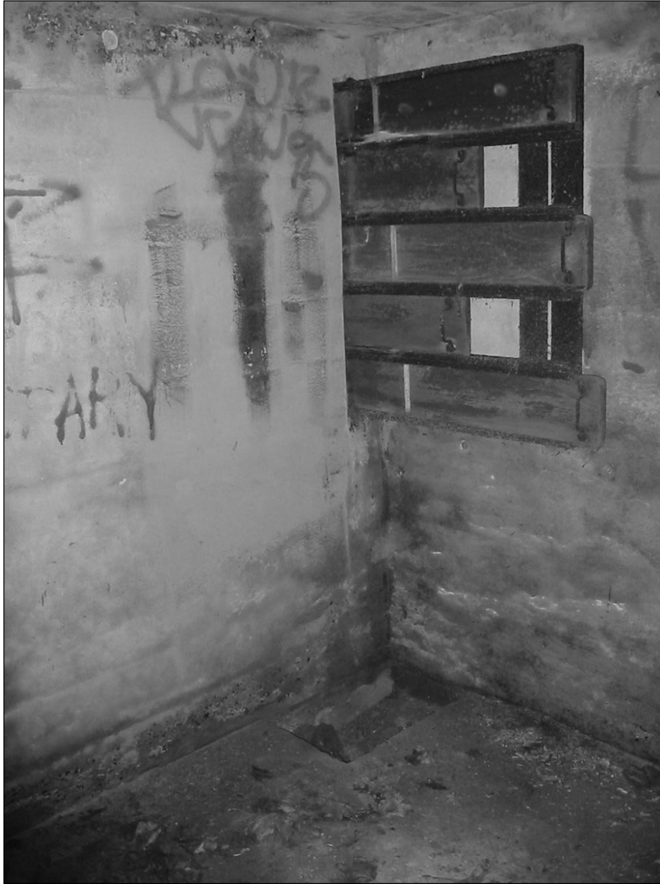
Photo 8. Interior, detail: sliding blackboard frame in southeastern corner, facing east.
