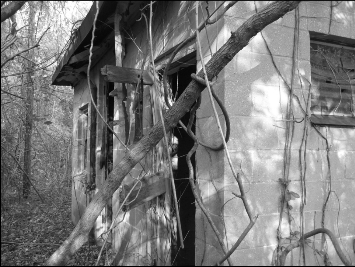
Photo 2. Northwestern façade, facing northeast.
