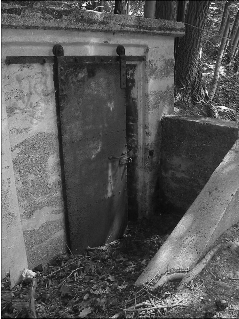
Photo 6. Western façade, detail: entrance and hollow steel door, facing southeast.
