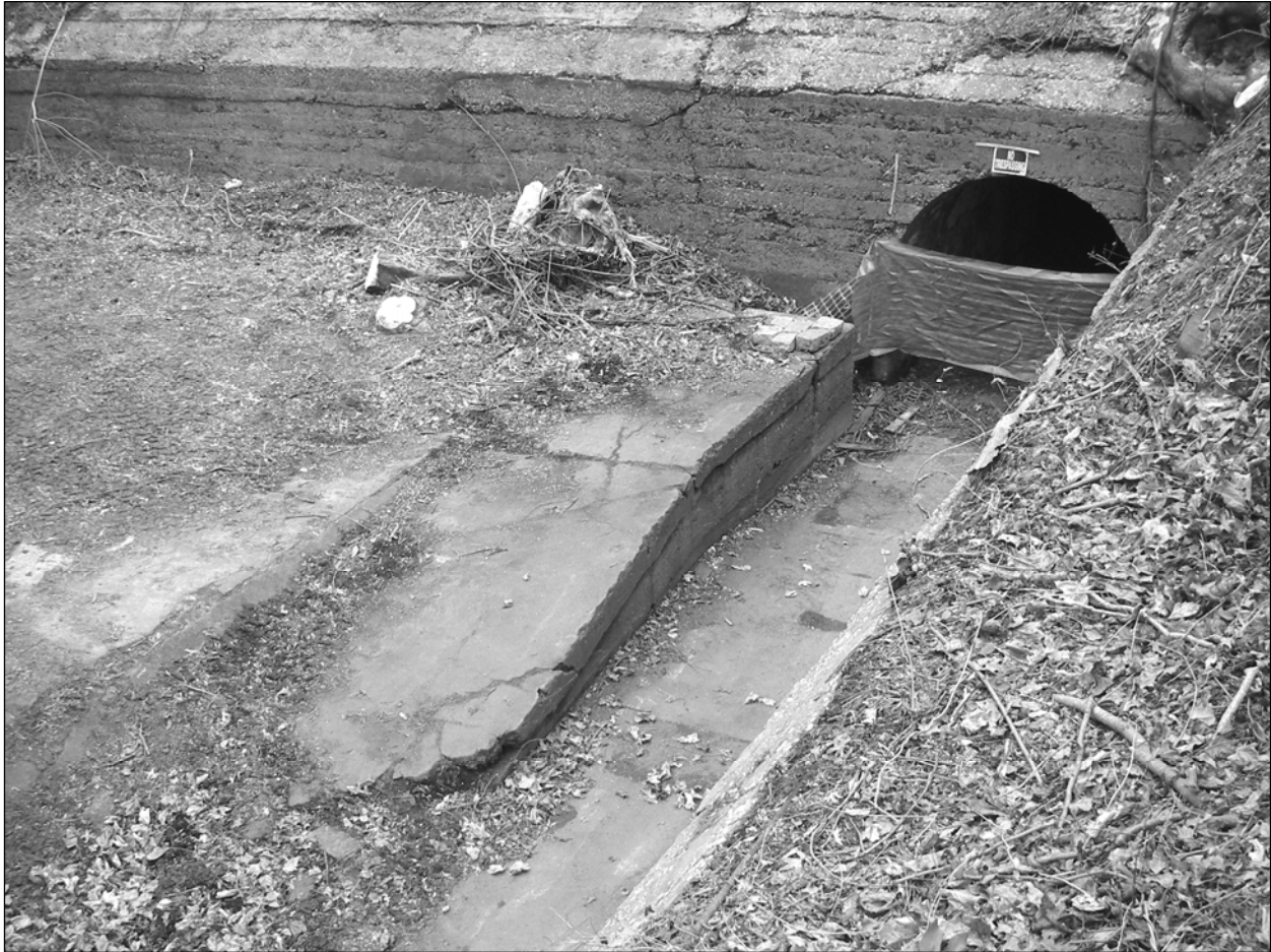
Photo 6. Southern end of Battery Haskin Pit B after removal of opportunistic growth of trees from pit walls and floor in fall 2008, facing east. Ramp to left climbs to level of mortar emplacements, while that to right slopes into the Haskin Lateral Tunnel.
