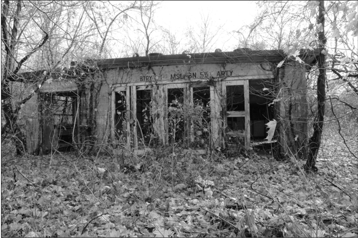
Photo 1. Southwestern façade, facing northeast.
