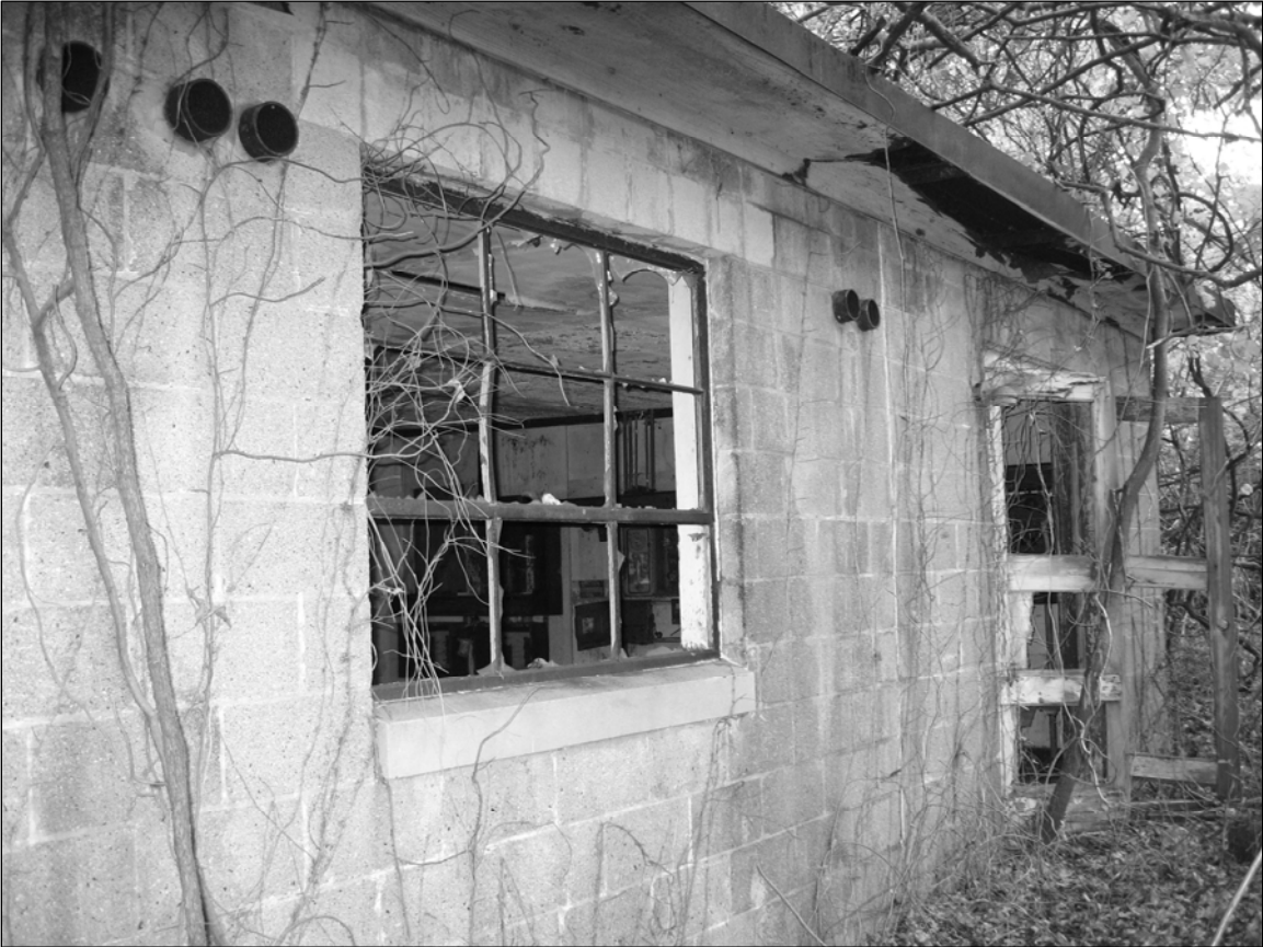
Photo 4. Southeastern façade, facing north.
