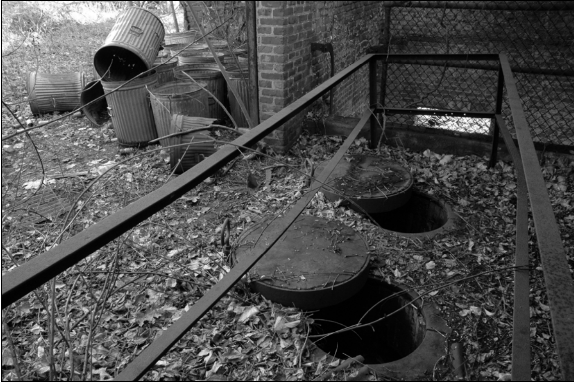
Photo 3. Charging deck, detail showing two of three charging holes, facing southeast.
