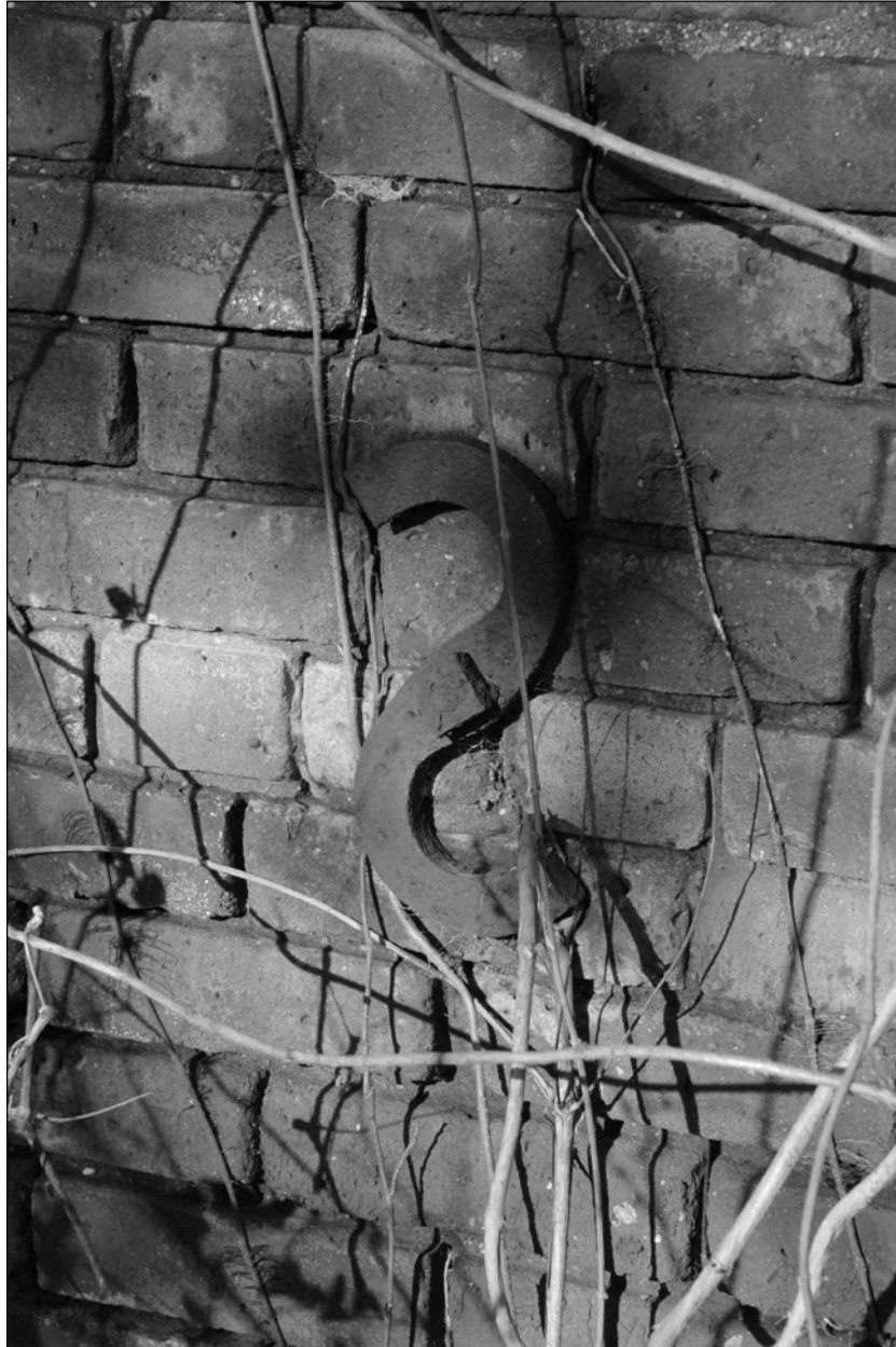
Photo 2. Southern façade, detail of S-shaped tie-rod anchor.
