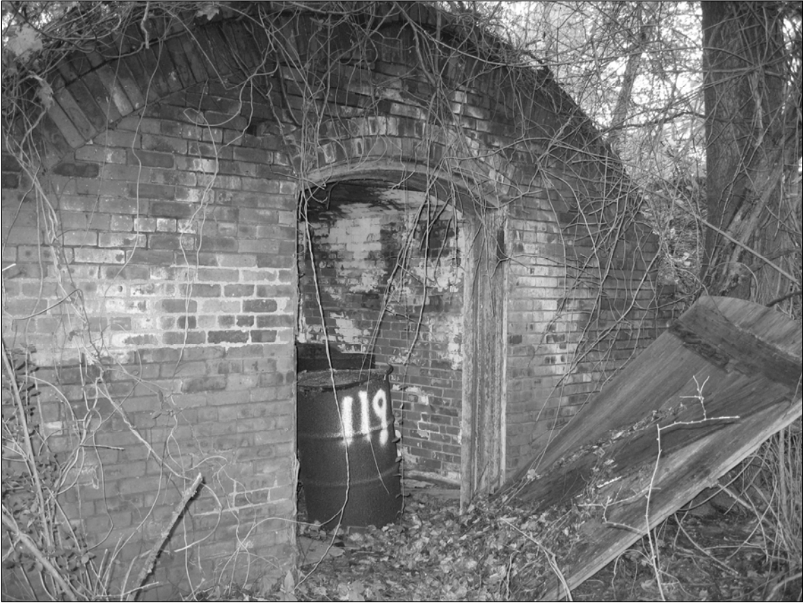
Photo 3. Southern façade, showing entrance and view into interior, facing southeast.
