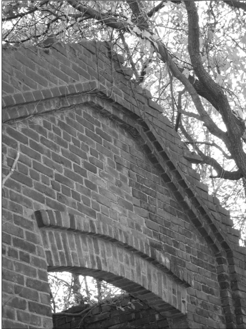
Photo 3. Northern façade, details of brickwork and segmental arch door opening, facing southwest.
