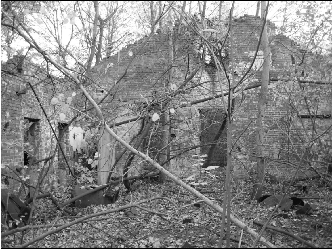
Photo 8. North wing, interior facing east toward original gable end.
