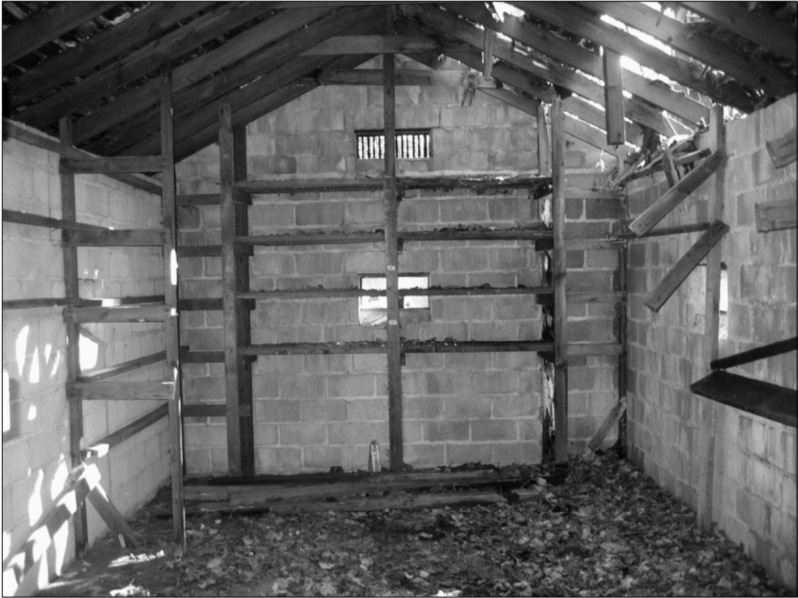
Photo 6. Interior, facing east.
