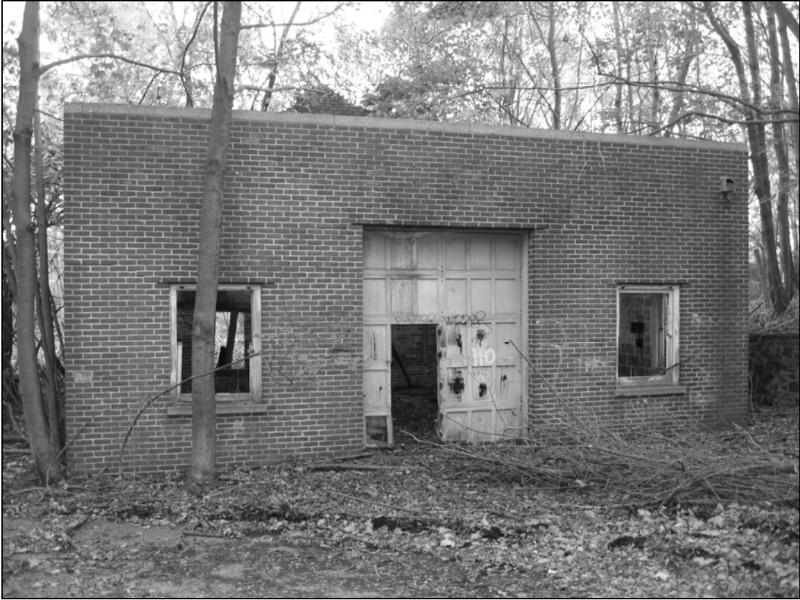
Photo 3. North wing, western façade of one-story addition, facing east.
