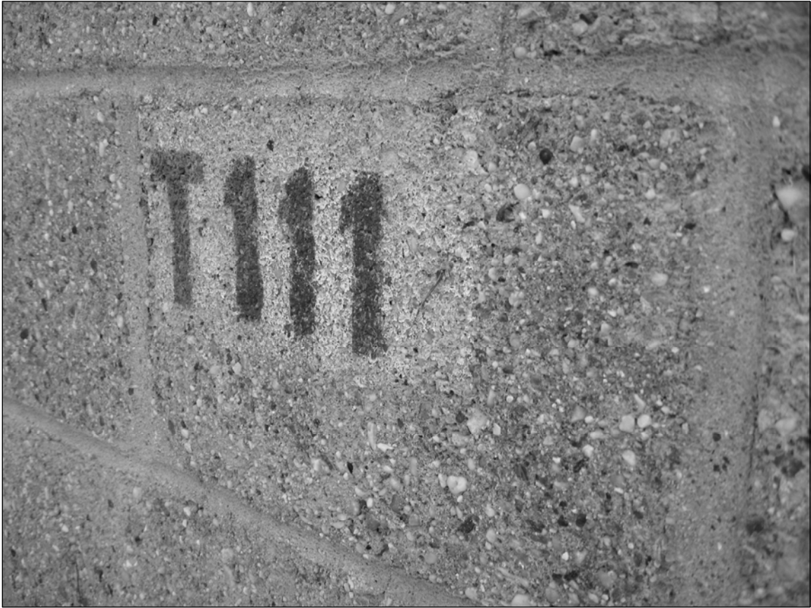
Photo 5. Western façade, detail: stenciled building number to right of doorway.
