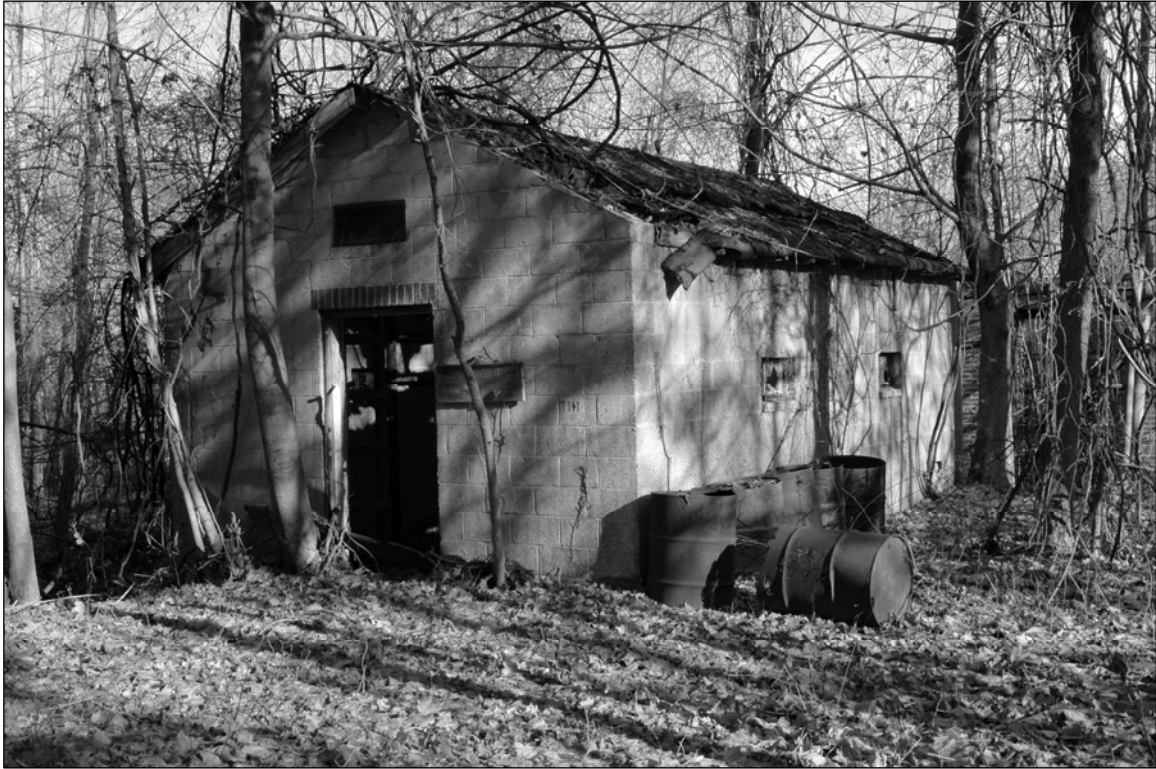
Photo 1. Western and southern façades, facing northeast.
