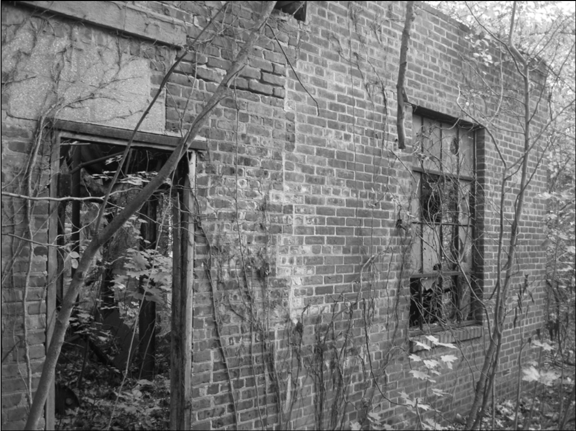
Photo 8. Western façade, detail: southern extension to building, looking southeast.
