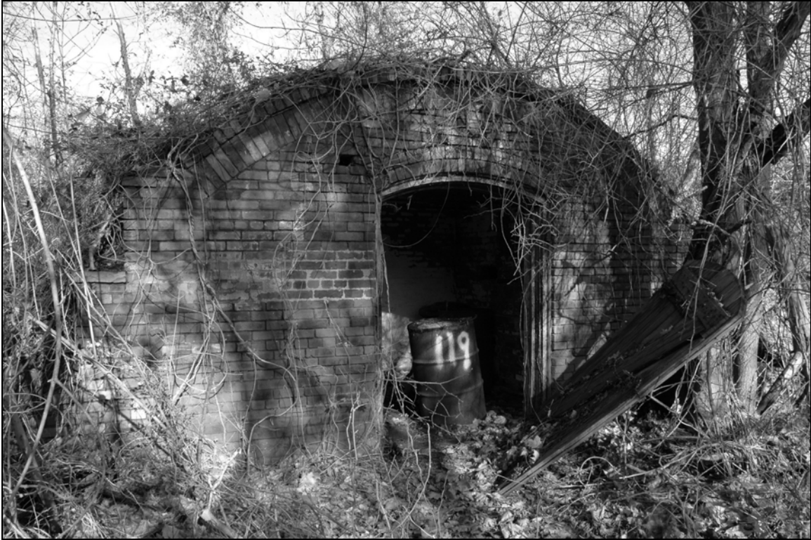
Photo 1. Southern façade, facing southeast.
