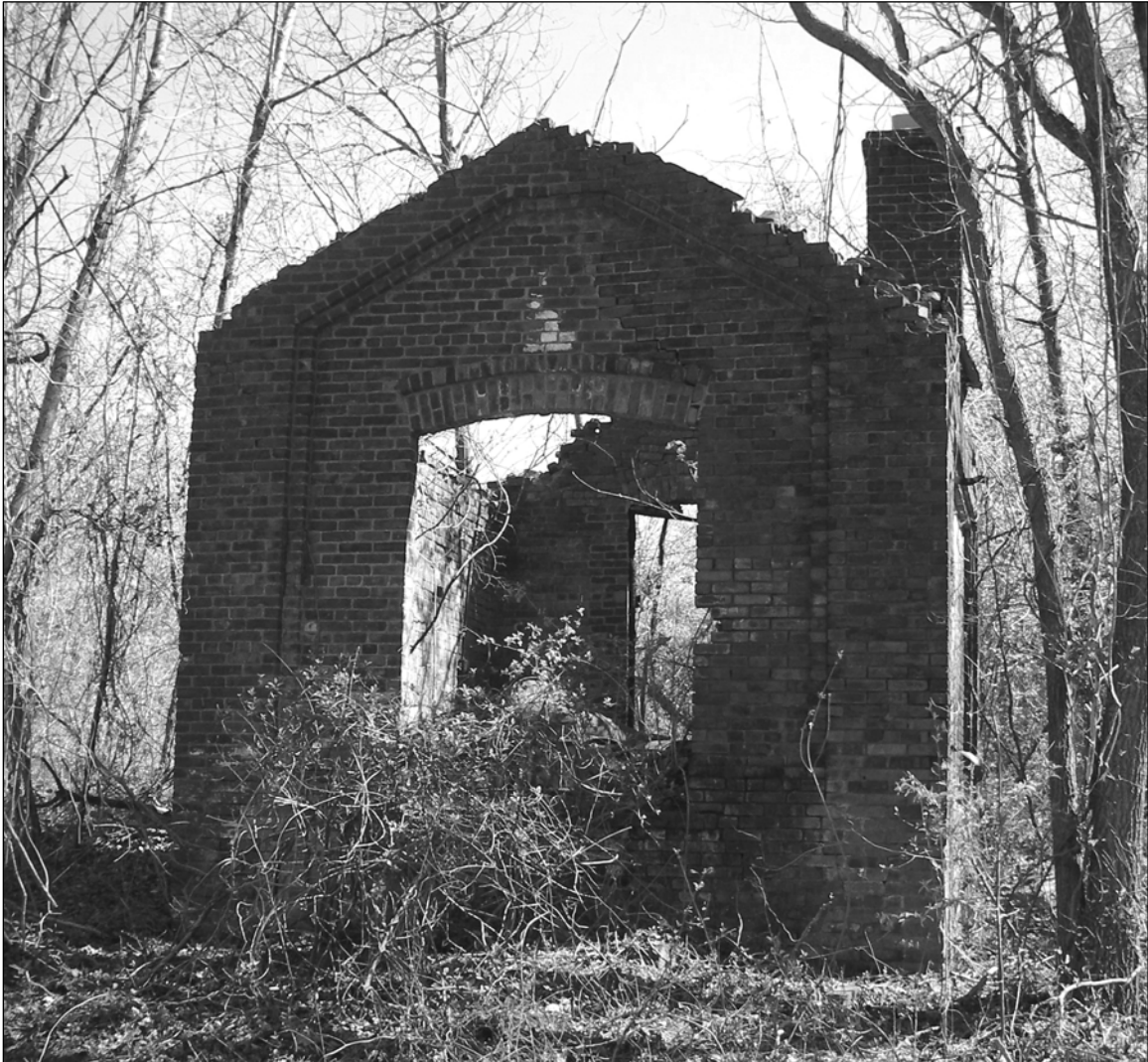
Photo 2. Northern façade, facing south.
