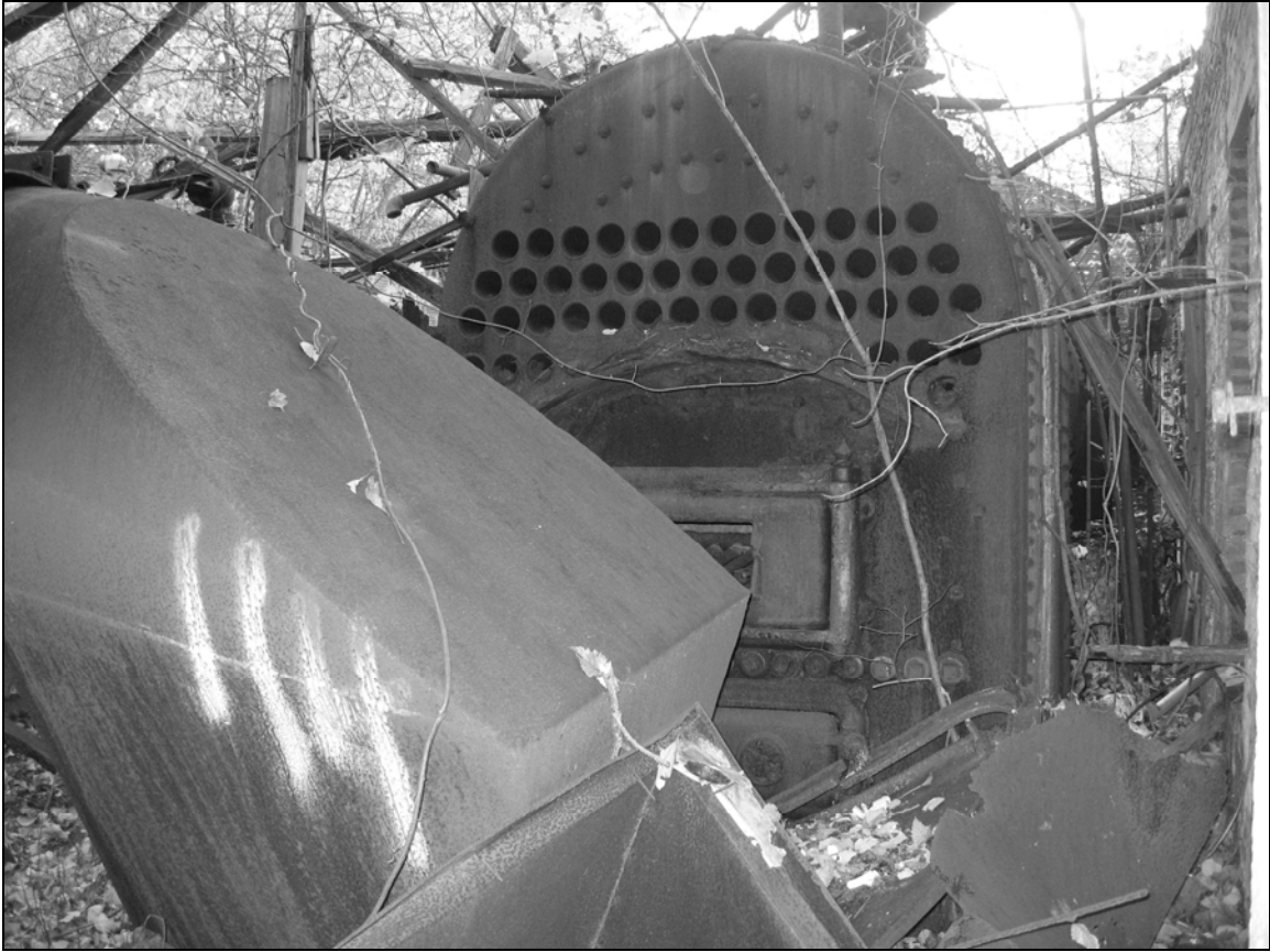
Photo 9. Northern section of building, interior, showing ruins of boiler system.
