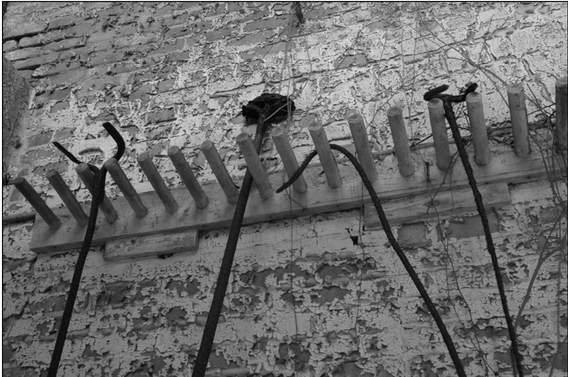
Photo 6. Building interior, detail—stoking floor tool rack.
