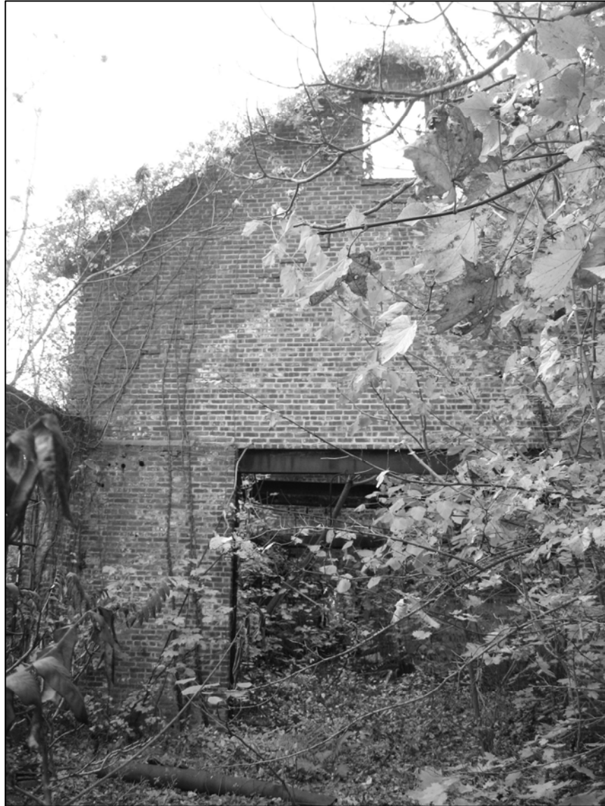
Photo 13. East wing, interior, facing south toward two-story addition.
