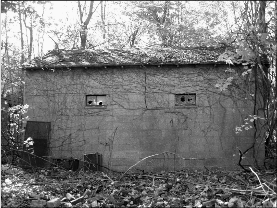
Photo 2. Southern façade, facing north.
