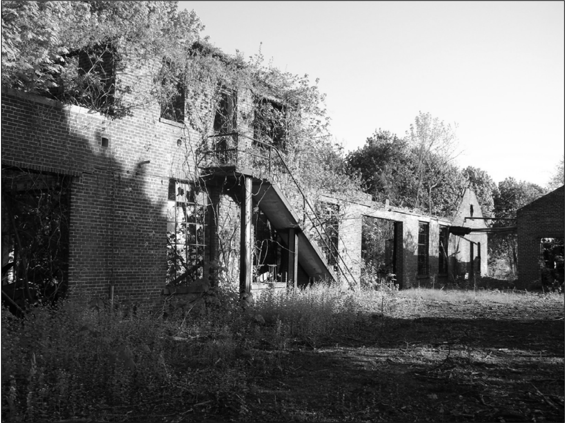
Photo 17. East wing, eastern façade, facing northwest.
