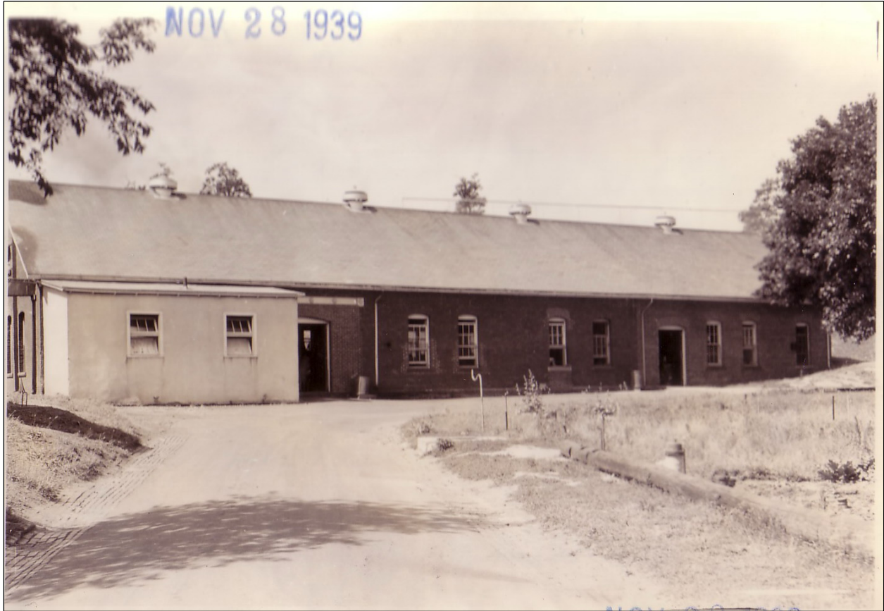
Figure 4. Inventory photo, ca. 1939. North façade of north wing of Building 110. View to south-southwest. Record Group 77, National Archives, College Park, MD.
