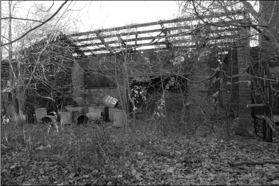
Photo 2. Northern façade of building as viewed from work yard, facing south.
