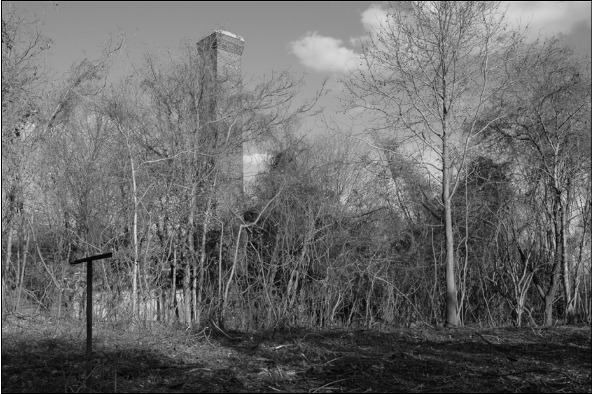
Photo 1. Incinerator chimney, facing east-northeast.
