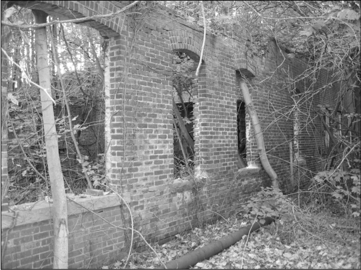
Photo 5. North wing, original section of building, northern façade, facing southwest.
