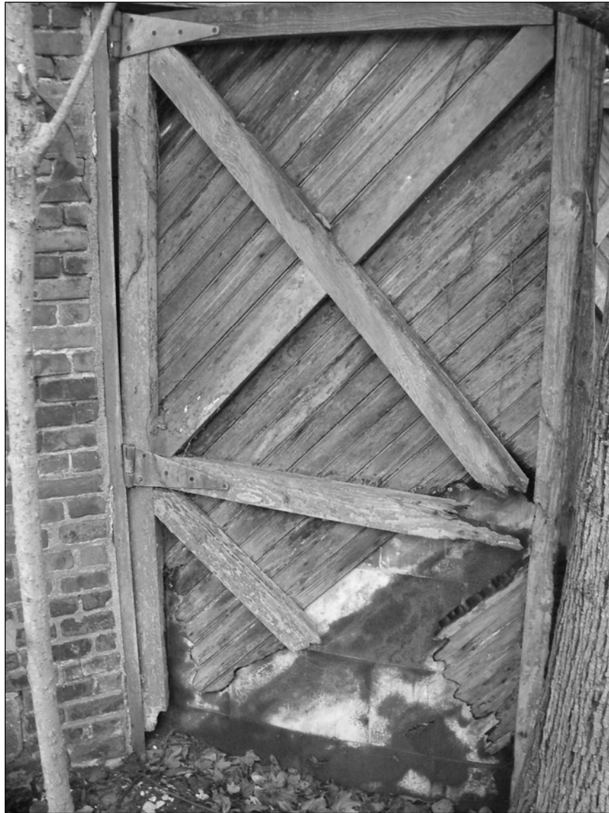
Photo 3. Northern façade, detail: cross-braced door in eastern section of main portion of façade.
