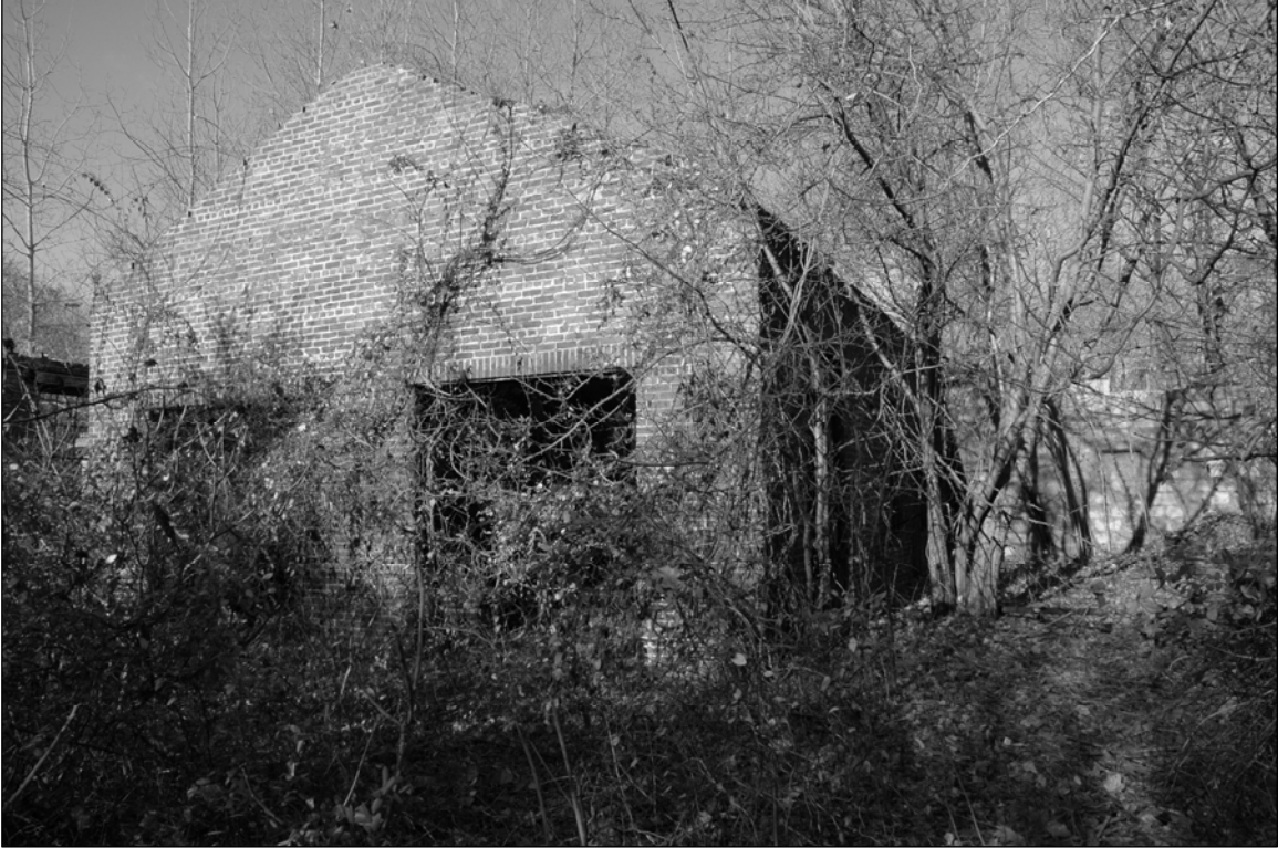
Photo 5. Southern façade, looking northwest.
