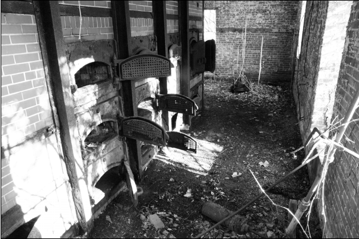
Photo 5. Building interior, stoking floor, showing stoking and ash doors, facing southeast.
