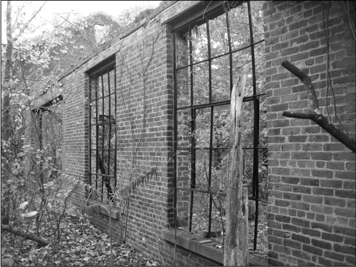
Photo 11. One-and-a-half story main section of east wing, eastern façade, facing southwest.
