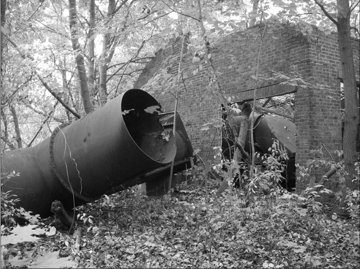
Photo 1. Northern façade, facing southeast. Collapsed smokestack at left. The smokestack's T-joint, which projects to the right in the photo, once extended into Building 114.
