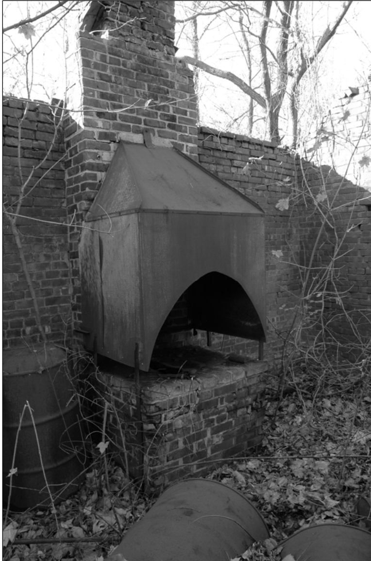
Photo 6. Interior, detail: blacksmith hearth with hood and chimney, facing west-northwest.
