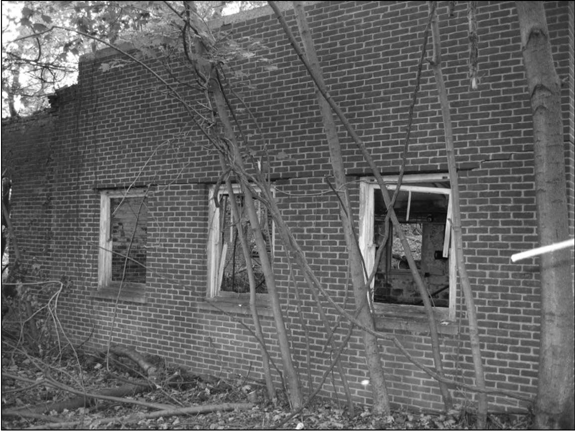
Photo 4. North wing, northern façade of one-story addition, facing southeast.
