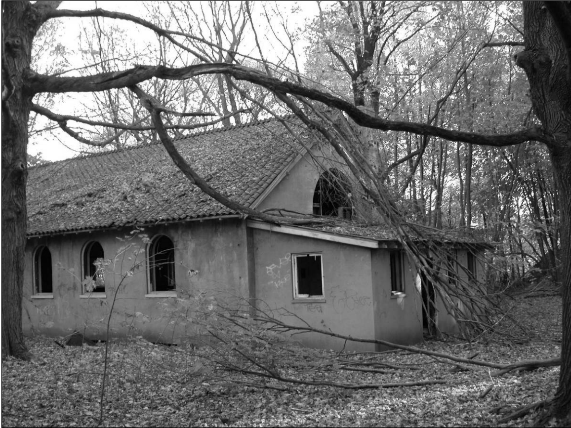
Photo 5. Southern and eastern façades, including rear shed addition, facing northeast.
