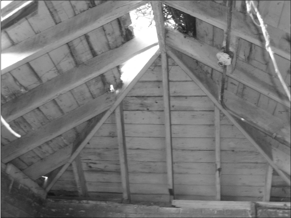
Photo 4. Interior, detail of roof framing, facing west.
