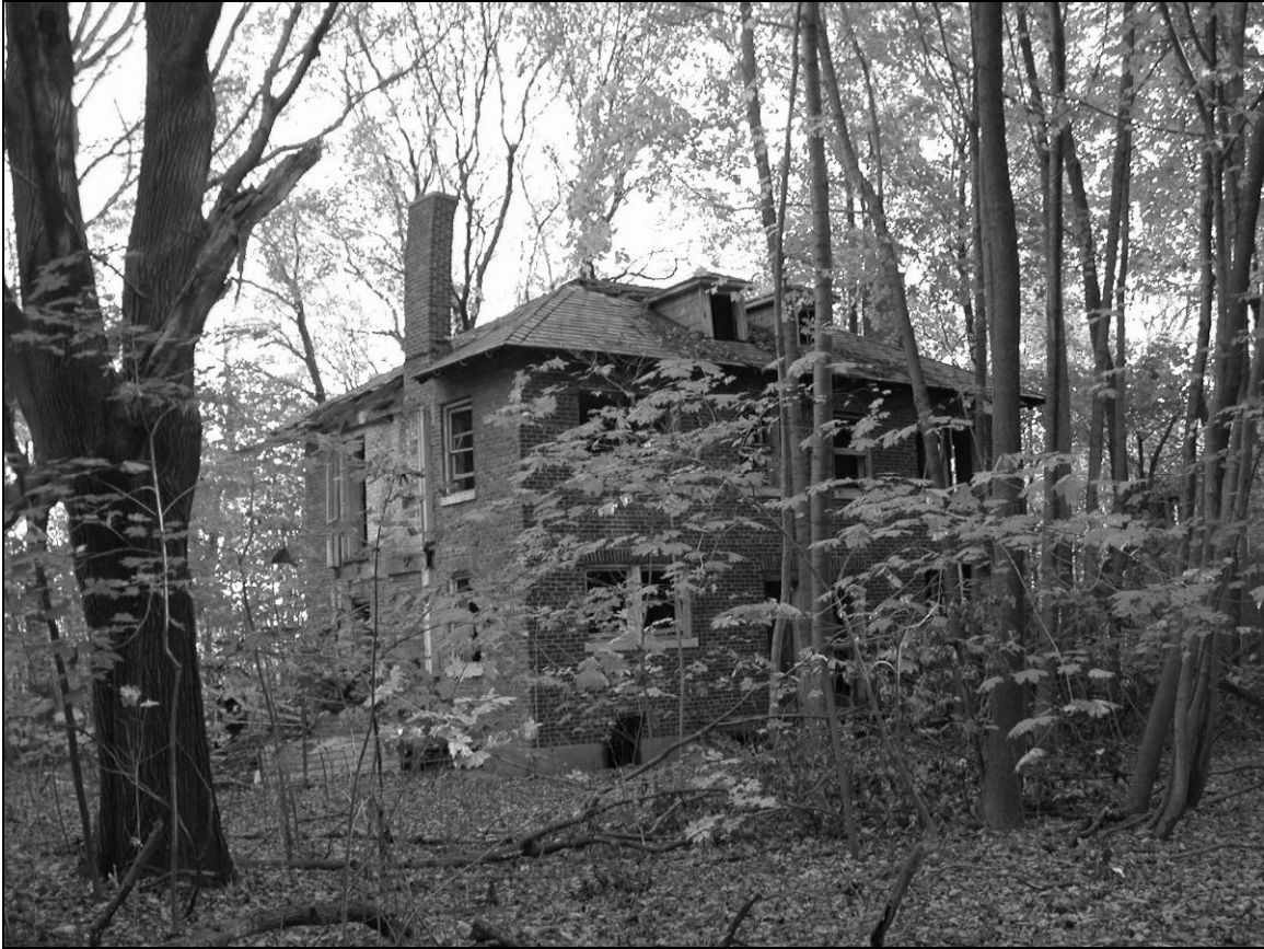
Photo 3. Southern and western façades, facing northeast.
