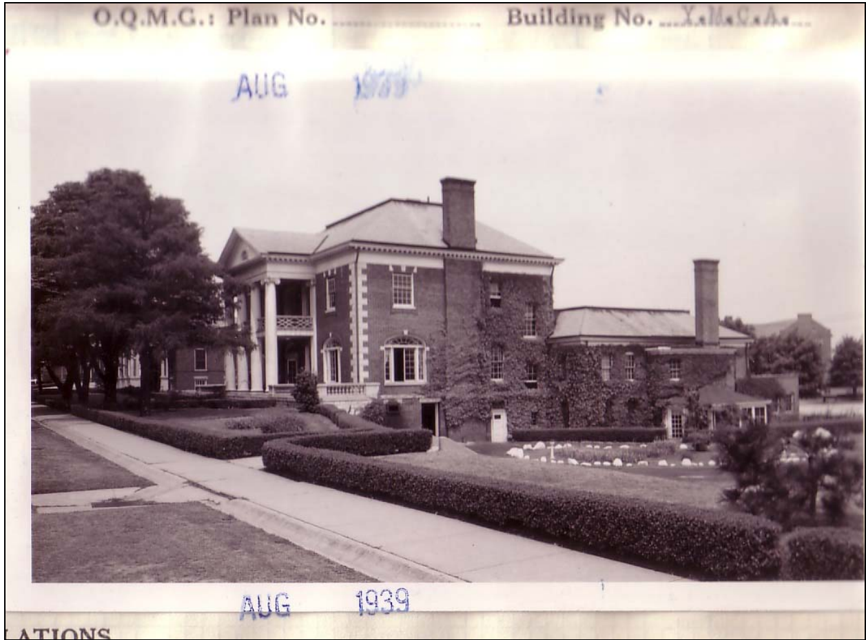
Figure 9. YMCA, facing northeast, August 1939. Detail of Quartermaster Property Record. Record Group 77, National Archives, College Park, MD.
