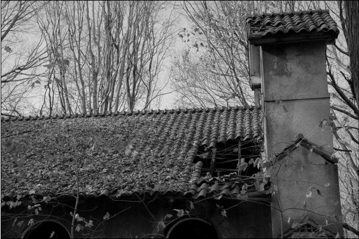
Photo 4. Detail of roof at northern end of building, facing west.
