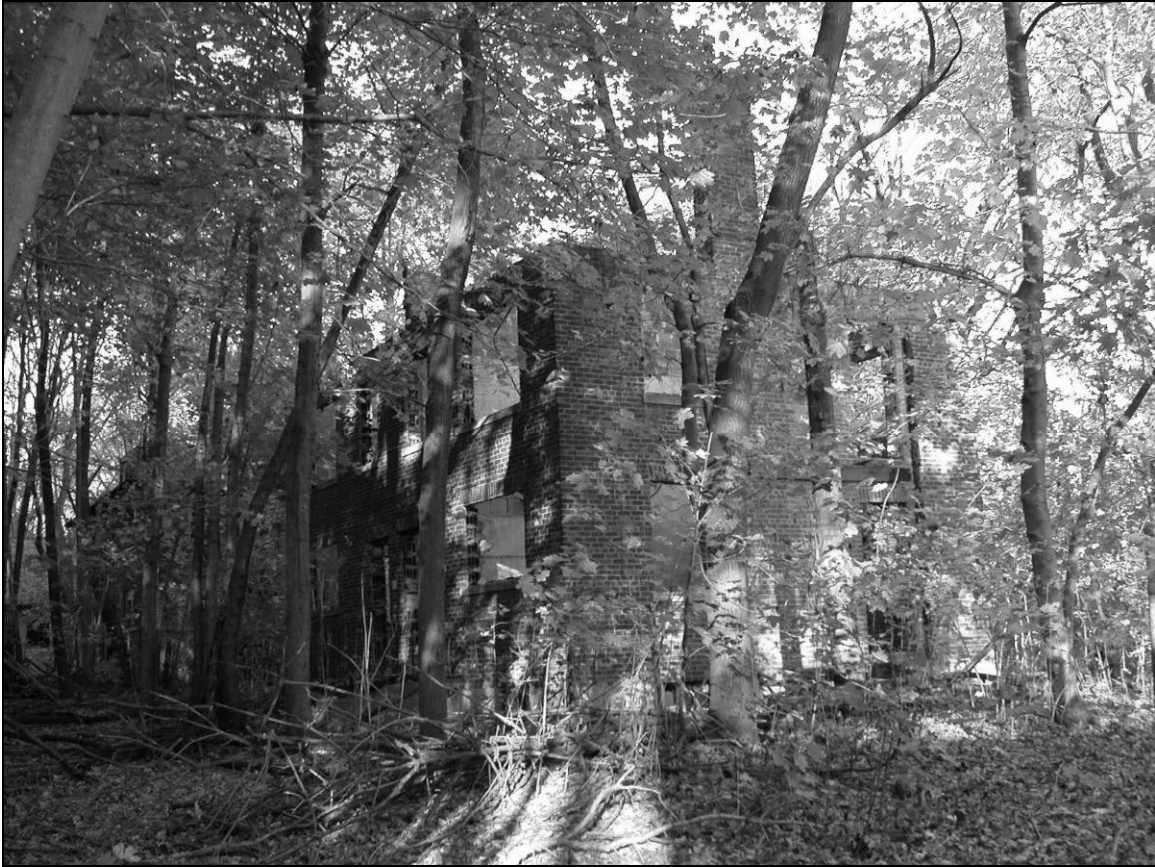
Photo 3. Eastern and northern façades, facing northwest.
