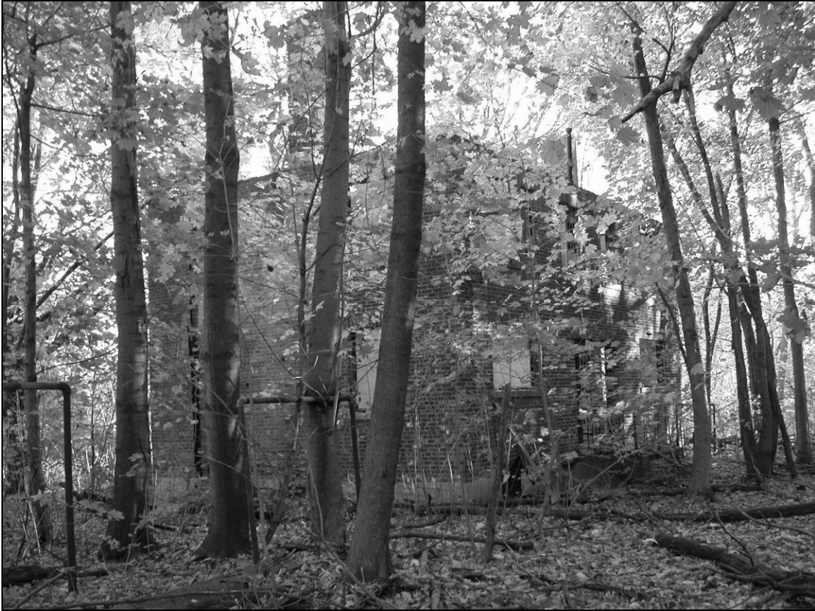
Photo 2. Western and northern façades, facing east.
