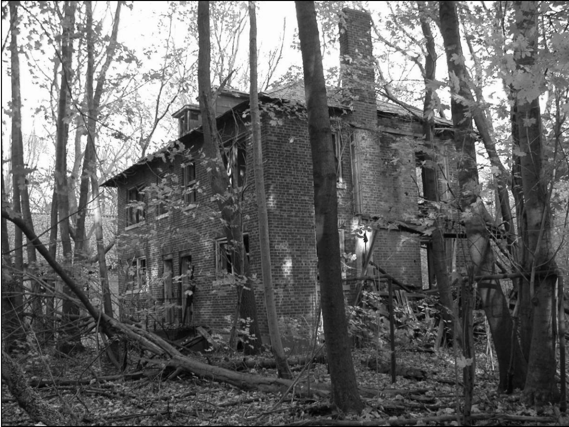
Photo 4. Southern and eastern façades, facing northwest.
