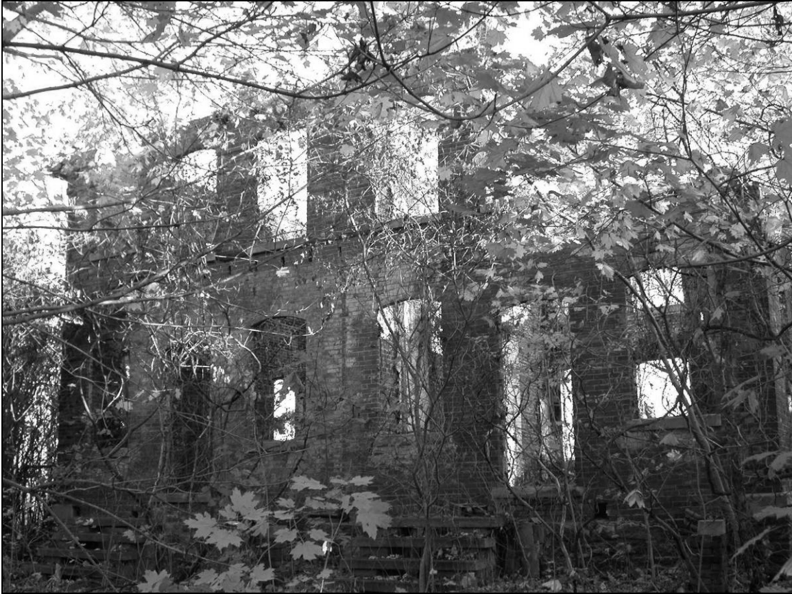
Photo 2. Western façade, facing northeast.
