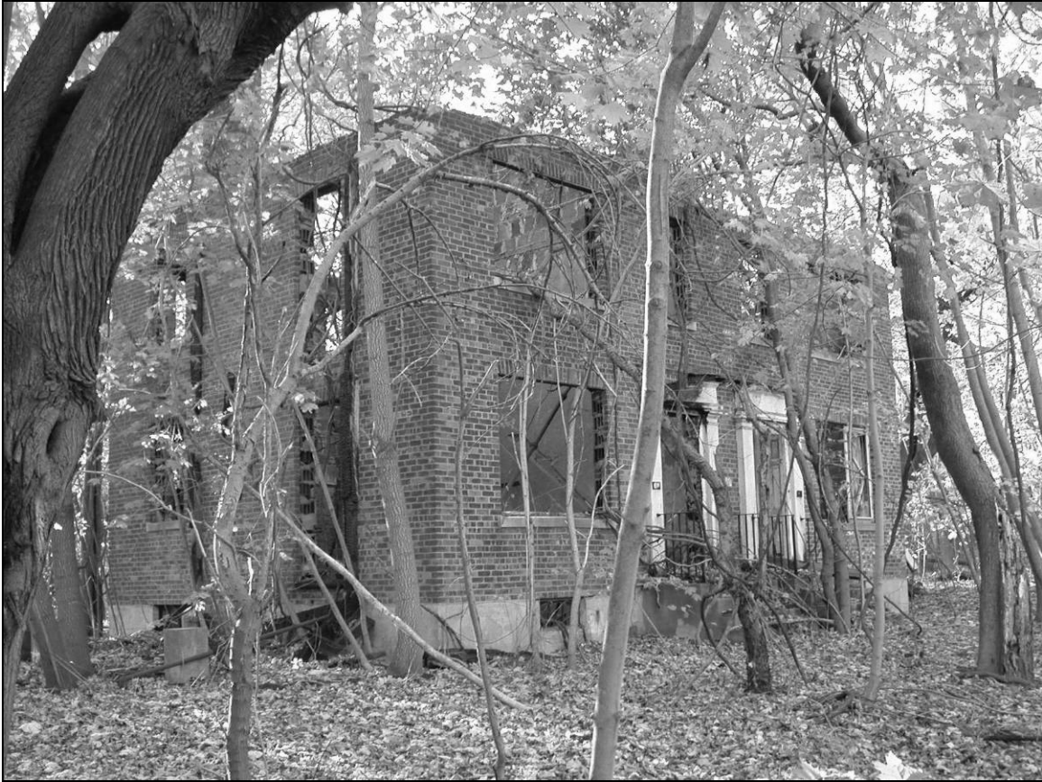
Photo 4. Western and southern façades, facing north.
