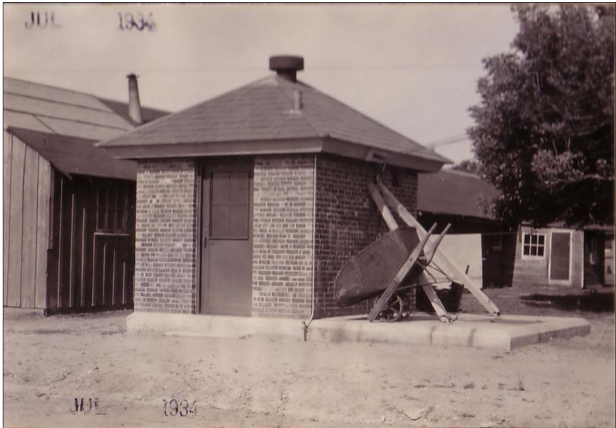
Figure 4. Inventory Photograph, July 1934. View southwest. Building 74 was built between three wood-frame temporary barracks of First World War vintage, which were removed in ca. 1936. Two of the temporary barracks are shown here, to the left of and behind Building 74. Record Group 77, National Archives, College Park, MD.
