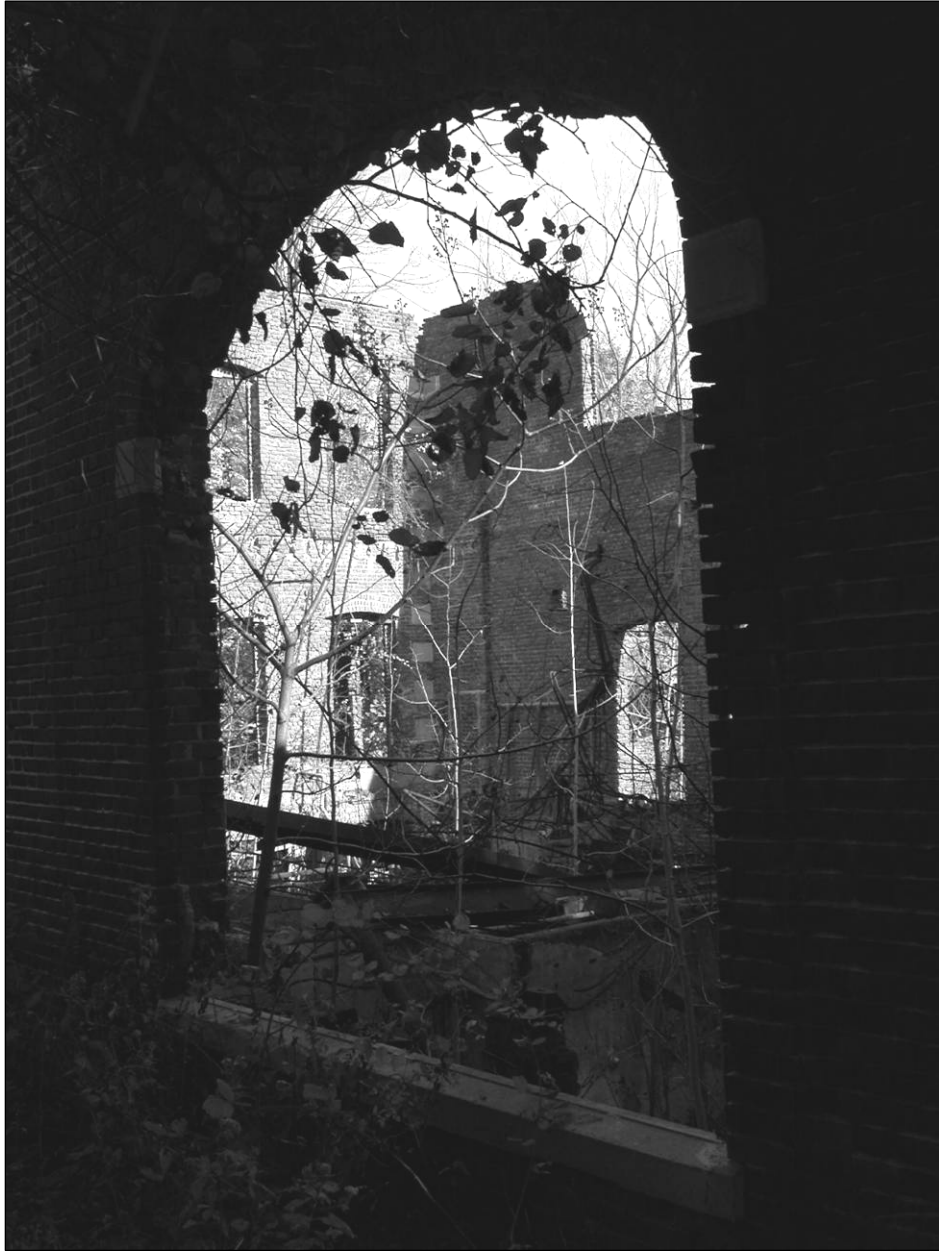
Photo 6. Interior, facing northeast.
