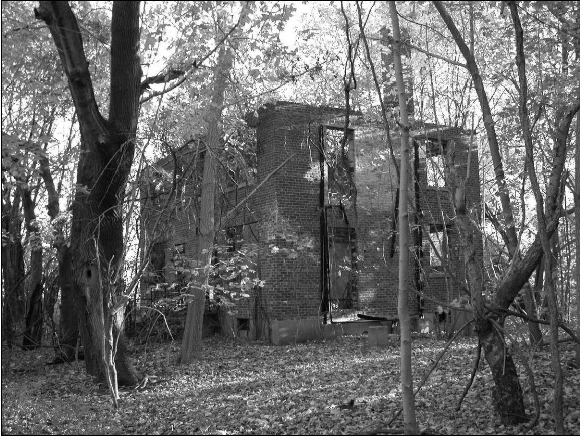
Photo 1. Western and southern façades, facing northeast.
