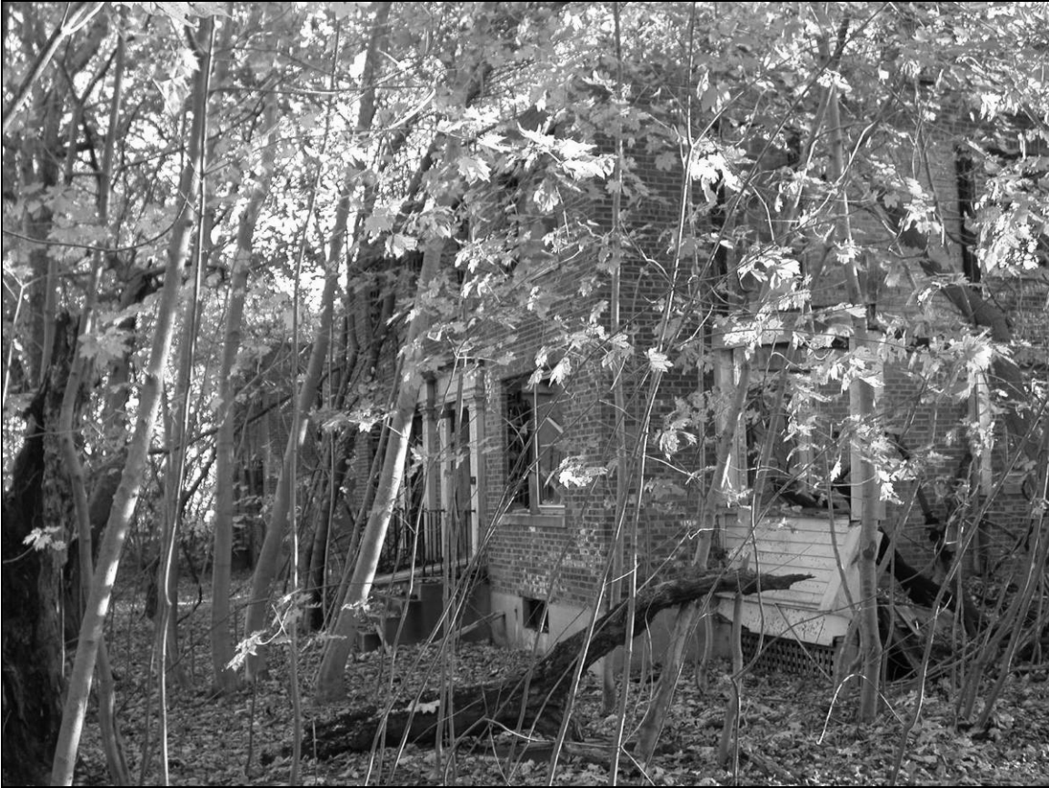
Photo 3. Northern and western façades, facing east.
