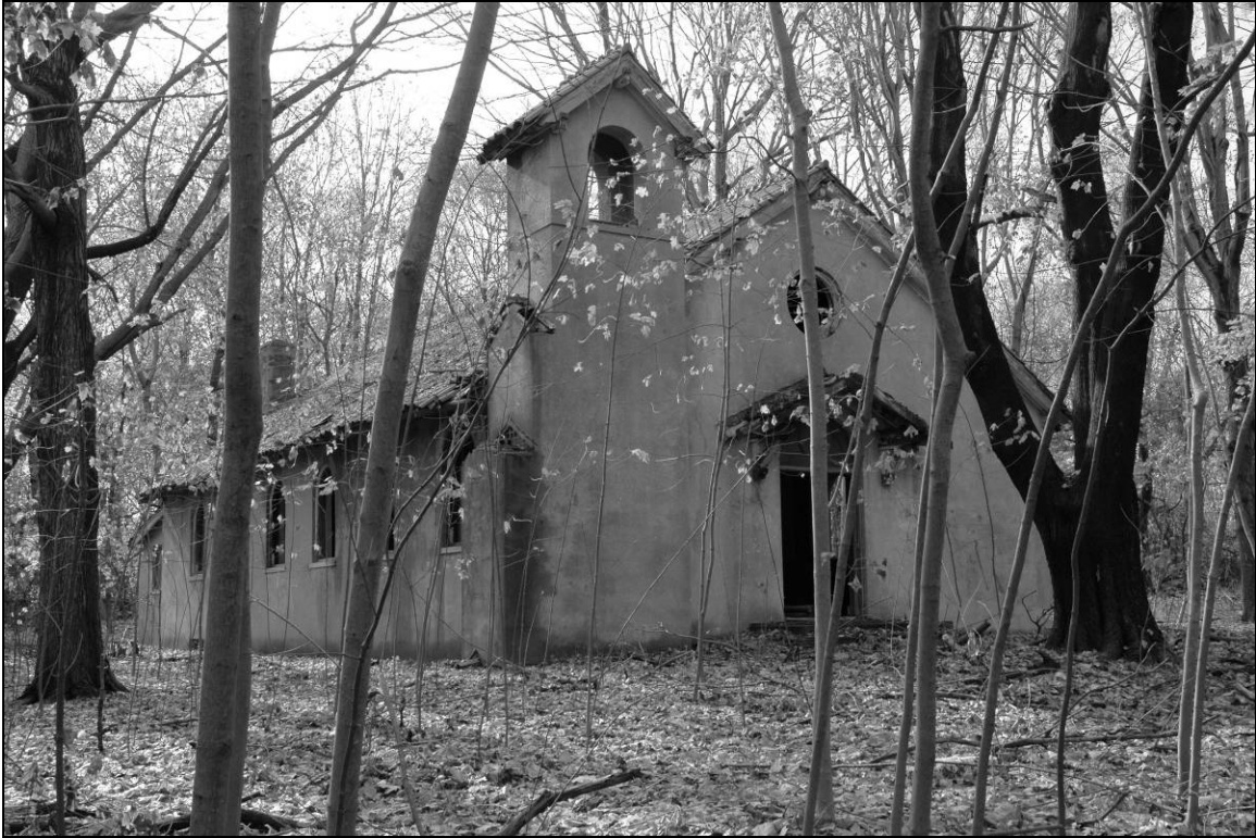
Photo 1. Northern and eastern façades, facing southwest.
