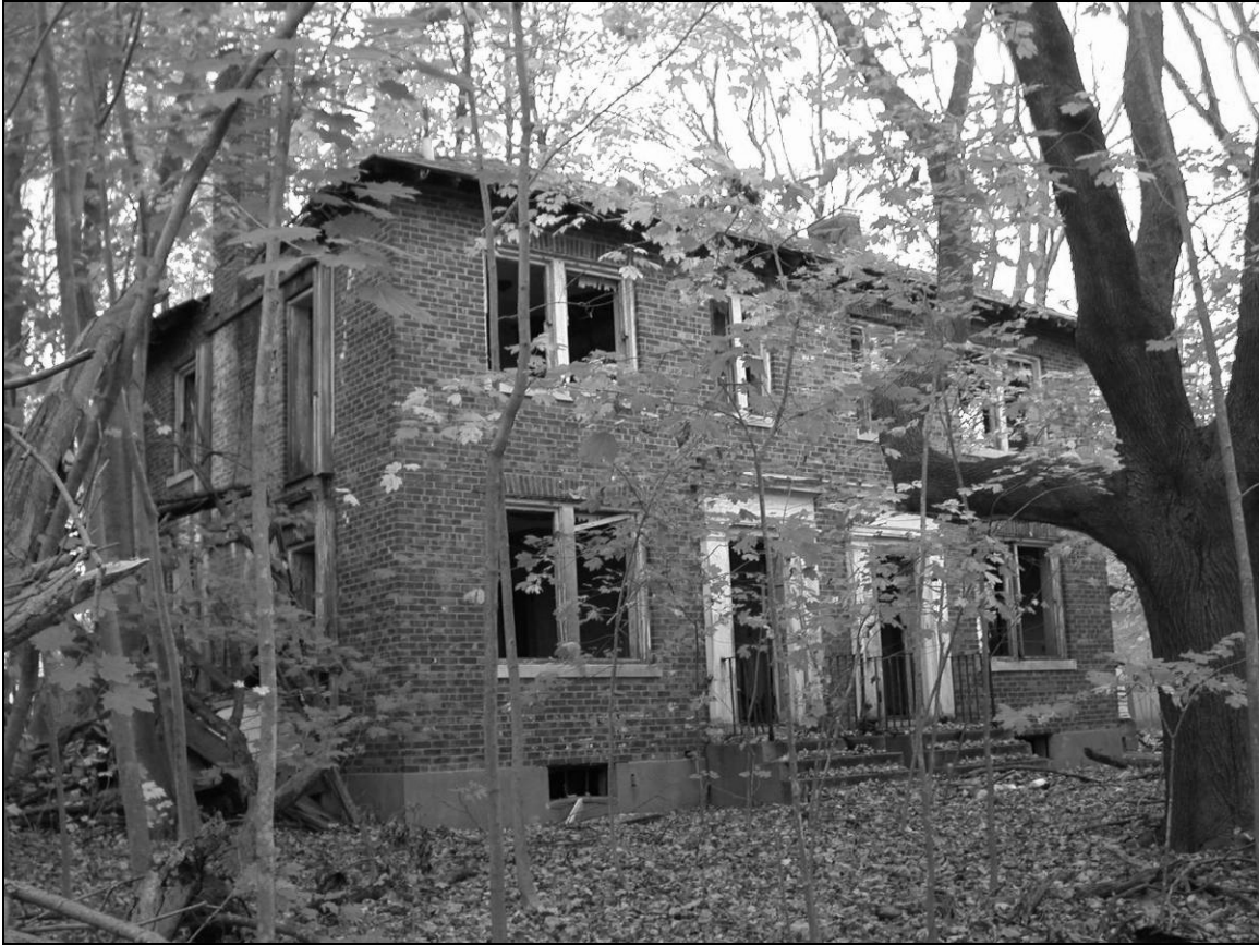
Photo 1. Northern and eastern façades, facing southwest.
