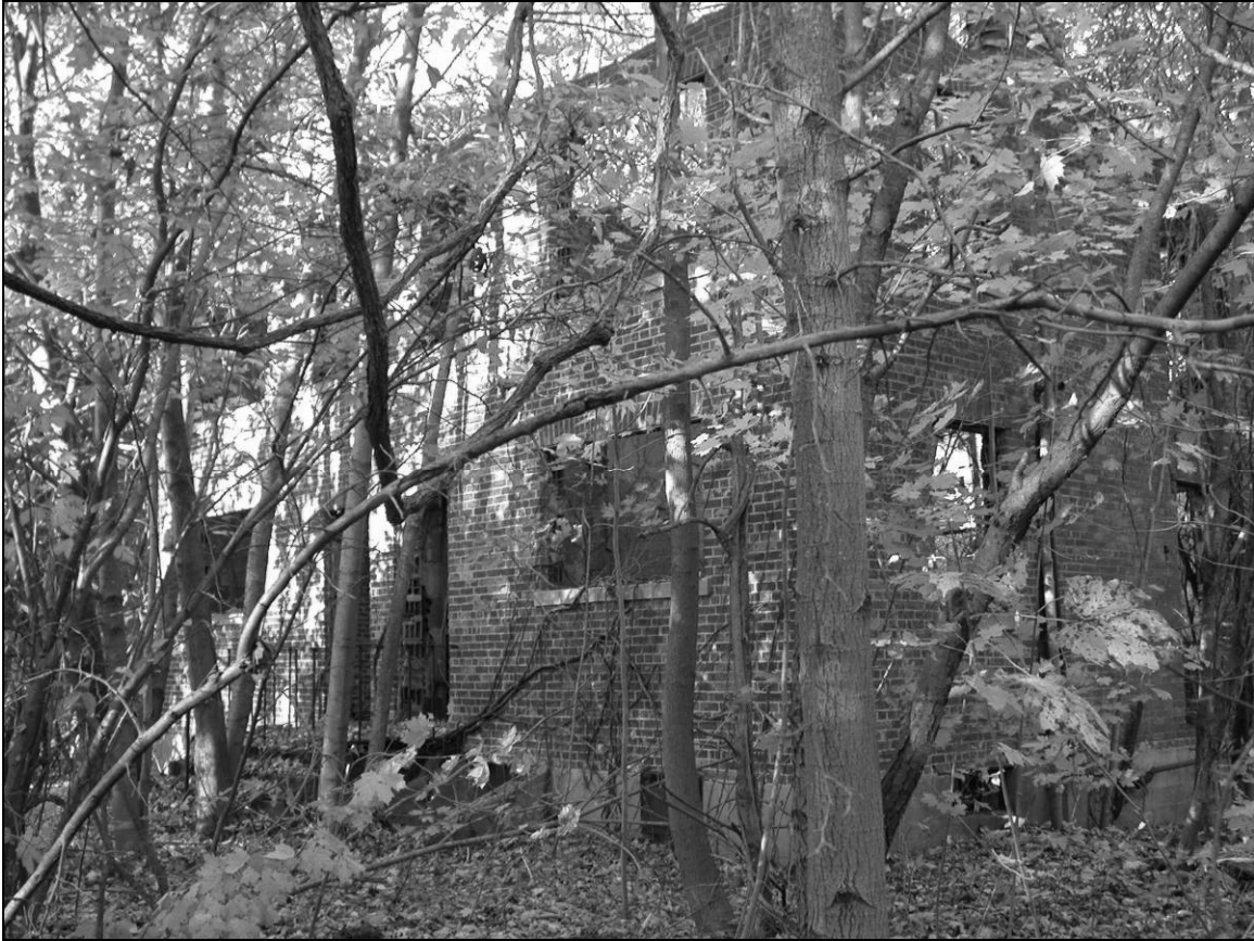
Photo 3. Northwestern façade, facing southeast.
