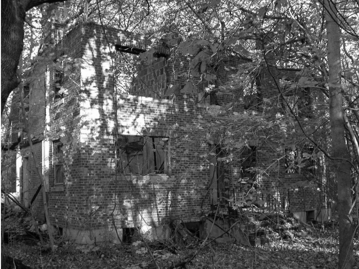
Photo 2. Eastern and northern façades, facing south.
