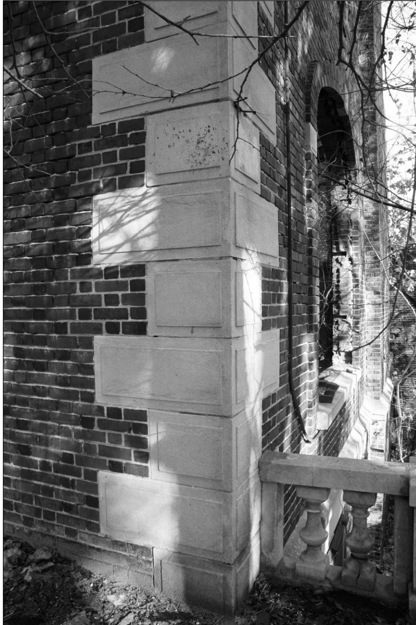
Photo 3. Western façade, detail—quoin at northwestern corner, facing southeast.
