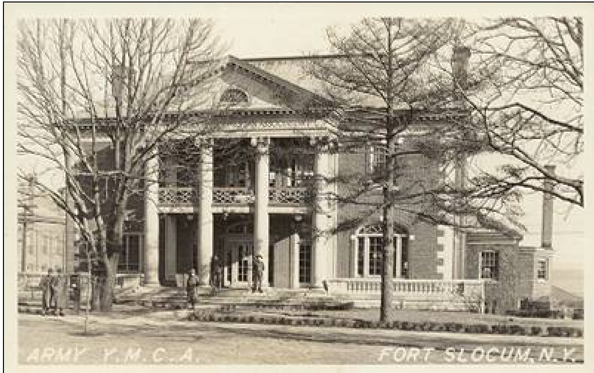
Figure 10. "Army Y.M.C.A., Fort Slocum, N.Y.," ca. 1940. Postcard view of Building 71, facing east. Real-photo postcard. Unknown publisher and date of publication. Fort Slocum Collection, New Rochelle Public Library, New Rochelle, New York.
