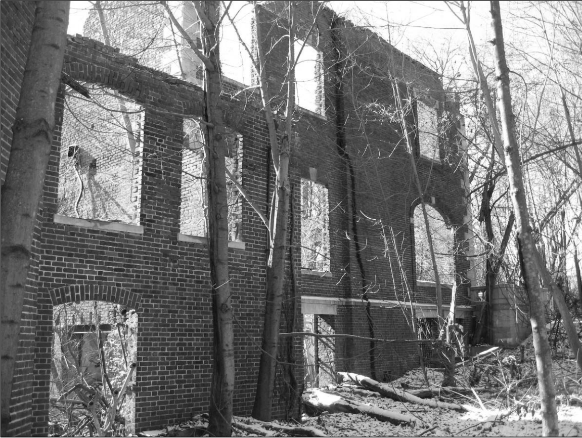
Photo 5. Western end of northern façade, facing southwest.
