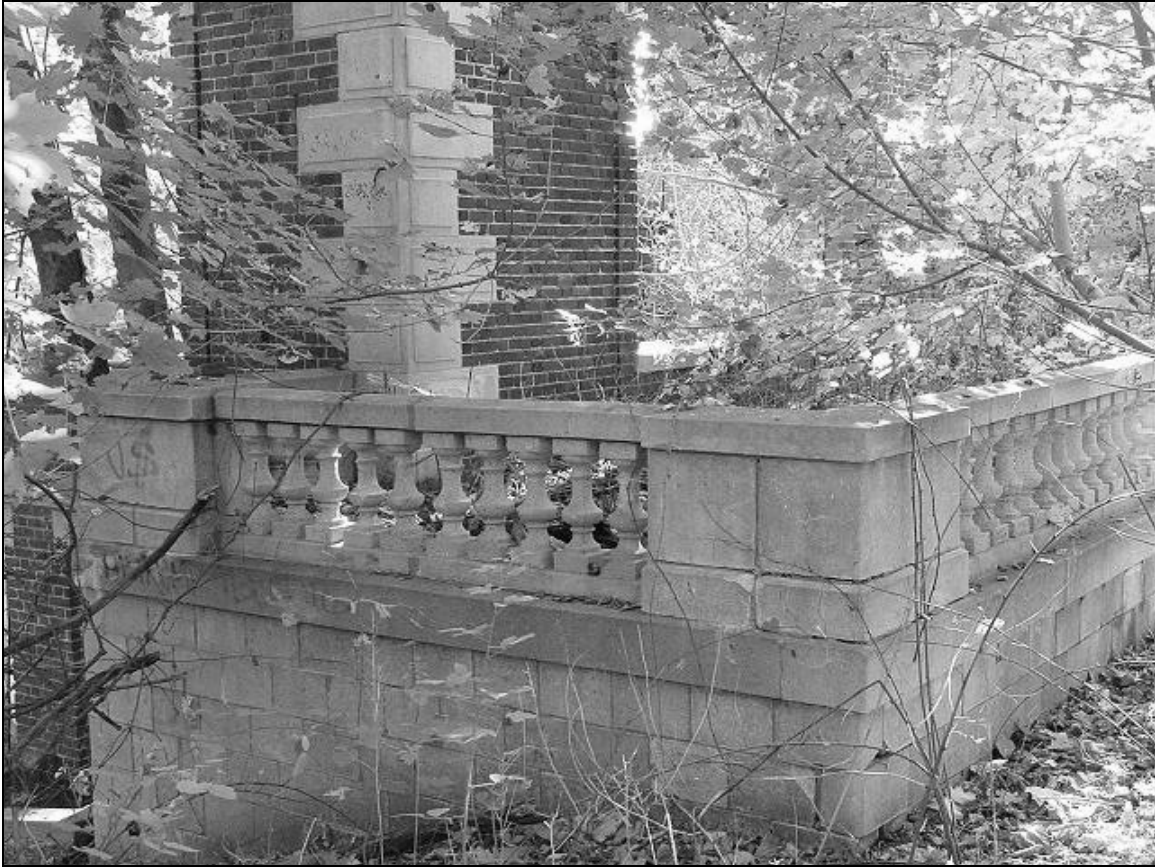
Photo 4. Western façade, detail—northern end of porch balustrade, facing southeast.
