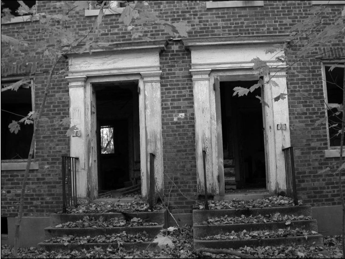
Photo 2. Northern façade, detail showing entrances.
