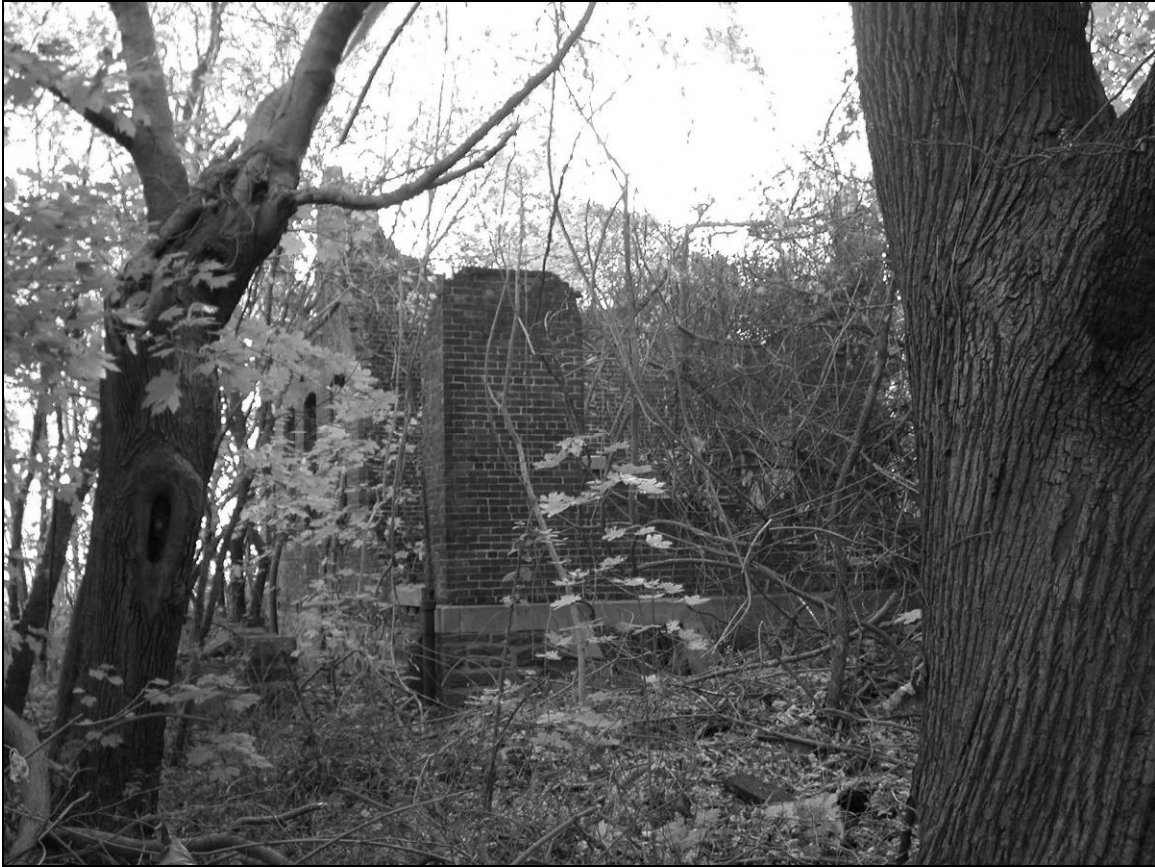
Photo 2. Northern and western façades, facing east.
