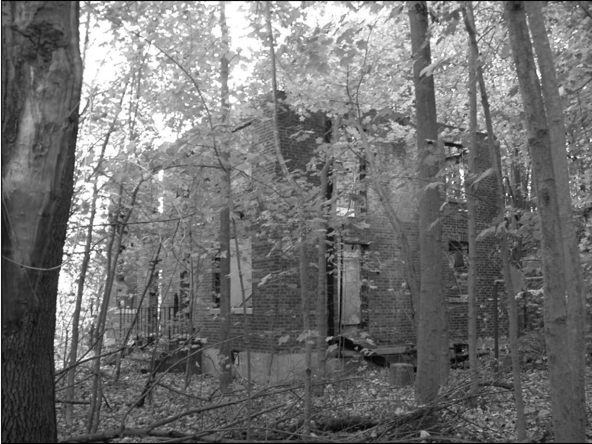
Photo 4. Southern and western façades, facing northeast.
