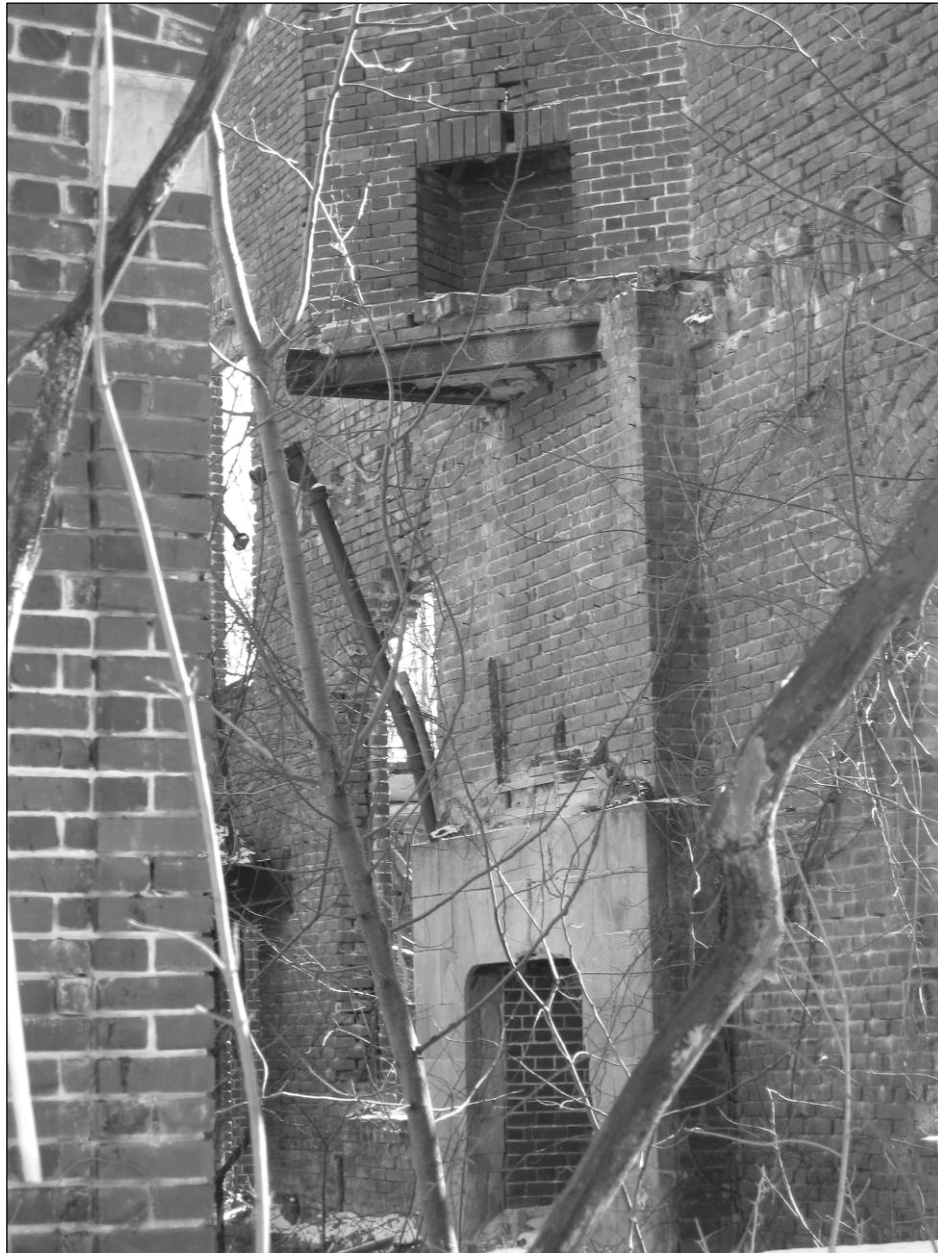
Photo 7. Interior—first- and second-story fireplaces in front section of building, facing southeast.
