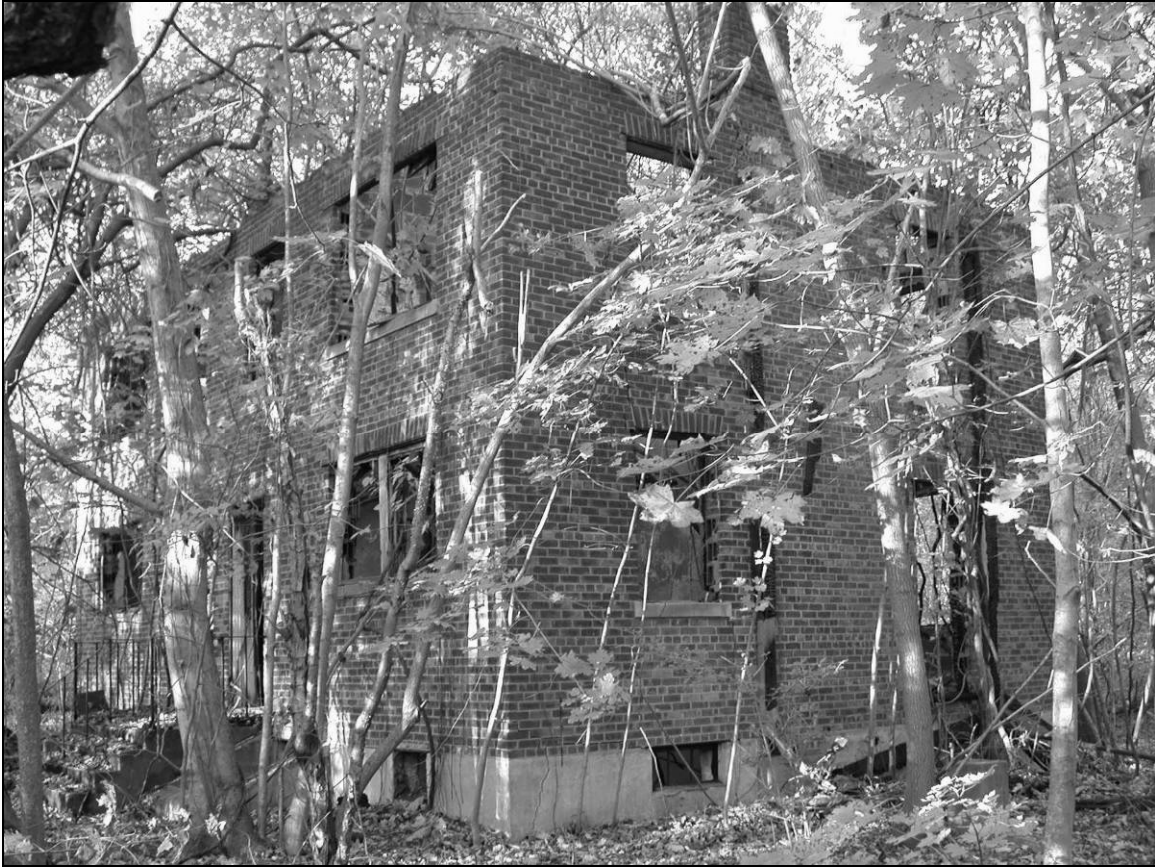
Photo 5. Southern and eastern façades, facing southwest.
