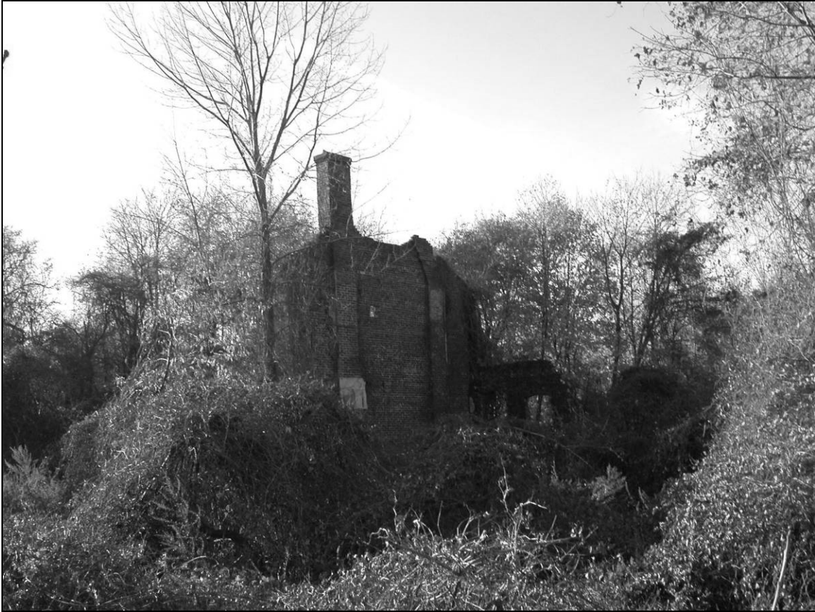
Photo 3. Remnant interior wall, facing south.
