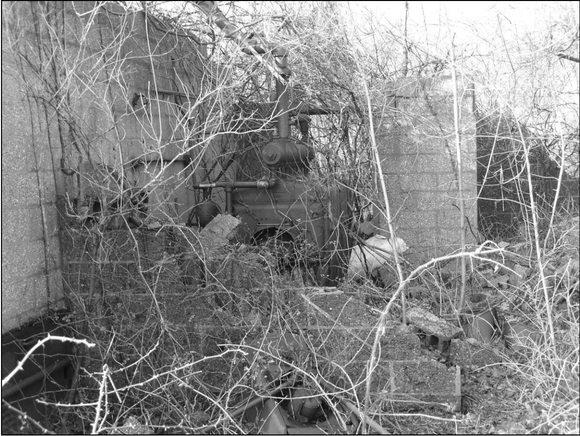
Photo 2. Interior view of auxiliary mechanical remains, facing west.
