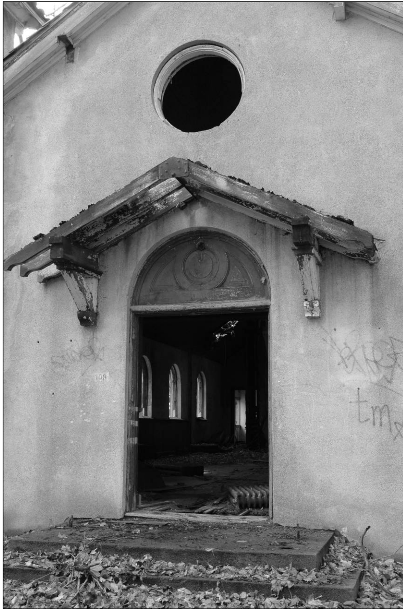
Photo 3. Northern façade, detail, showing main entrance, facing south.
