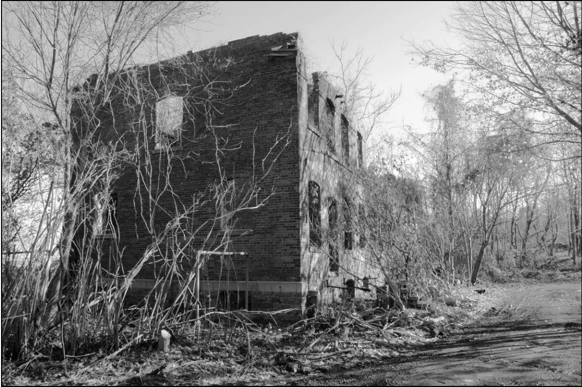
Photo 1. Northern and western façades, facing southeast.
