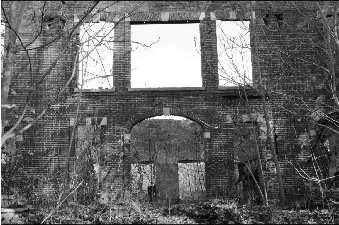
Photo 2. Western façade, detail—main entrance and adjoining window openings, facing east.
