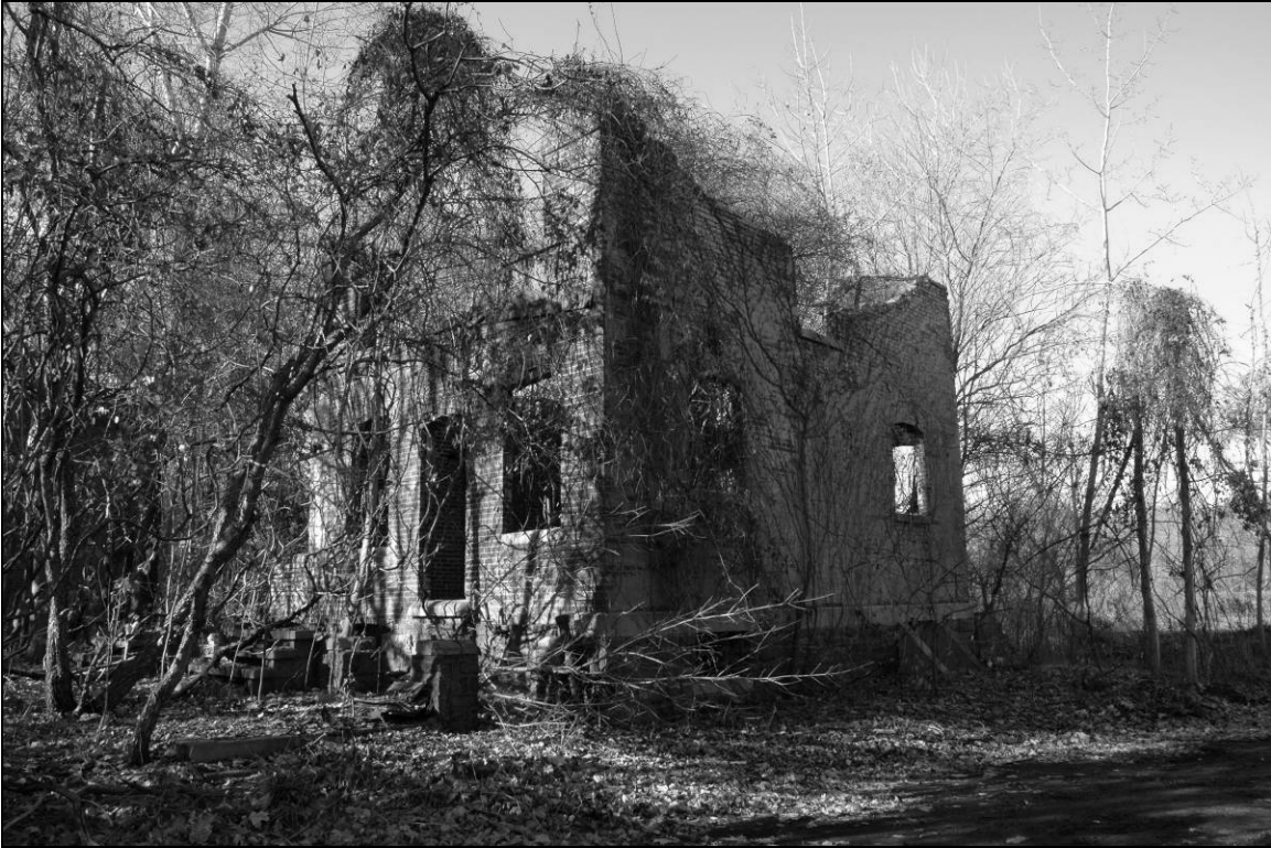
Photo 1. Southern and eastern façades, facing northwest.
