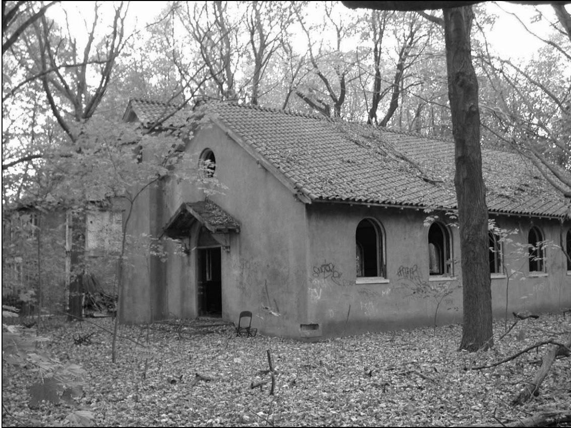
Photo 2. Northern and western façades, facing southeast.
