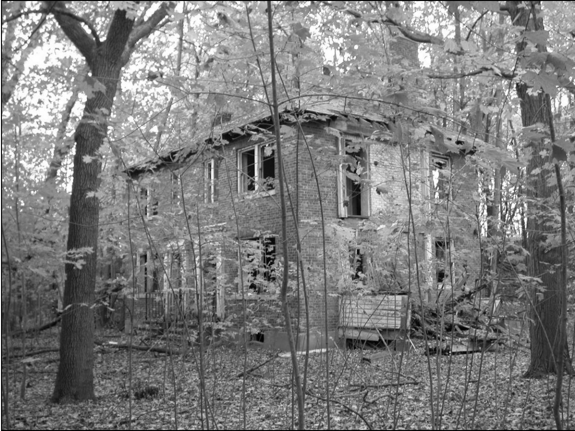
Photo 5. Northern and western façades, facing southeast.
