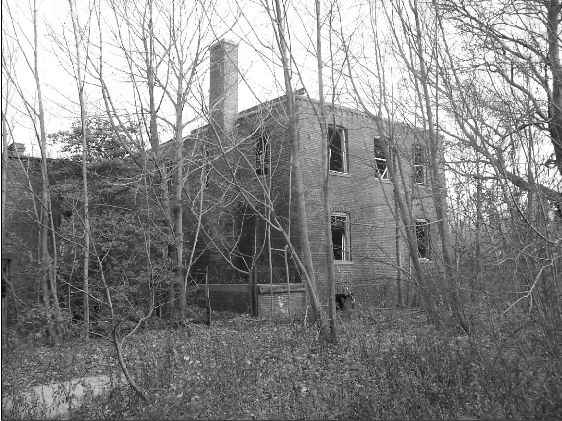
Photo 7. Southern façade, facing northeast.
