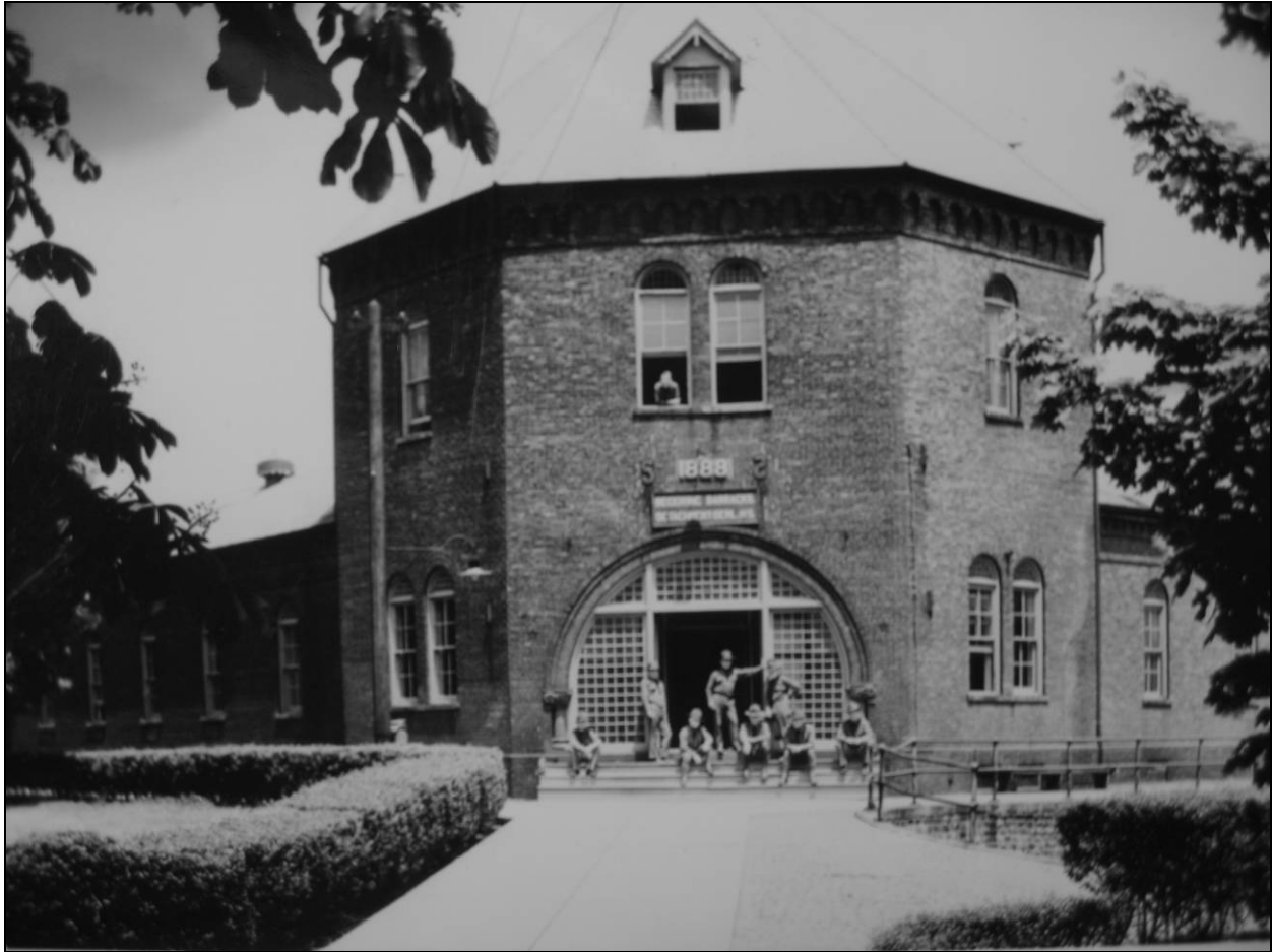
Figure 7. Building 69, ca 1918. View northeast. Record Group 111, National Archives, College Park, MD.
