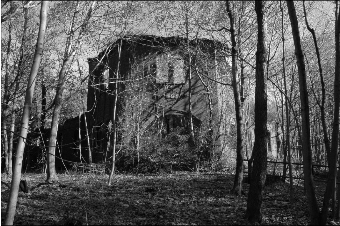
Photo 1. Southwestern façade of tower, facing northeast.
