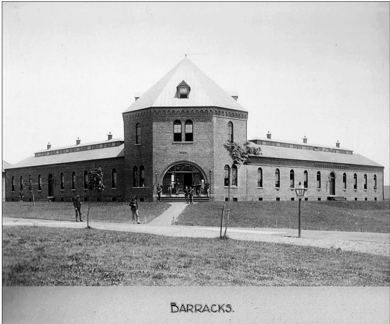
Figure 4. "Barracks" [Building 69], ca. 1893. View northeast. Original in National Archives, College Park, MD; digital copy from Fort Slocum Alumni and Friends Collection, Michael A. Cavanaugh, Los Angeles, CA, custodian.
