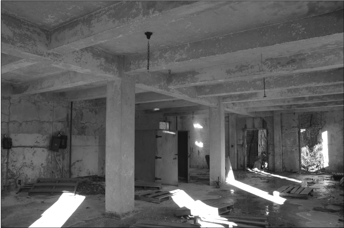
Photo 10. Interior of southern 1940 addition, facing northwest.
