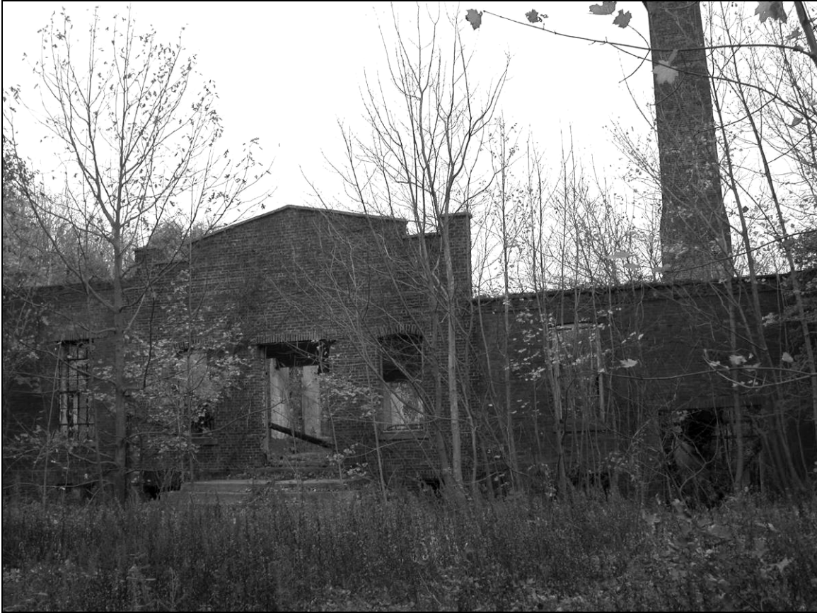
Photo 3. Southern façade, detail of gabled parapet and adjoining sections, facing north.
