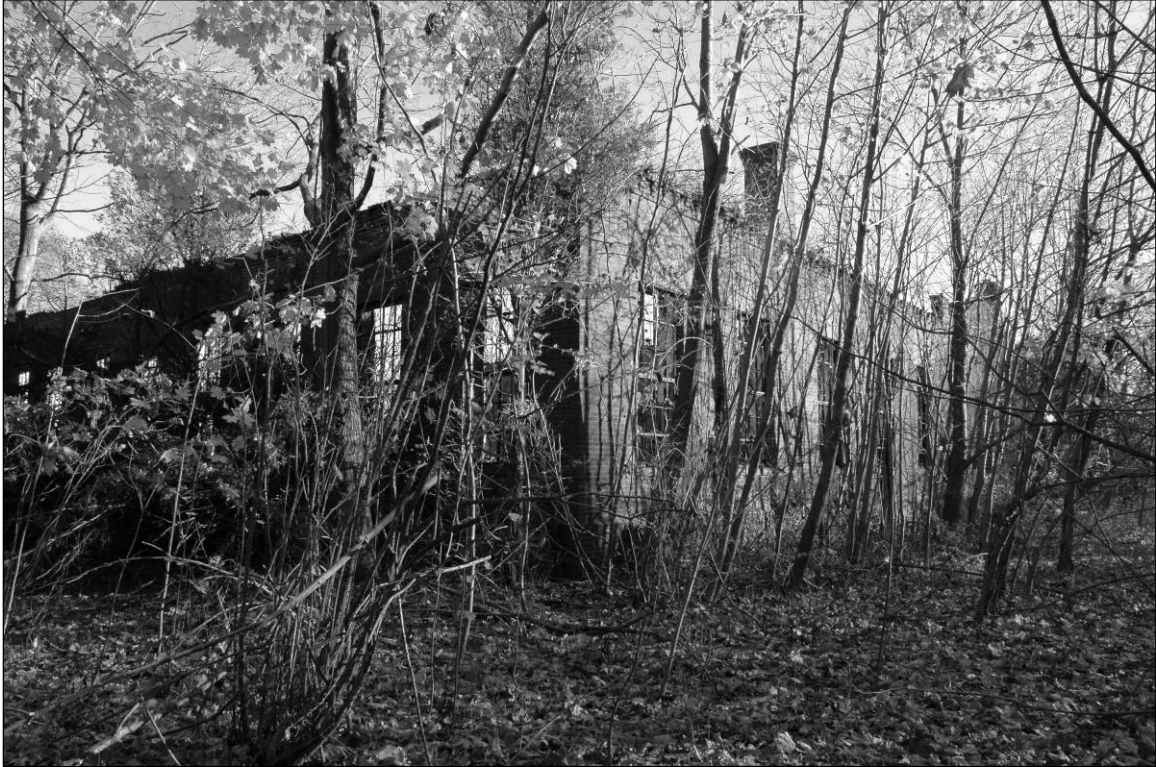
Photo 1. Southwestern corner of building, facing northeast.
