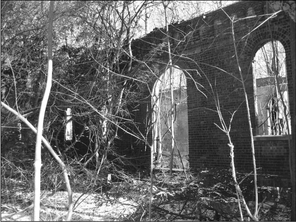
Photo 15. Western façade, showing door and window openings, facing northeast.
