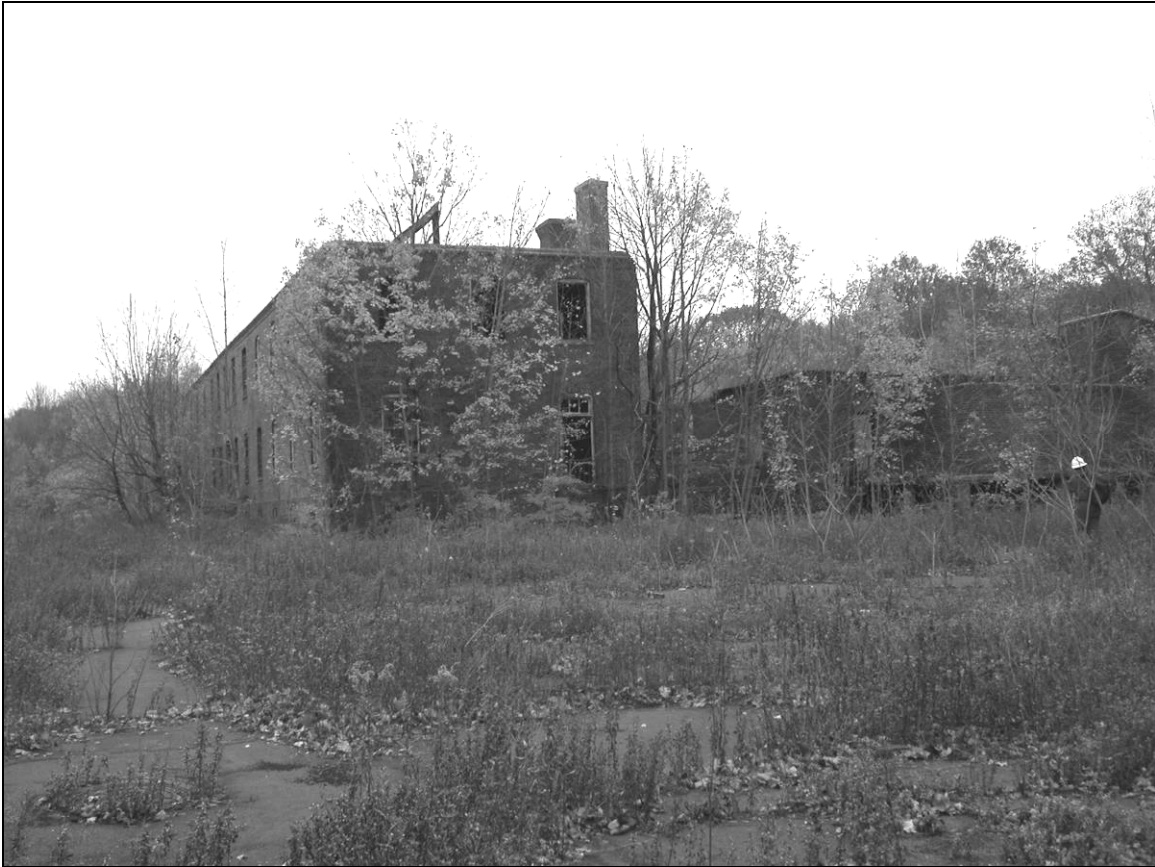
Photo 5. Northern end of Building 65 (left), facing south, with kitchen wing of Building 67 at right.
