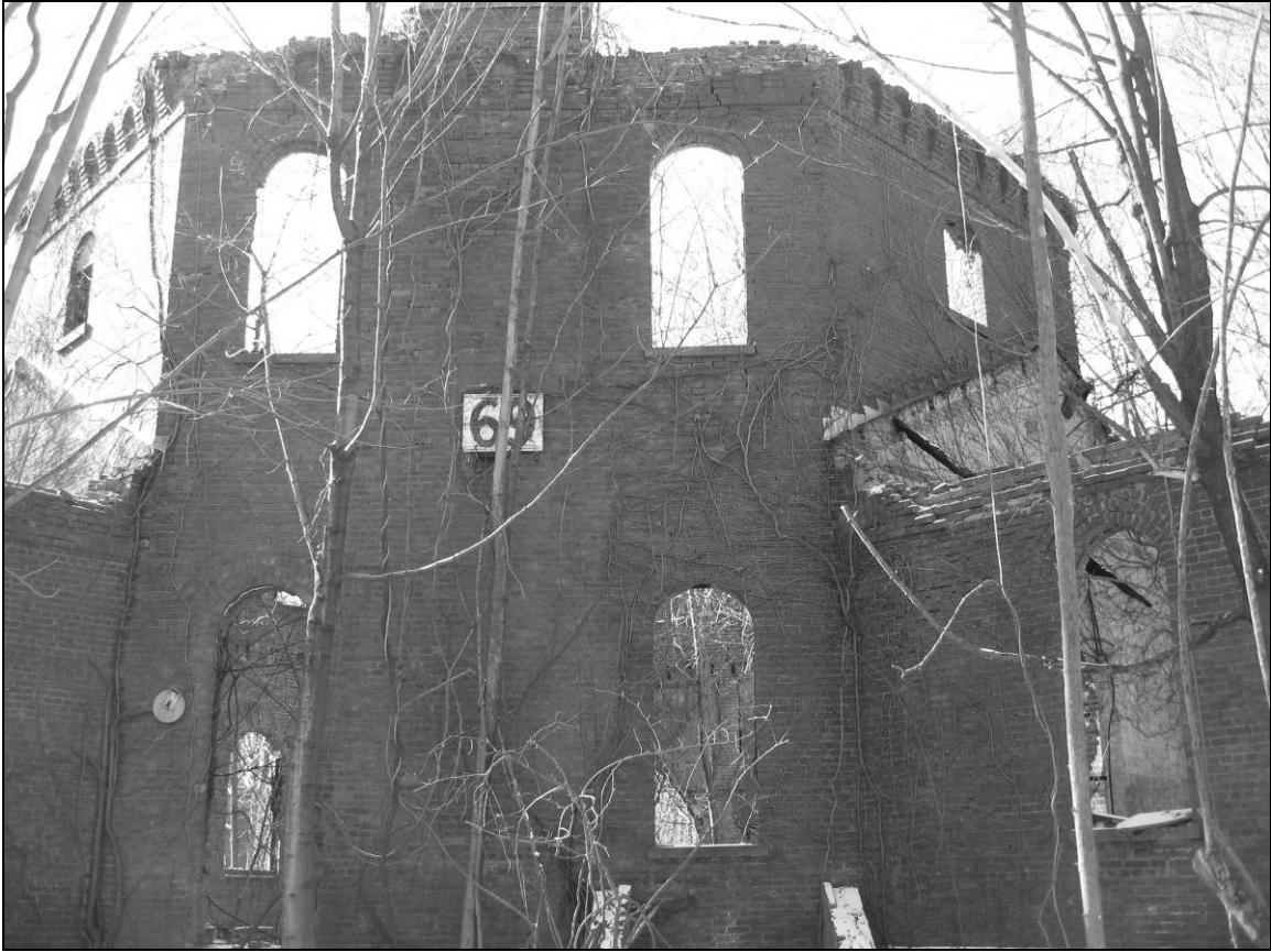
Photo 8. Back (northeastern façade) of tower, facing southwest.
