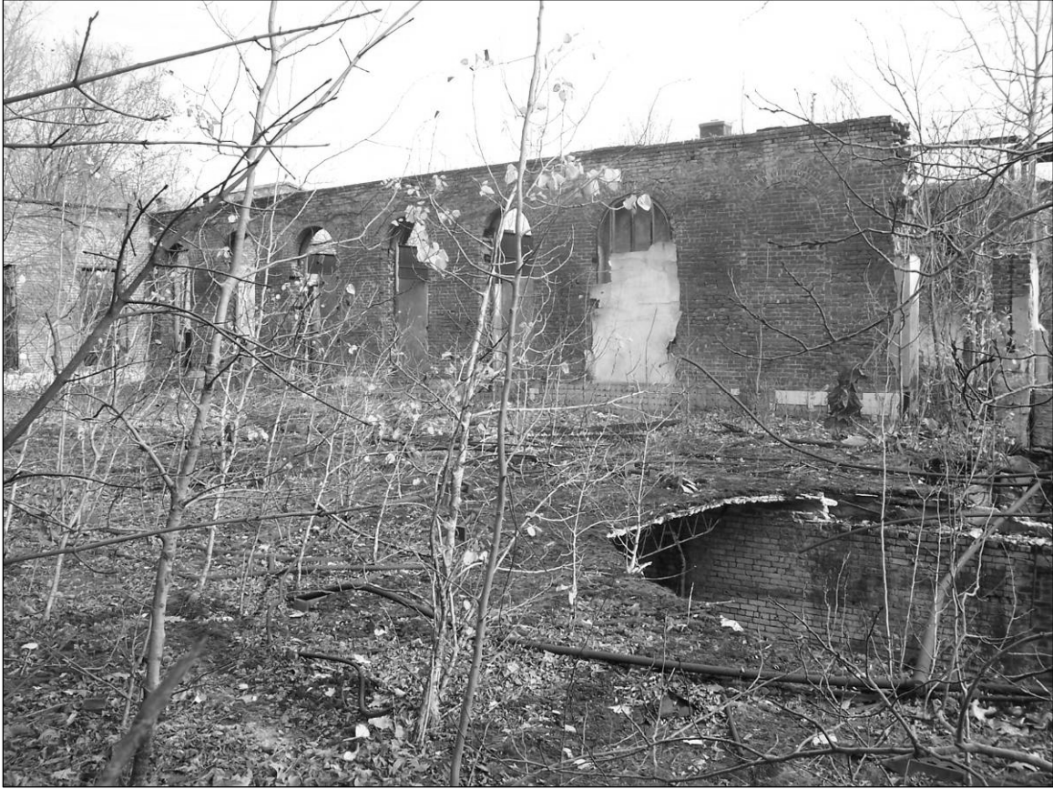
Photo 7. Interior—original dining hall section, looking northeast.
