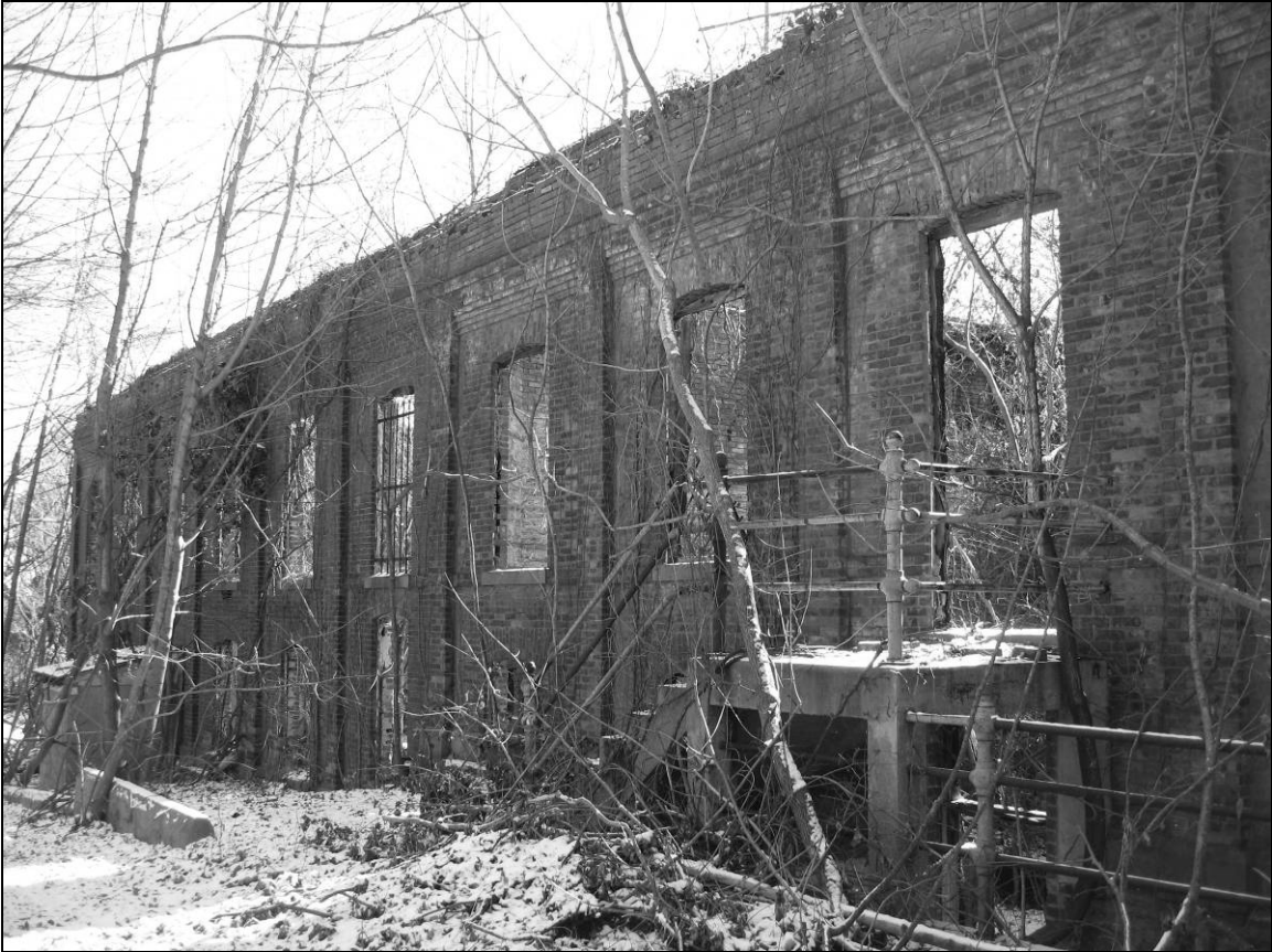
Photo 7. Northern façade, facing south.
