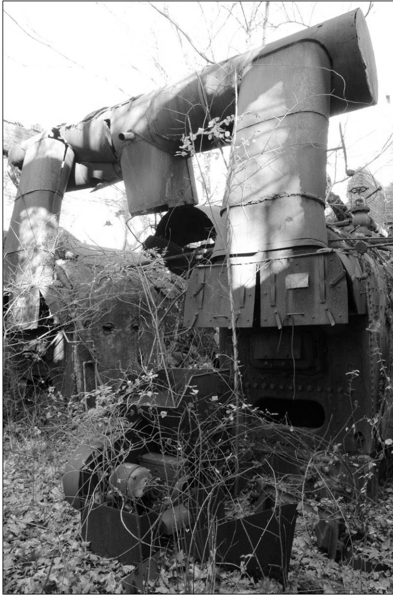
Photo 9. Interior—boiler room, looking north-northwest.
