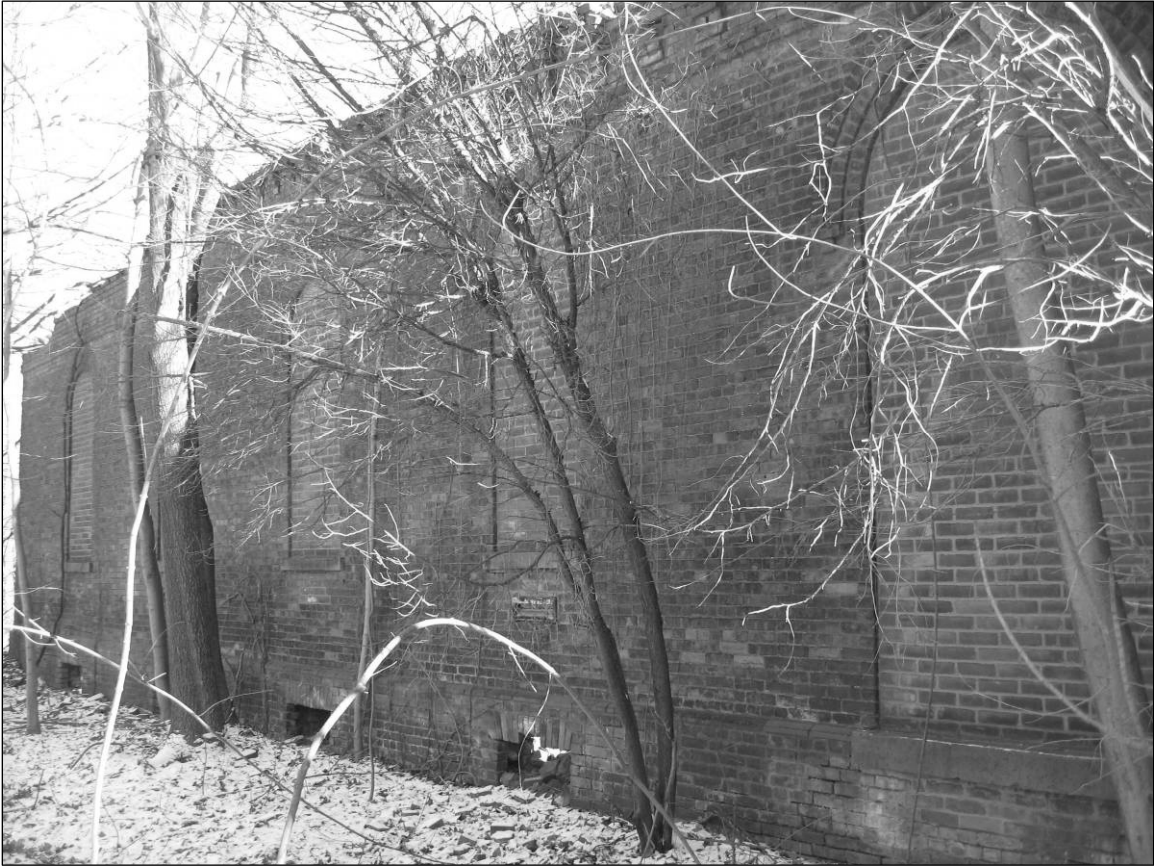
Photo 5. Western façade, north wing showing bricked-up window openings, facing northeast.
