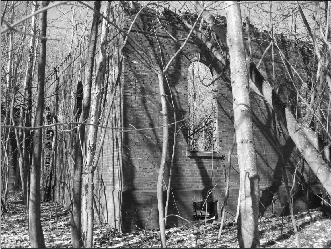
Photo 10. Eastern and southern façades of south dormitory dependency, facing west-northwest.
