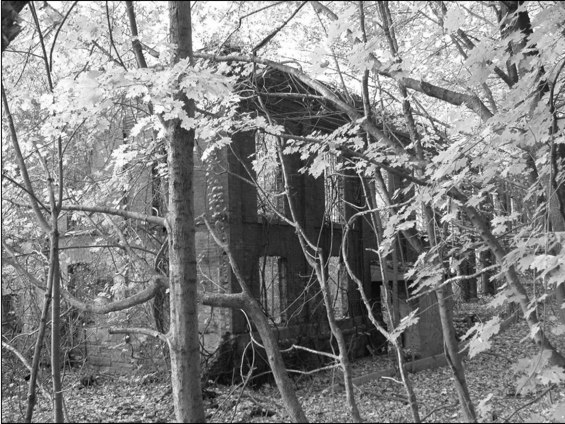
Photo 1. Northern façade, facing southwest.
