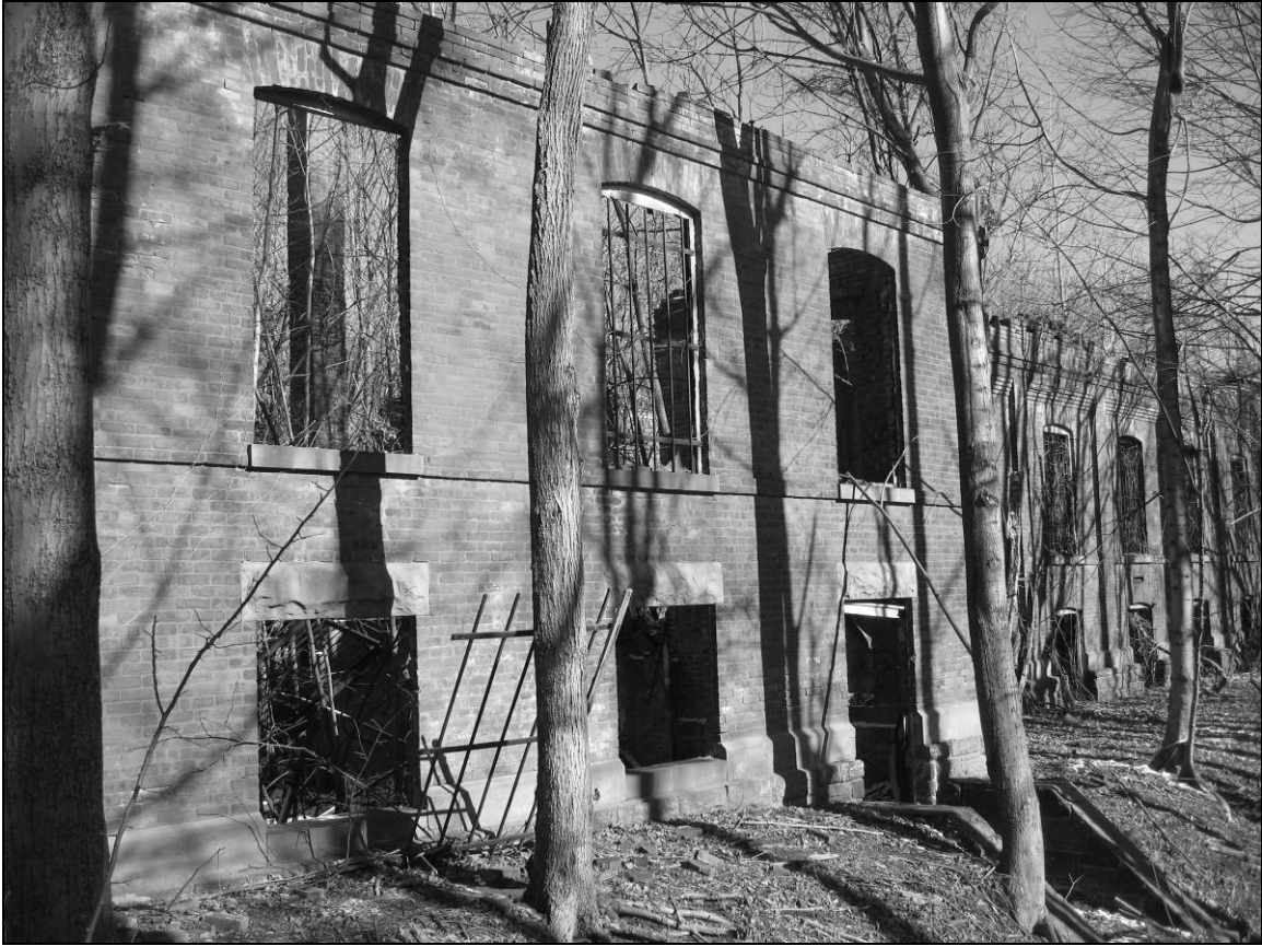
Photo 9. Southern façade, facing northeast.
