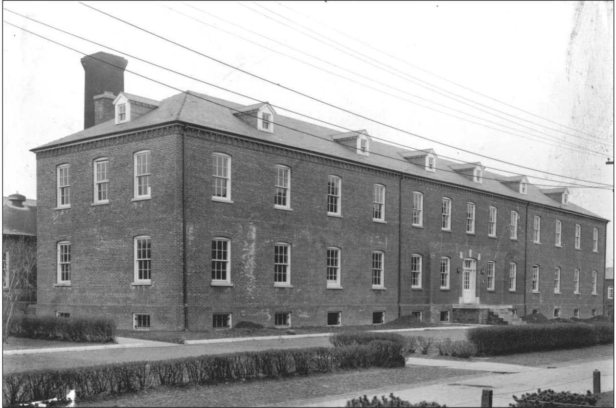
Figure 5. Inventory photograph, October 1940. Record Group 77, National Archives, College Park, MD.
