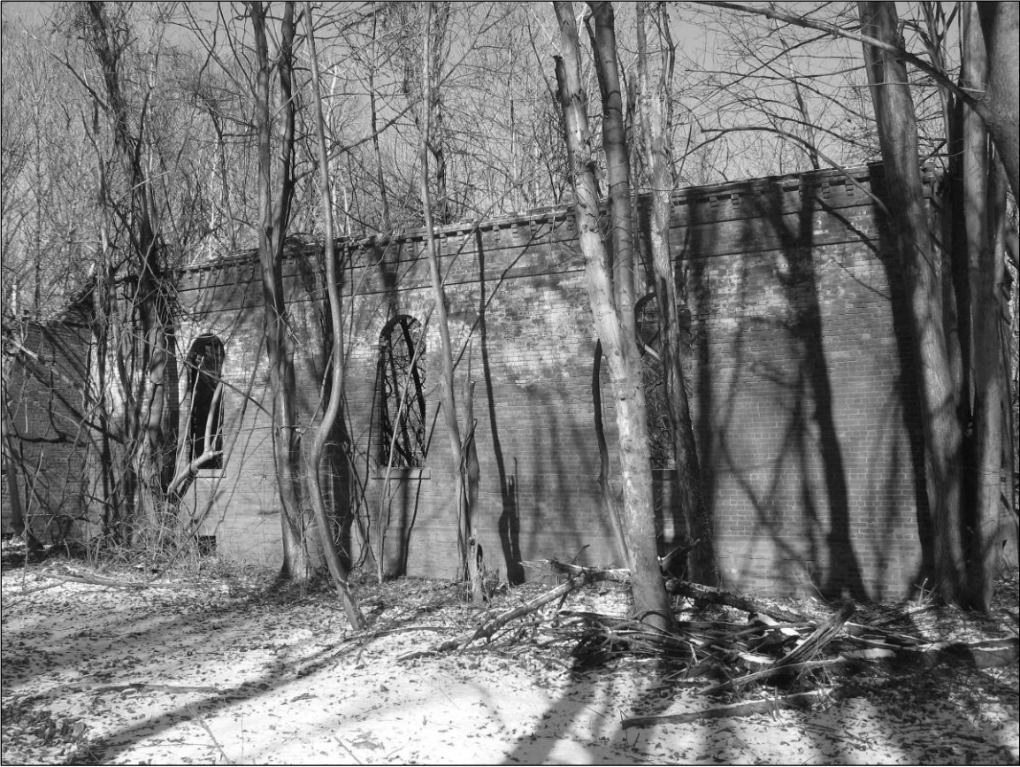
Photo 9. Southern façade of south dormitory dependency, facing northwest.
