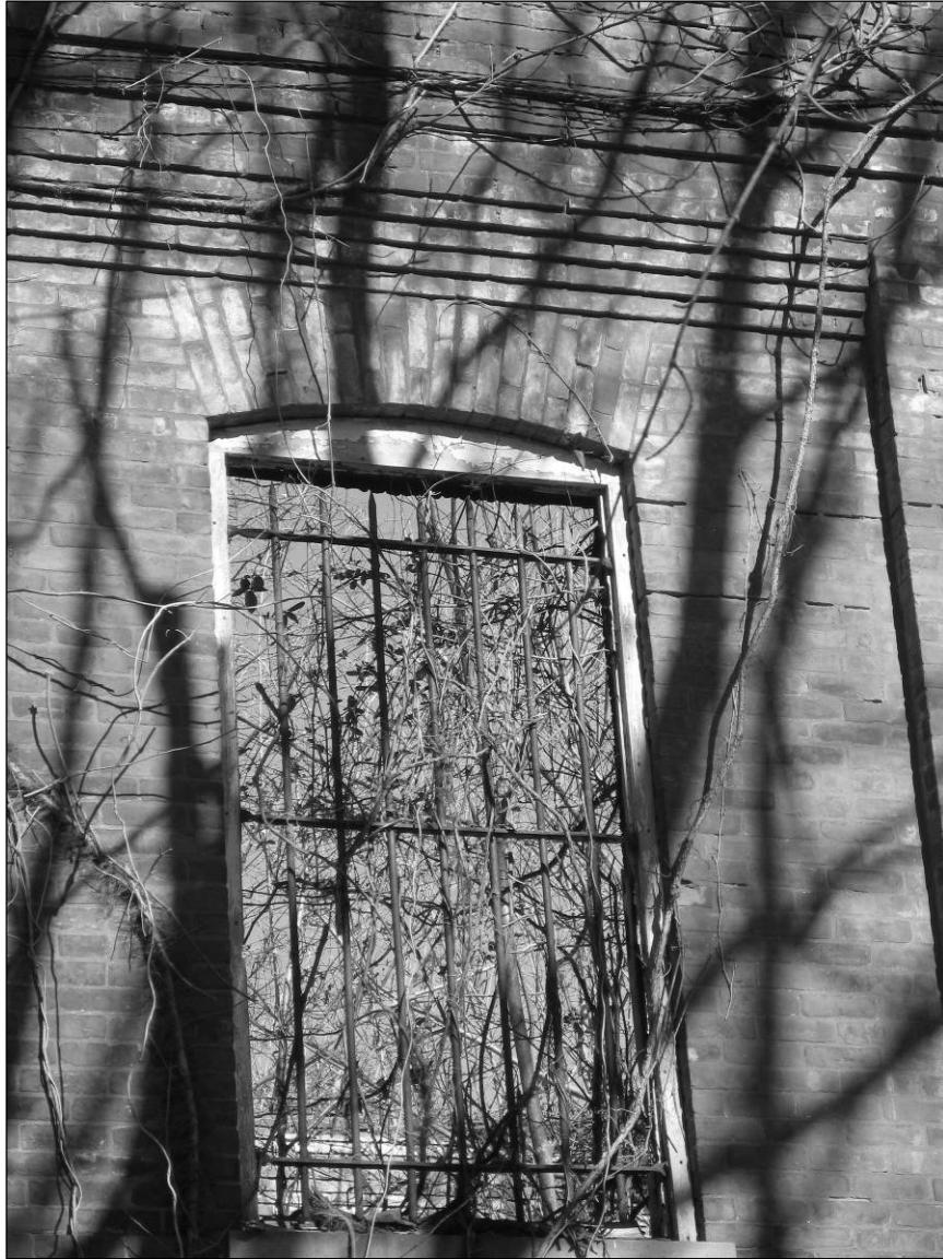
Photo 10. Southern façade, detail.
