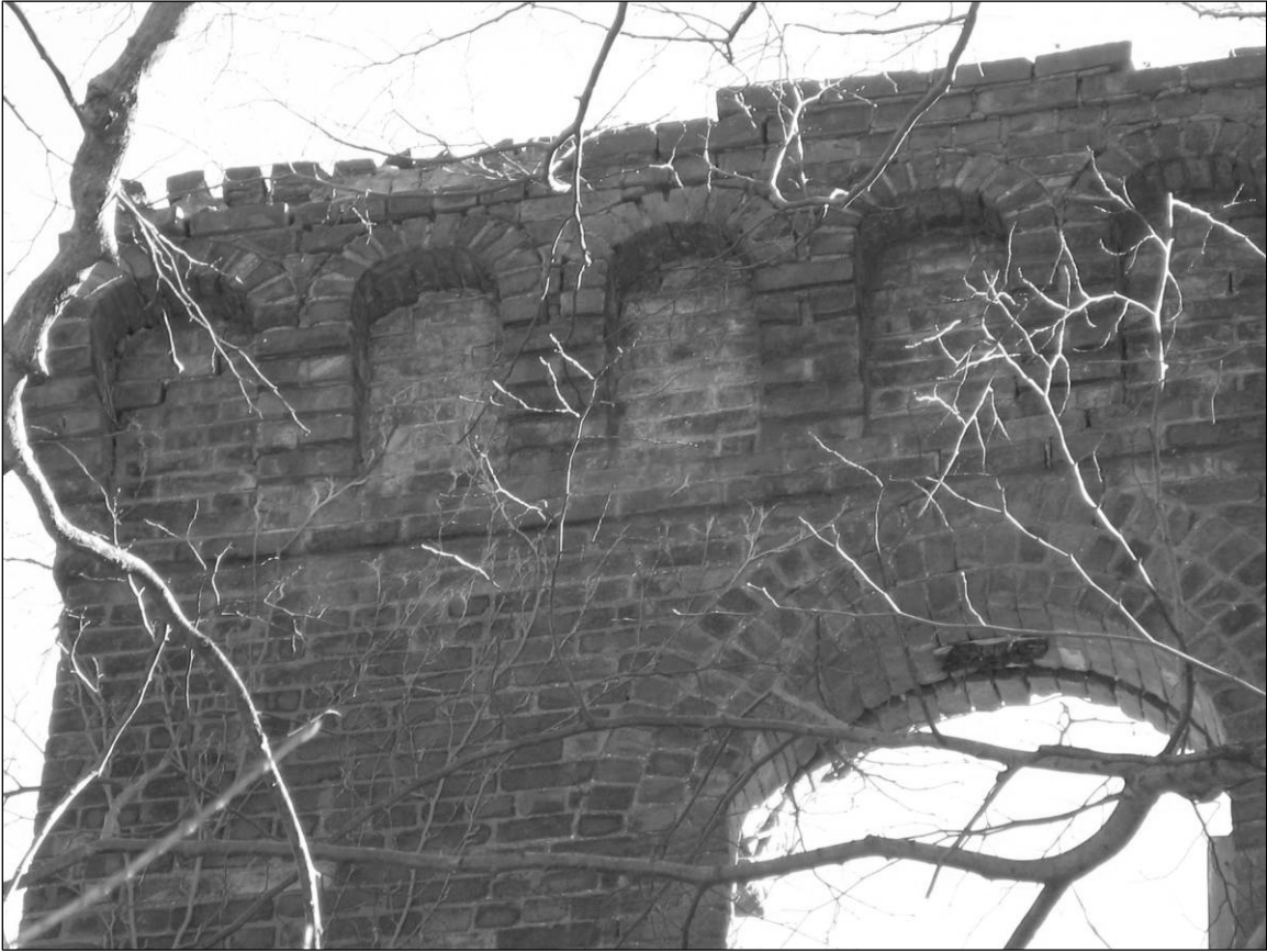
Photo 4. Western façade, center tower, detail—blind arcade (Lombard band) cornice.
