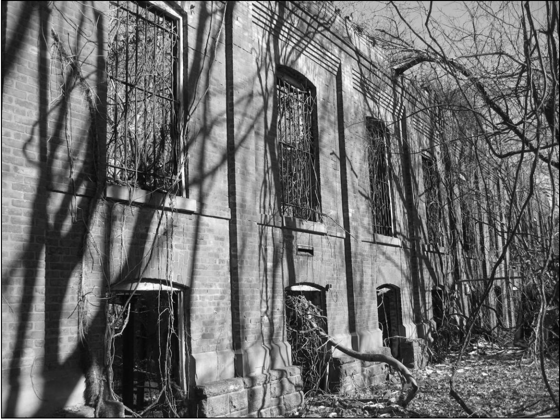
Photo 11. Southern façade, facing north.
