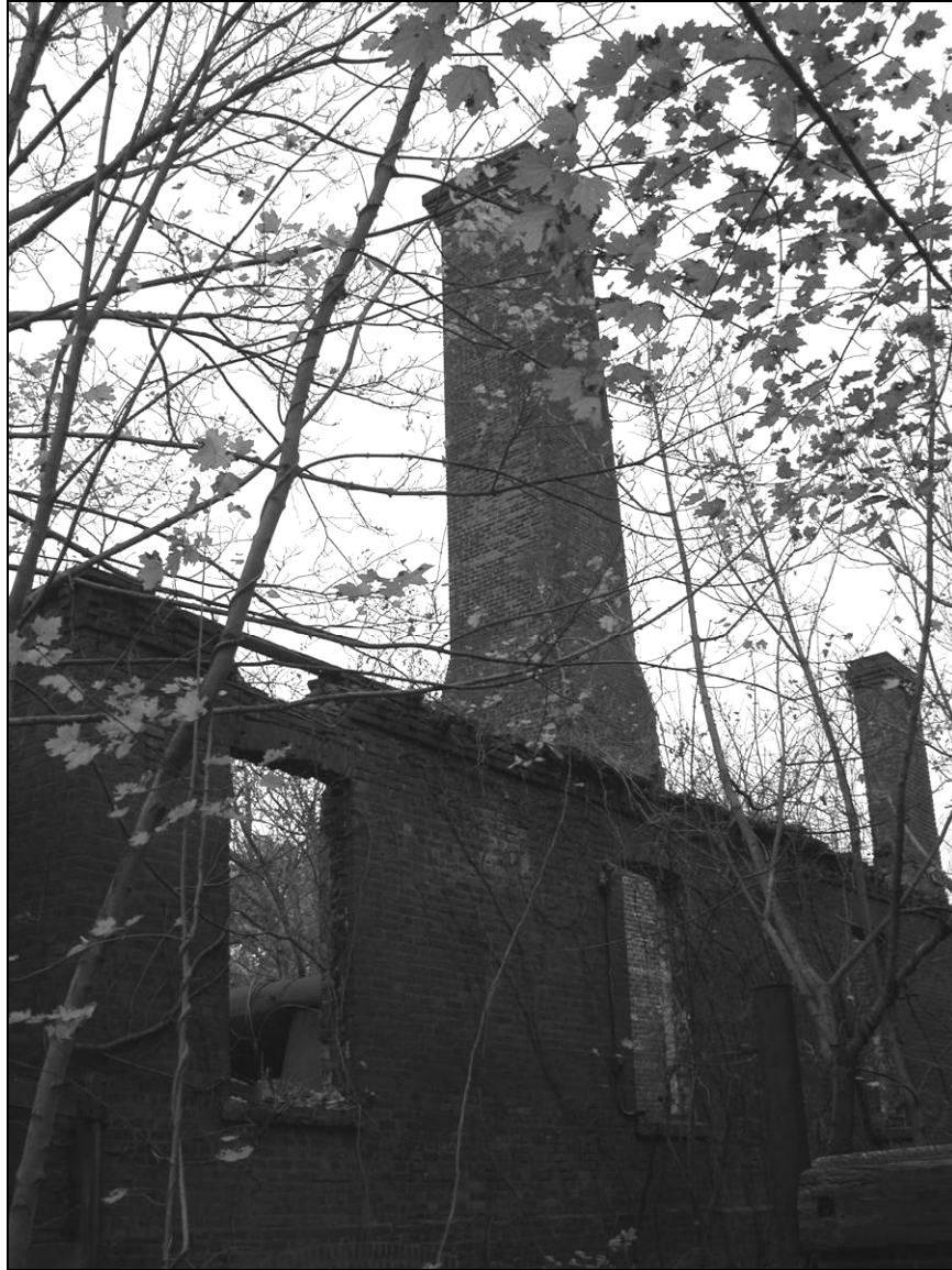
Photo 5. Eastern façade at southeastern corner, showing chimneys. View northwest.
