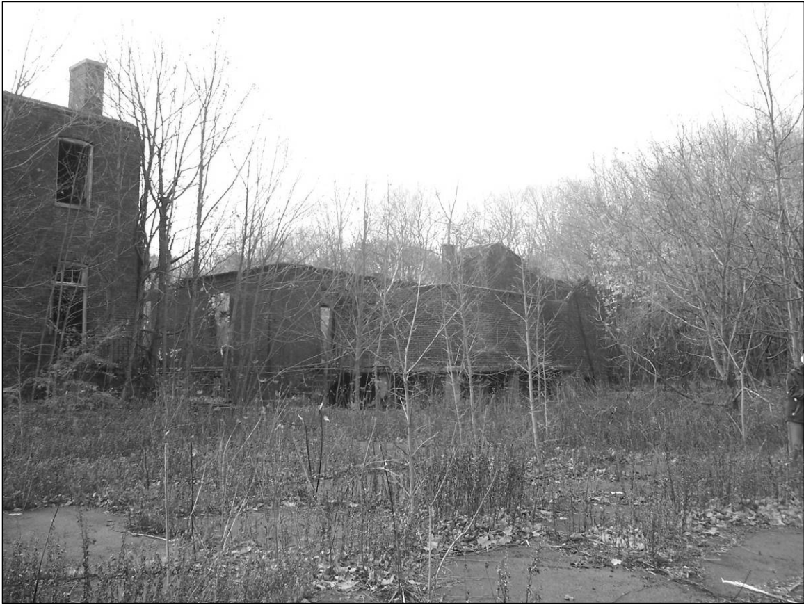
Photo 6. Northeastern side of Building 67 (right) and adjoining Building 65 (left) looking southwest.
