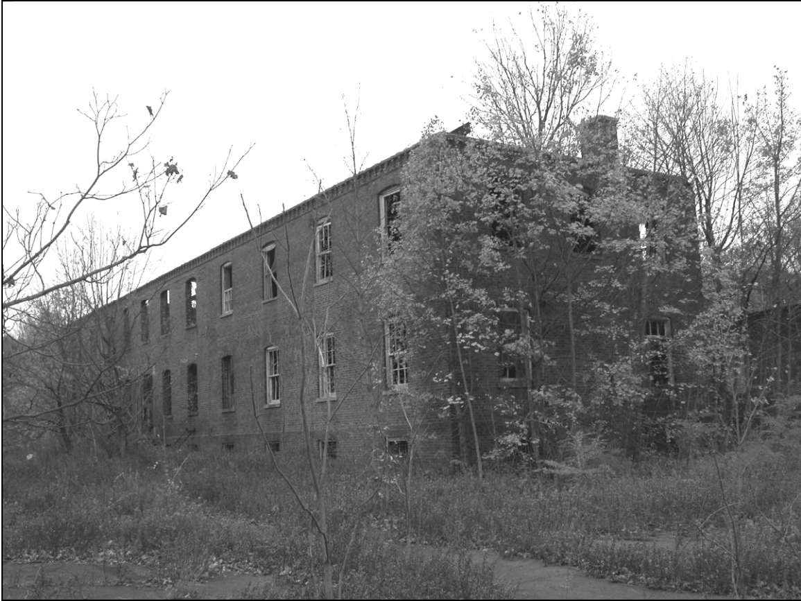
Photo 4. Eastern façade, facing southwest.
