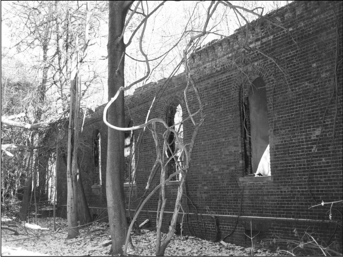
Photo 14. Western façade of north wing, facing northeast.
