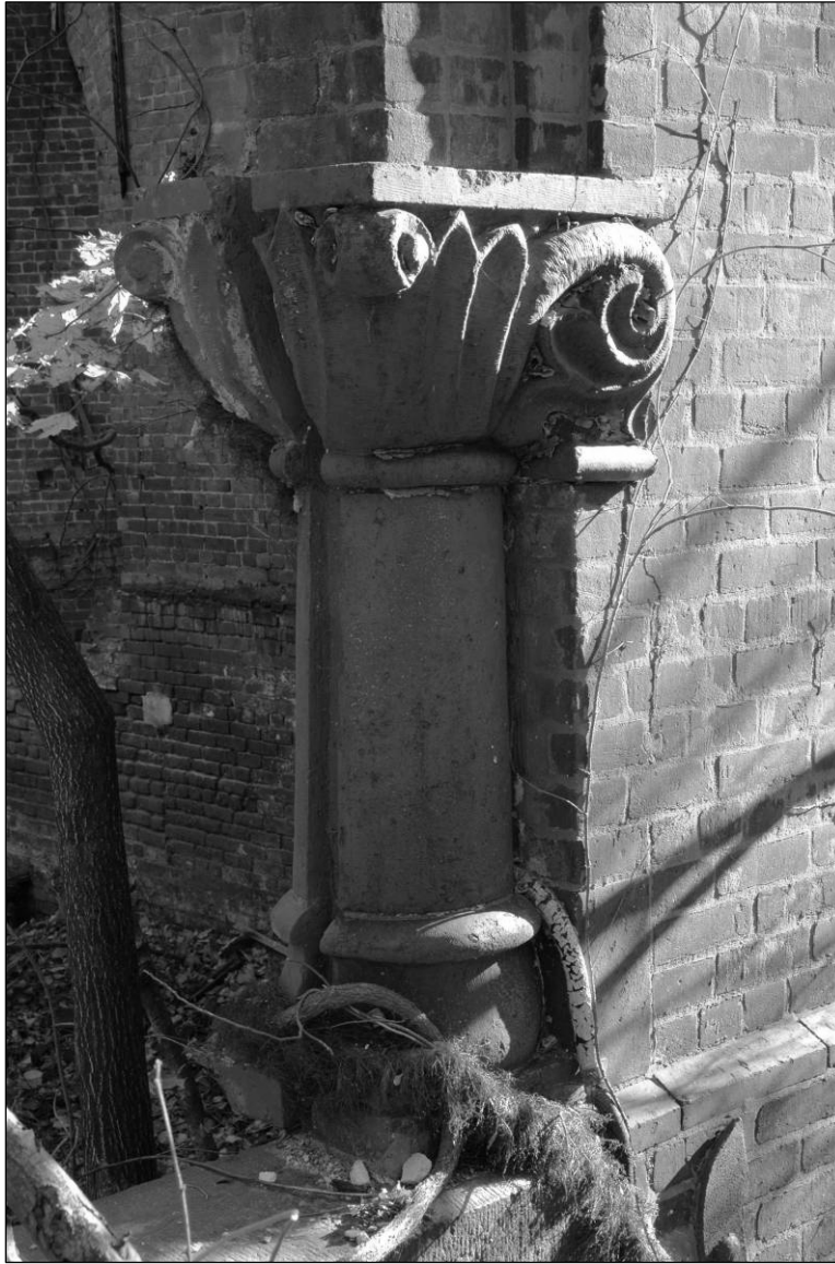
Photo 2. Detail of entrance in southwestern façade of center tower, showing engaged dwarf terracotta column.
