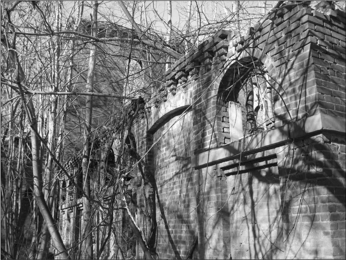
Photo 12. Southern façade of rear lavatory block with center tower in background, facing west-northwest.
