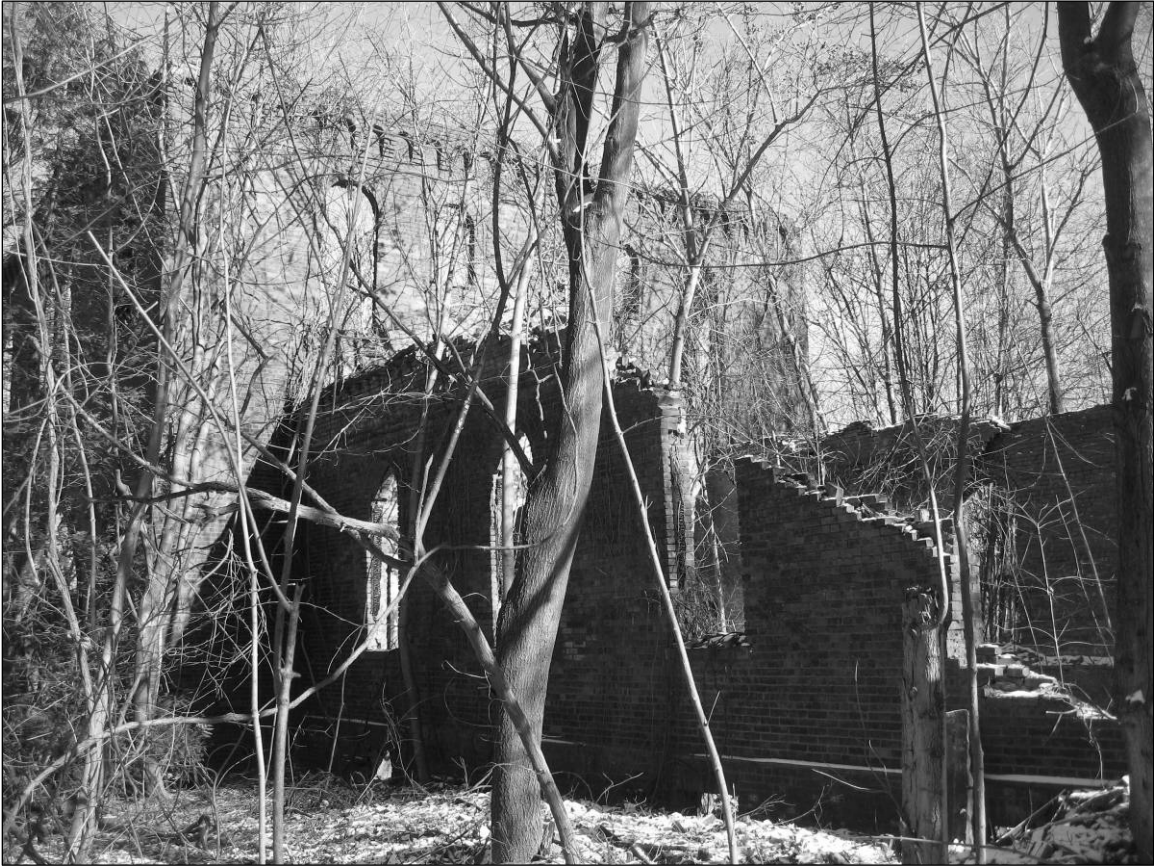
Photo 6. Western façade, south wing and center tower, facing northeast.
