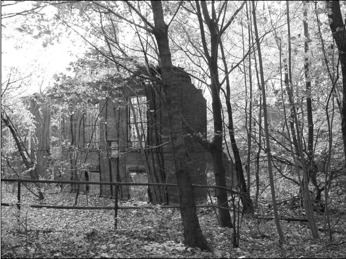
Photo 5. Northern façade, facing southeast.
