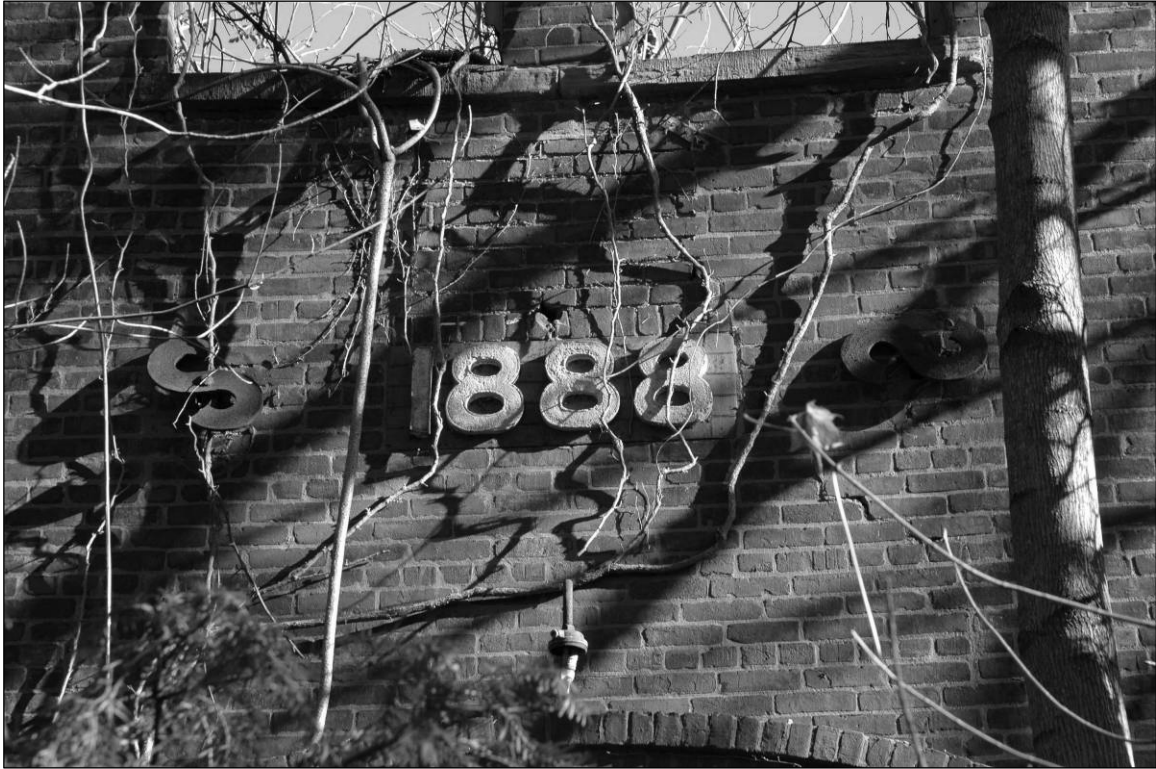
Photo 3. Southwestern façade of center tower, detail—terracotta plaque with building date.
