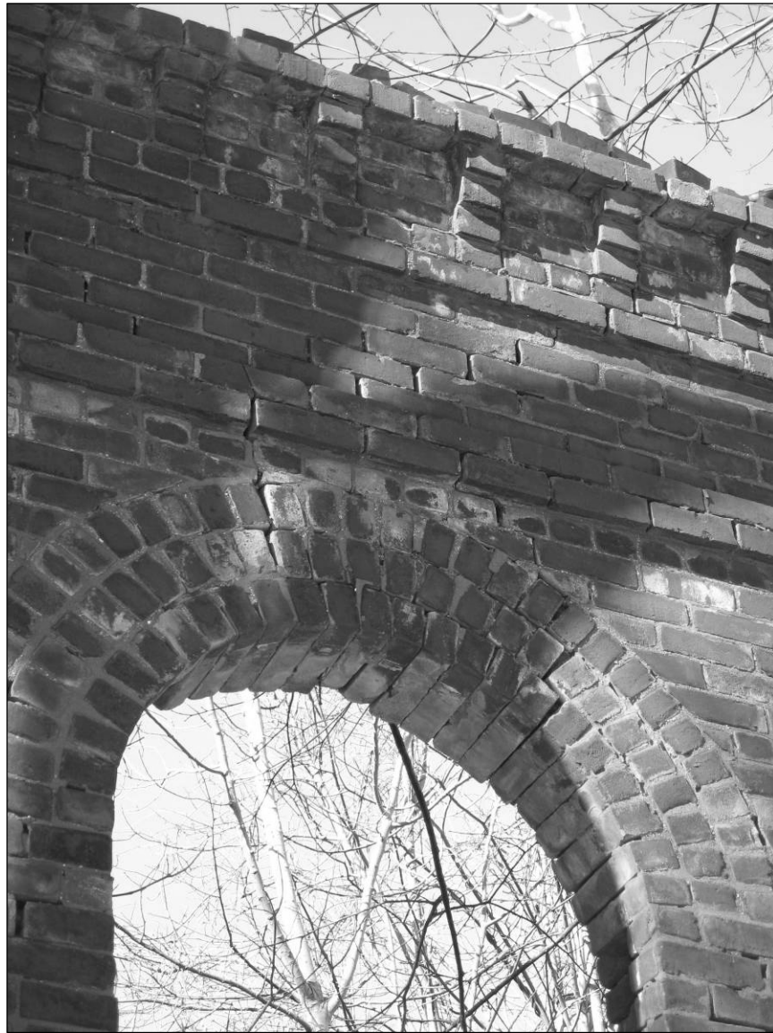
Photo 11. South dormitory dependency, eastern wall, detail—brick semicircular arch window opening and brickwork cornice of machicolations.
