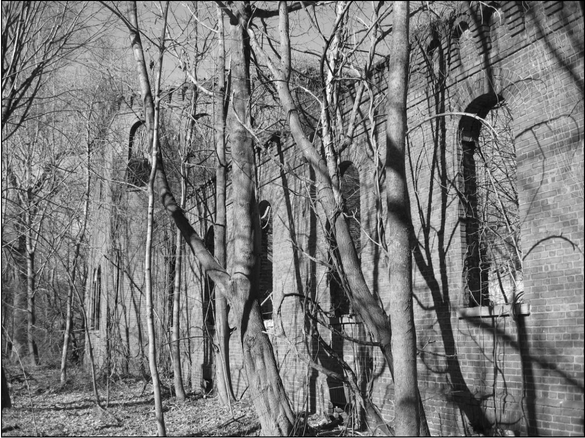
Photo 12. Southern façade of east wing, facing west.
