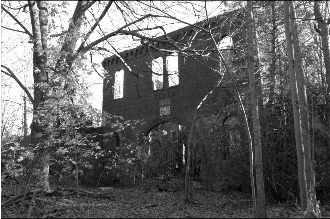
Photo 1. Western façade, center tower, facing northeast.
