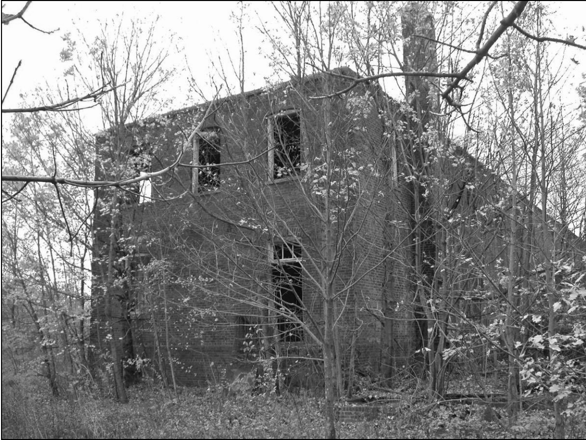
Photo 6. Northern façade, facing southeast.
