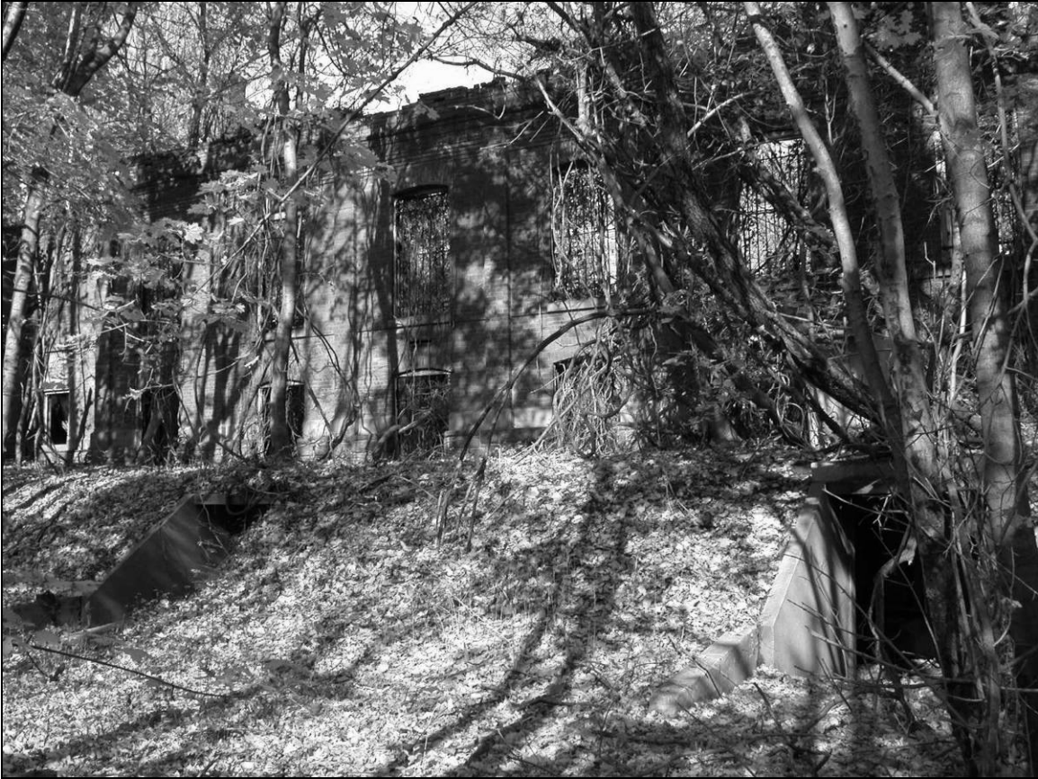
Photo 2. Southern façade, facing north.
