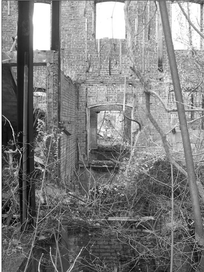
Photo 9. Collapsed interior of ca. 1909 center section, facing west.
