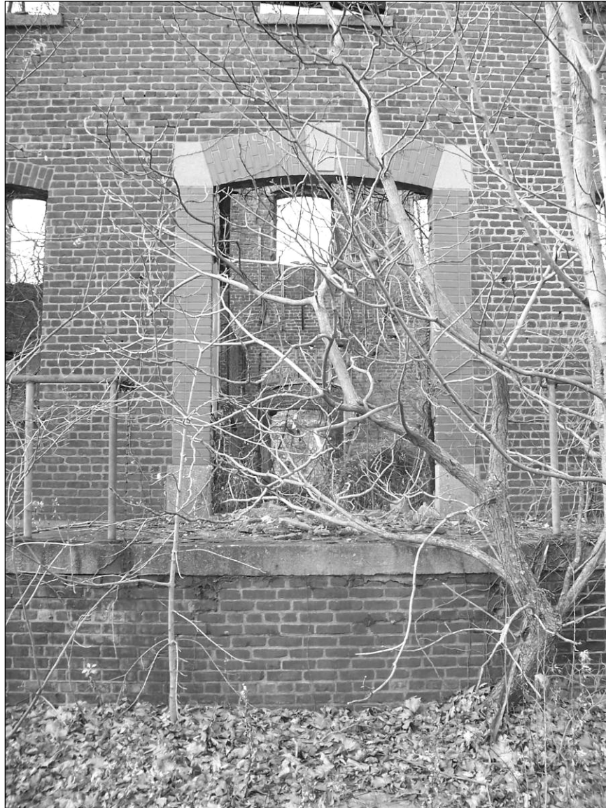
Photo 3. Eastern façade, detail—main entrance facing west.
