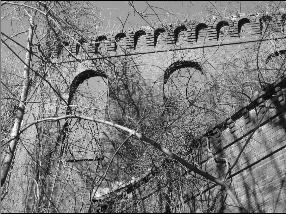
Photo 13. Cornices of southeastern façade of tower (above) and southern façade of east wing (below), facing northwest.
