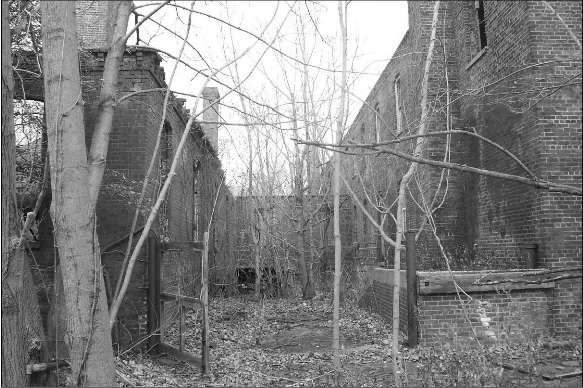
Photo 8. Southern courtyard between Building 65 (right) and Building 67 (left).
