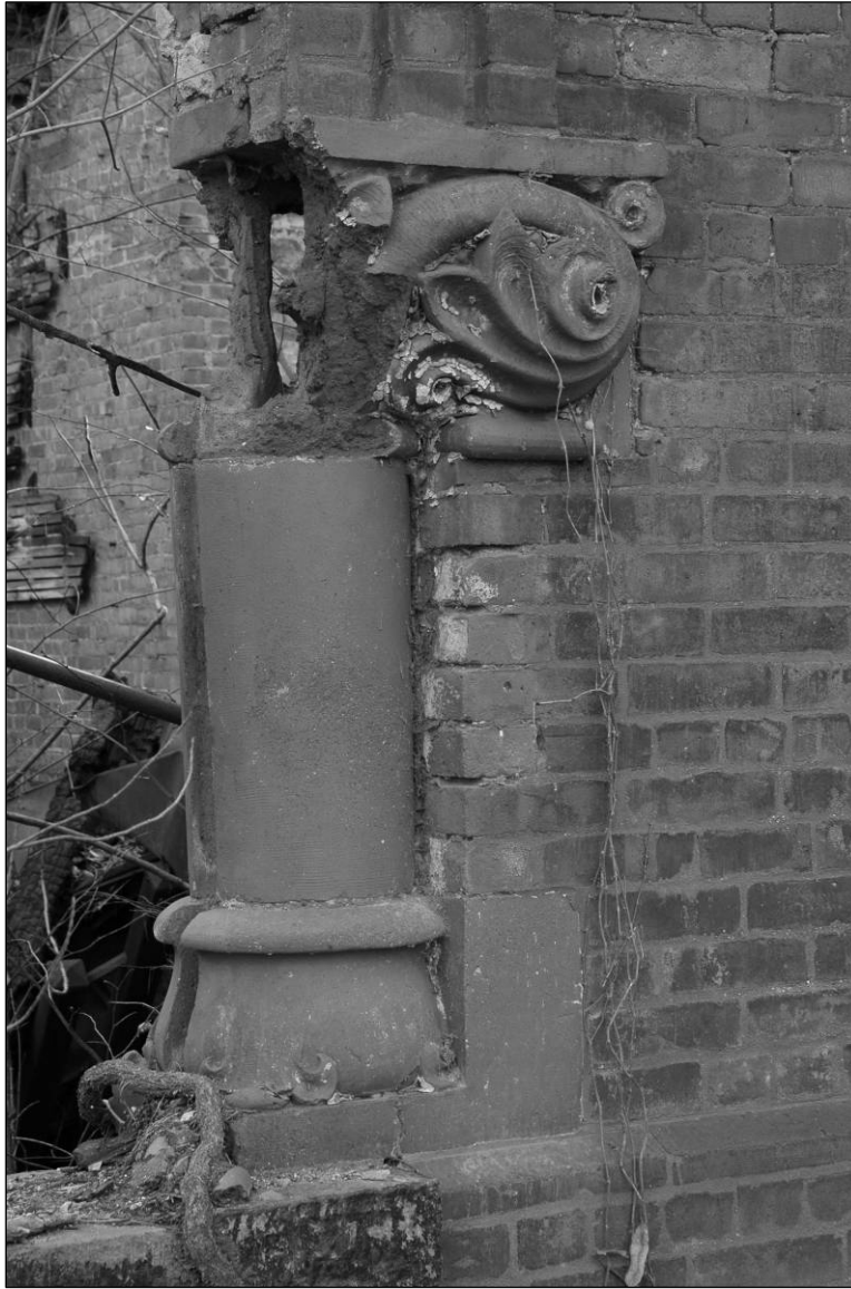
Photo 2. Western façade, center tower, detail—decorative engaged column of terracotta on south side of main entrance.
