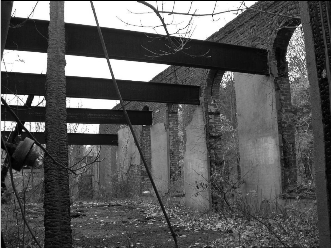
Photo 8. Interior—former courtyard between dining hall and kitchen wings, looking south-southwest.
