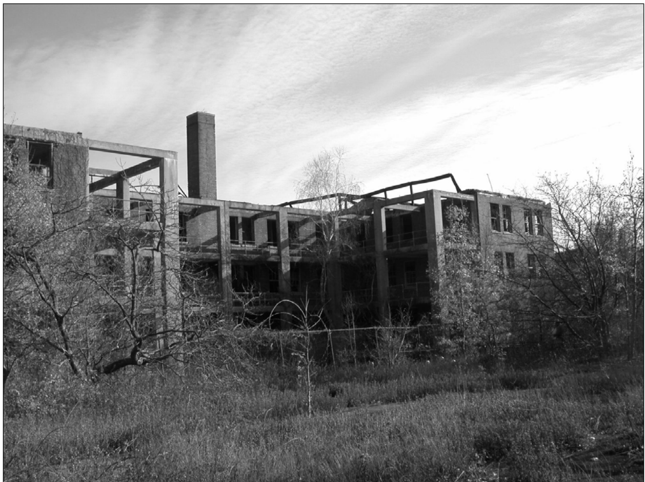
Photo 9. Western façade, facing southeast.
