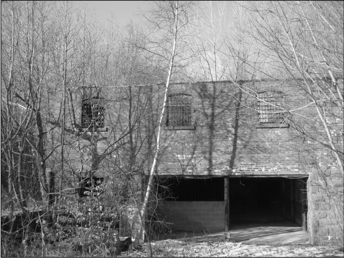
Photo 7. South end of eastern façade, facing west.
