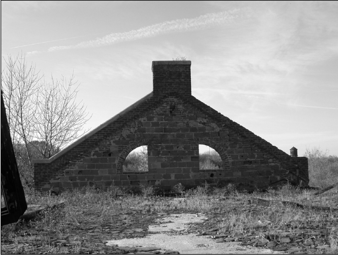
Photo 3. Parapetted brick gable end on north ell, interior view, looking west.
