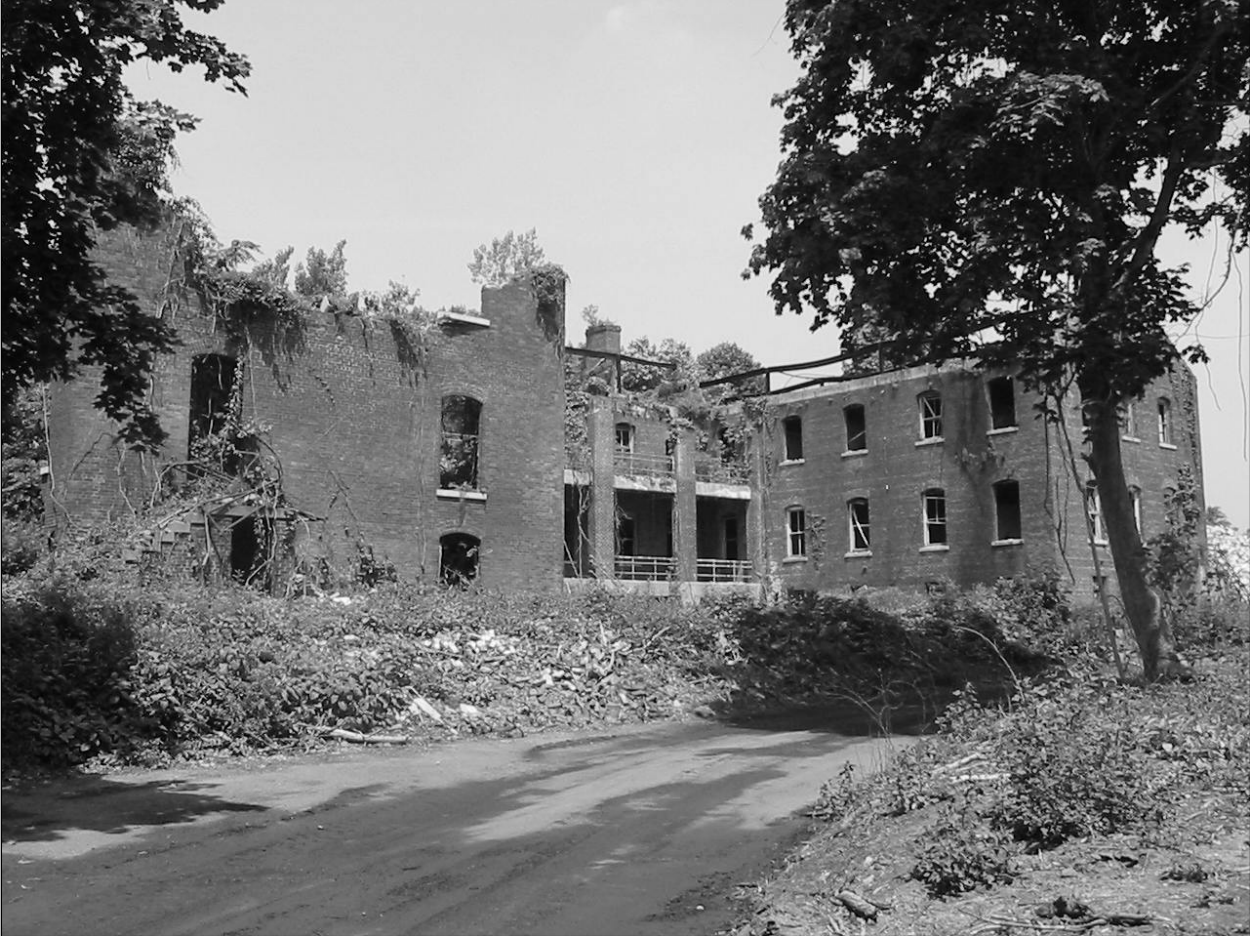
Photo 6. Rear of building, after removal of vegetation and shortly before demolition, facing northwest.
