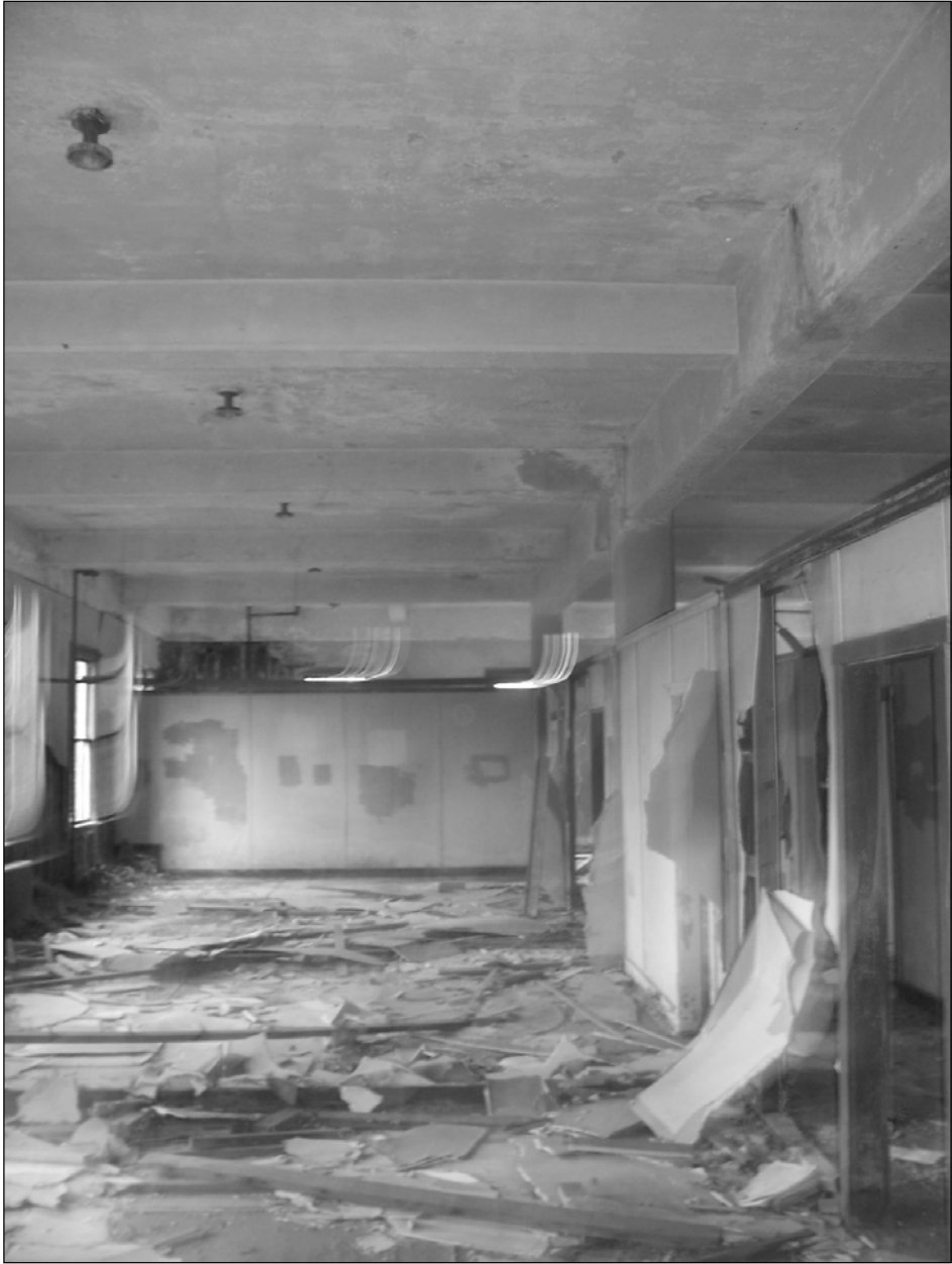
Photo 11. Interior, north half of building, showing room and corridor.
