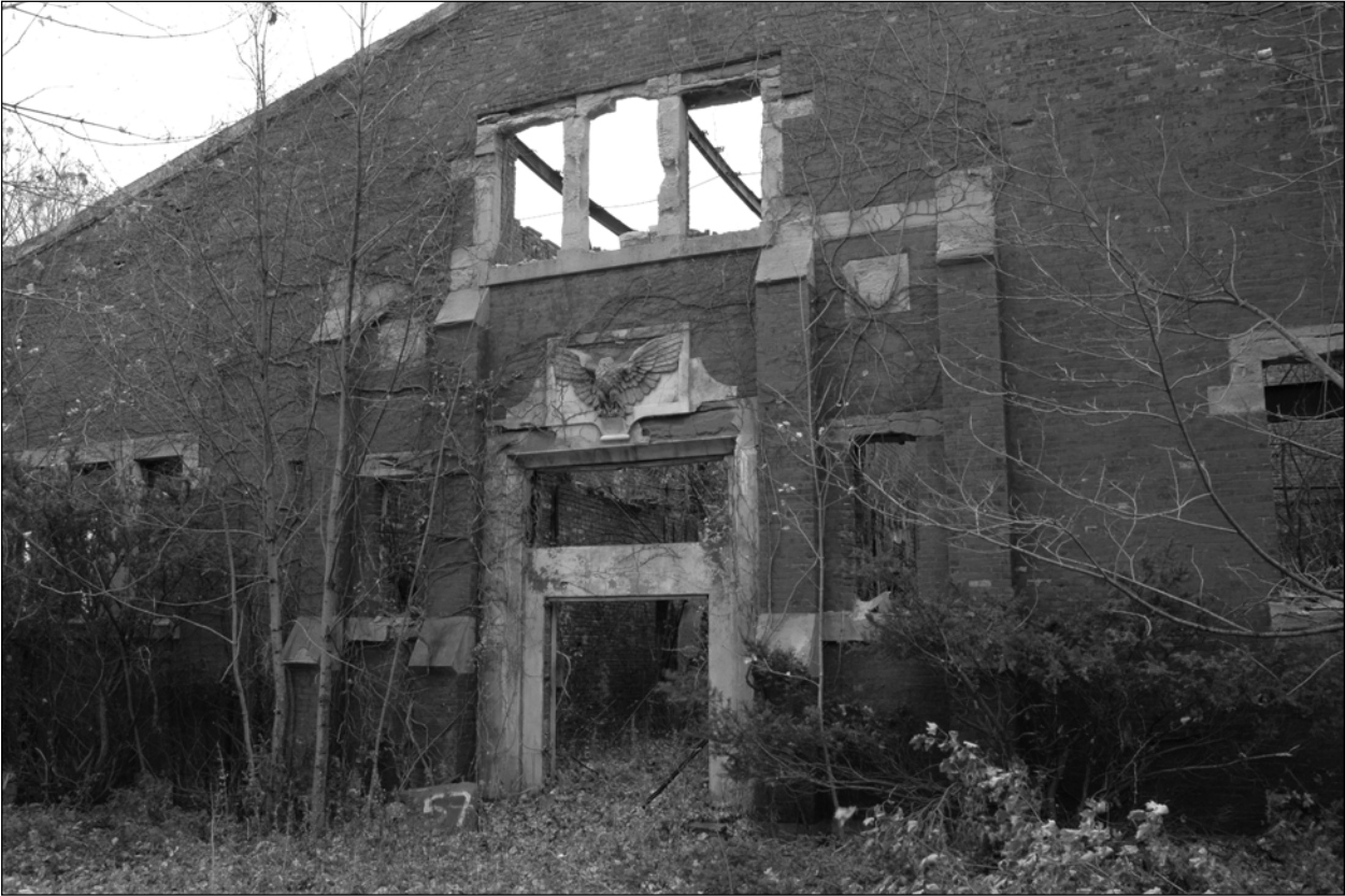
Photo 2. Western façade, detail of frontispiece surrounding main entrance, facing east.
