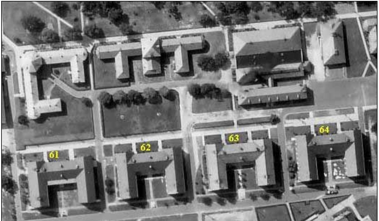
Figure 7. Vertical aerial photograph, September 1940, detail showing Buildings 61-64. North is to right. Numbers have been added to this reproduction to identify the buildings. Original in National Archives, College Park, MD; digital copy from Fort Slocum Alumni and Friends Collection, Michael A. Cavanaugh, Los Angeles, CA, custodian.
