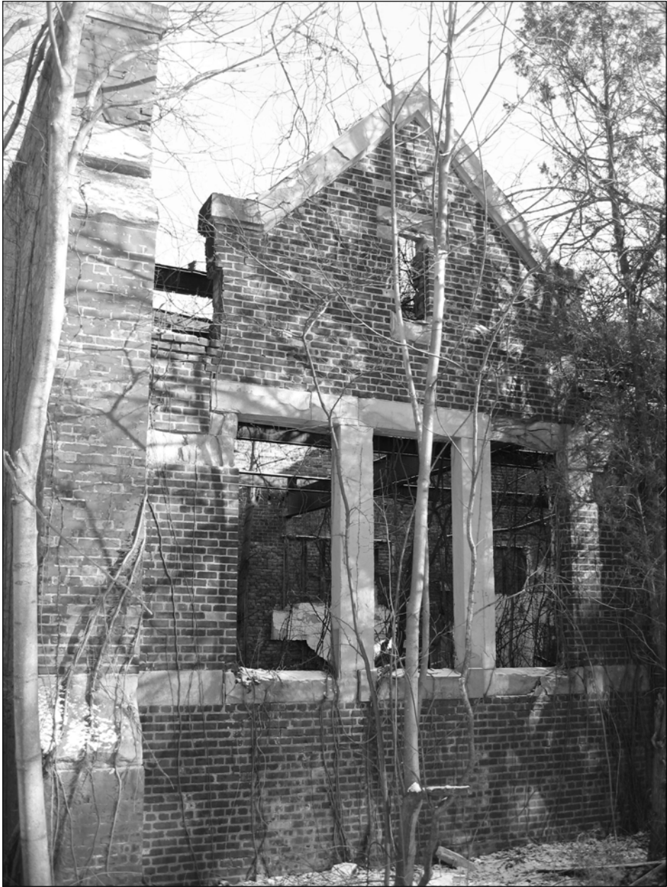
Photo 5. Southern façade, detail of wall dormer at western end, facing north.
