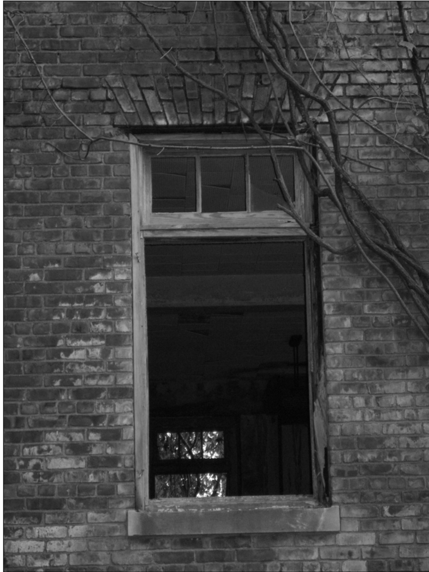
Photo 9. Façade detail: window opening.
