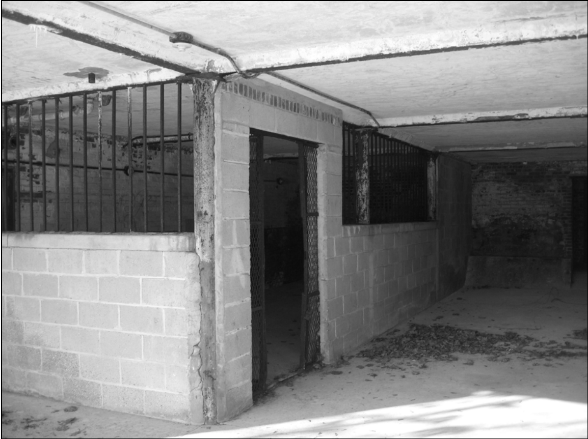
Photo 9. Vehicle bay interior, facing west-southwest.
