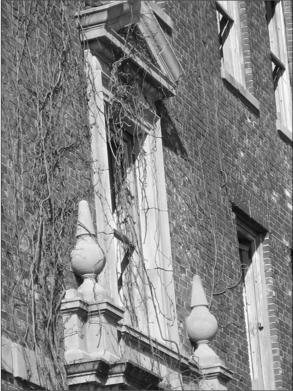
Photo 7. Eastern façade, detail: second-story window over main entrance, facing northwest.
