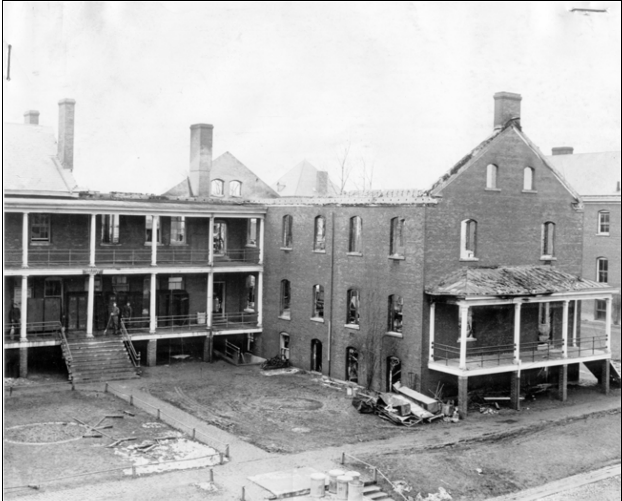
Figure 5. Building 61 after fire of January 20, 1937, illustrating destruction of north wing, as seen from rear of building. View northwest. The damaged wing was demolished and entirely rebuilt in 1939. Record Group 77, National Archives, College Park, MD.
