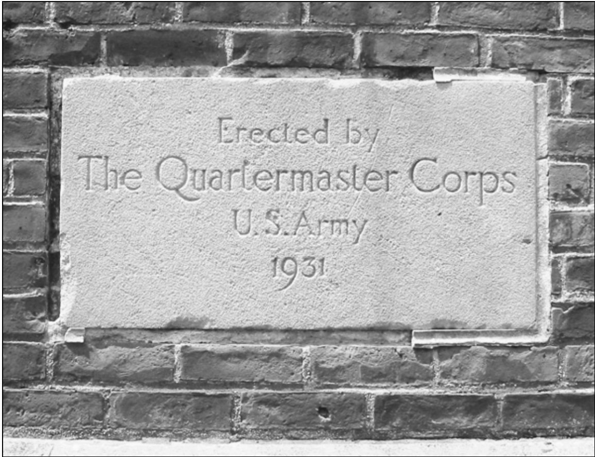
Photo 3. East façade, detail: date stone at southeastern corner.
