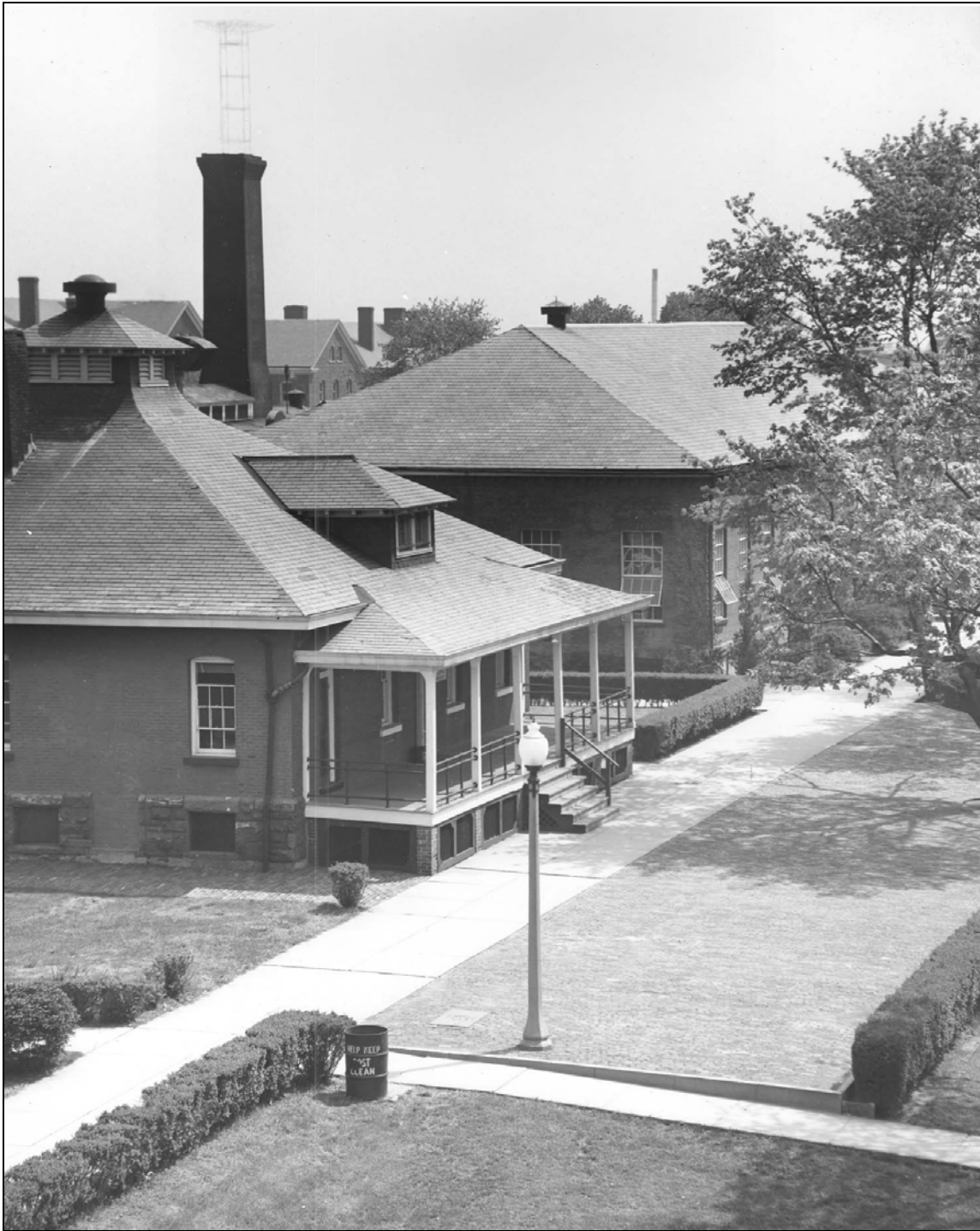
Figure 7. Barracks Area, ca. 1950. Guardhouse is the building in foreground with porch. View southeast. Fort Slocum Collection, New Rochelle Public Library, New Rochelle, NY.
