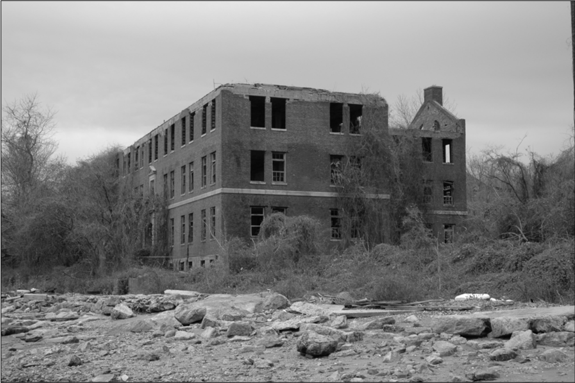
Photo 2. Northern end of building, facing southwest.
