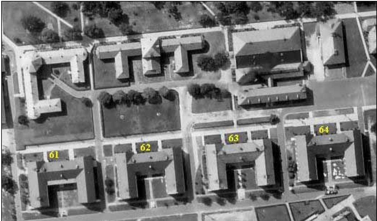
Figure 6. Vertical aerial photograph, September 1940, detail showing Buildings 61-64. North is to right. Numbers have been added to this reproduction to identify the buildings. Original in National Archives, College Park, MD; digital copy from Fort Slocum Alumni and Friends Collection, Michael A. Cavanaugh, Los Angeles, CA, custodian.
