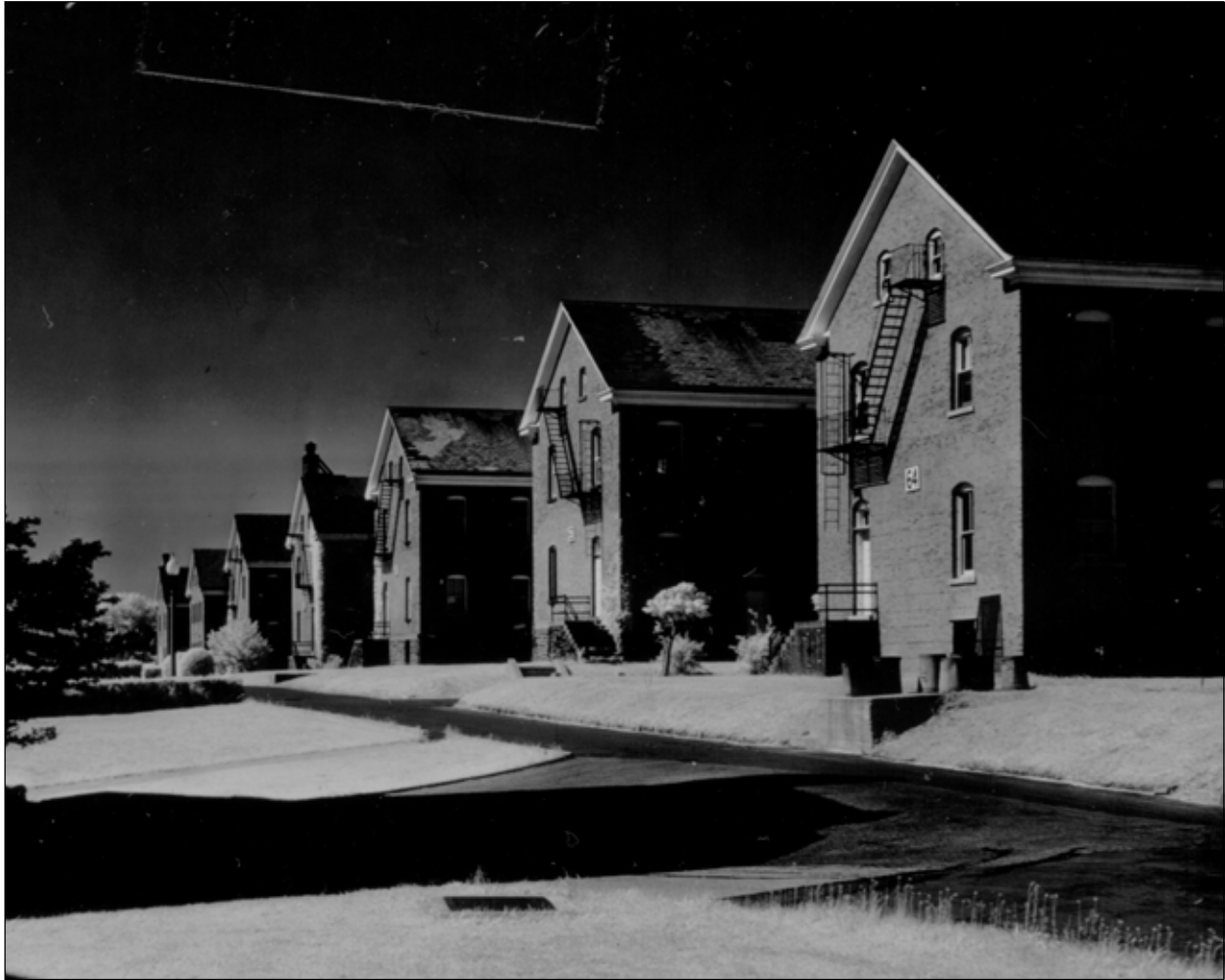
Figure 7. The rear gables of the Quadrivium, as seen from Douglass Drive in ca. 1958. View southwest. The first gable at right is at the eastern end of the south wing of Building 64. Record Group 111, National Archives, College Park, MD.
