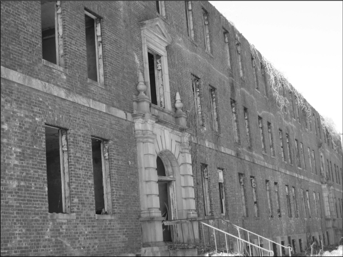
Photo 1. East façade, facing northwest.
