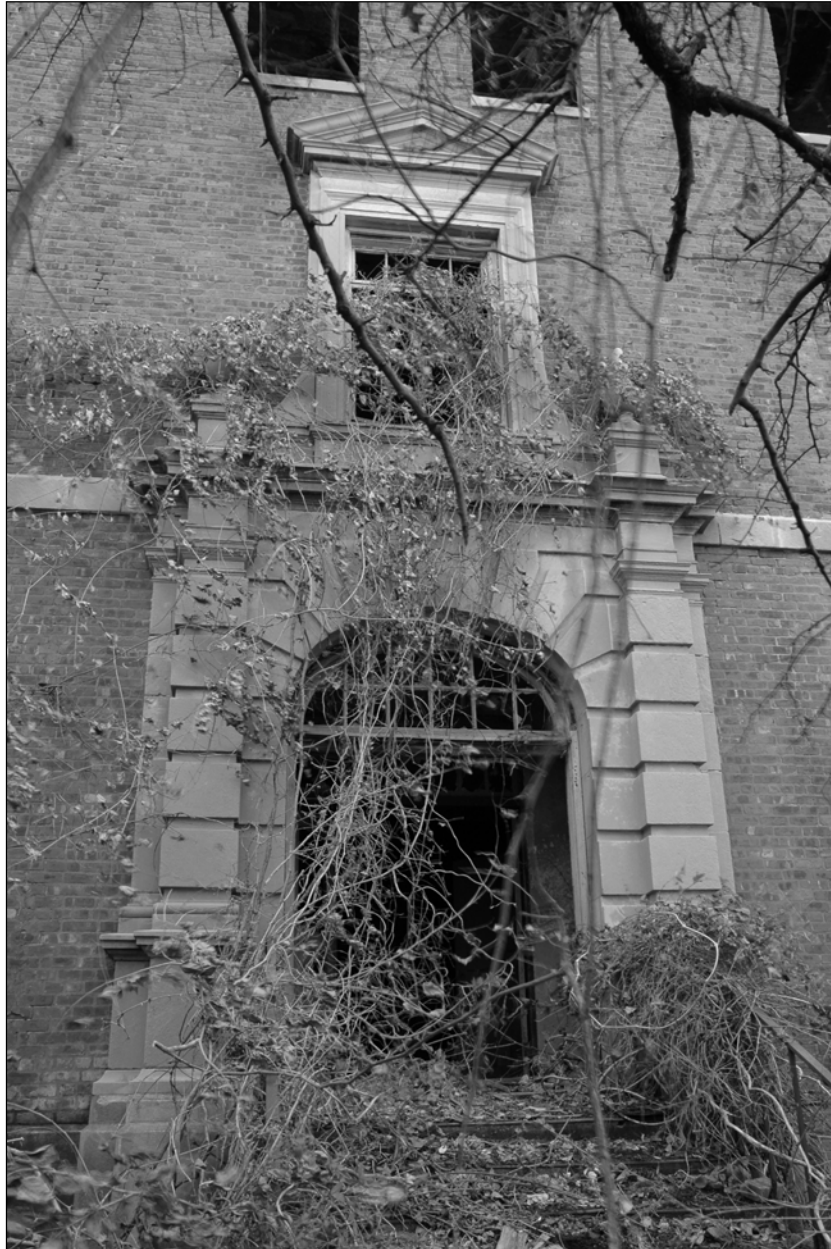
Photo 6. Eastern façade, detail: northern main entrance, facing west.
