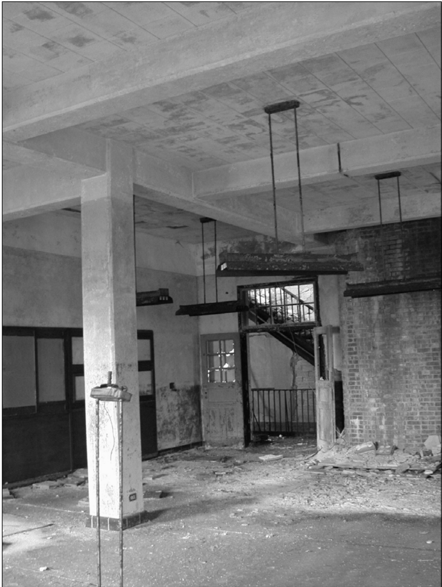
Photo 10. Interior, north half of building.
