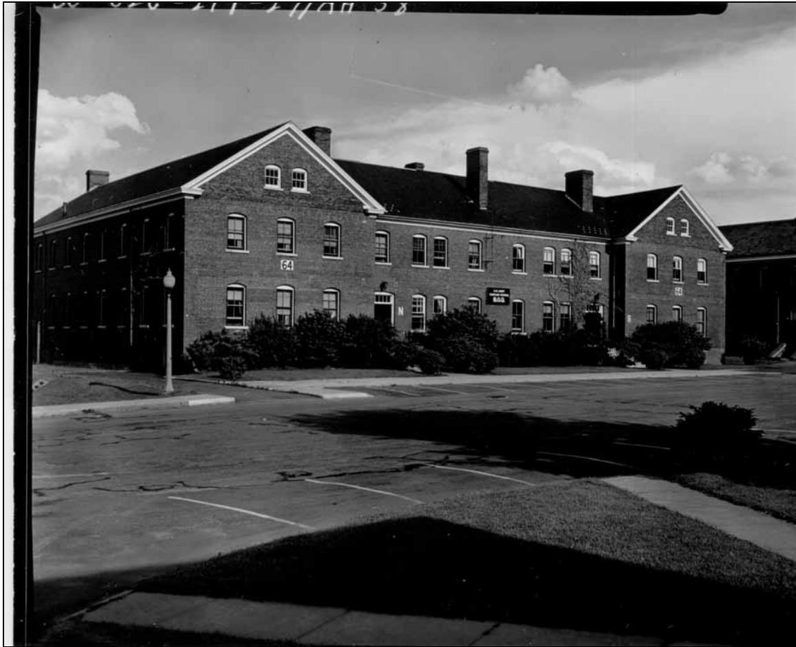
Figure 8. Exterior, Building 64, circa 1958. View southeast. Record Group 111, National Archives, College Park, MD.
