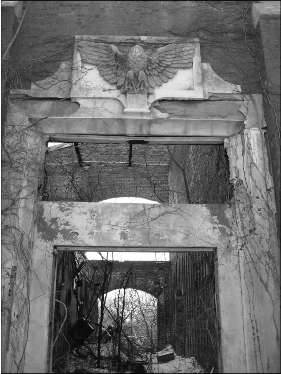
Photo 3. Western façade, detail of entrance with view into interior, facing east.
