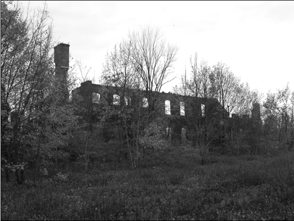
Photo 4. Western façade, facing southeast.
