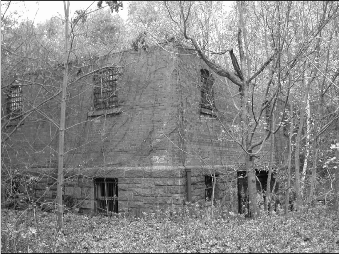
Photo 1. Southern and eastern façades, facing northwest.
