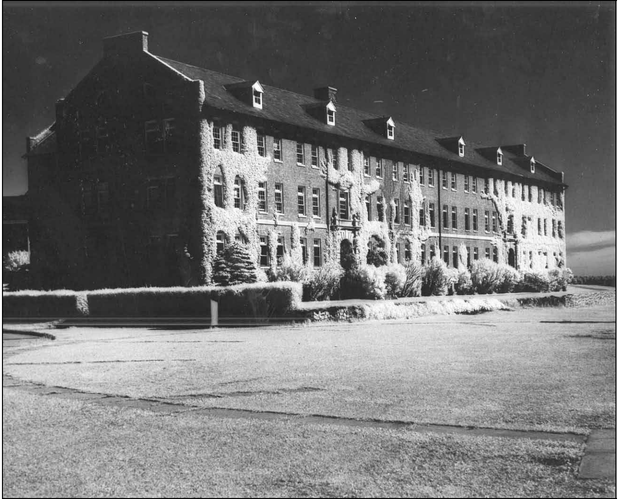
Figure 7. Inventory photo, circa 1950. View northwest. Fort Slocum Collection, New Rochelle Public Library, New Rochelle, NY.
