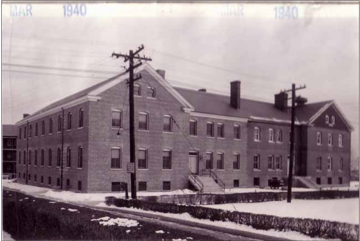
Figure 9. Inventory photograph, March 1940. Difference in tone of brickwork differentiates original section (right) from rebuilt section (left). Record Group 77, National Archives, College Park, MD.
