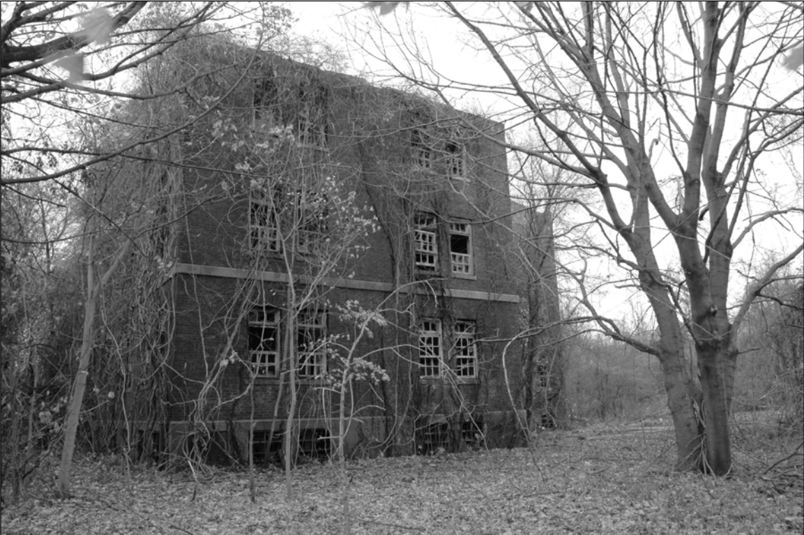
Photo 4. Northern façade, facing south.
