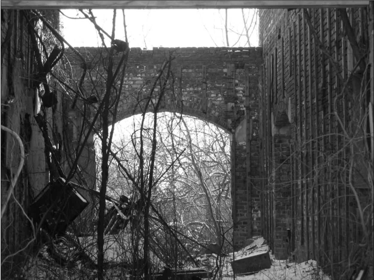
Photo 8. Headhouse, interior detail, facing east from main entrance.
