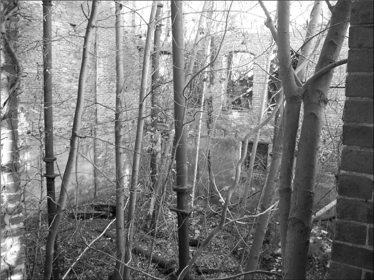
Photo 9. Central pavilion, south half, first story and basement of open interior, facing southwest.
