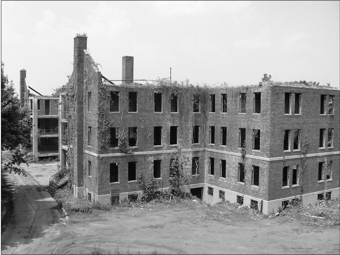
Photo 8. Building after removal of window frames in preparation for demolition.
