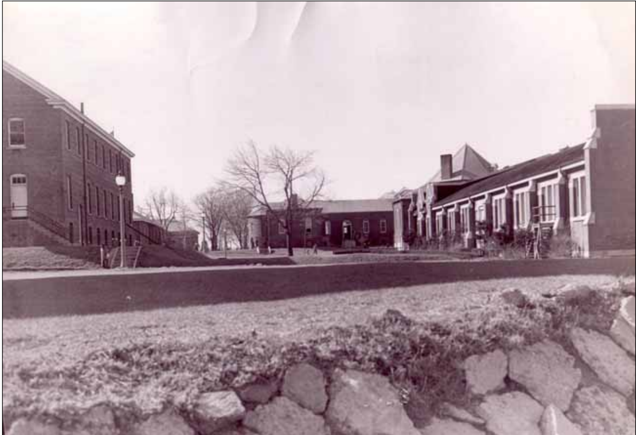
Figure 7. Southern façade of Building 57 (right) and neighboring buildings, including north side of Building 64 (left), ca. 1943. View to west. Fort Slocum Alumni and Friends Collection, Michael A. Cavanaugh, Los Angeles, CA, custodian.
