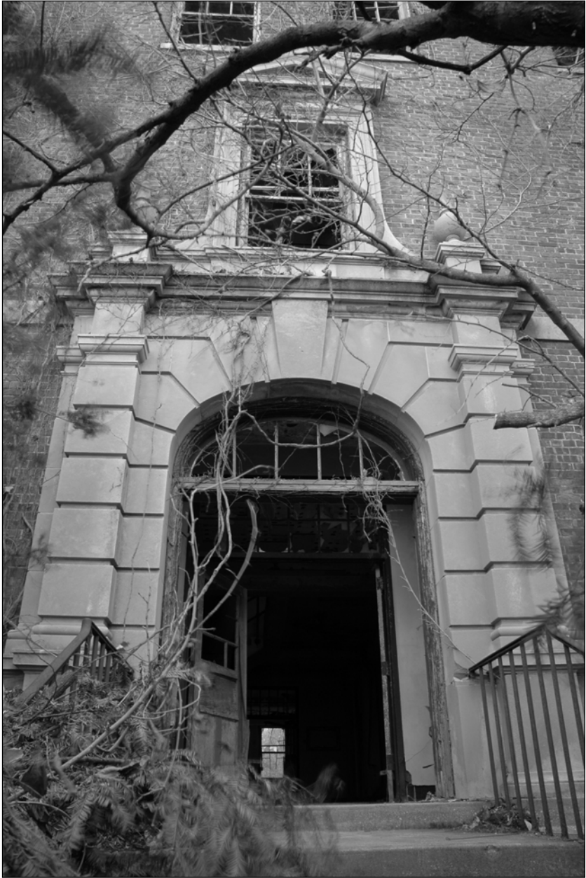
Photo 6. Eastern façade, detail: one of two main entrances, facing west.
