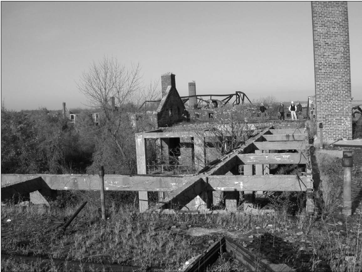
Photo 4. Roof of Building 58 overlooking porches around courtyard, facing north.
