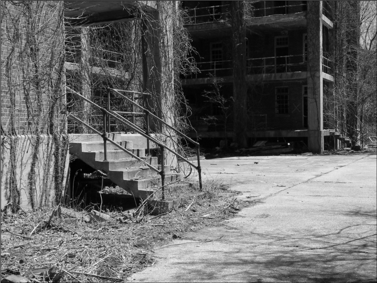
Photo 11. Western side of building, showing courtyard and porch stairs, facing southeast.
