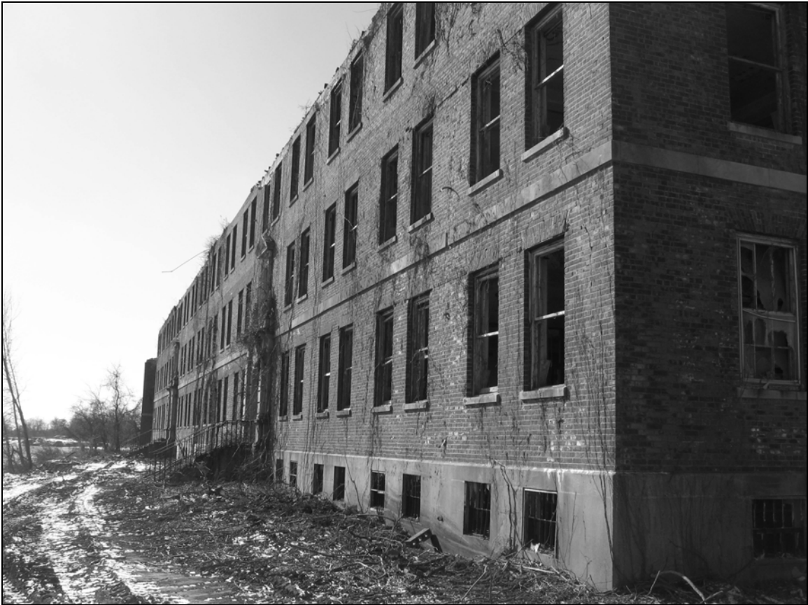
Photo 4. Eastern façade, facing south.
