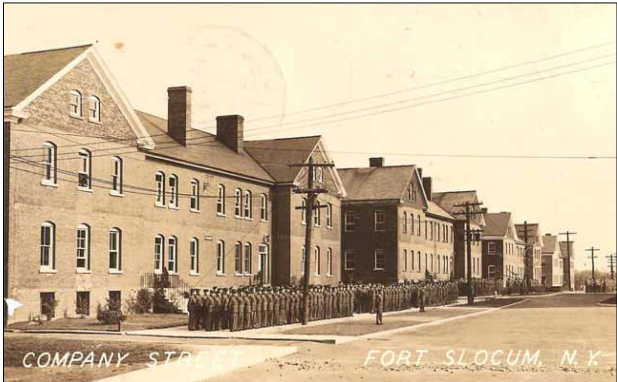
Figure 10. "Company Street, Fort Slocum, N.Y.," ca. 1940. Real photo postcard; publisher unknown. This view shows the stark main facades of Buildings 64 to 61 (left to right) along Bomford Road after the front porches were removed in the late 1930s. View southeast. Collection of Christopher L. Borstel, Tetra Tech EC, Inc., Morris Plains, N.J.
