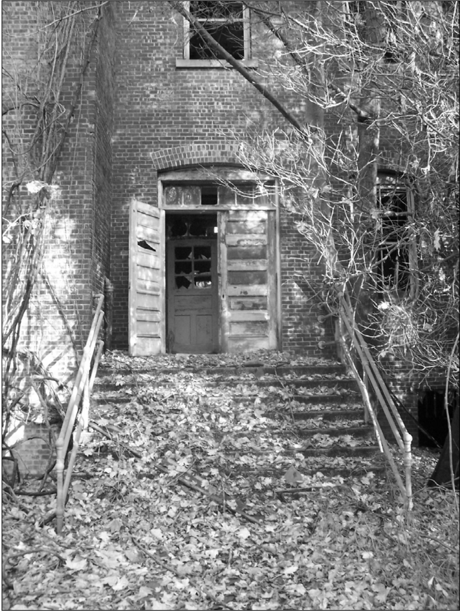
Photo 3. Western façade, detail: northern main entrance.
