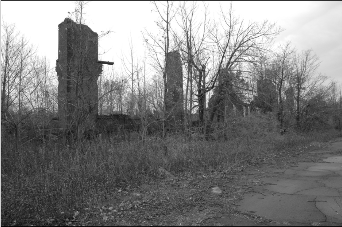
Photo 1. Building 63 ruins, facing southeast.
