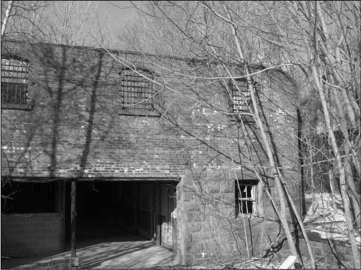
Photo 8. North end of eastern façade, facing west.
