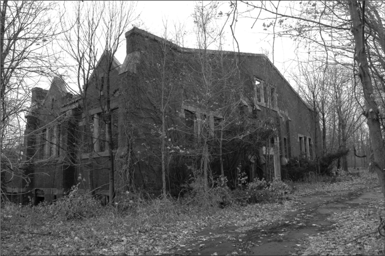
Photo 1. Headhouse, showing main (western) and northern façades, facing southeast.
