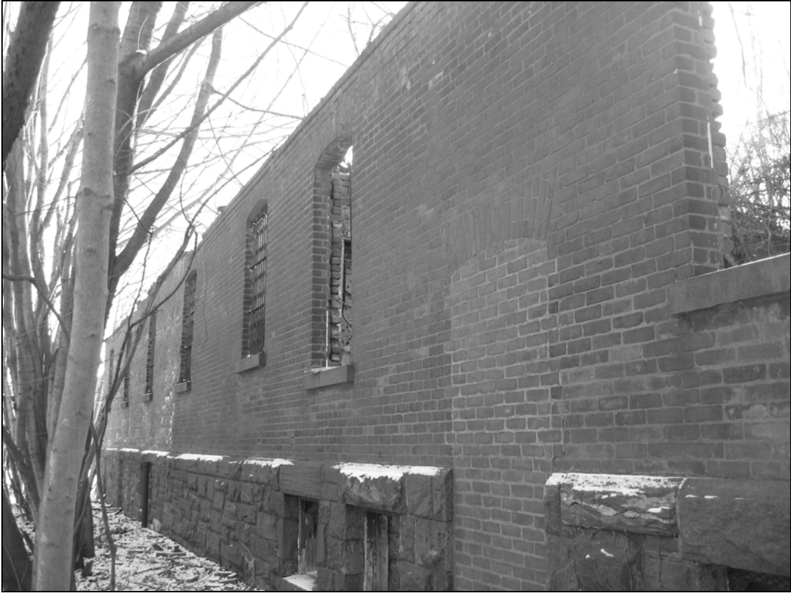
Photo 3. Northern façade, facing east.
