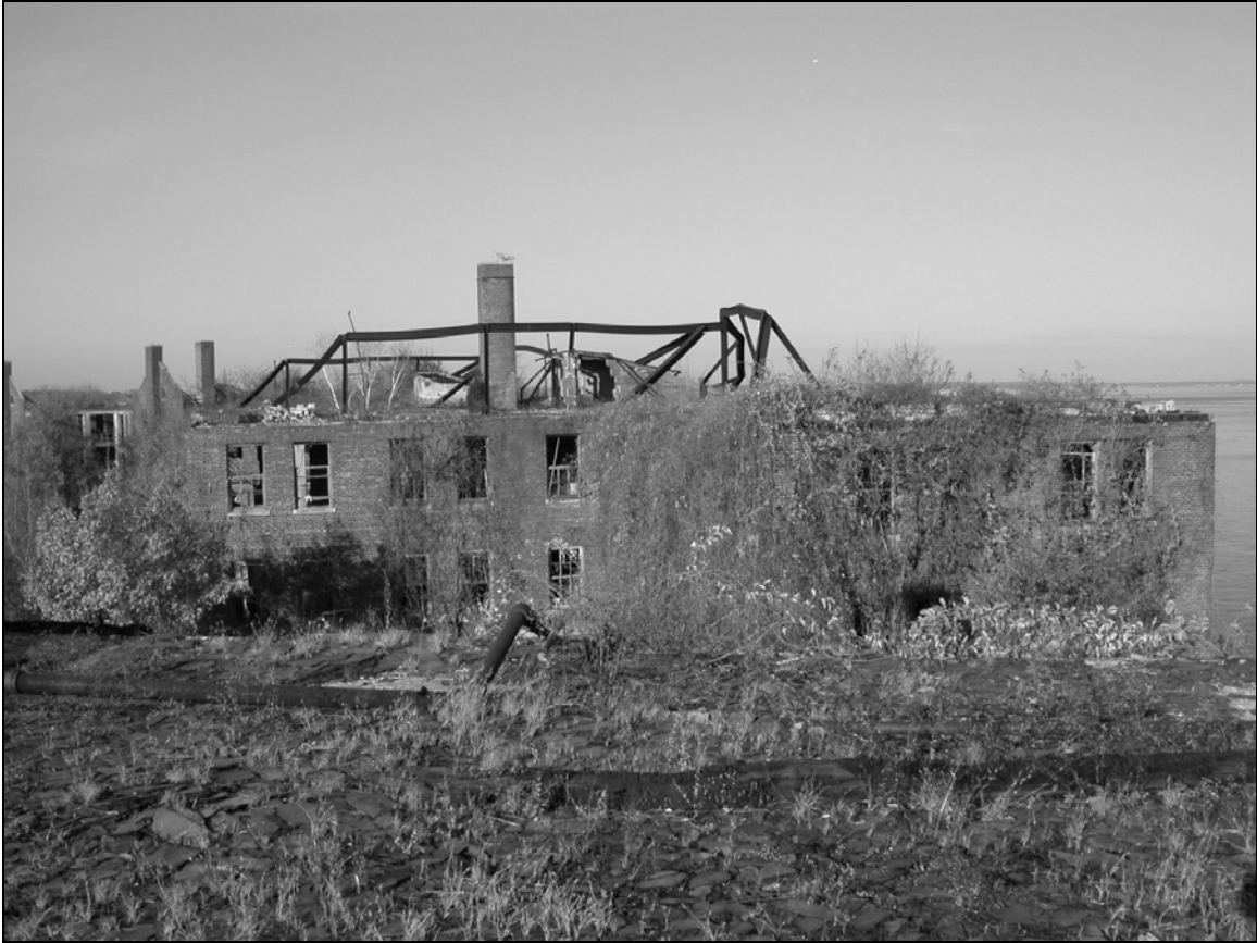
Photo 3 Roof of Building 59 from Building 58, facing north.
