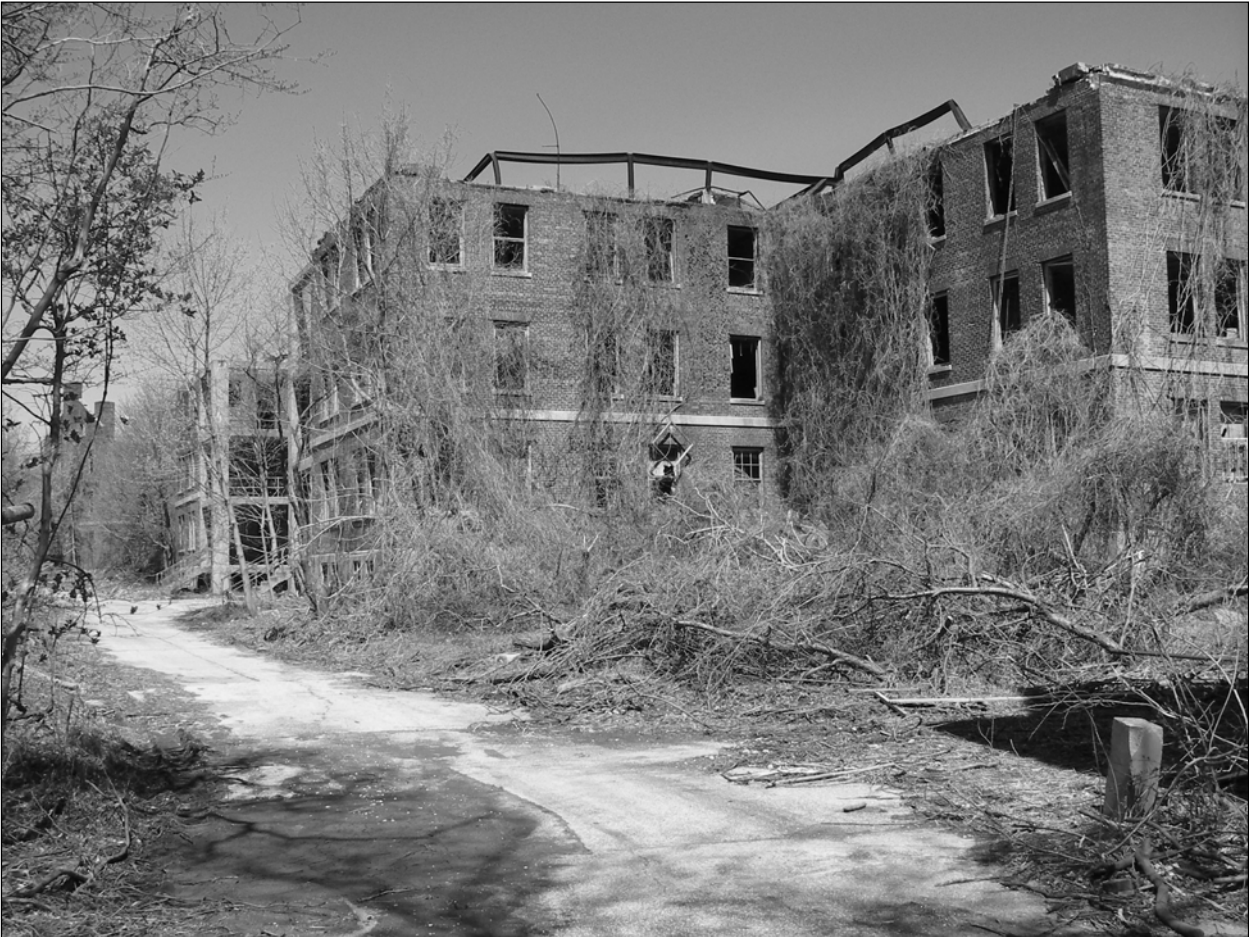
Photo 12. General view of building from Parker Road, facing northeast.
