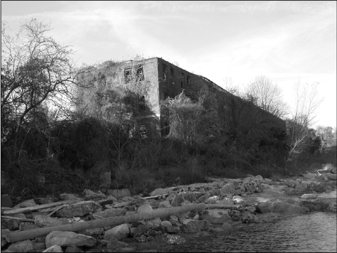
Photo 2. General view of building, facing northwest.
