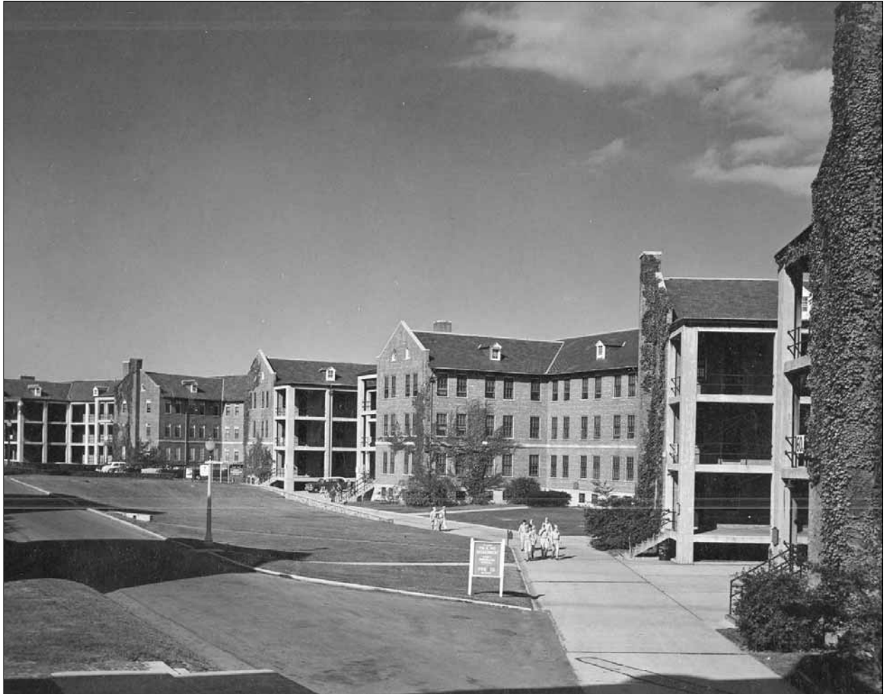
Figure 6. Buildings 58, 59, and 60 (left to right) ca. 1950. View north-northeast. Fort Slocum Collection, New Rochelle Public Library, New Rochelle, New York.
