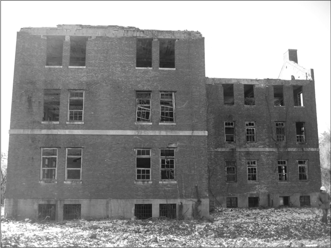
Photo 7. Northern façade, facing south.
