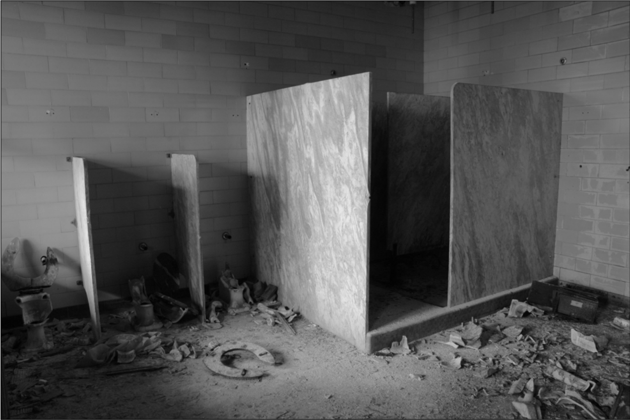
Photo 12. Interior, north half of building, showing shower and toilet stalls.
