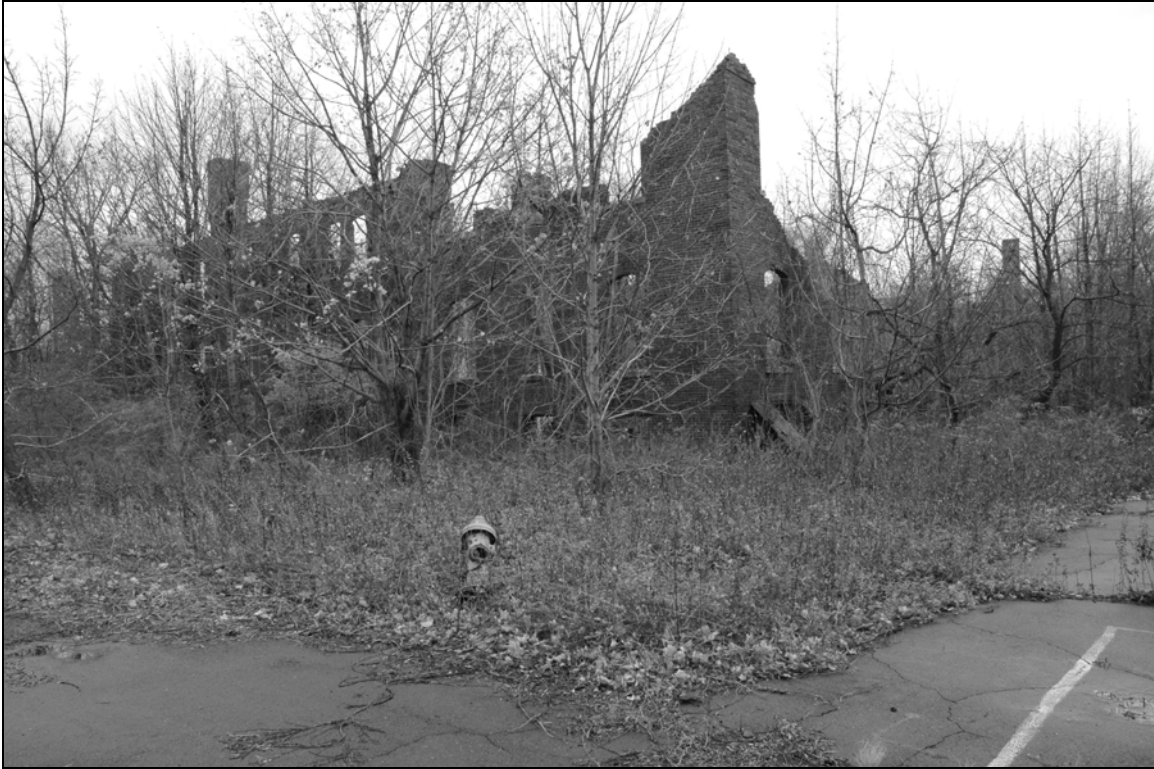
Photo 1. General view facing east-northeast from intersection of Bomford and Andrus Roads.
