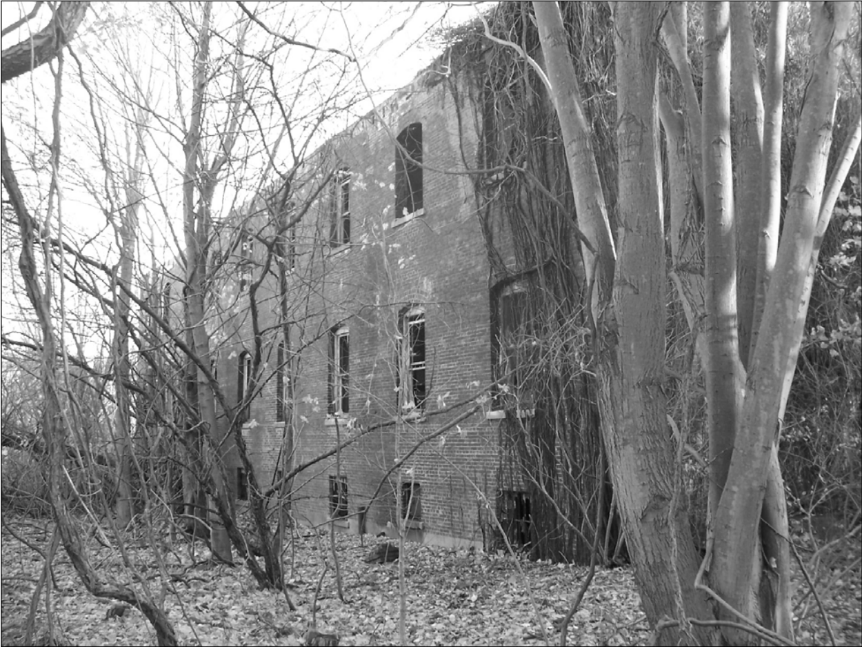
Photo 5. Northern façade of north wing, facing southeast.
