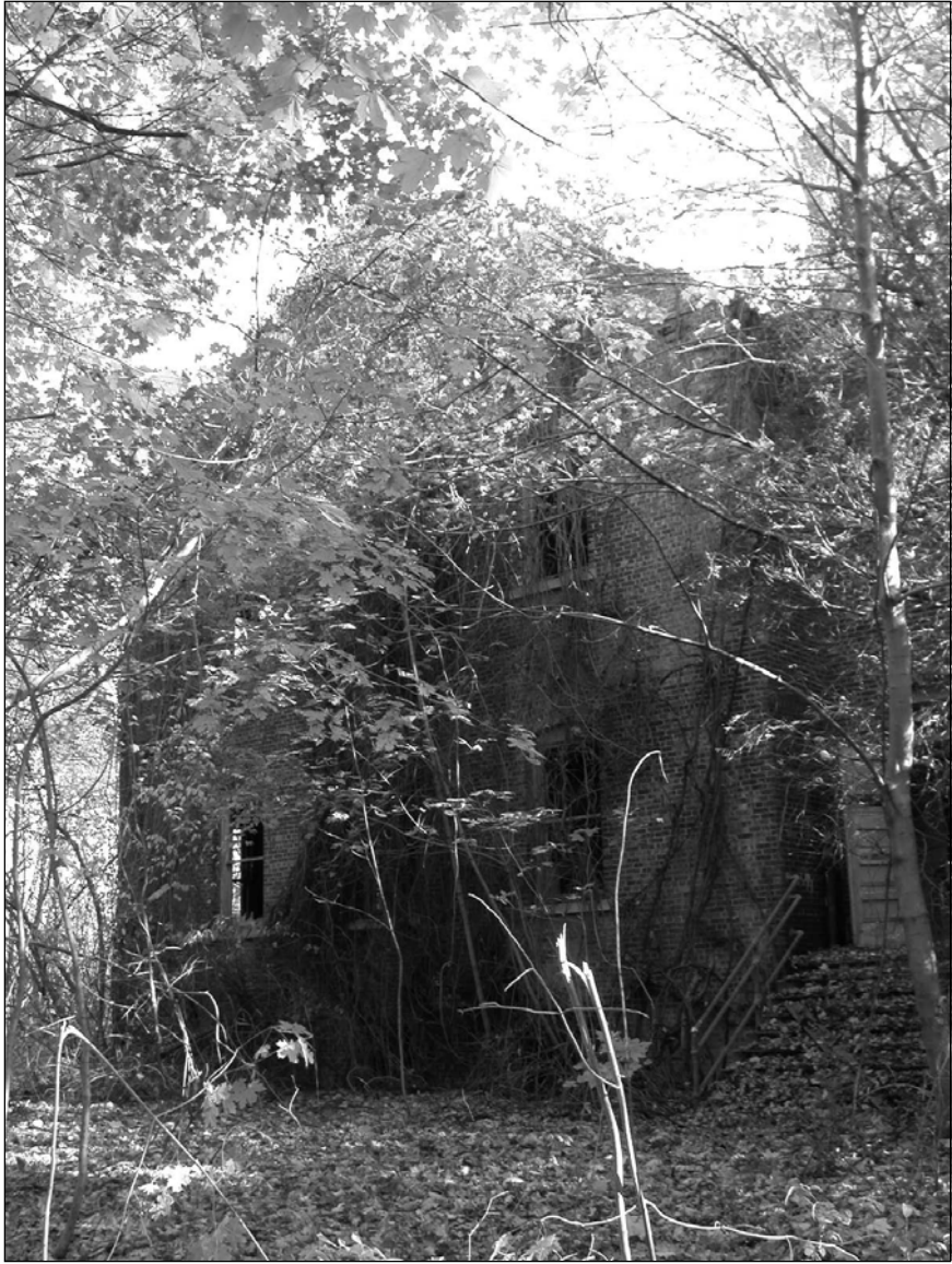
Photo 2. Western façade, north wing gable, facing east.
