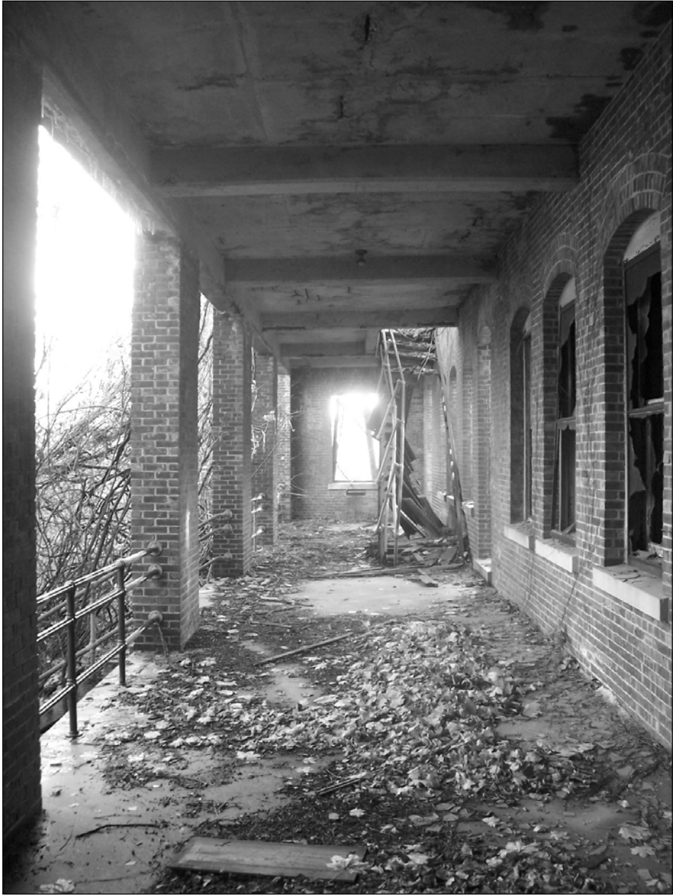
Photo 7. First story of concrete porch at rear center, facing south.
