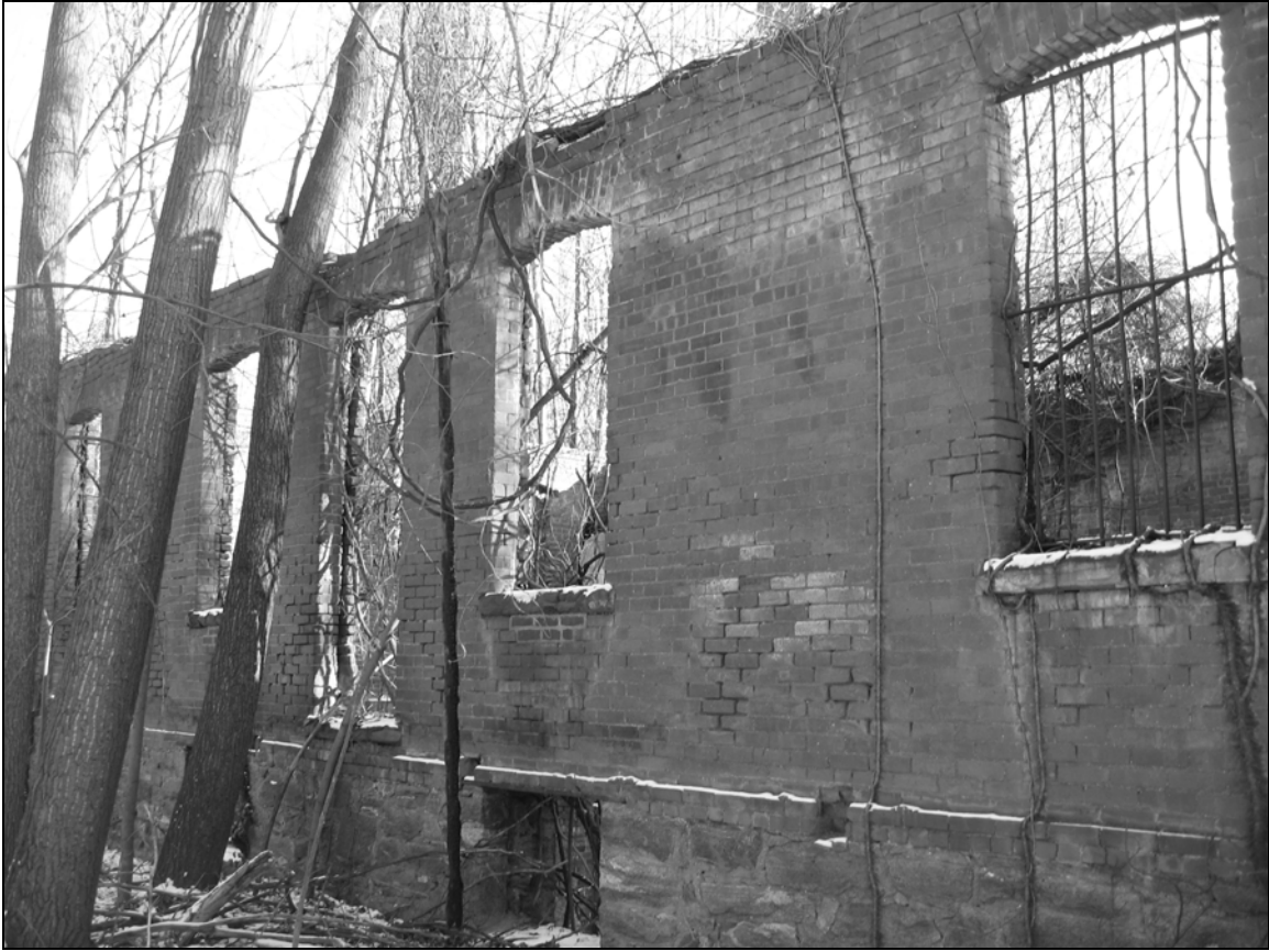
Photo 4. Western façade, facing northeast.
