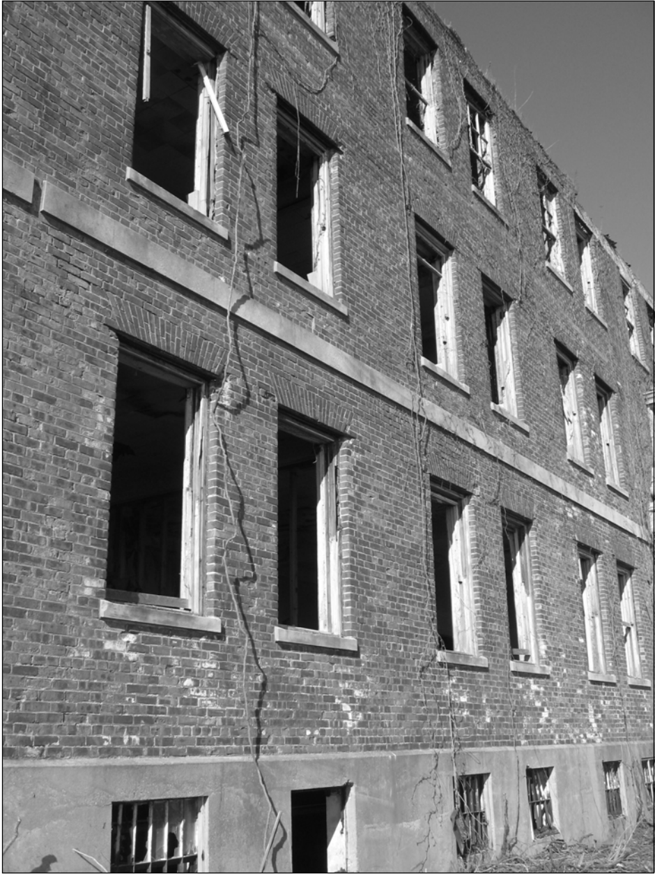
Photo 5. Southern end of eastern façade, detail, facing northwest.
