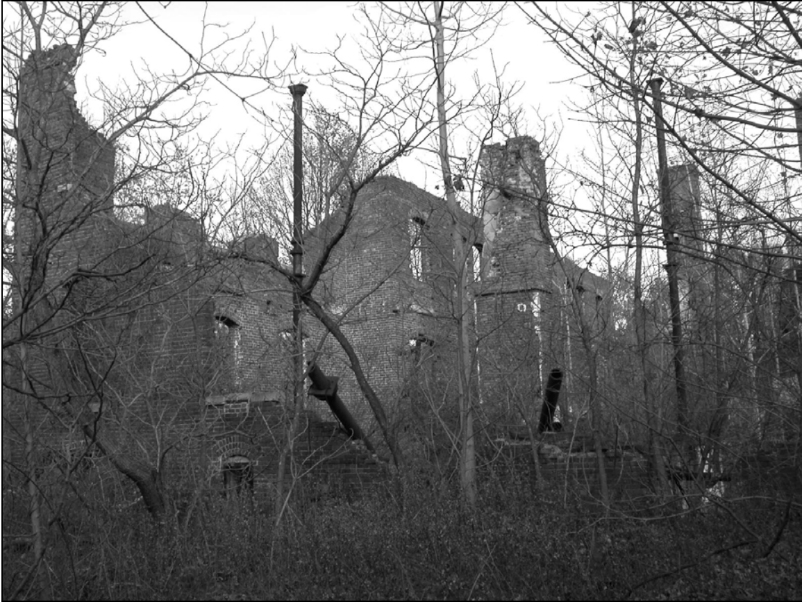
Photo 3. Southwestern section of building ruins, facing northwest.
