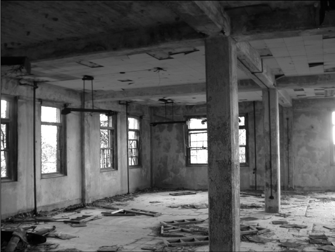
Photo 11. Interior detail, southeastern corner.
