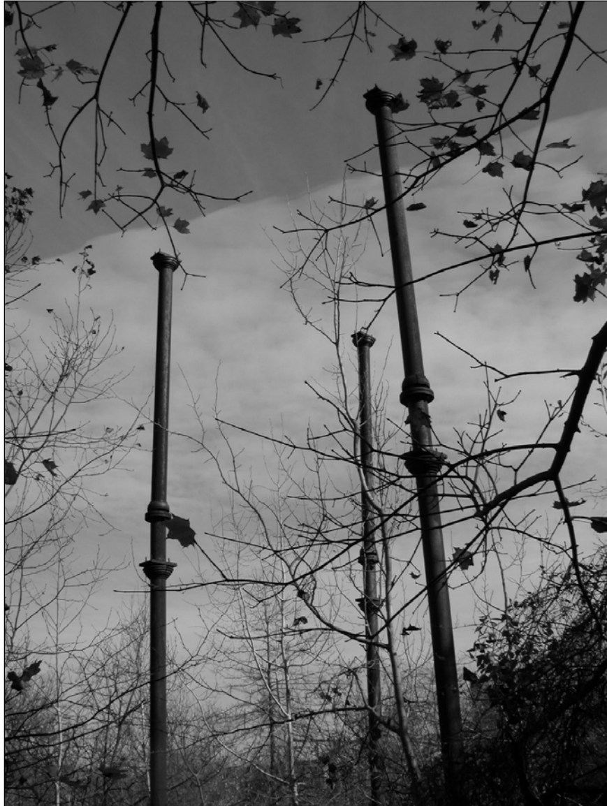
Photo 2. Detail of building ruins showing iron columns, which formerly supported floor beams.
