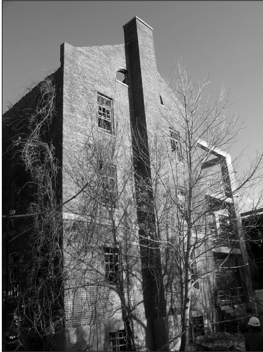
Photo 6. Western façade of northern wing, facing southeast.
