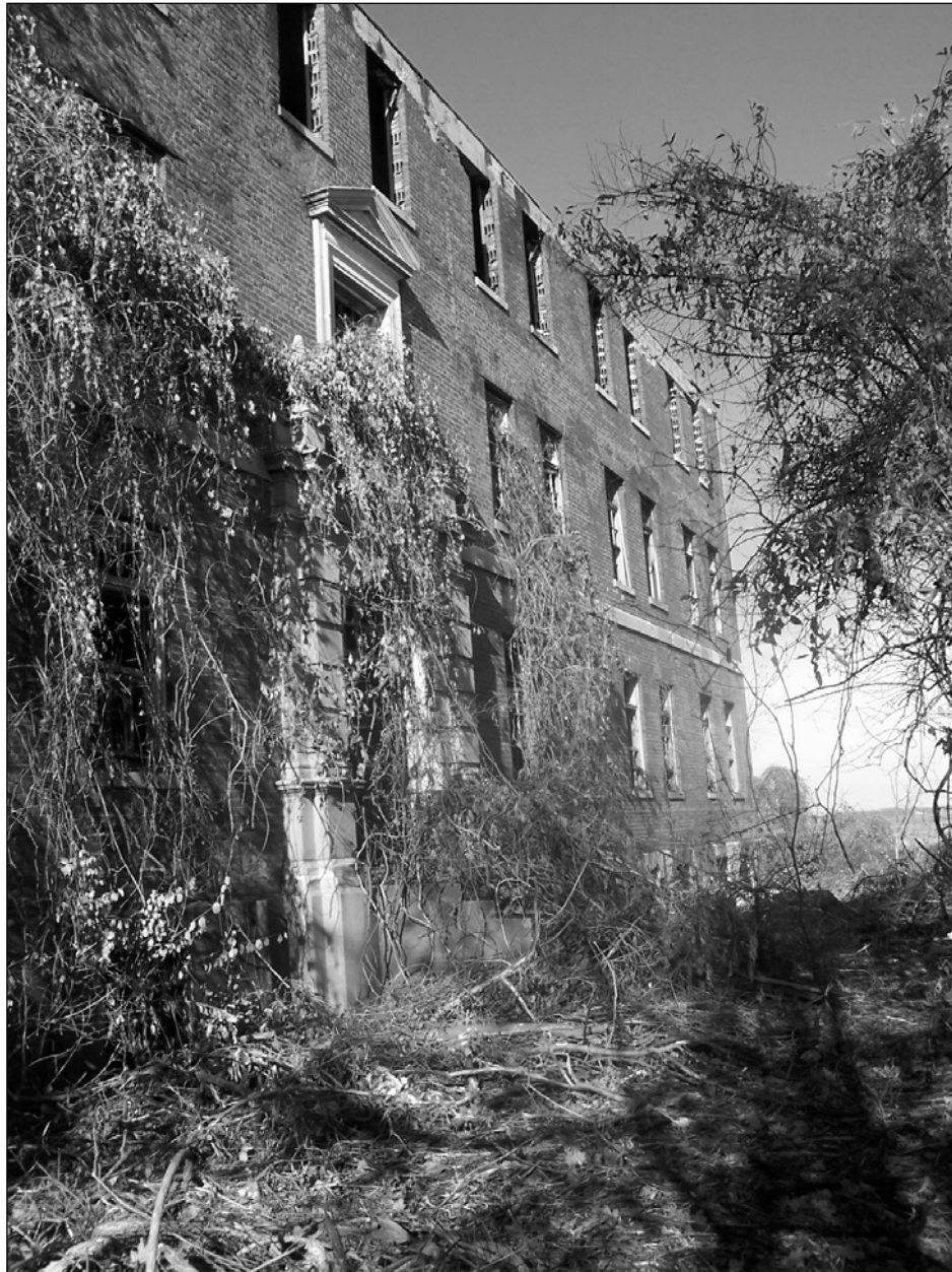
Photo 5. Northern end of eastern façade, facing northwest.
