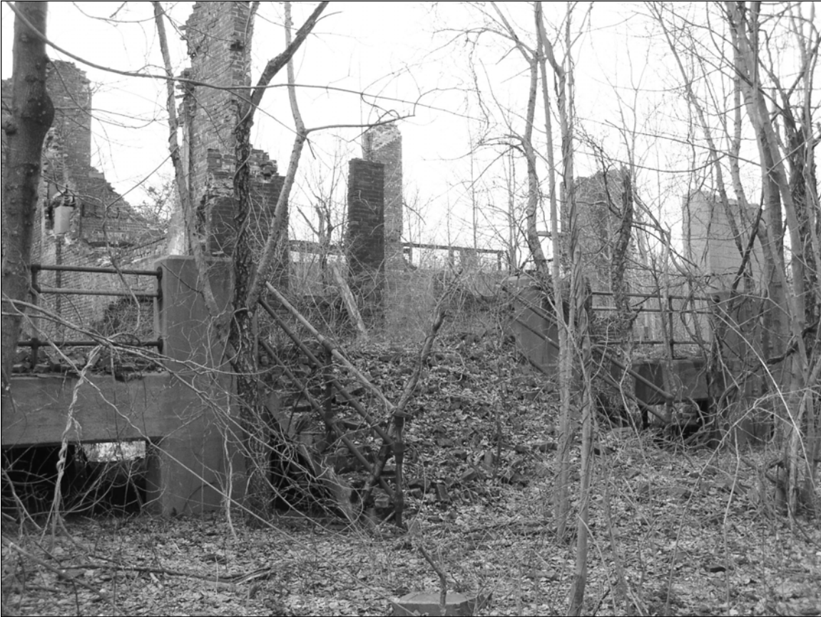
Photo 4. Stairway to concrete porch or stoop at center rear of building, facing northwest.
