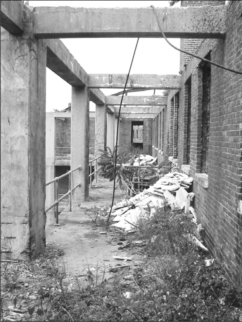
Photo 10. Third-story porch, western façade, facing north.
