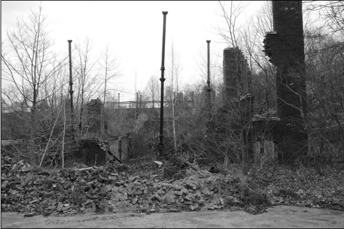
Photo 1. Northwestern corner of the ruins of Building 62, facing south.
