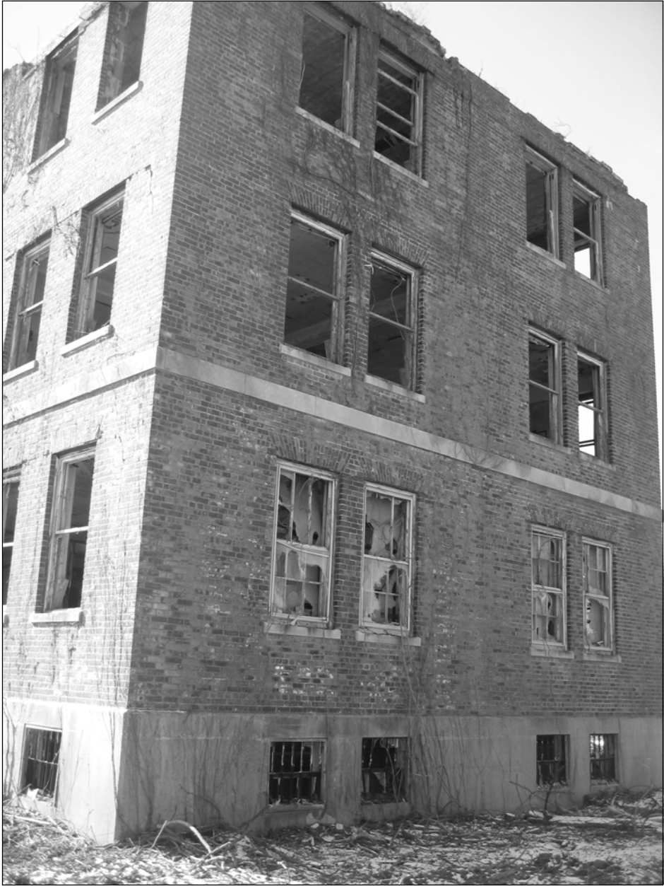
Photo 8. Northern façade, facing southwest.
