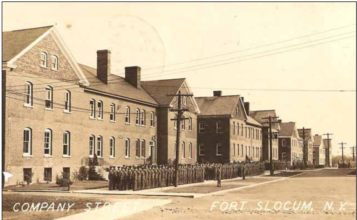
Figure 5. "Company Street, Fort Slocum, N.Y.," ca. 1940. Real photo postcard; publisher unknown. This view shows the stark main facades of Buildings 64 to 61 (left to right) along Bomford Road after the front porches were removed in the late 1930s. View southeast. Collection of Christopher L. Borstel, Tetra Tech EC, Inc., Morris Plains, N.J.
