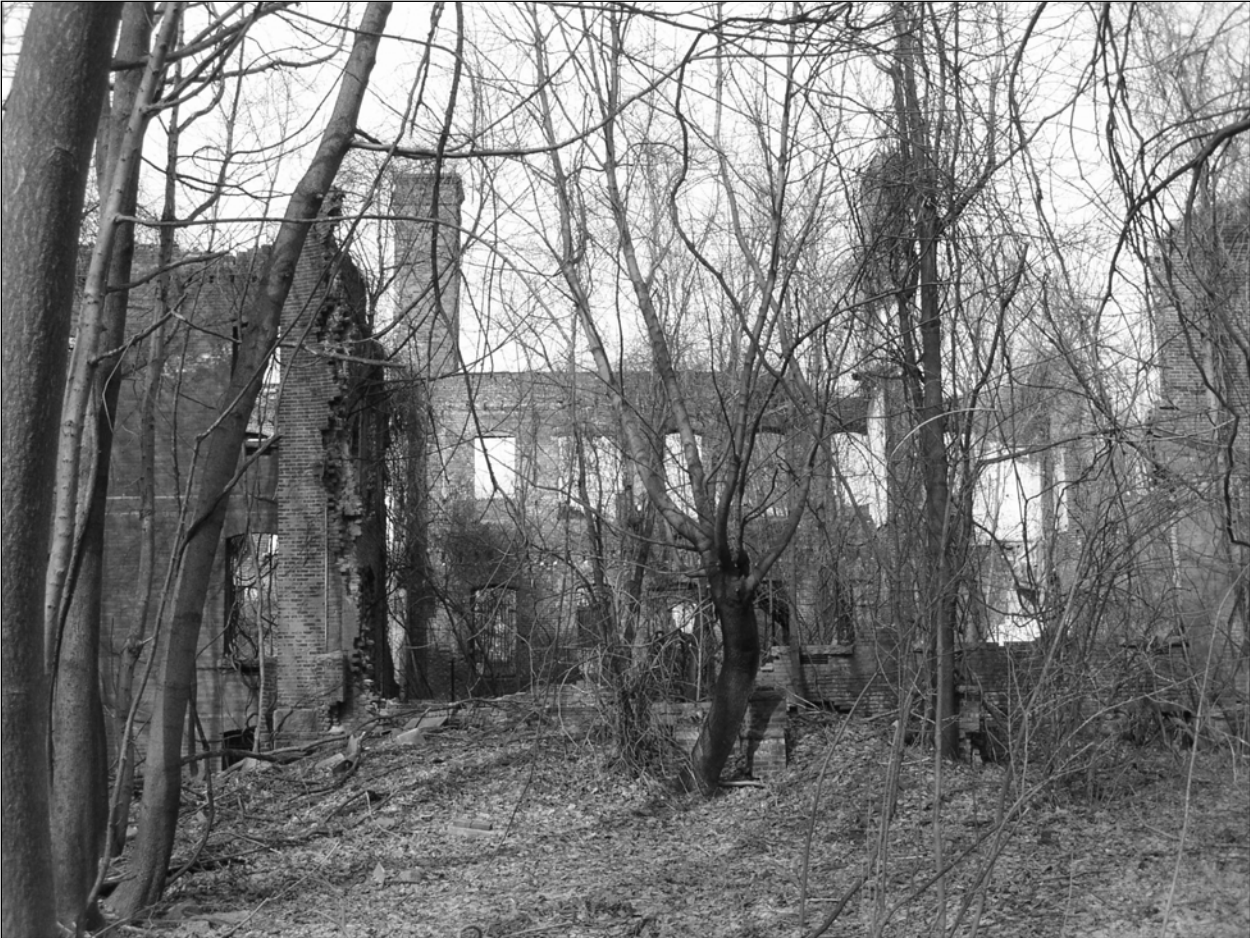
Photo 2. Ruins of central pavilion, southern façade, facing north.
