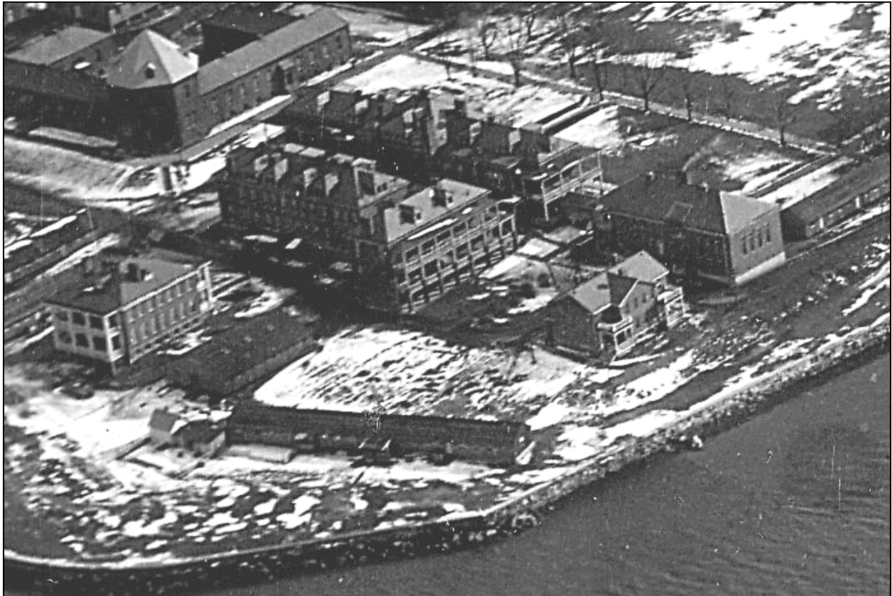
Figure 5. Oblique aerial photo, detail. View southeast. Ca. 1922, winter. Building 46 is the large two-and-a-half-story building at the center. Original in National Archives, College Park, MD; digital copy from Fort Slocum Alumni and Friends Collection, Michael A. Cavanaugh, Los Angeles, CA, custodian.
