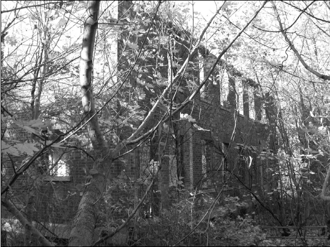
Photo 4. Eastern façade, facing northwest.
