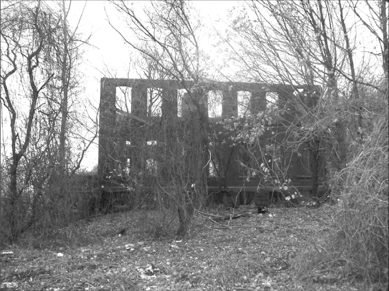
Photo 5. Western façade, looking east.
