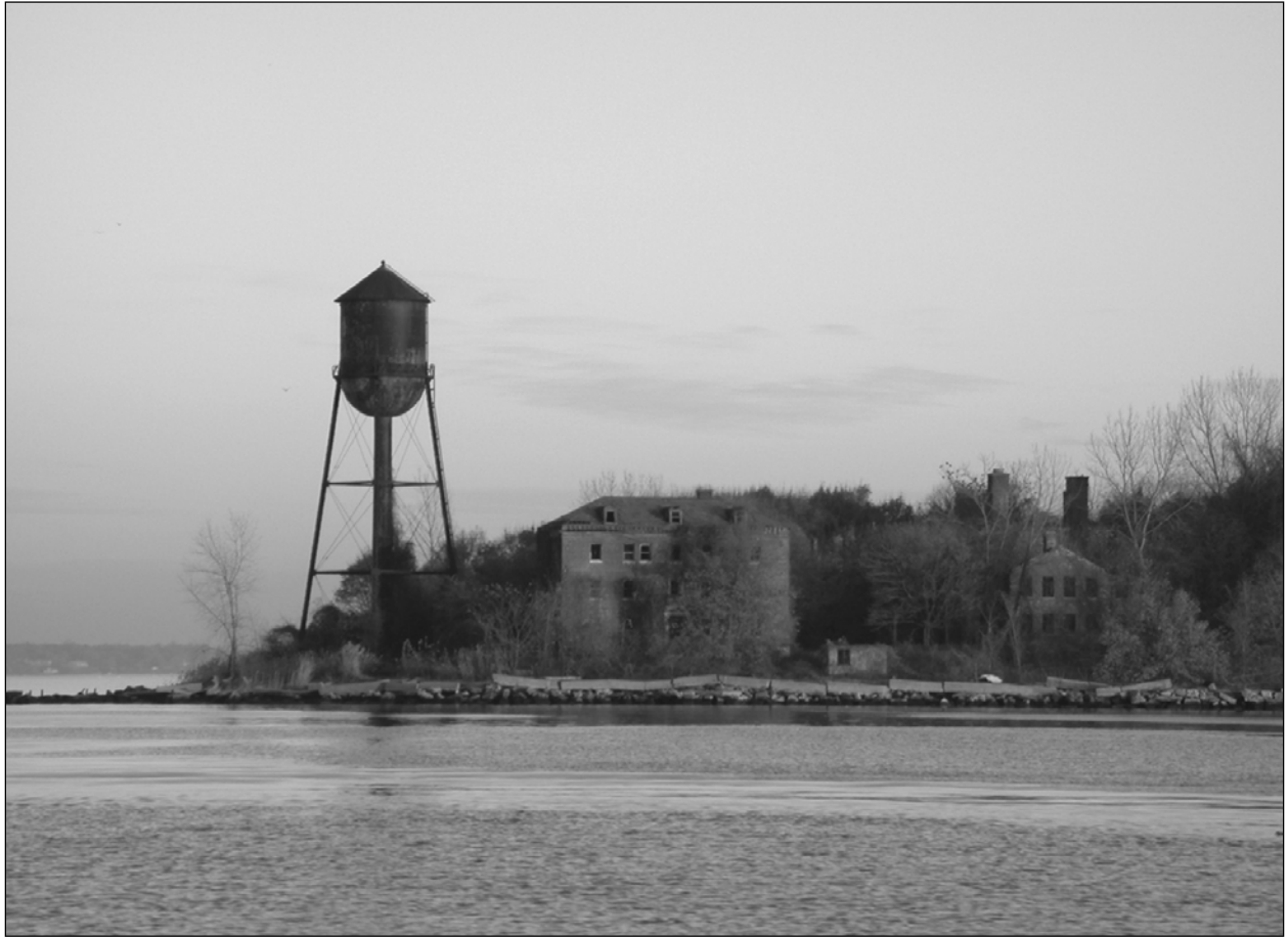
Photo 2. The Water Tower at the northwestern tip of Davids Island as viewed from the channel between Davids Island and the New Rochelle mainland, facing east.
