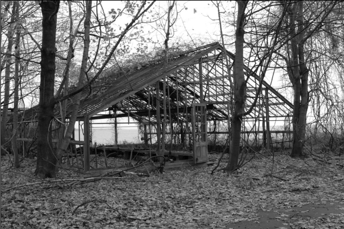
Photo 1. Southern façade with view of interior, facing northeast.
