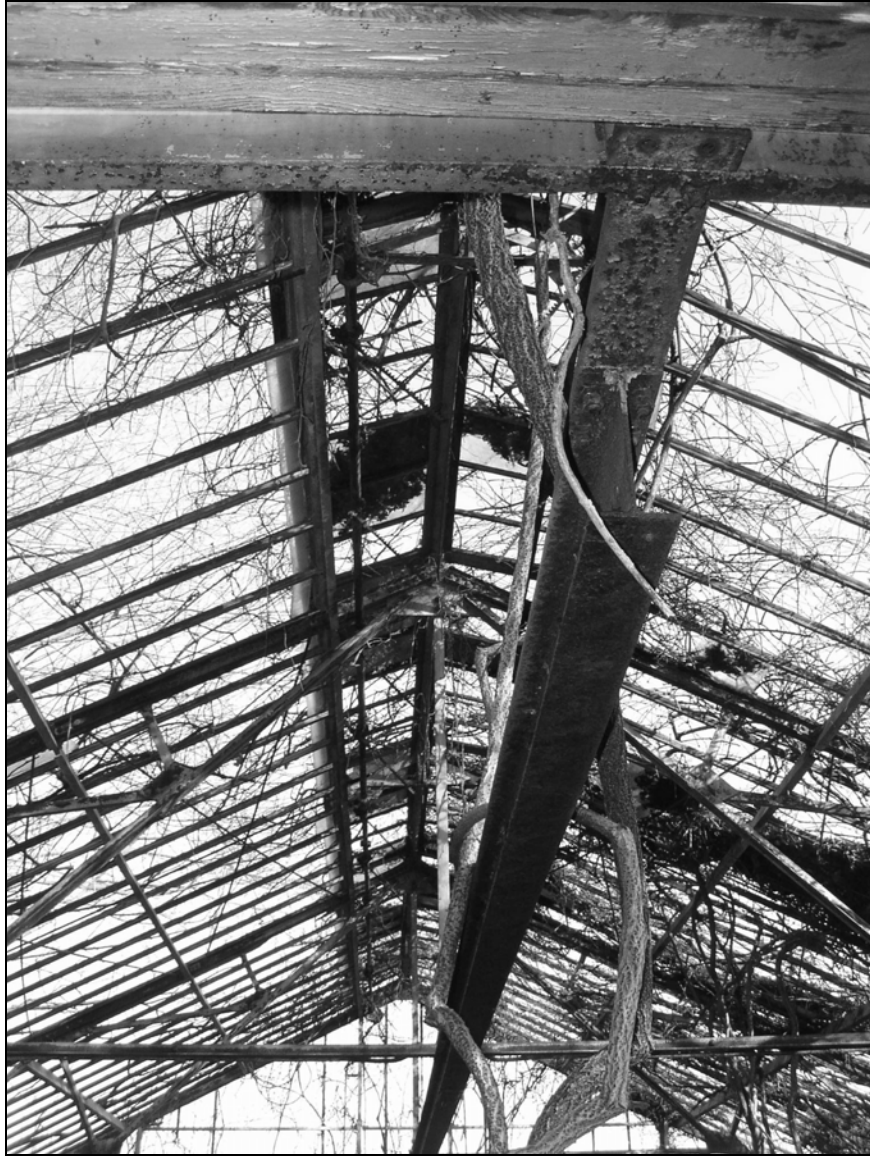
Photo 5. Interior, showing I-beam rail and details of roof structure, facing north.
