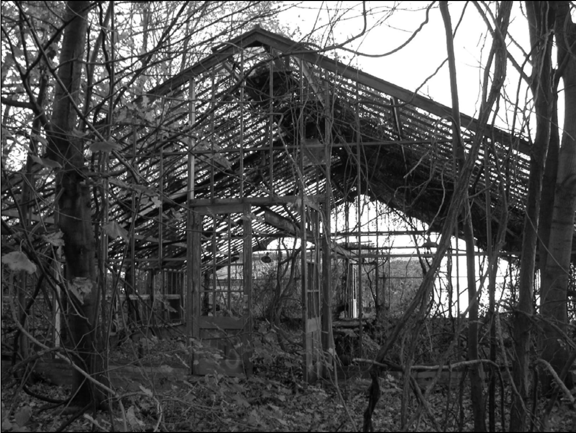
Photo 3. Southern façade, detail, with view of interior, facing north.
