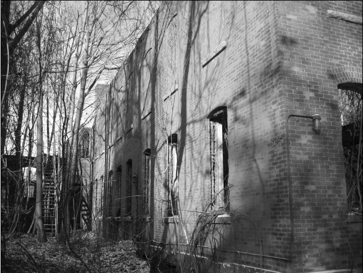
Photo 11. Southern façade of rear east wing, facing northwest.
