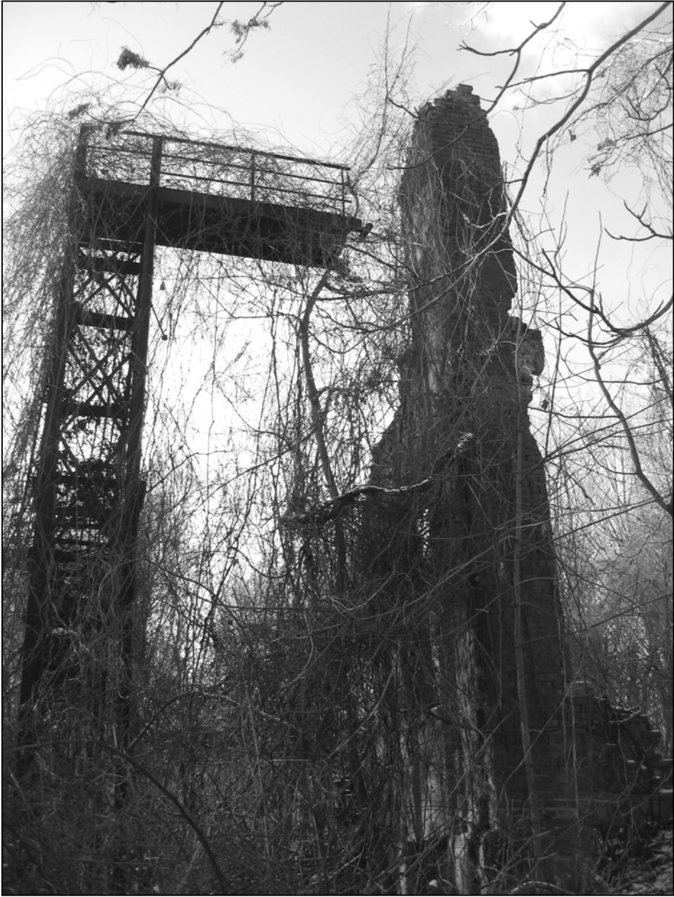
Photo 8. Self-supporting steel fire escape near southeastern corner of front east wing, facing south.
