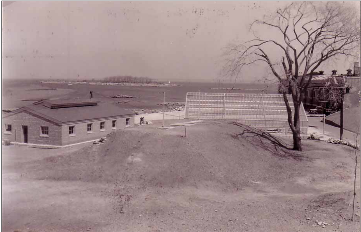
Figure 4. Inventory photograph of Fort Slocum's sewage treatment plant, October 1940. The plant included the Tank House (present-day Building 52) at left; Digesting Tanks Nos. 1 and 2 (not currently numbered), in the earth mound at center; and the Sludge Drying Bed Building (Building 53) at center right. Record Group 77, National Archives, College Park, MD.
