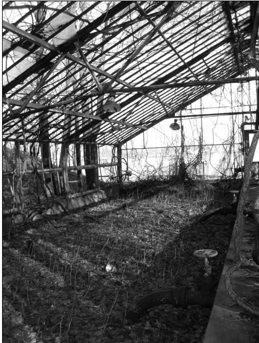
Photo 6. Western side of interior, facing north.
