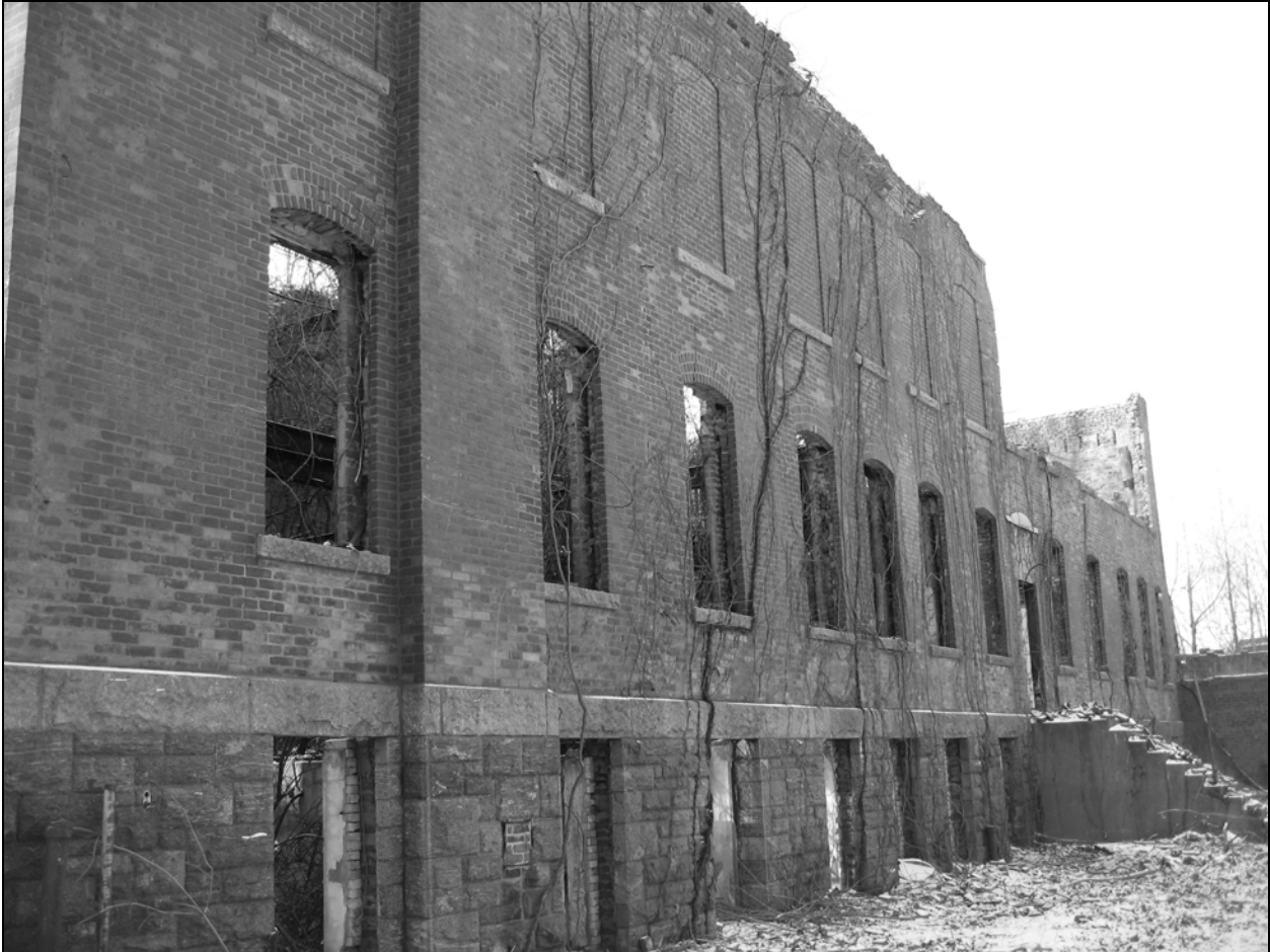
Photo 13. Northern façade of rear east wing, facing southwest.
