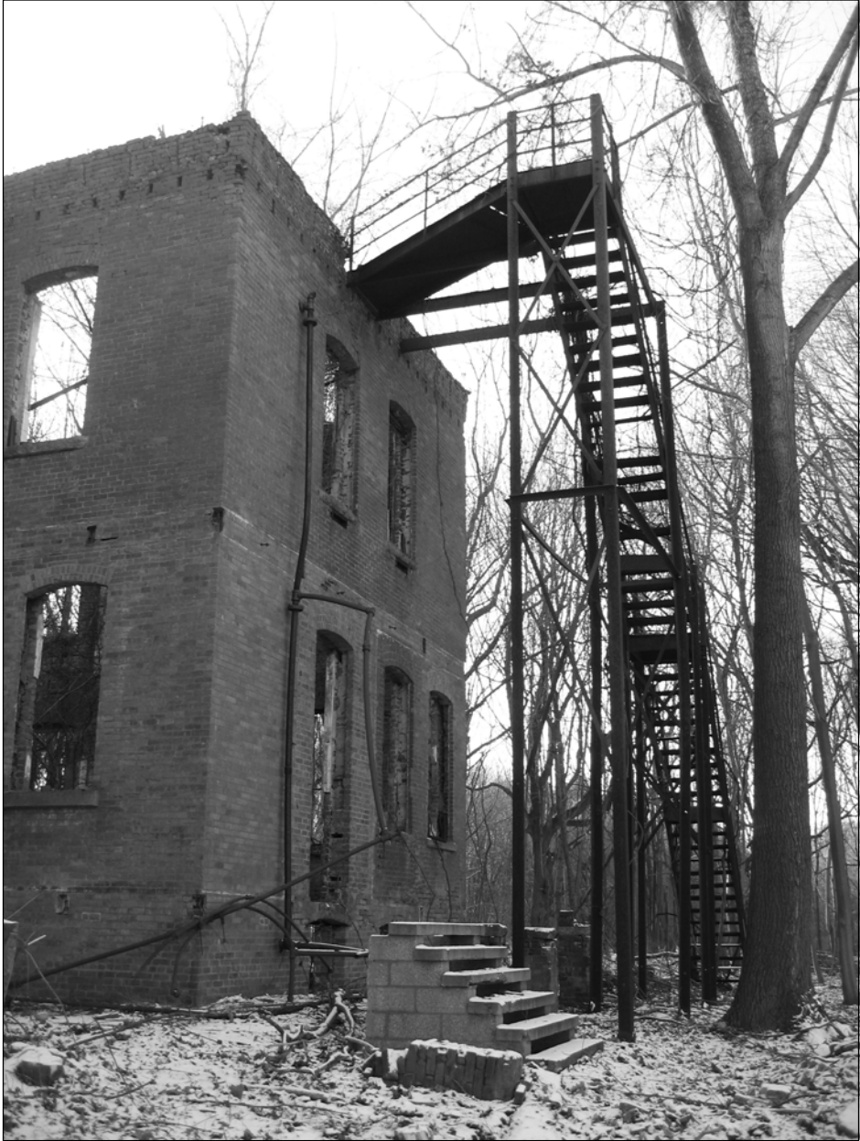
Photo 19. Western end of front west wing with self-supporting steel fire escape, facing south-southeast.
