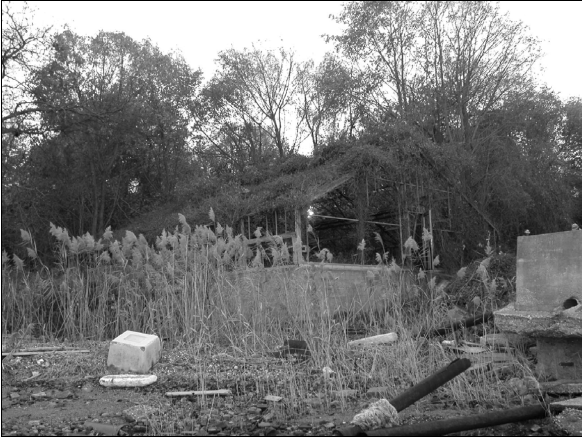
Photo 4. Northern and eastern façades with view of interior, facing southwest.
