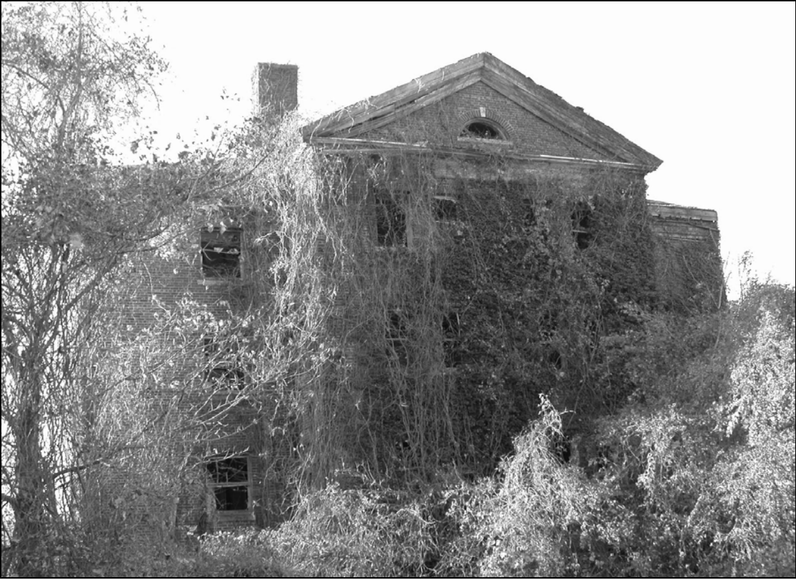
Photo 1. East façade, looking west.
