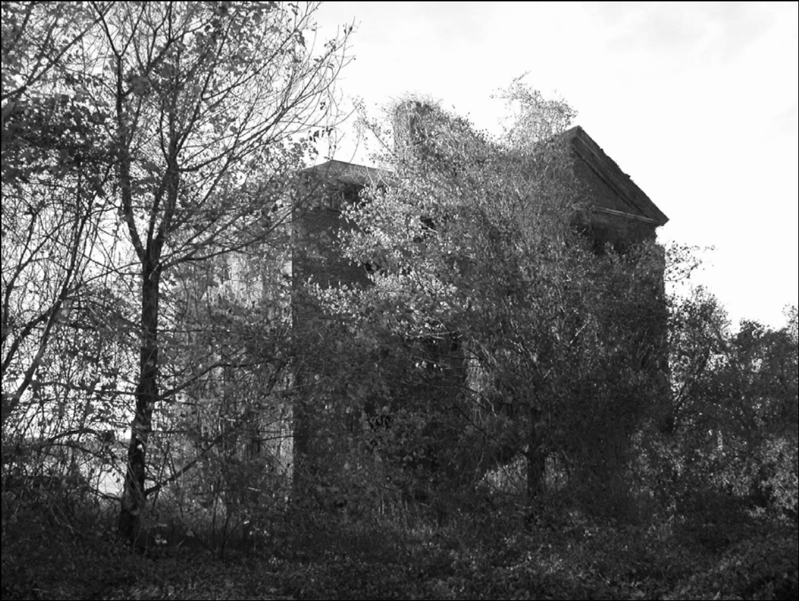
Photo 4. East façade, looking northwest.
