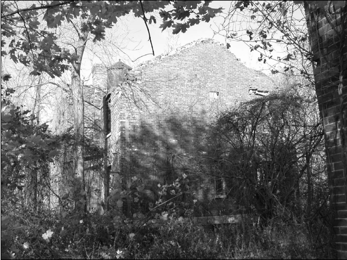
Photo 3. Southern and western facades, facing north.
