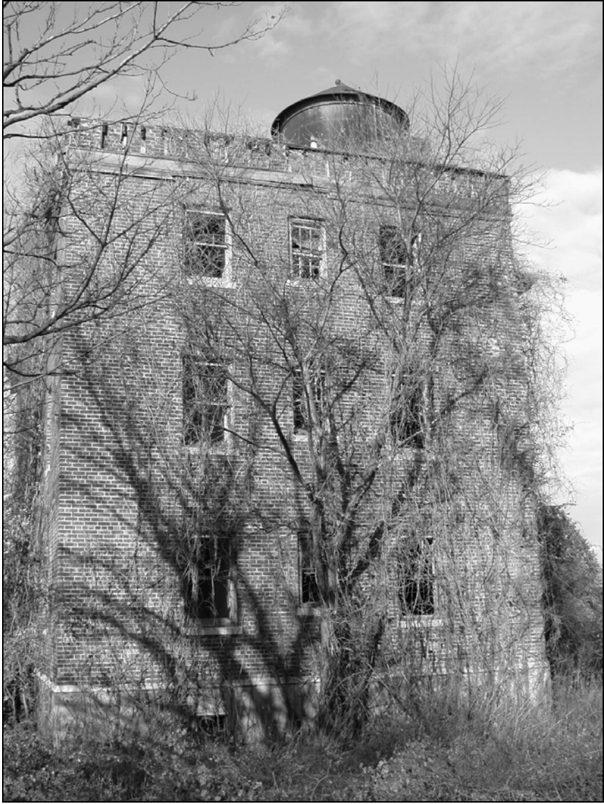
Photo 2. South façade, looking north.
