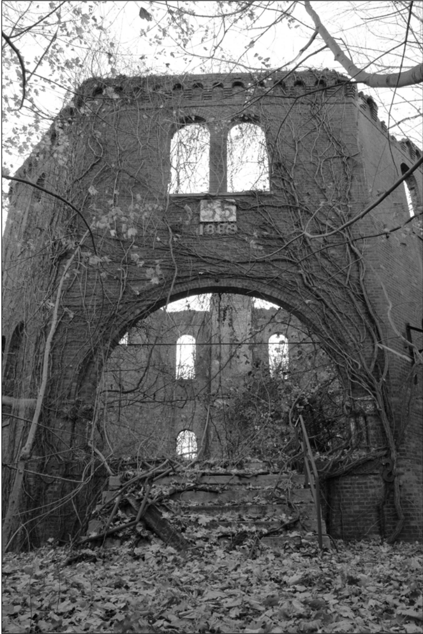
Photo 2. Northwestern façade of tower, facing southeast.
