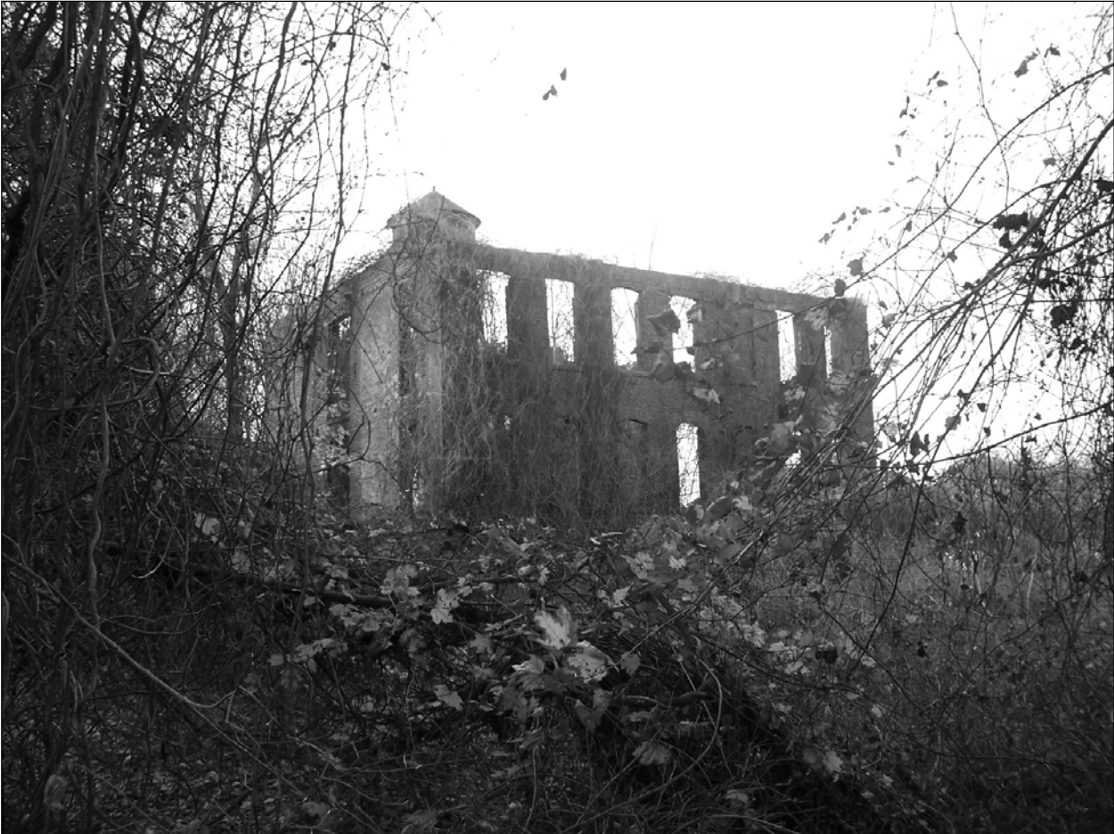
Photo 8. Eastern and southern façades, looking northwest.
