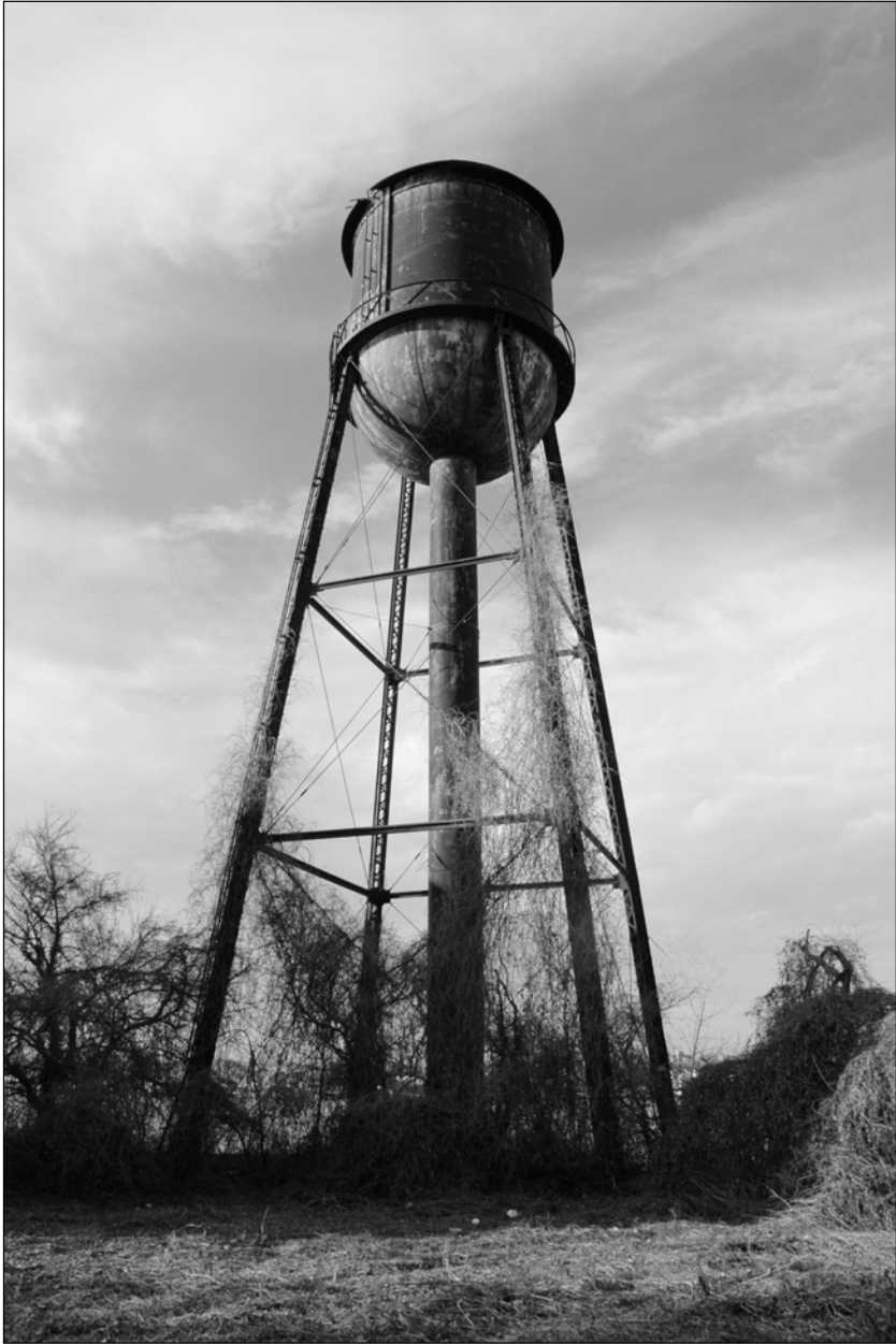
Photo 4. Water Tower, facing northwest.
