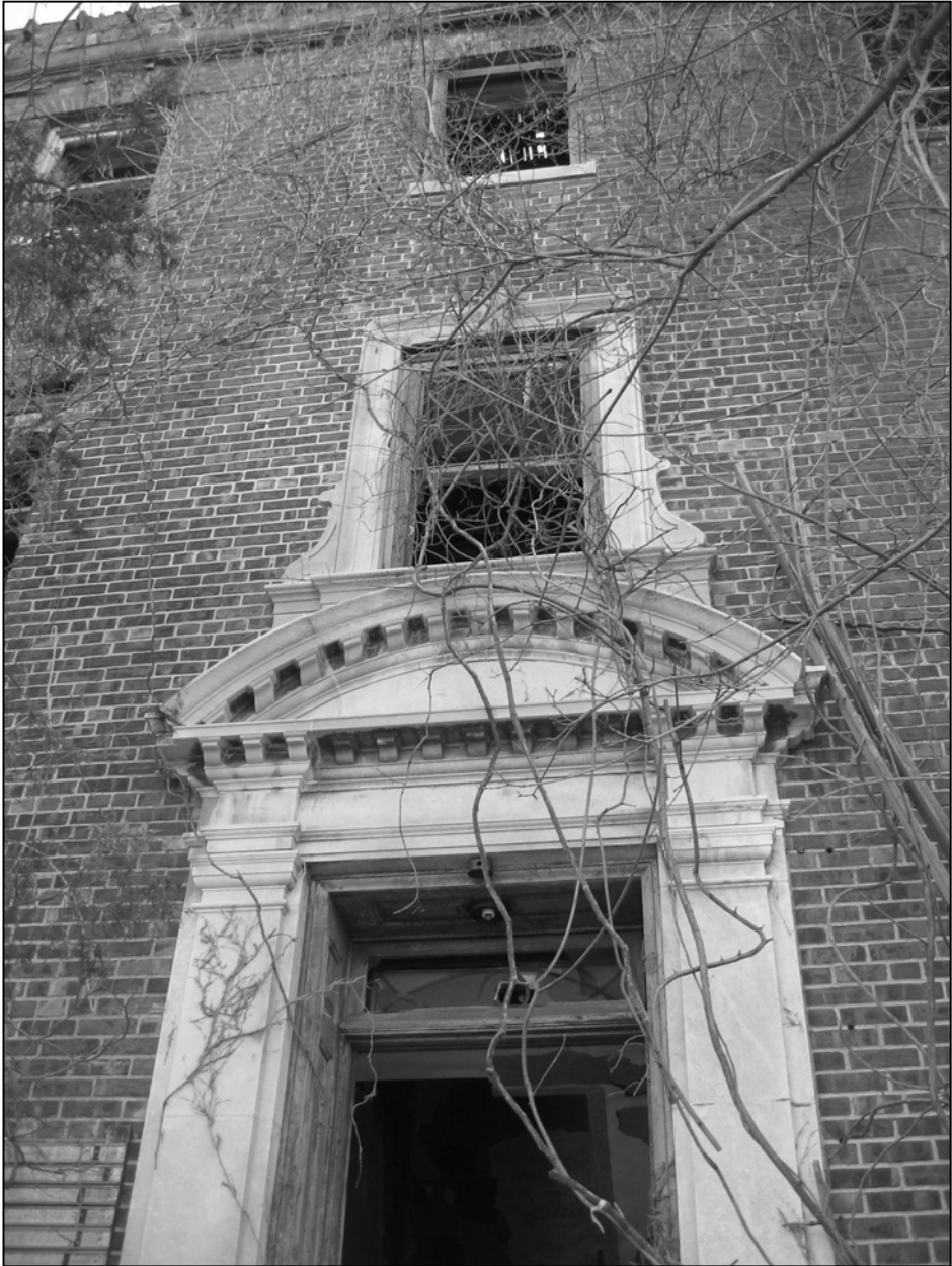
Photo 6. West façade, detail.
