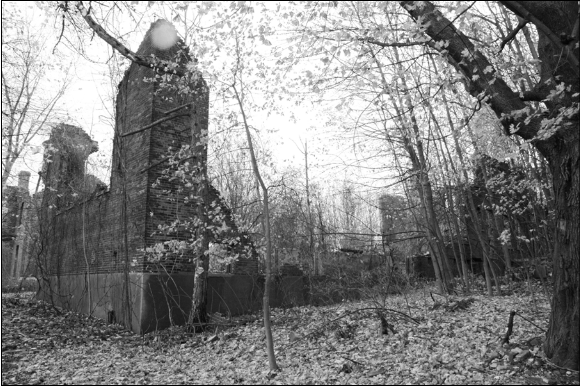
Photo 1. Southwestern corner, showing remnants of adjoining façades, facing northeast.
