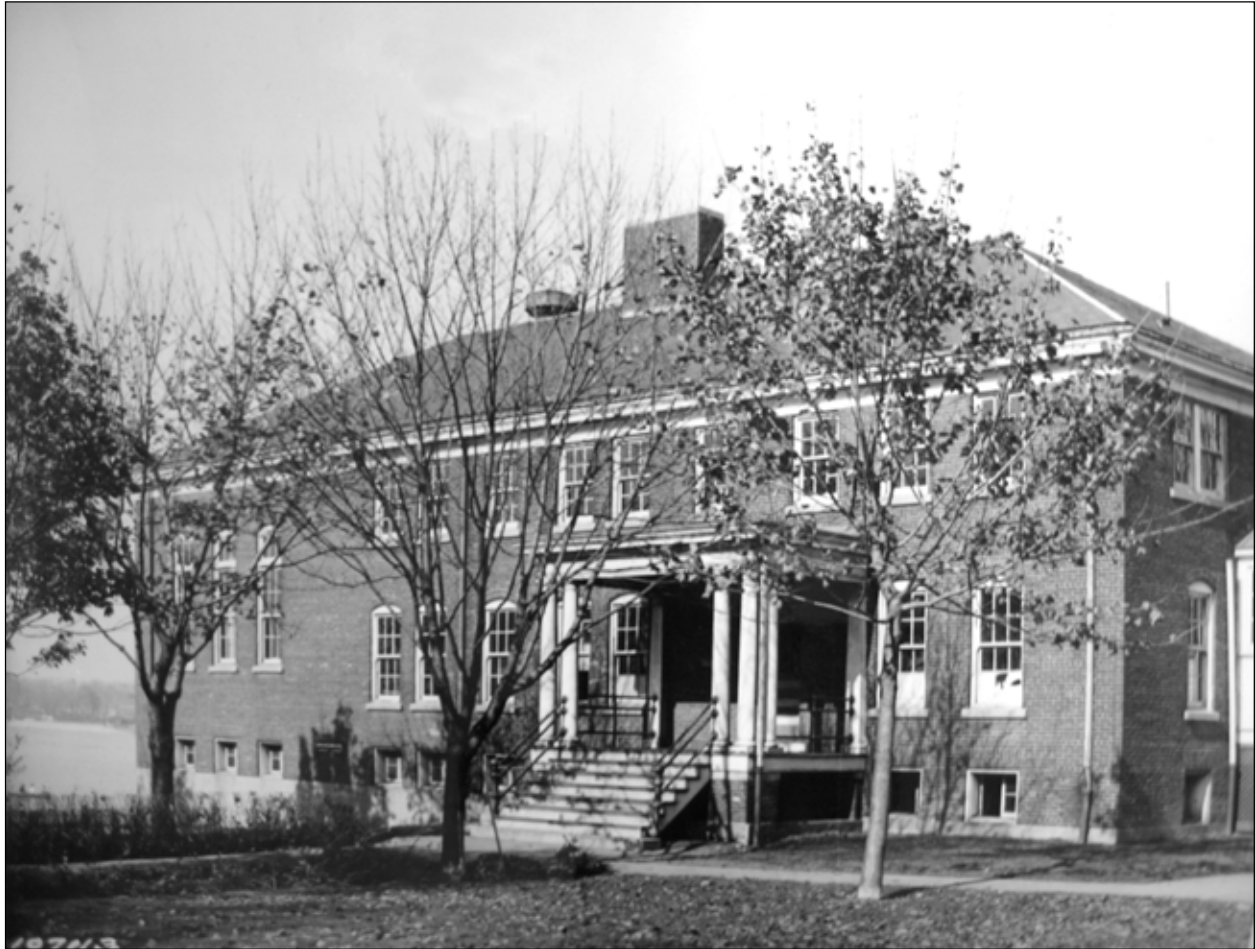
Figure 4. Inventory photograph, probably mid-1930s. View northwest showing main (southern) façade. Record Group 111, National Archives, College Park, MD.
