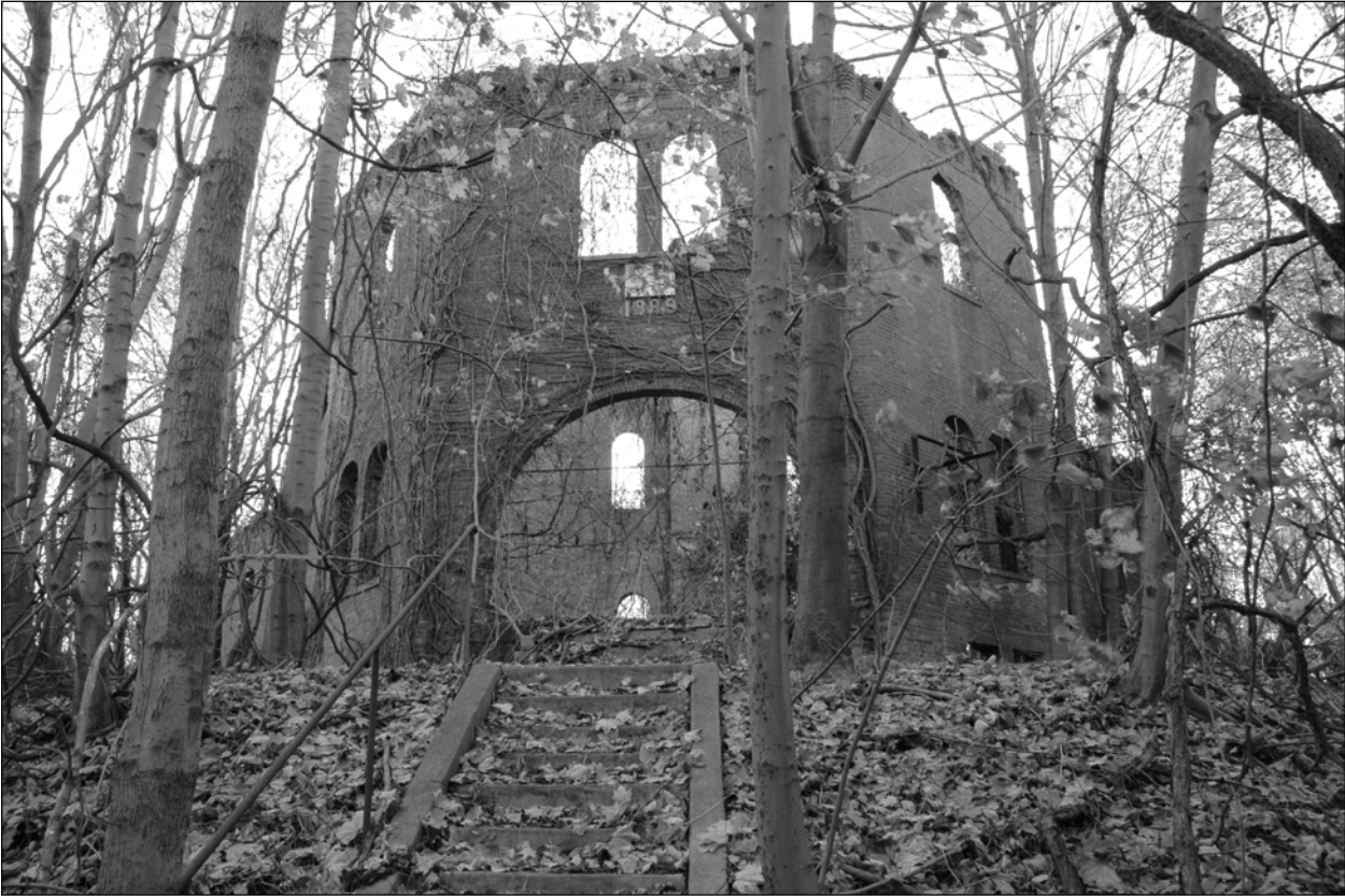
Photo 1. Northwestern side of tower with set of steps up fill prism in foreground, facing southeast.
