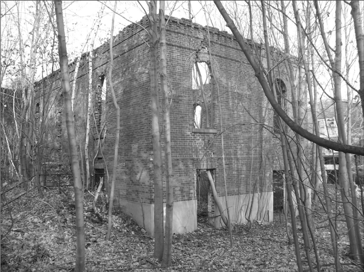
Photo 7. South and west walls of south dependency, facing northeast.
