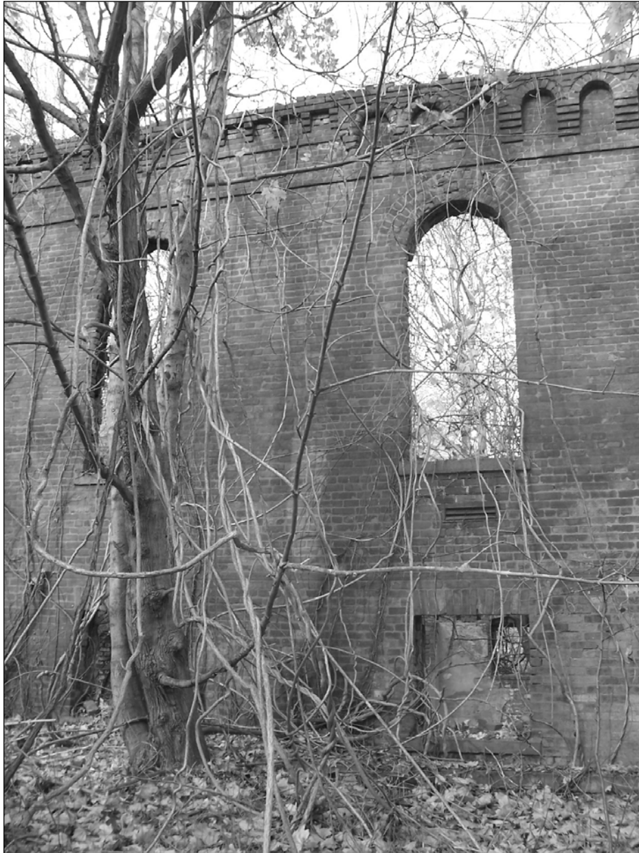
Photo 8. Detail of building wall showing its two cornice types: Lombard arch at right and rectangular machicolations at left.
