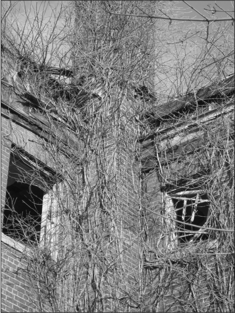
Photo 9. West façade, detail.
