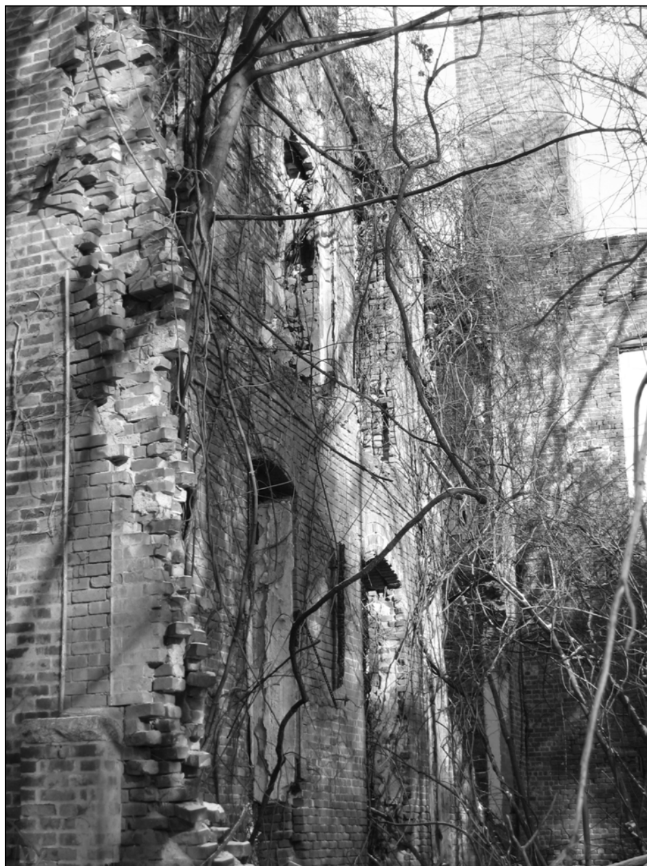
Photo 5. Interior of central pavilion, showing west wall detail, facing north-northwest.
