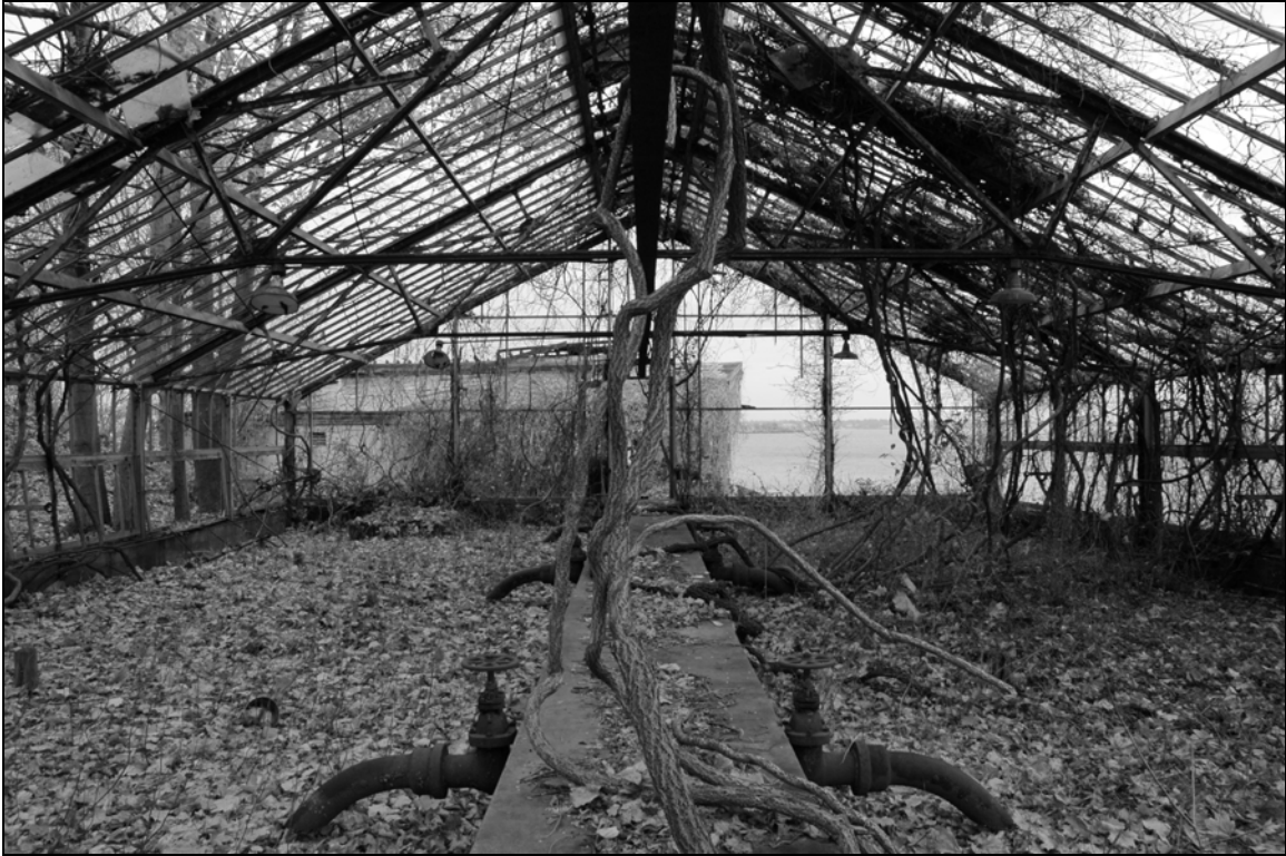
Photo 2. Interior, facing north.
