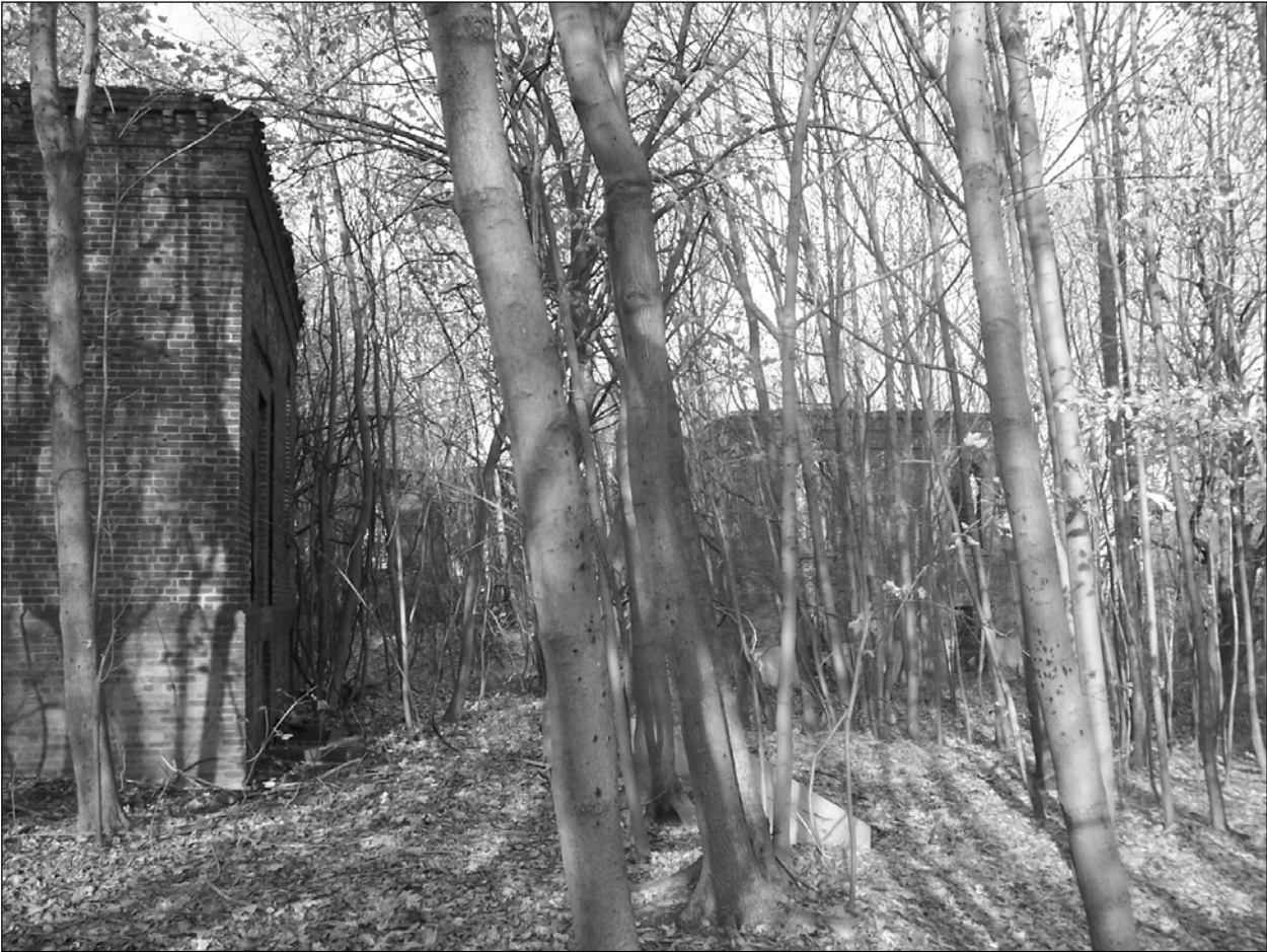
Figure 6. Rear of building, facing north. End of east dependency at left; south dependency is partly visible through trees at right.
