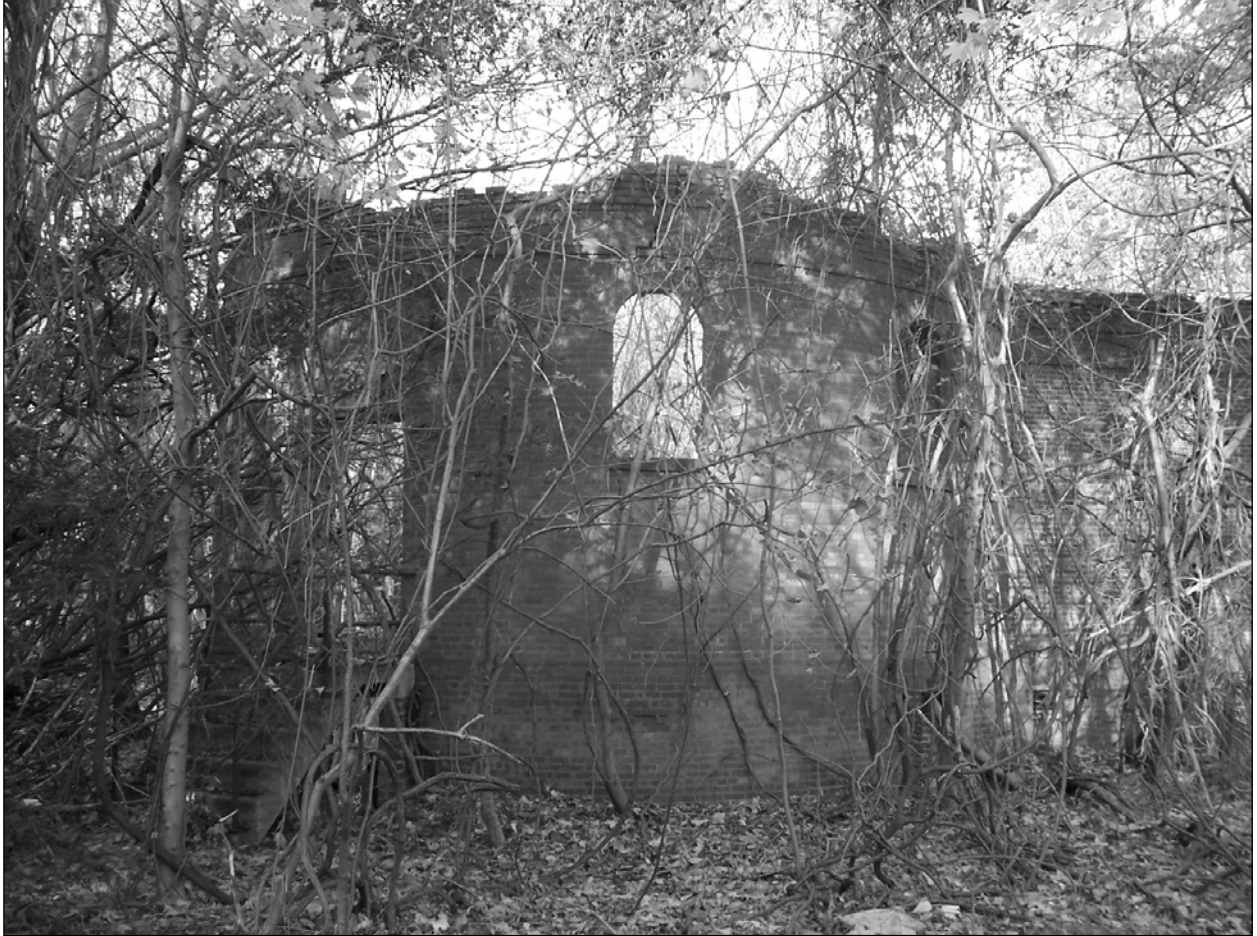
Photo 5. Apse at end of south main wing, facing north. Note stairway installed during late alteration at left and western end of attached dependency at right.
