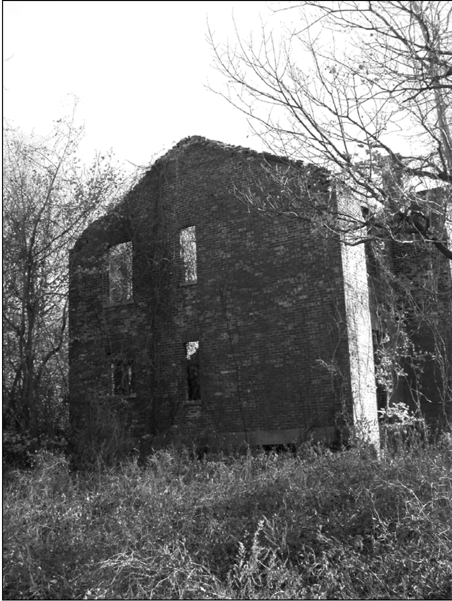
Photo 6. Northern façade, facing southeast.
