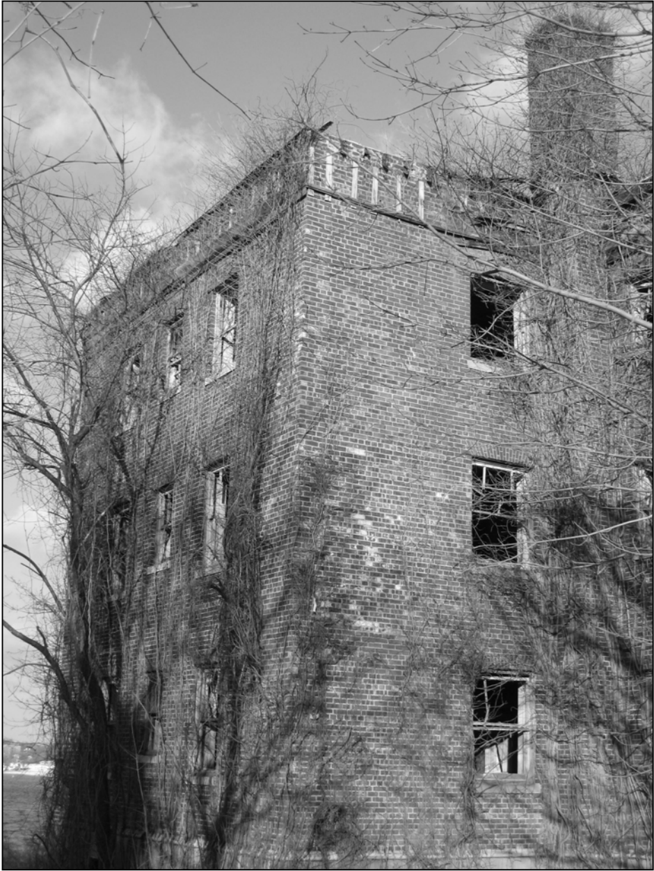
Photo 8. South façade, looking northeast.
