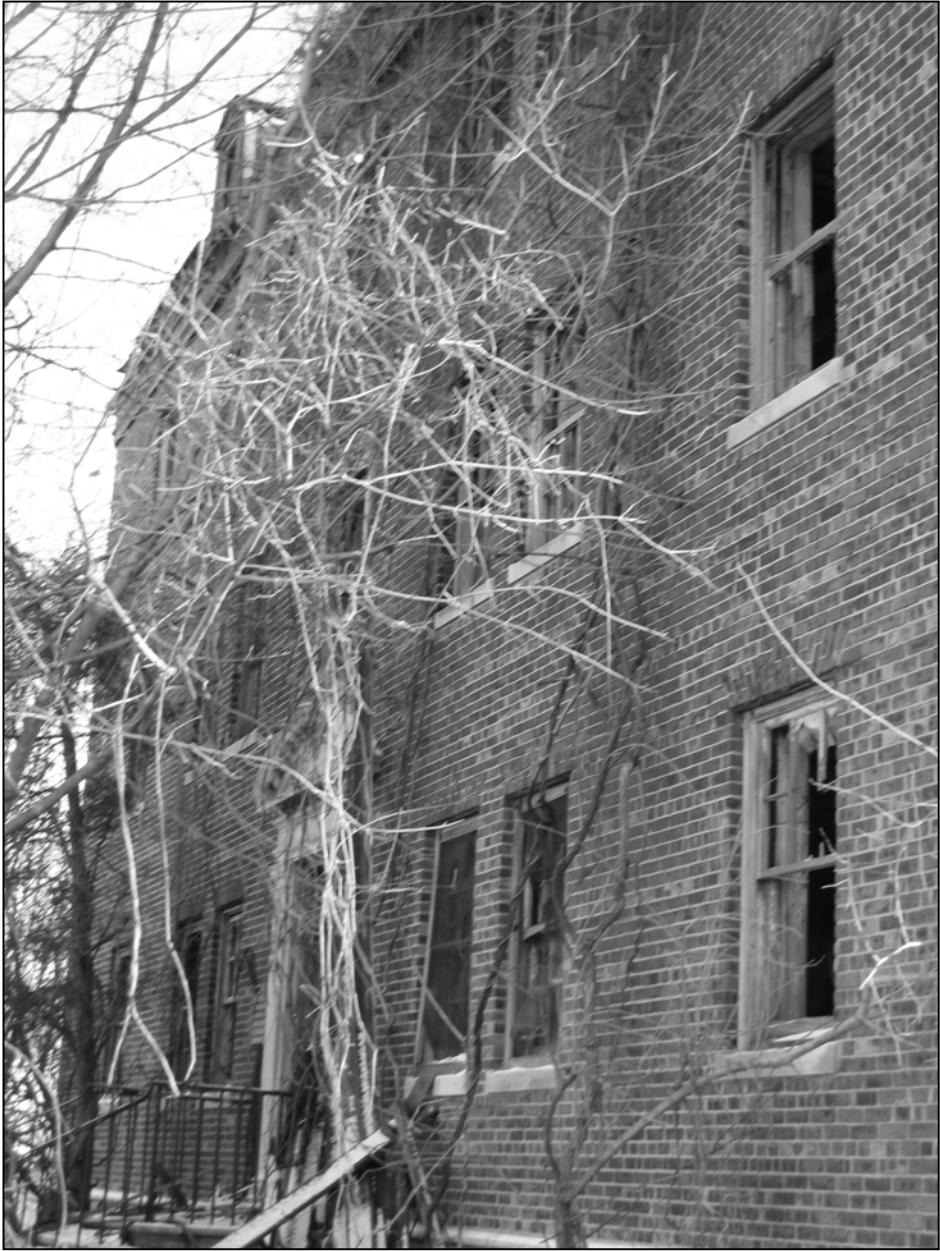
Photo 10. West façade, looking northeast.
