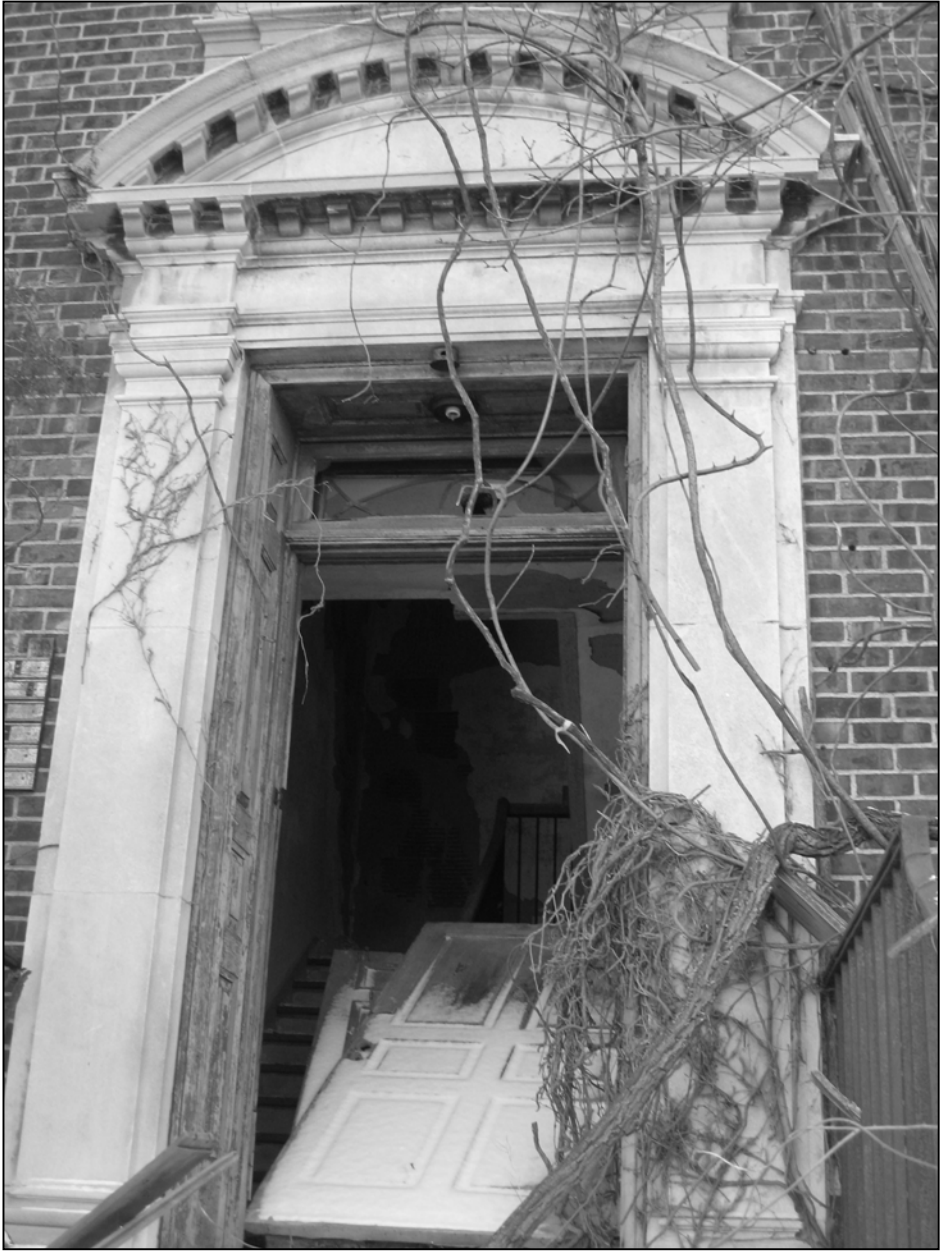
Photo 12. West façade, detail.
