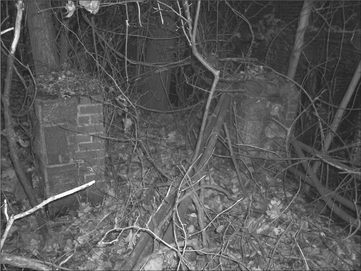
Photo 4. Brick and schist-block piers for front (south) porch, looking northwest.
