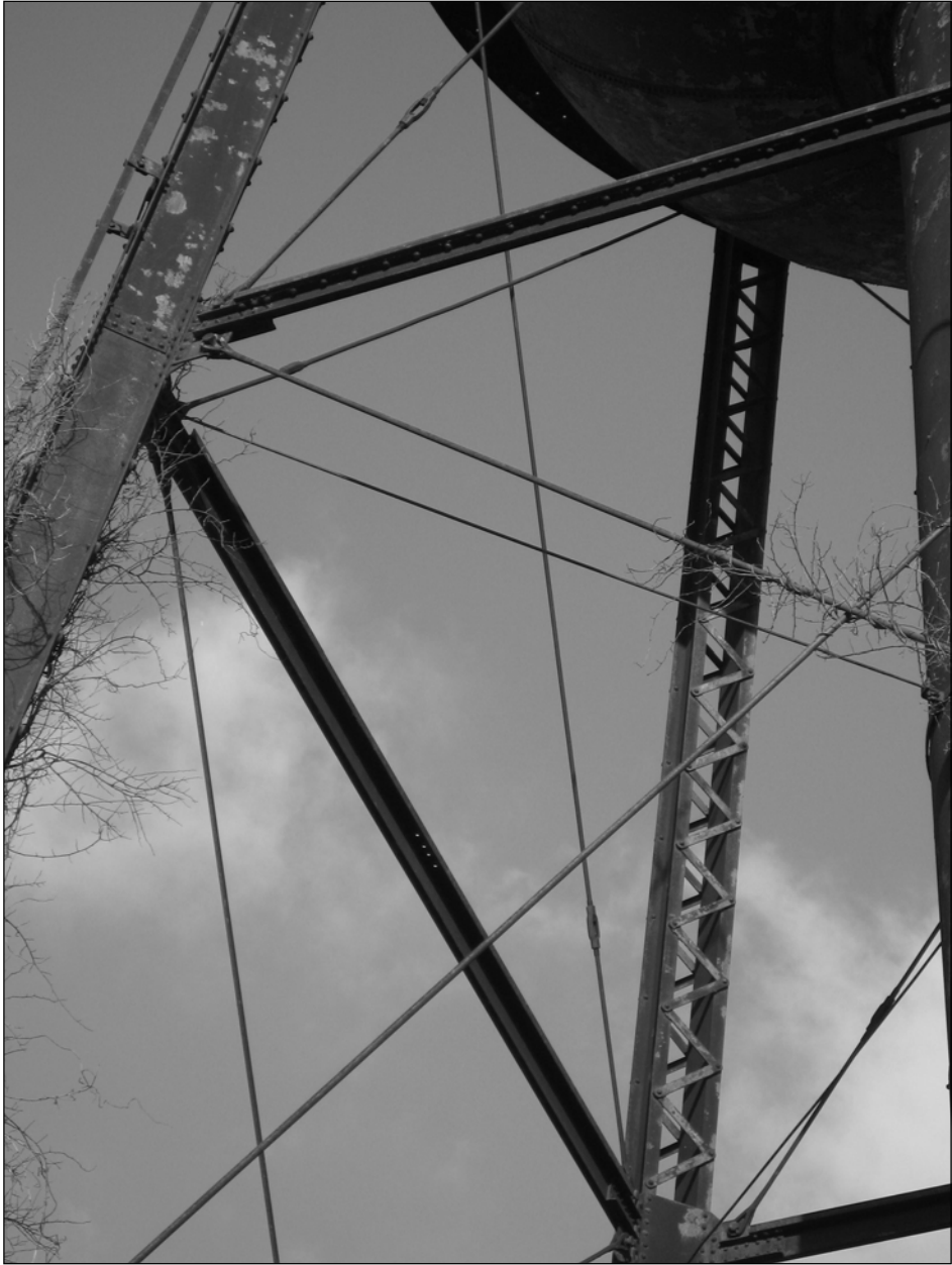
Photo 6. Detail showing tower legs, horizontal bracing, and steel rod cross-braces.
