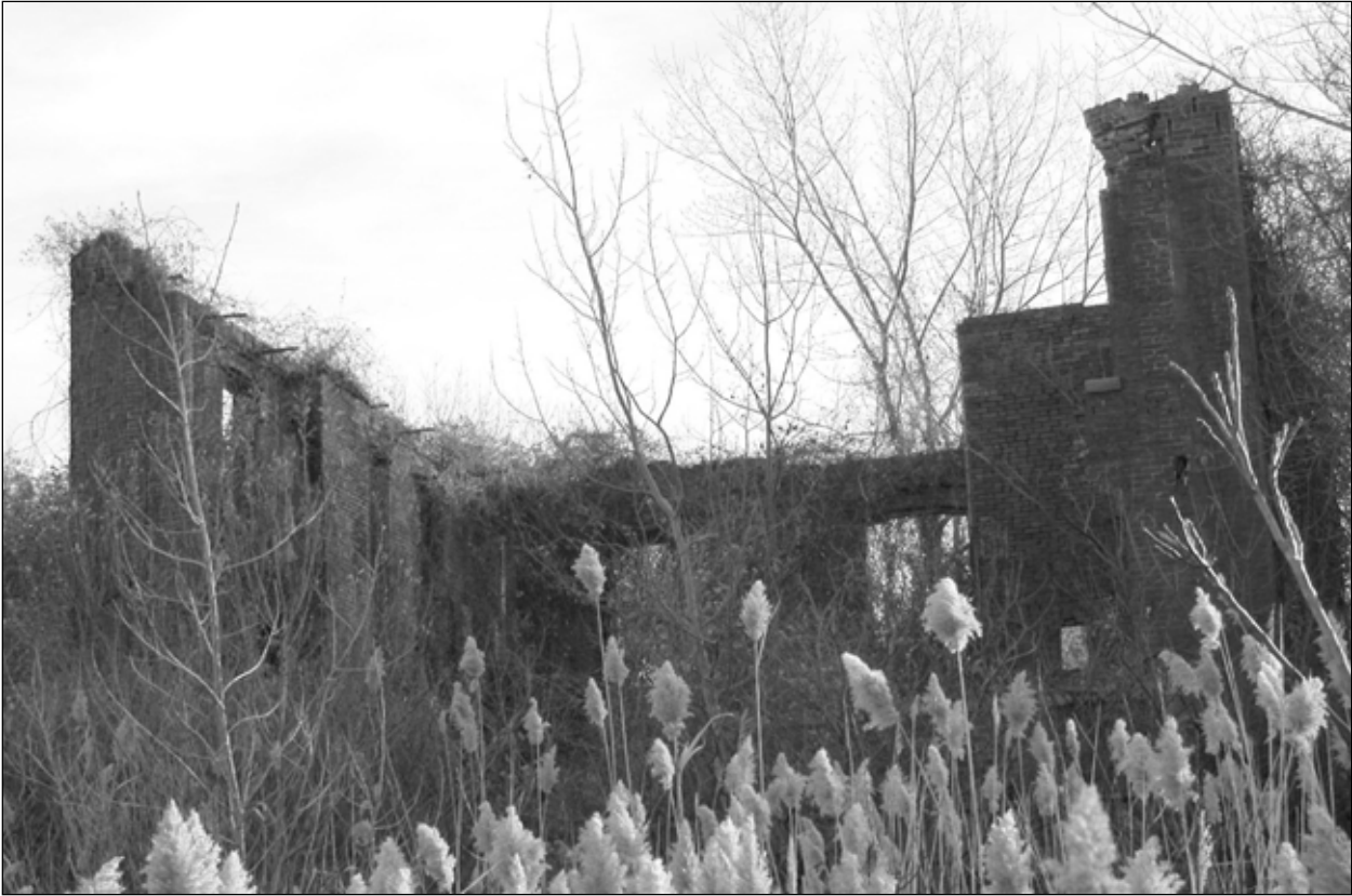
Photo 7. Northern end of building, looking south.
