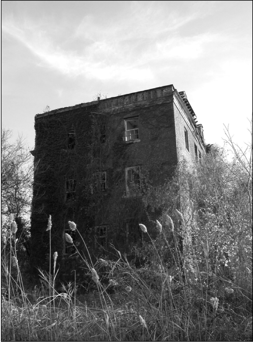
Photo 5. North façade, looking south.
