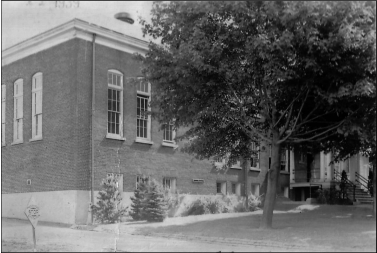
Figure 7. Inventory photograph, September 1939. View northeast showing the tall windows that lit the two-story room at the western end of the building. Record Group 77, National Archives, College Park, MD.
