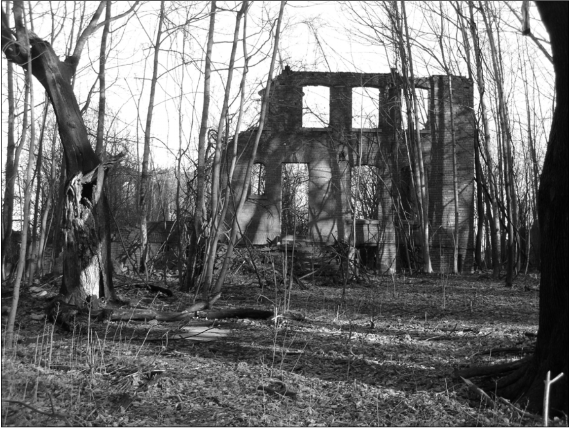
Photo 2. Eastern end of southern façade, facing north.
