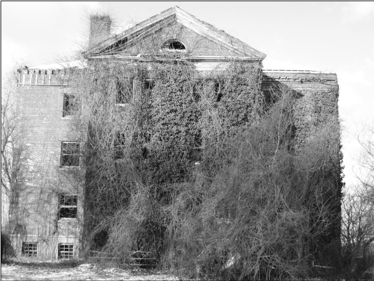
Photo 7. East façade, looking west.
