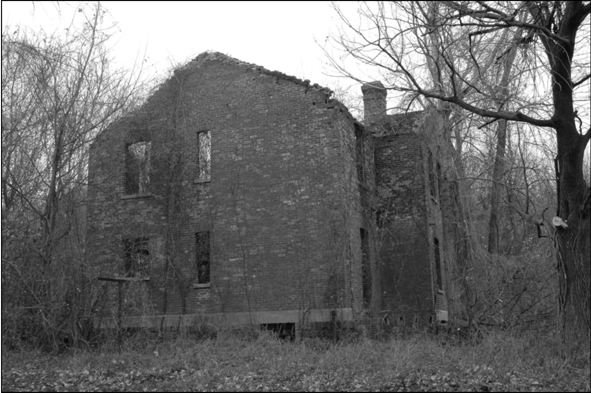
Photo 1. Northern façade, facing south.
