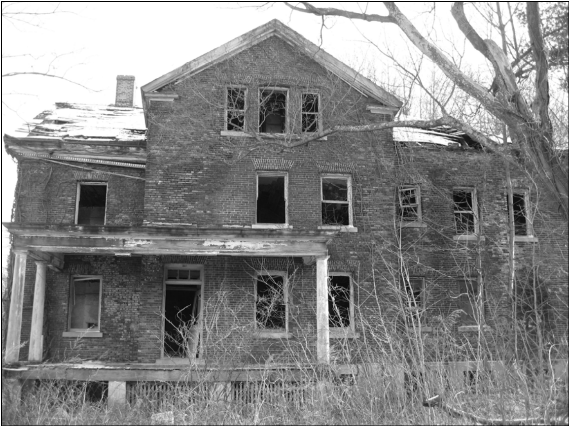
Photo 7. Southwestern façade, facing northeast.
