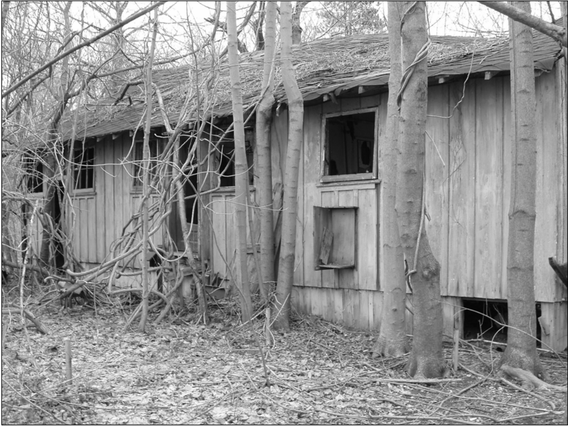
Photo 2. Northwestern façade, facing northeast.
