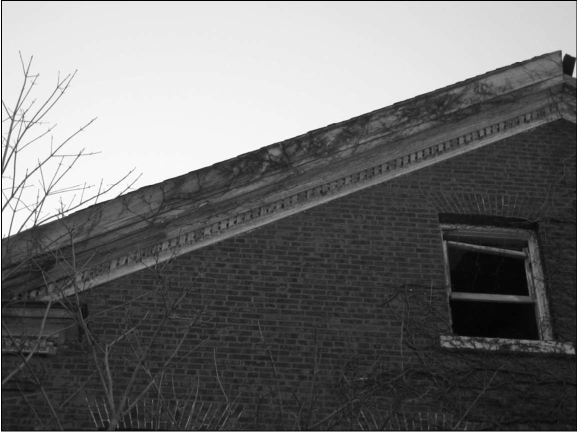
Photo 2. Northwestern façade, detail of gable cornice.
