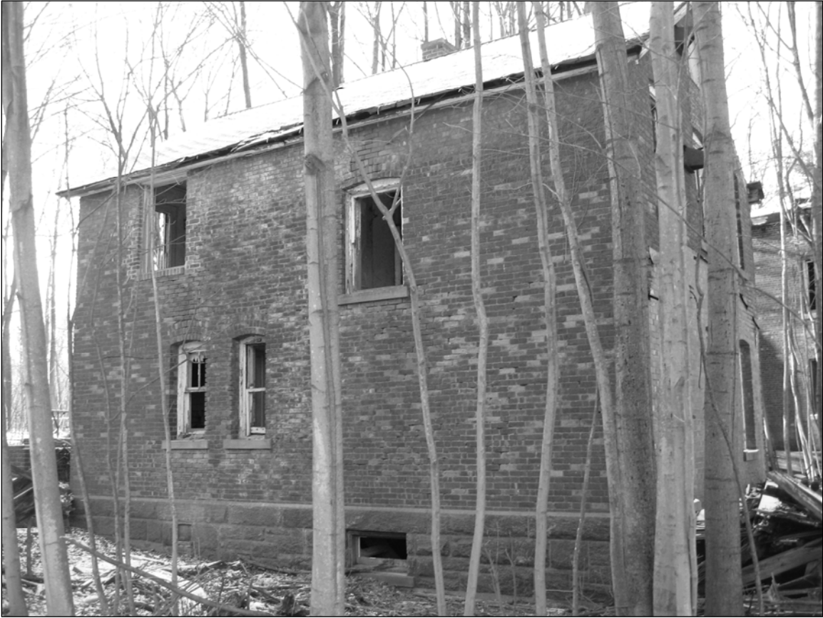
Photo 2. Northeastern façade, facing south.
