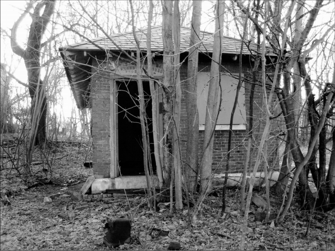
Photo 2 Northwestern façade, facing southeast.
