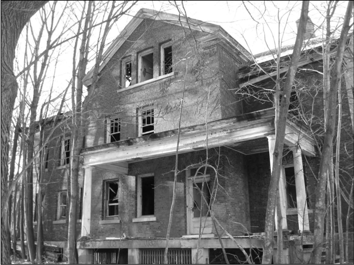
Photo 3. Northeastern façade, facing south.
