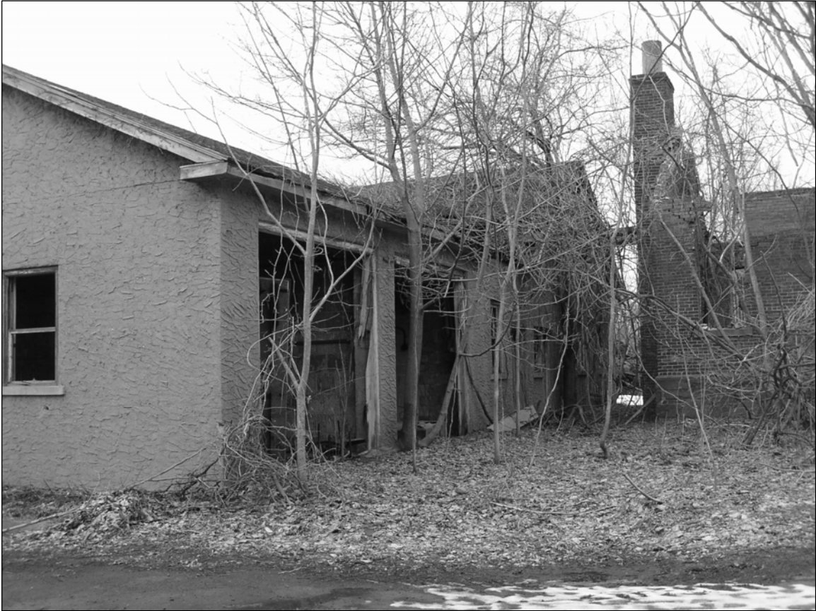
Photo 9. Eastern wing section of eastern façade, facing north-northwest.
