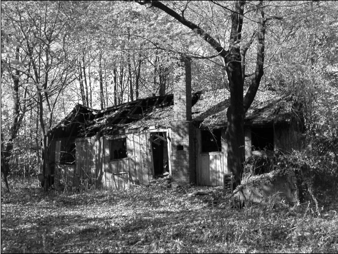
Photo 4. Northeastern façade, facing northwest.
