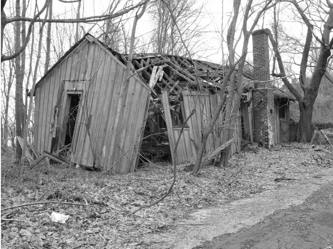
Photo 1. Southwestern and southeastern façades, facing north.
