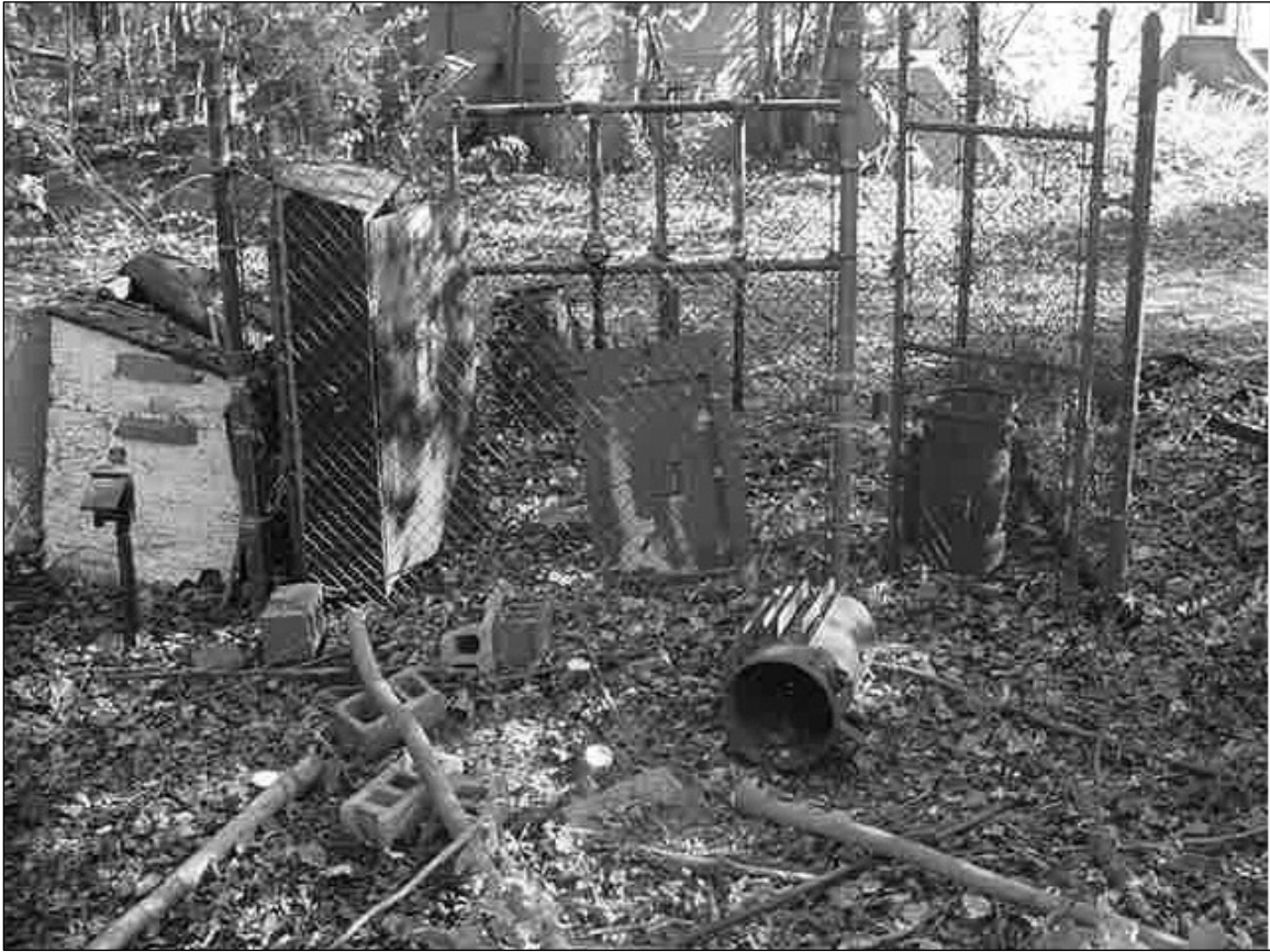
Photo 3. Building 32A immediately prior to demolition, facing southeast.
