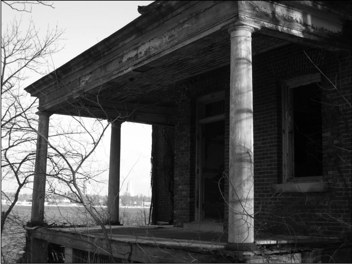
Photo 9. Southwestern façade, detail of porch.
