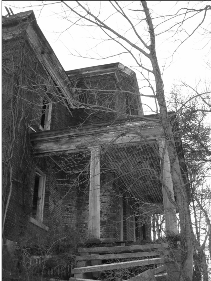
Photo 8. Southwestern façade, detail of porch and front steps.
