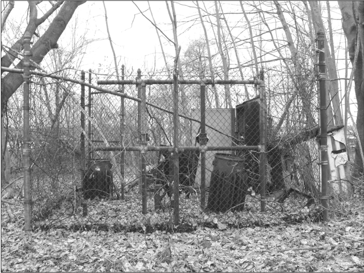
Photo 2. Building 32A viewed from Howard Road, facing northwest.
