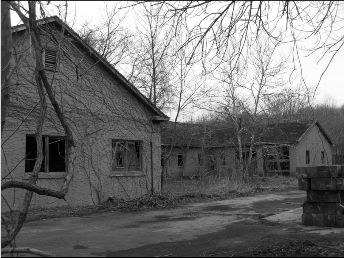
Photo 12. Western addition and courtyard, facing northeast.
