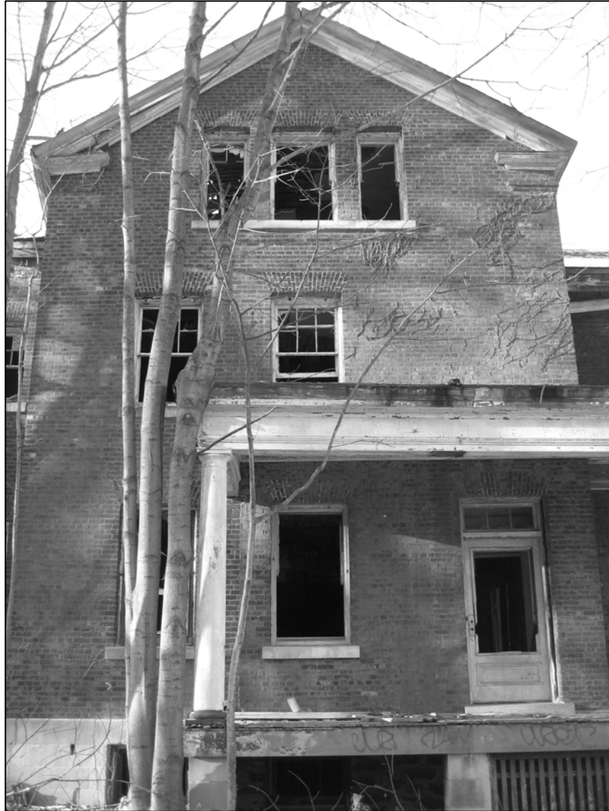
Photo 5. Northeastern façade, cross gable (center) section.
