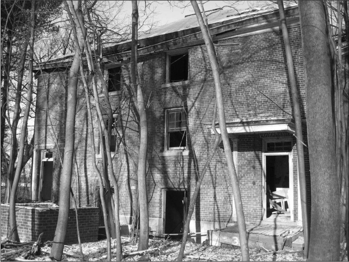
Photo 10. Southeastern (rear) façade, facing northwest.
