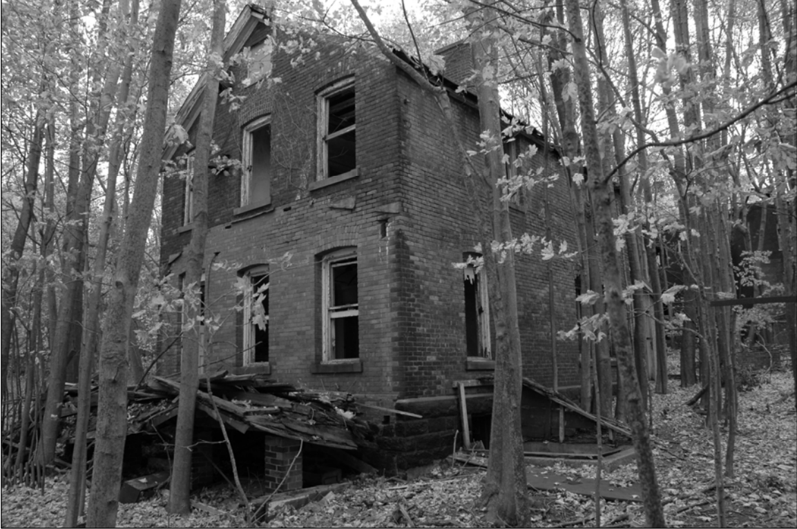
Photo 1. Northwestern façade, facing east.
