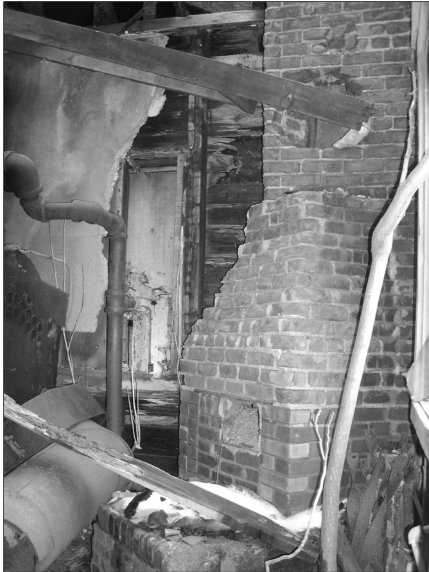
Photo 3. Interior—boiler room in western end of building, facing south.
