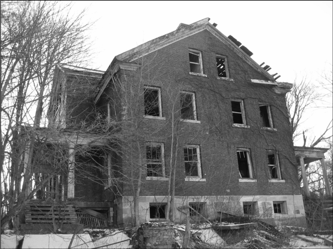
Photo 1. Northwestern (front) façade, facing southeast.
