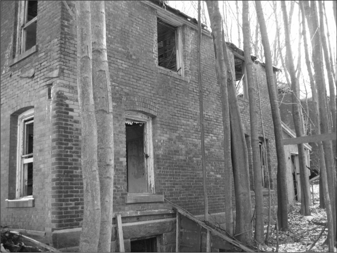
Photo 4. Southwestern façade, facing northeast.
