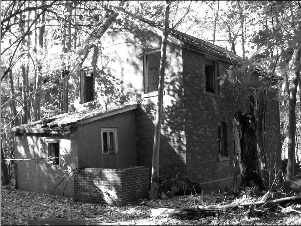
Photo 3. Southeastern and northeastern façades, facing west.
