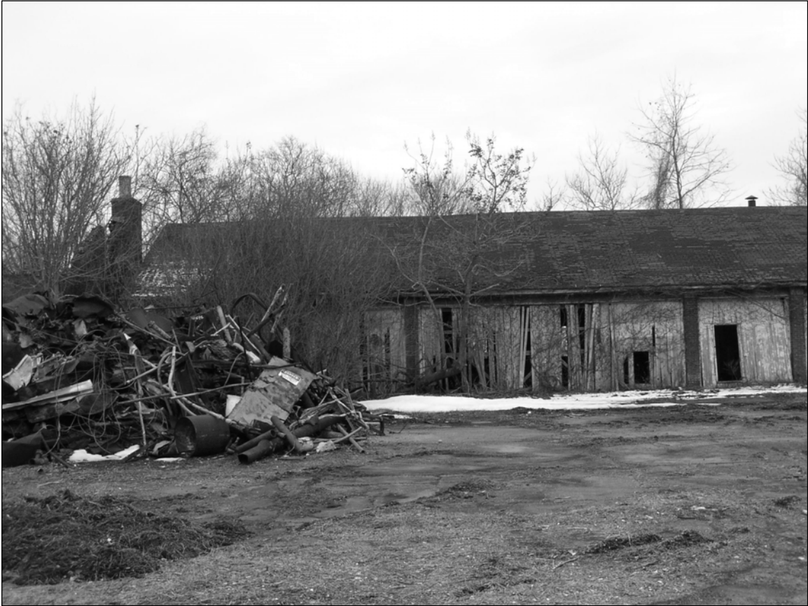
Photo 7. Eastern end of northern façade, facing south.
