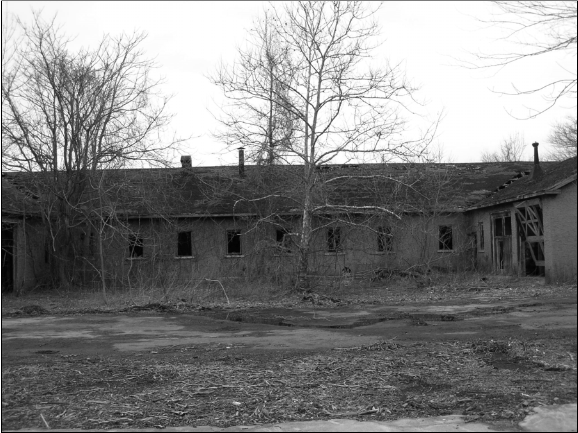
Photo 11. Courtyard between wings and northern façade, facing south.
