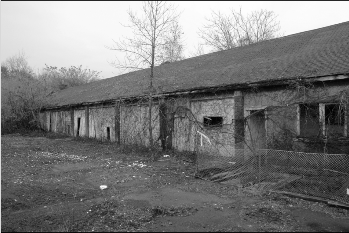
Photo 5. Northern façade, facing southeast.
