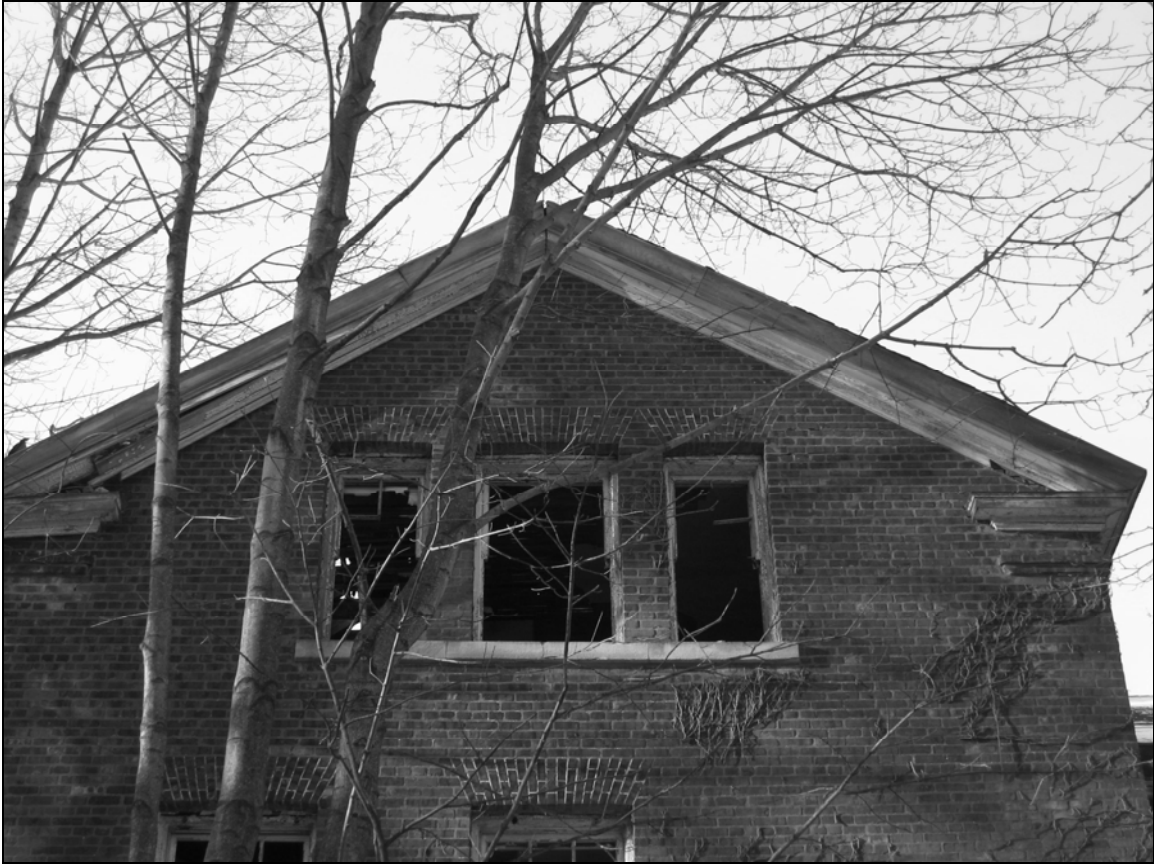
Photo 6. Northeastern façade, detail of cross gable cornice.
