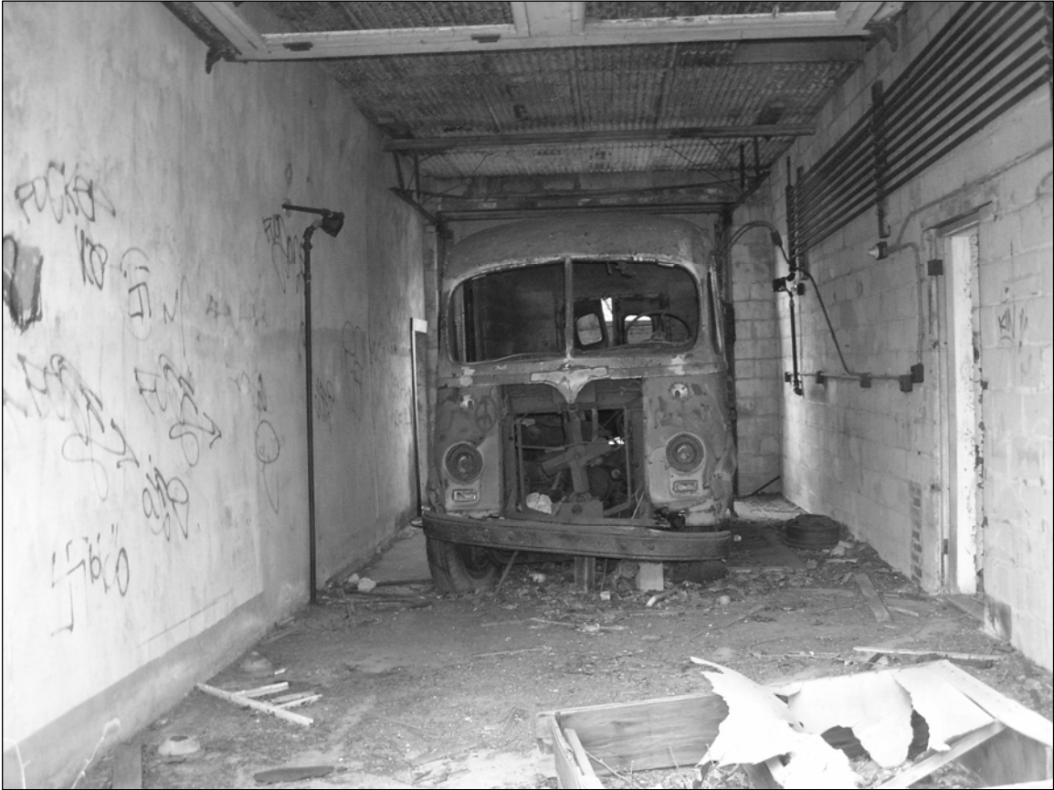
Photo 10. Interior of north vehicle bay of eastern wing, with abandoned step van, looking west.
