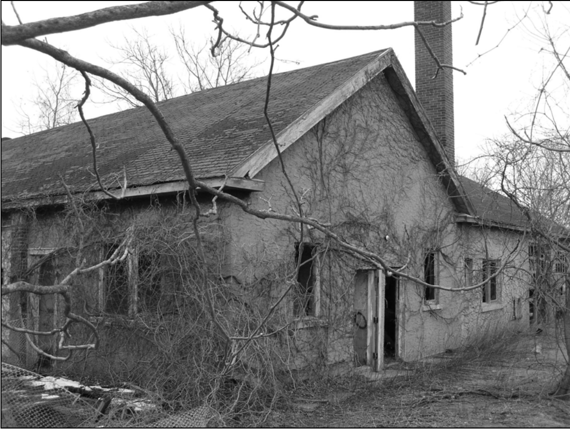
Photo 4. Western and northern façades, facing southeast.
