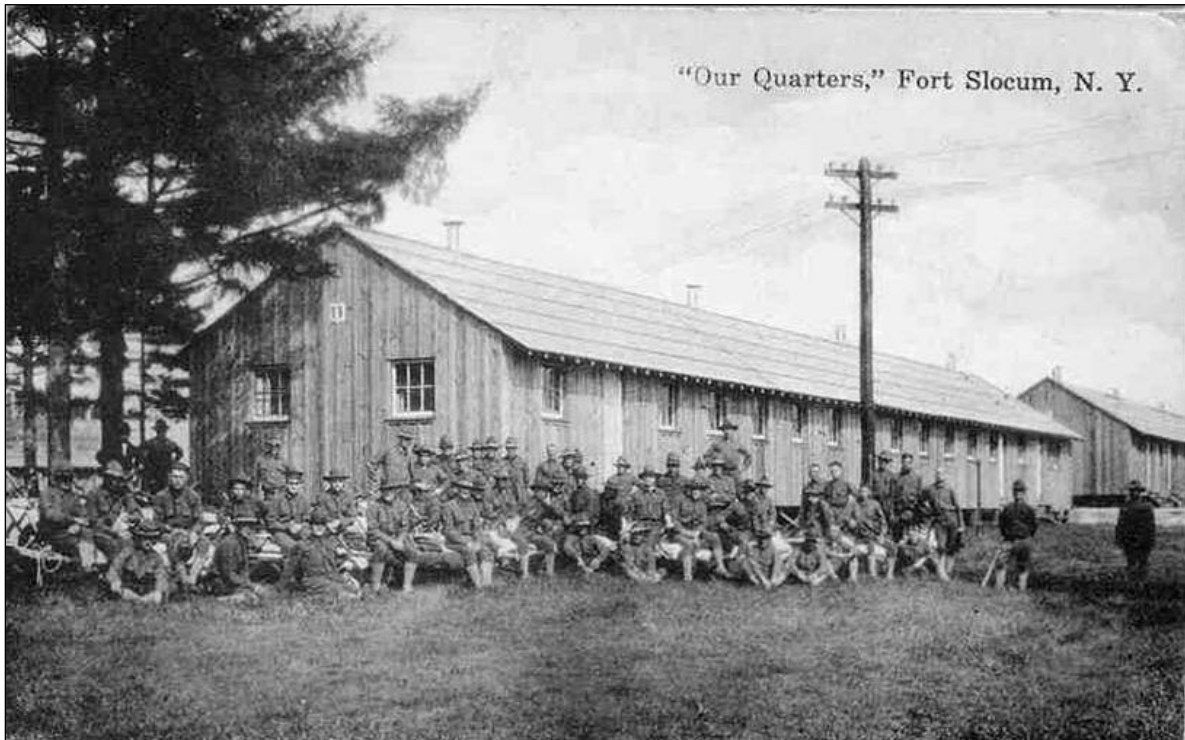
Figure 1. “‘Our Quarters,’ Fort Slocum, N.Y.,’ ca. 1917. Postcard view, unknown type and publisher. This view shows a typical First World War one-story temporary building, with board-and-batten siding and six-pane windows like that of Building T-34. Fort Slocum Alumni and Friends Collection, Michael A. Cavanaugh, Los Angeles, CA, custodian.
