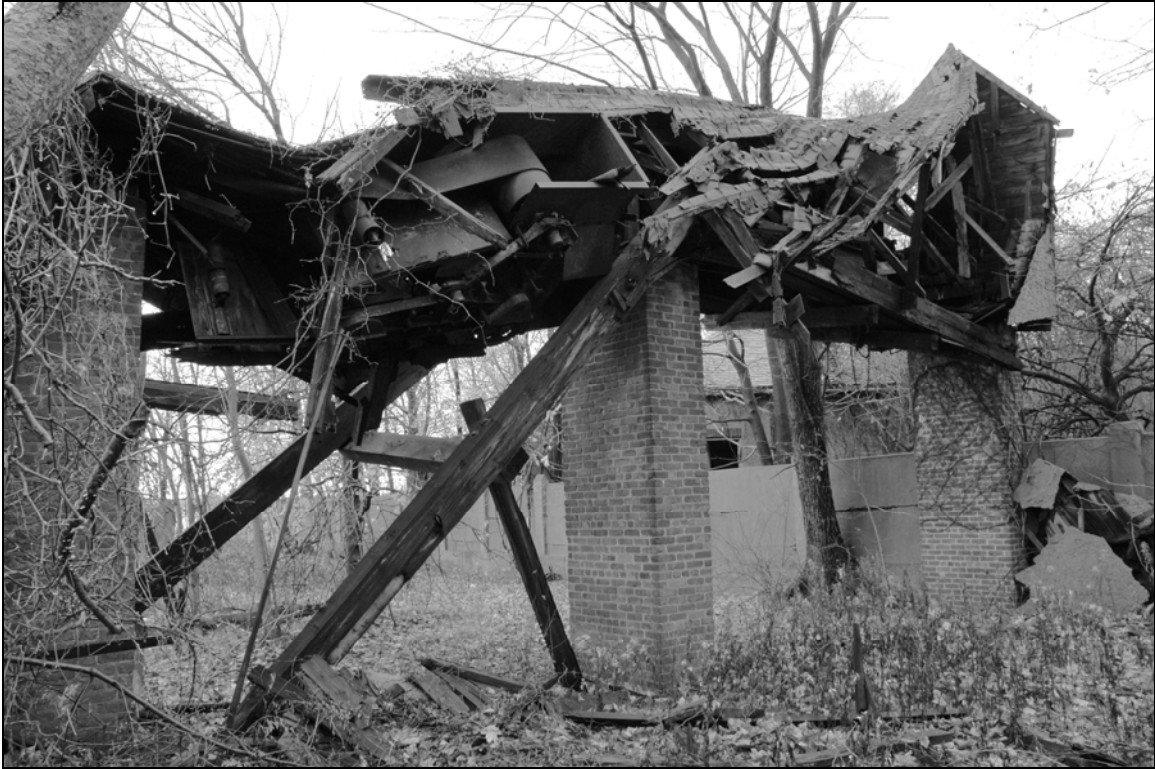
Photo 4. Conveyor belt feature, facing north.
