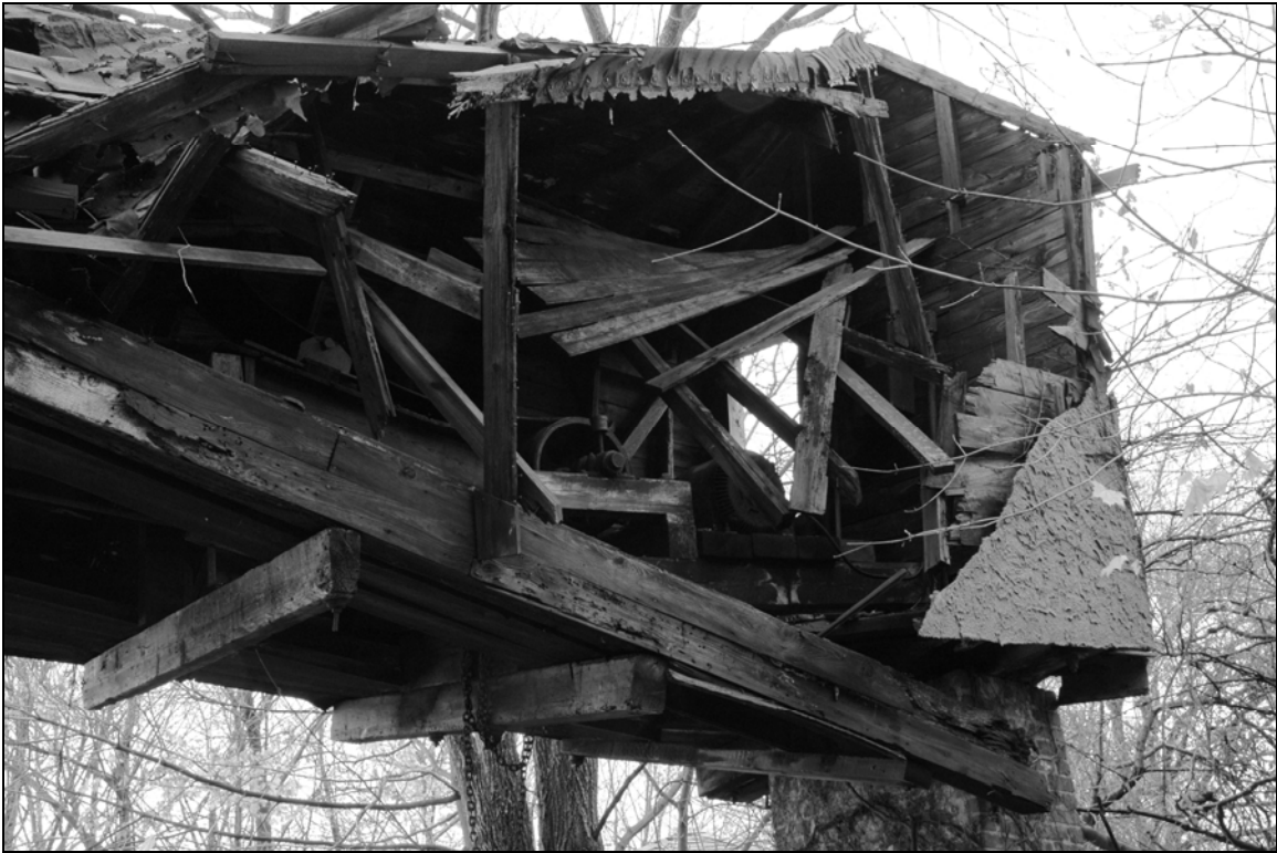
Photo 5. Conveyor belt feature, detail.
