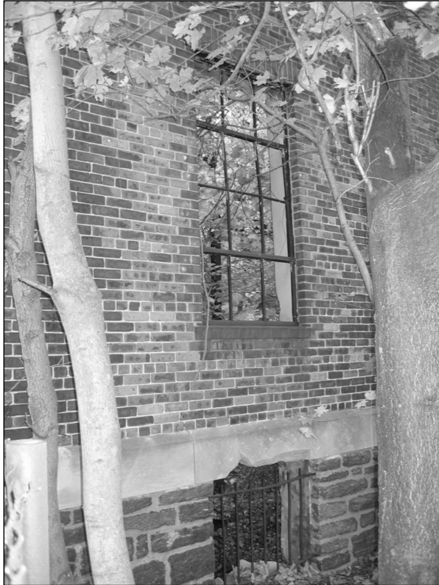
Photo 7. Northern façade, detail.
