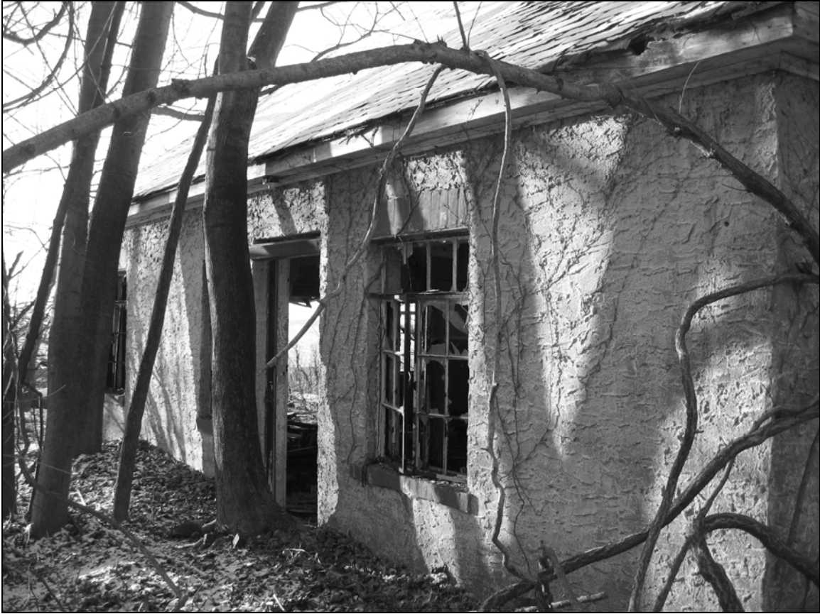
Photo 7. Eastern façade, looking southwest.
