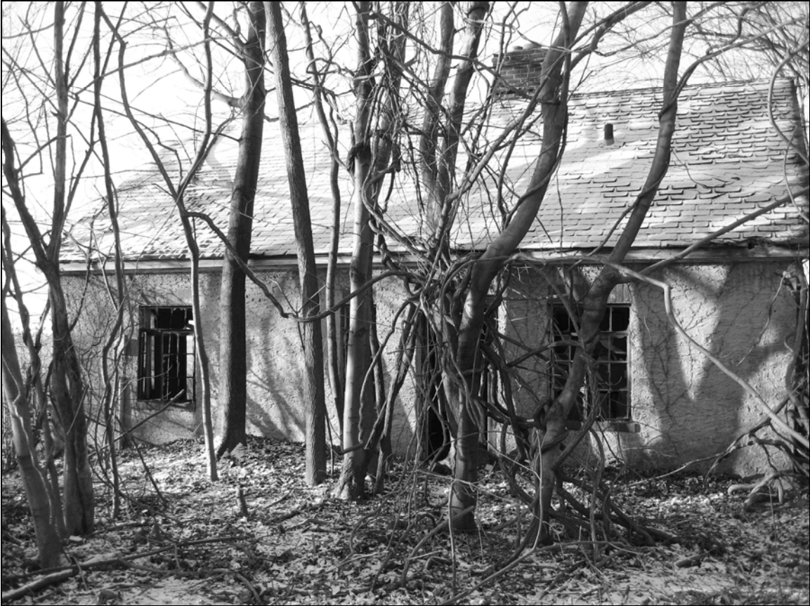
Photo 6. Eastern façade, looking west.
