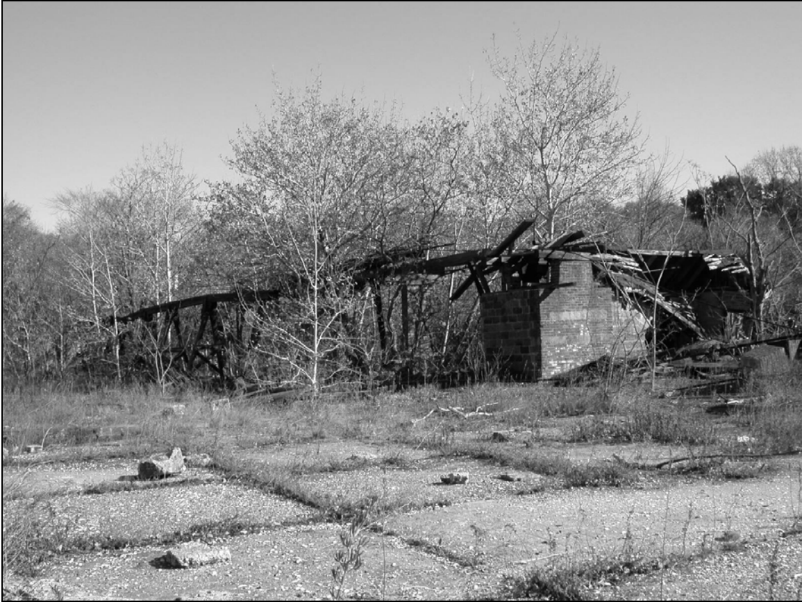
Photo 7. Coal yard and conveyor, facing east-northeast.
