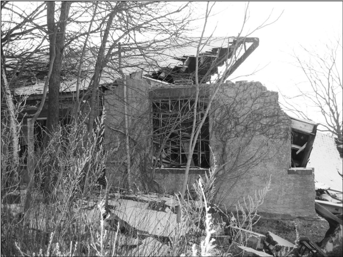
Photo 13. Northern façade, looking south.
