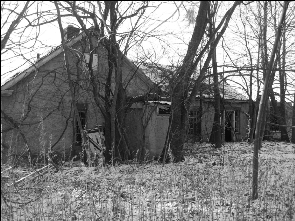
Photo 9. Northern façade, looking south.
