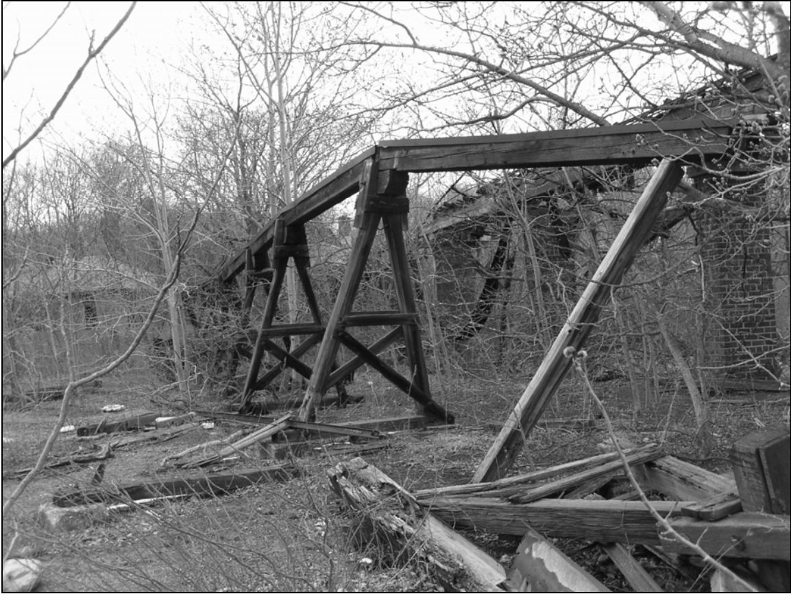
Photo 11. Conveyor, facing east.
