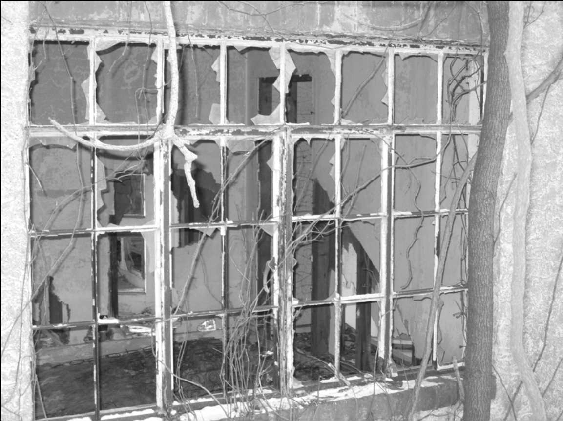
Photo 12. Northern façade, detail.
