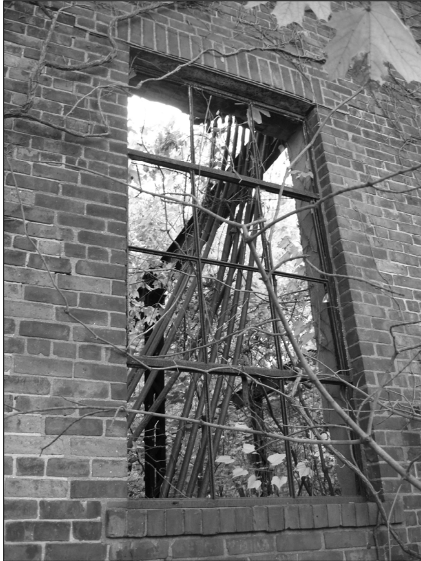
Photo 4. Northern façade, detail.
