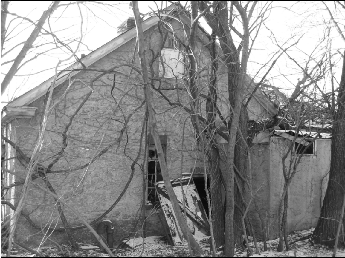
Photo 10. Northern façade, looking south.
