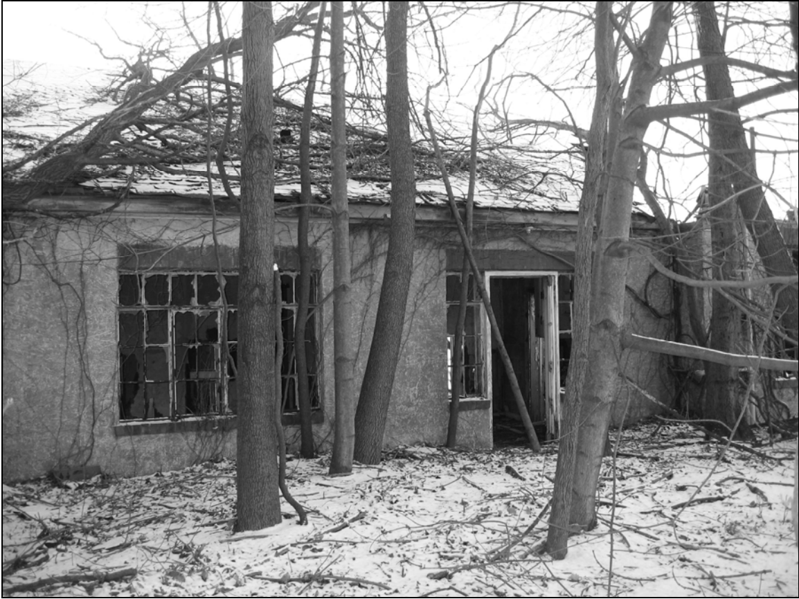
Photo 11. Northern façade, looking south.
