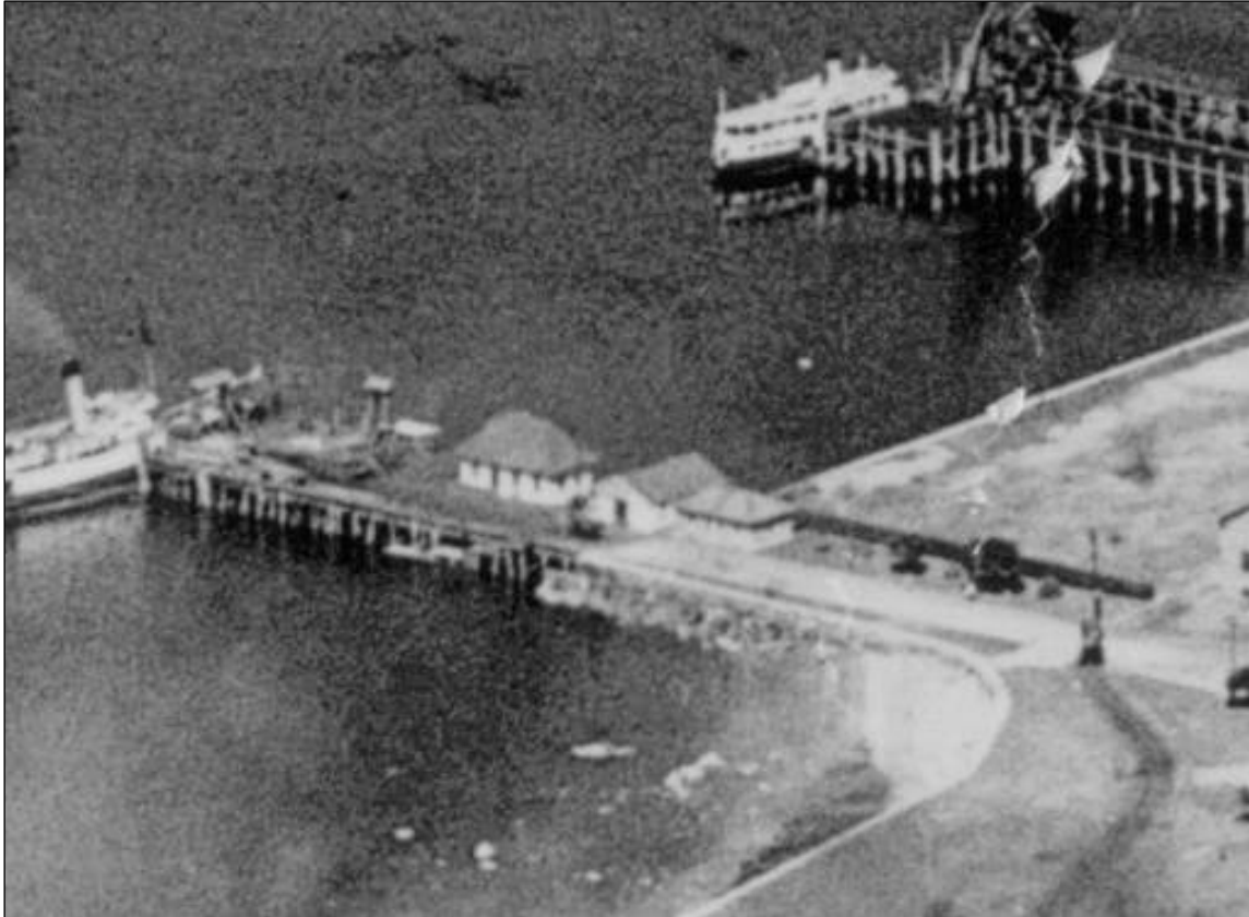
Figure 4. High angle oblique aerial photograph of Davids Island. 1926, detail. View west. Building 30 is the rightmost building along the foreground dock. Original in National Archives, College Park, MD; digital copy from Fort Slocum Alumni and Friends Collection, Michael A. Cavanaugh, Los Angeles, CA, custodian.
