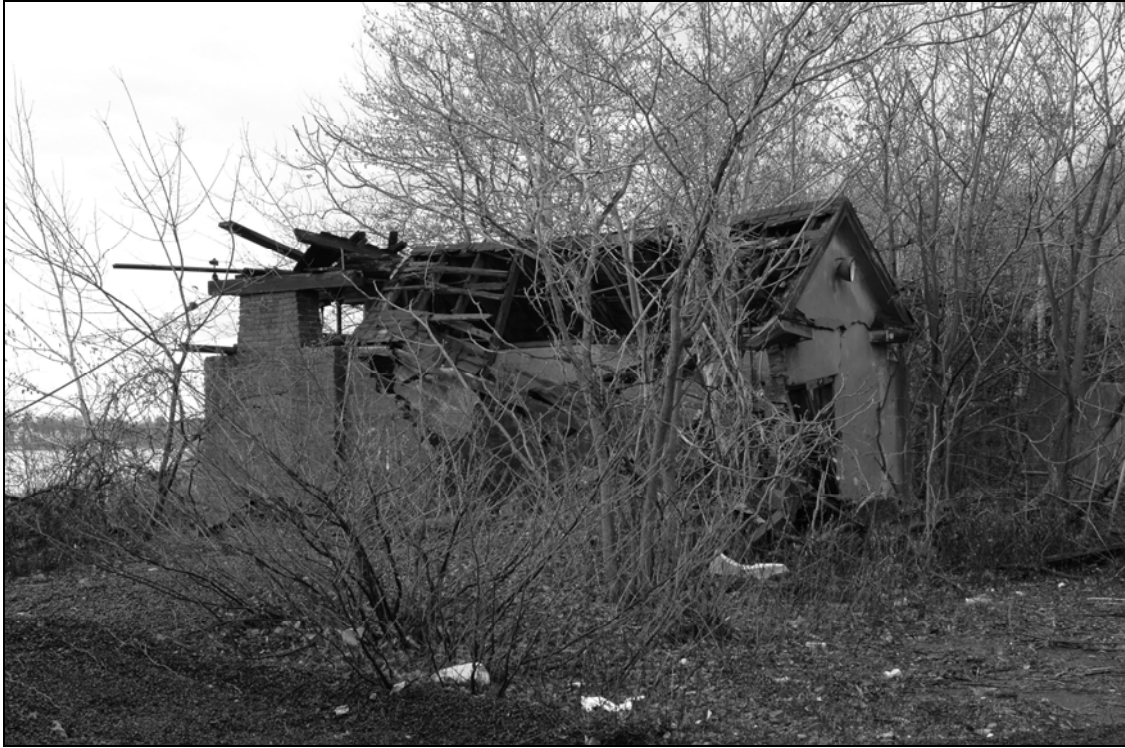
Photo 1. Context of Building 31, facing north-northwest.
