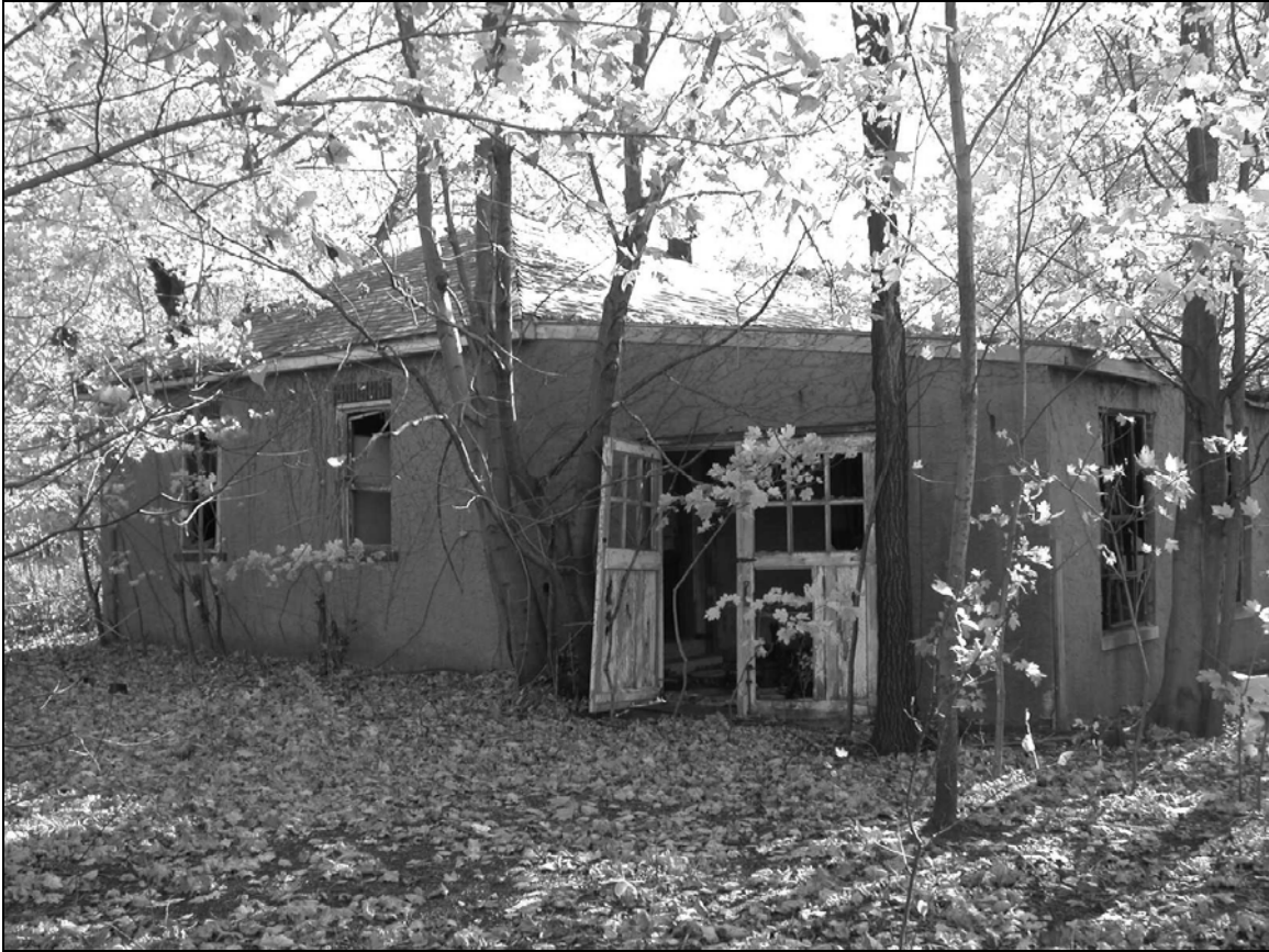
Photo 2. Northern façade, showing attached garage. Facing southeast.
