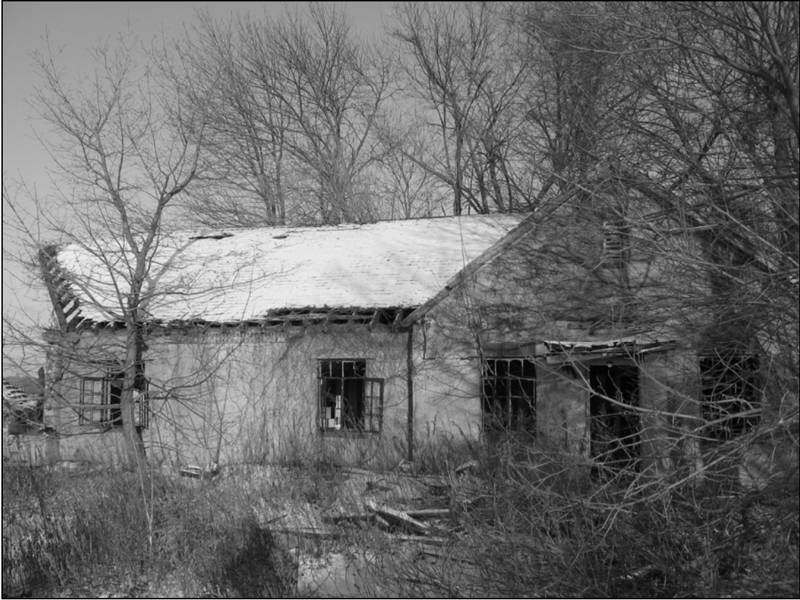
Photo 3. Southern façade, looking northwest.
