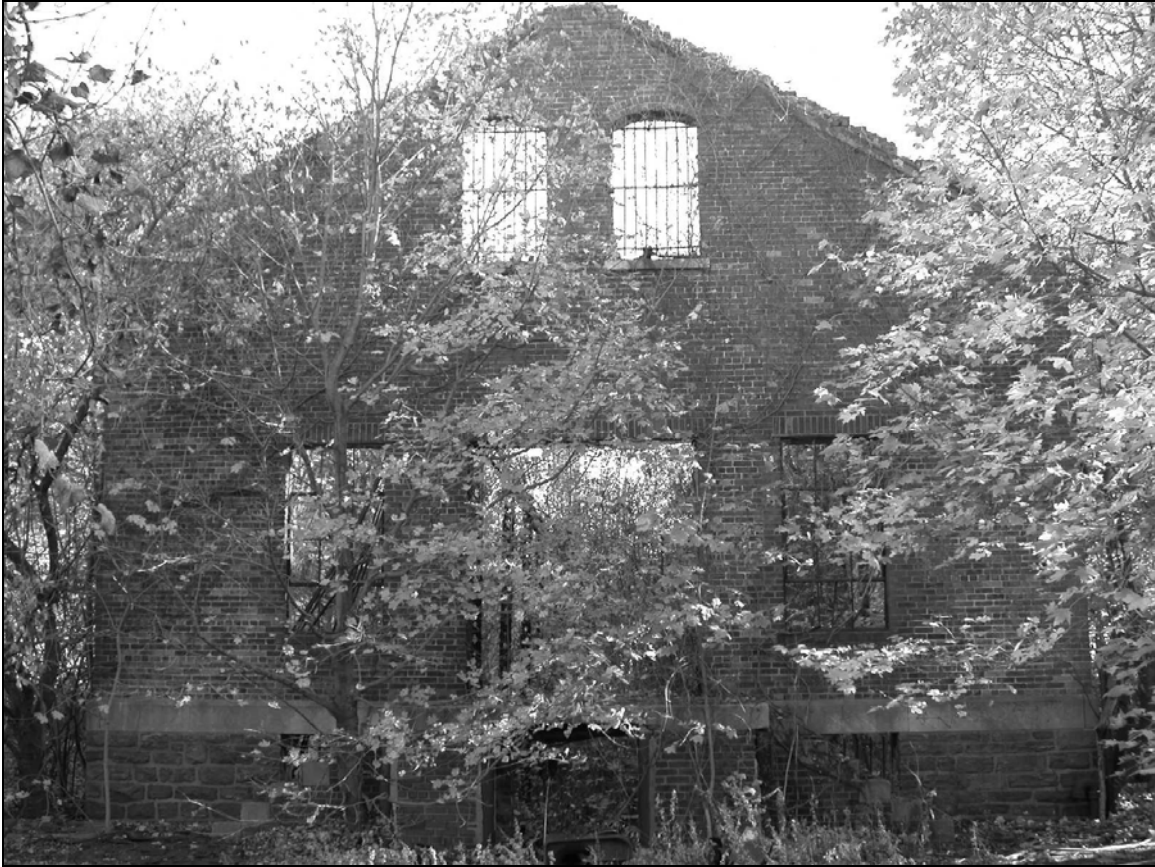
Photo 1. Northern façade, looking south.
