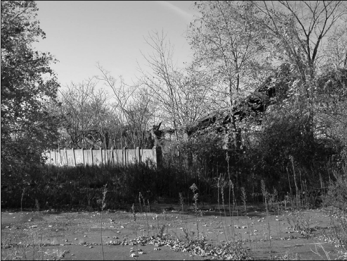
Photo 10. Coal bin, facing west.
