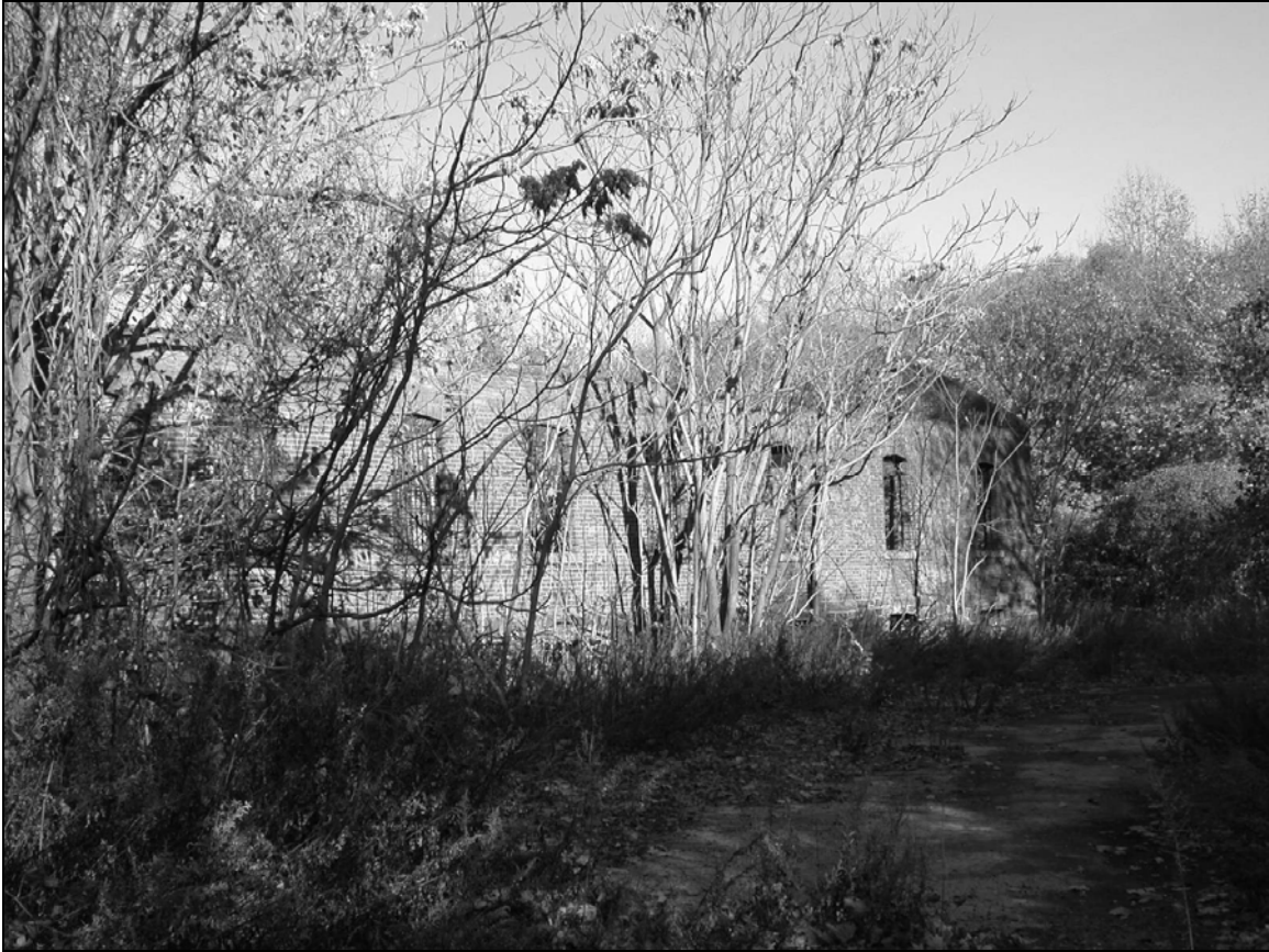
Photo 2. South façade, facing northeast.
