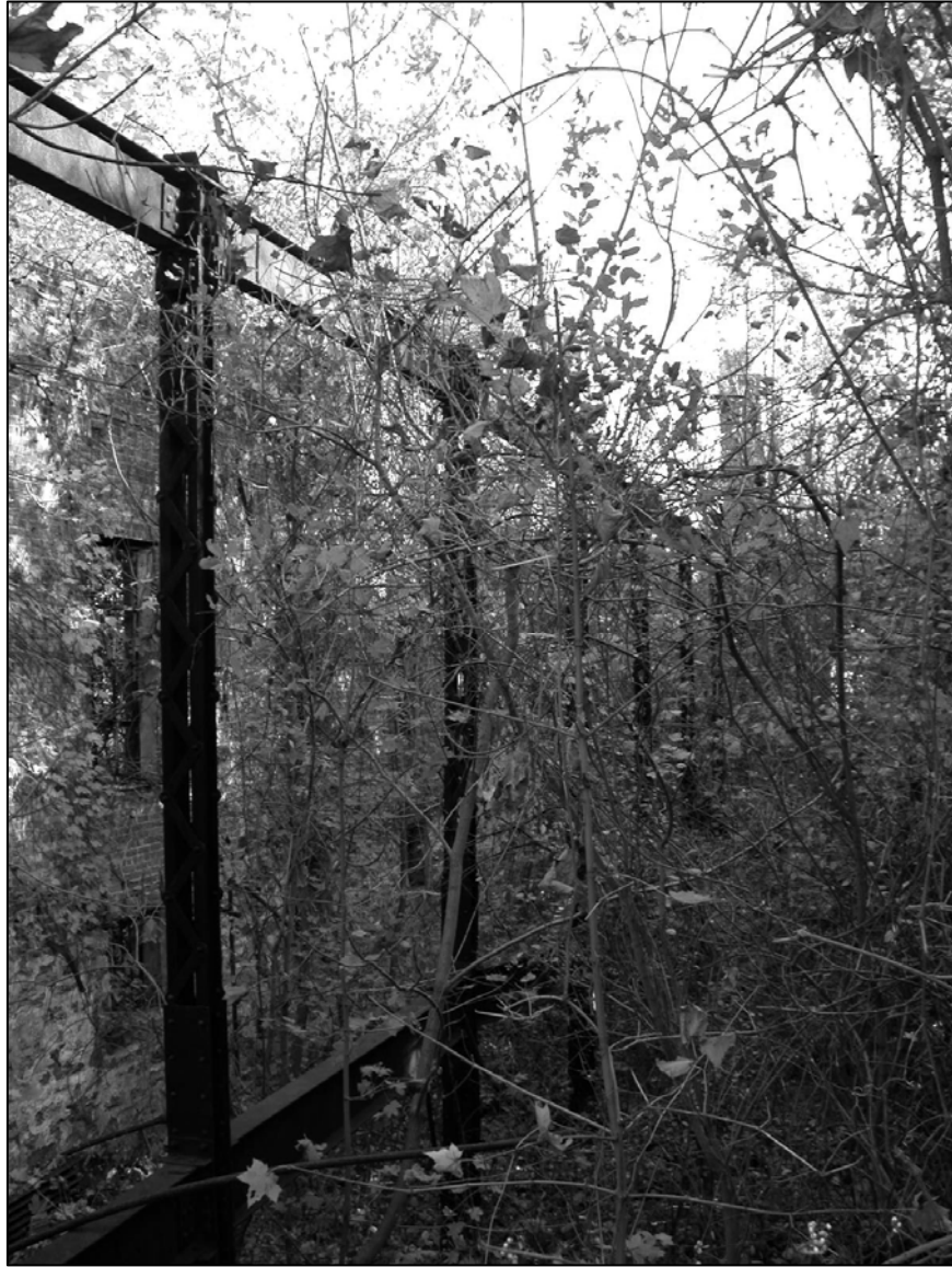
Photo 2. Interior, looking south.
