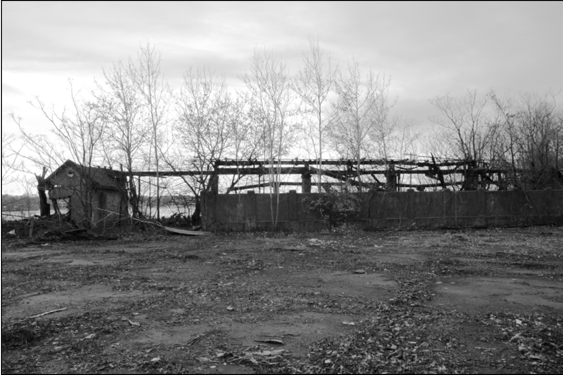
Photo 6. Conveyor belt feature, facing north.
