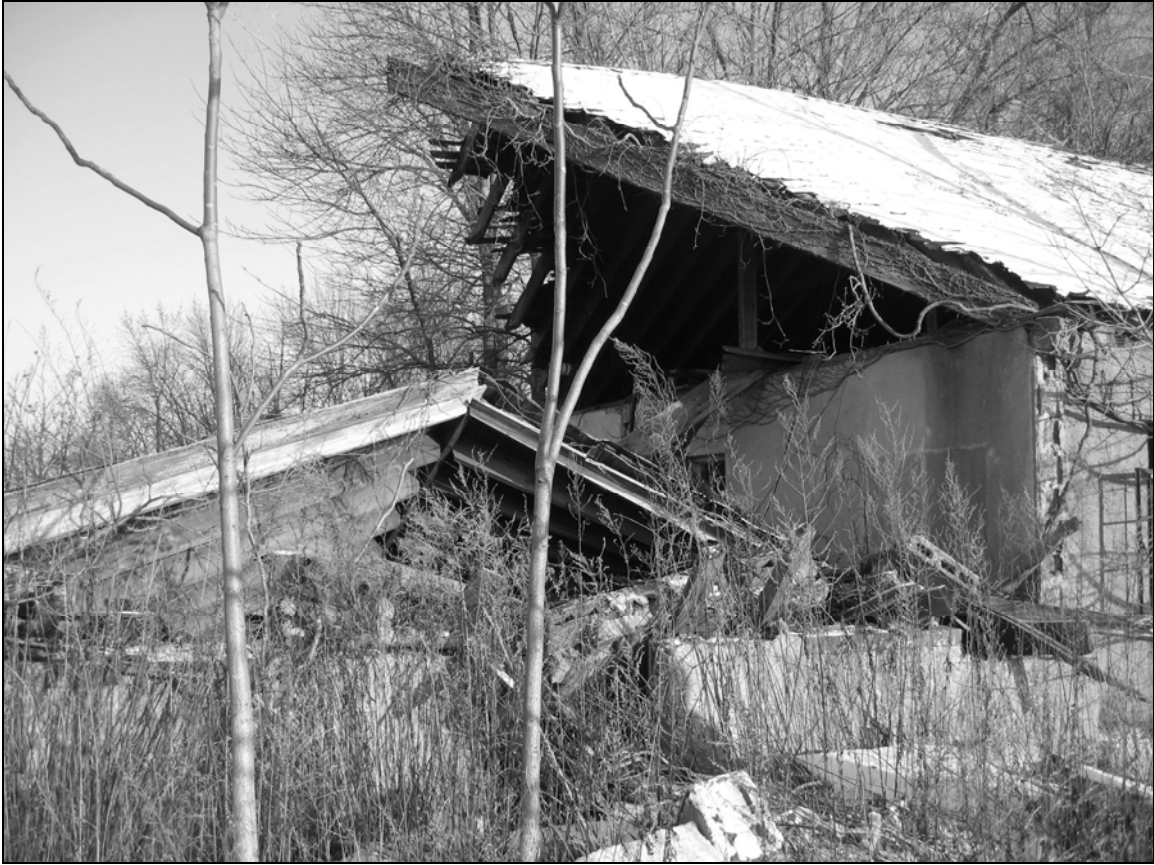
Photo 19. Western façade, looking northeast.
