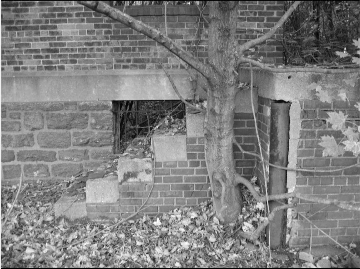
Photo 8. Northern façade, detail.
