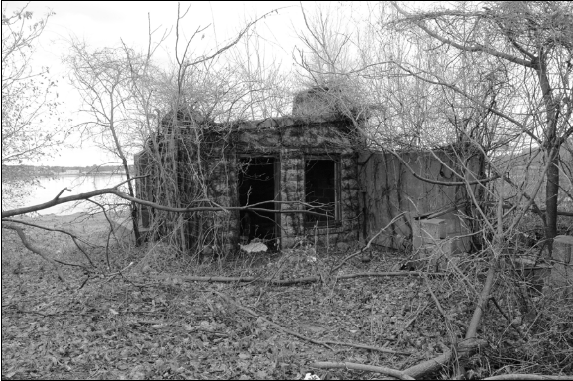
Photo 1. Southeastern façade, facing west.
