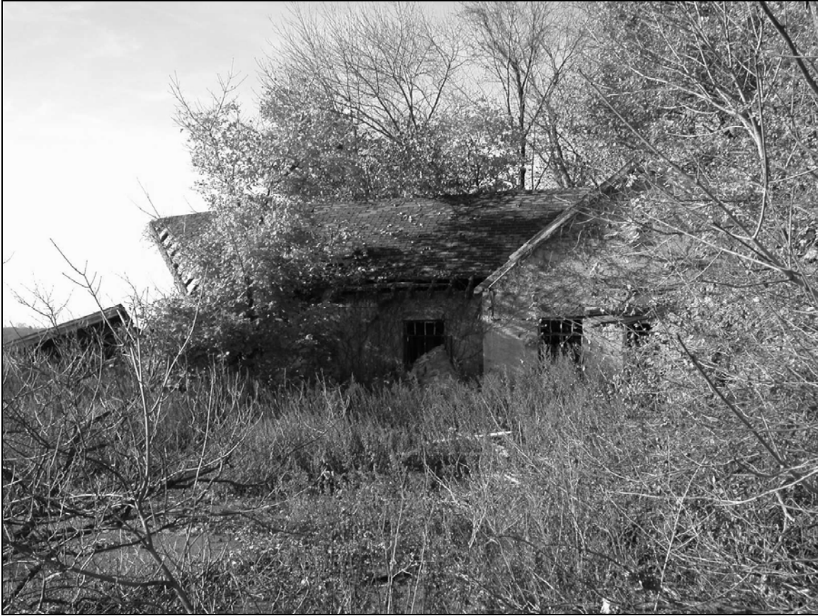
Photo 2. Southern façade, looking northwest.
