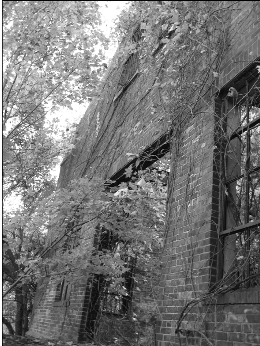
Photo 6. Northern façade, detail.
