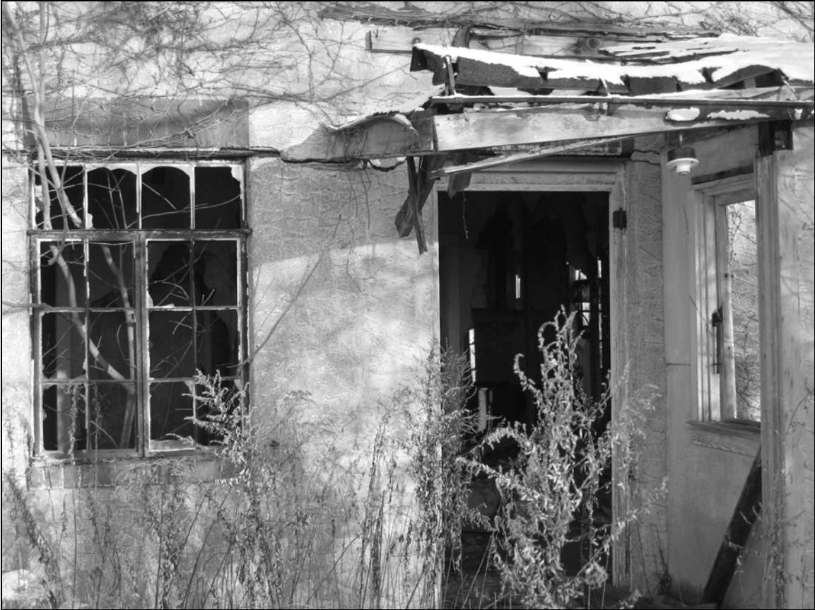
Photo 4. Southern façade, detail.
