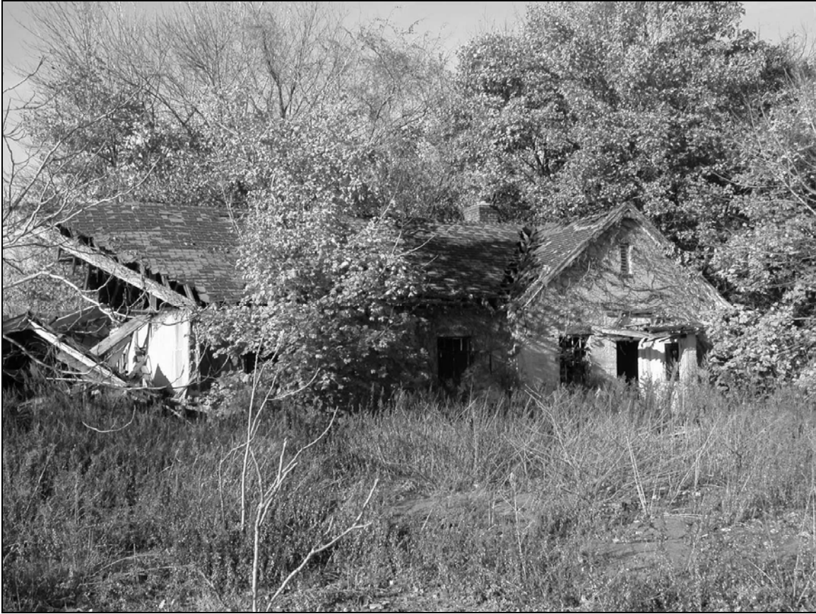
Photo 1. Southern façade, looking north.
