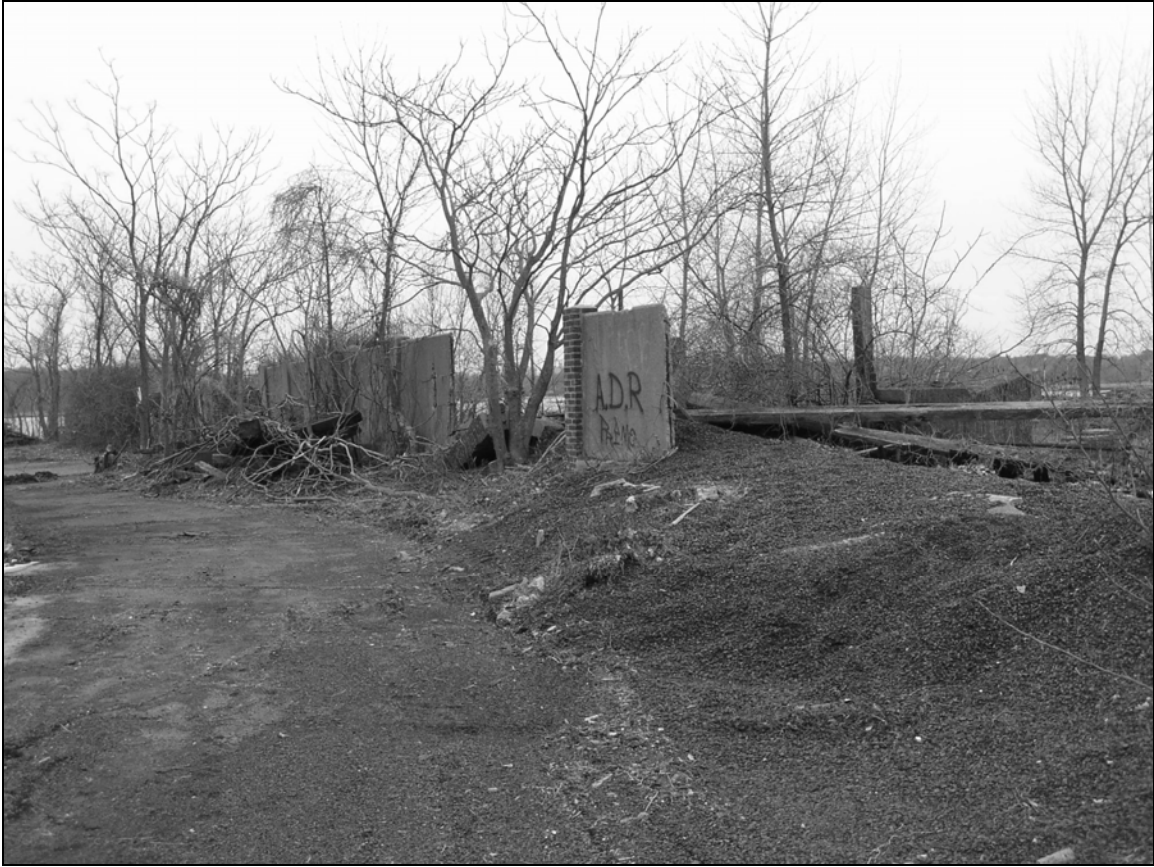
Photo 21. Coal yard, facing west.
