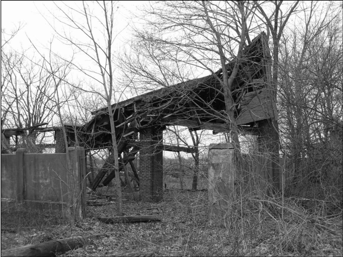
Photo 19. Coal yard and conveyor, facing north.
