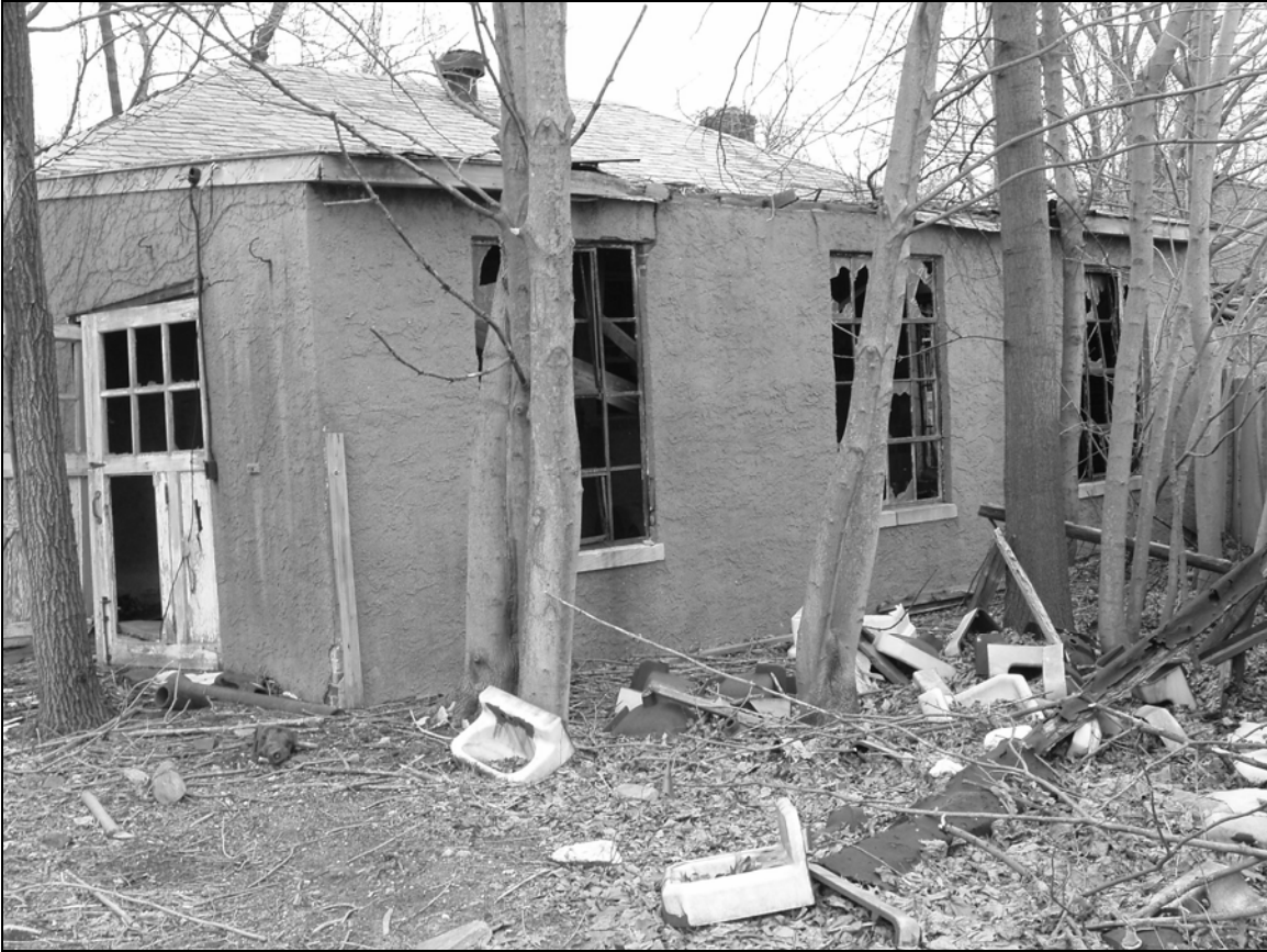
Photo 5. Western façade, facing south.
