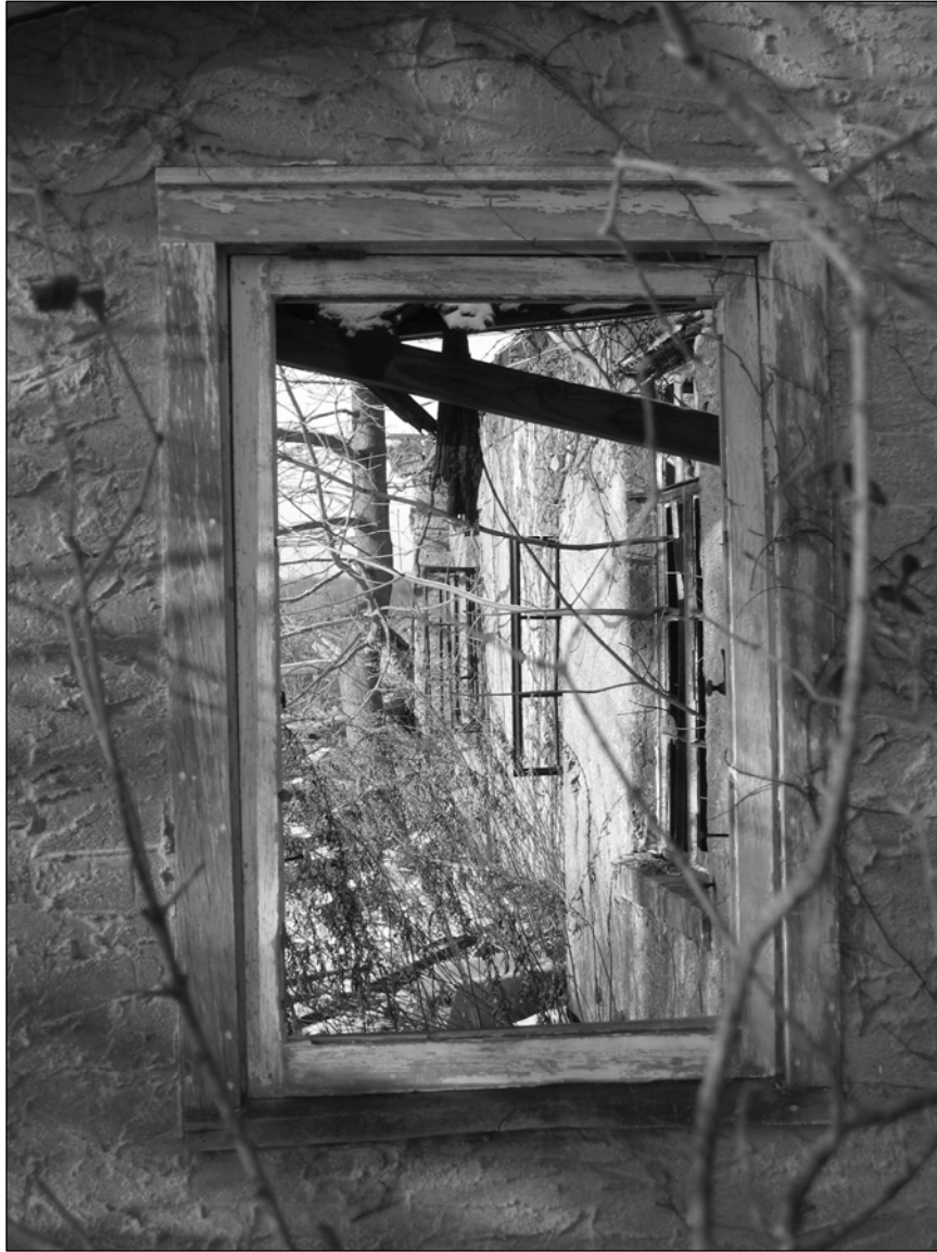
Photo 5. Southern façade, detail.
