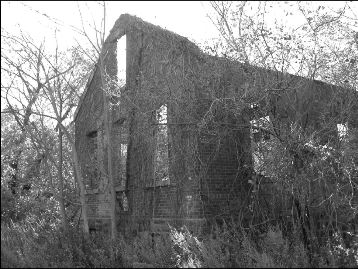
Photo 4. Northeast façade, facing southwest.
