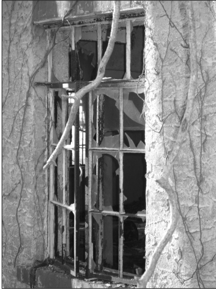
Photo 8. Eastern façade, detail.
