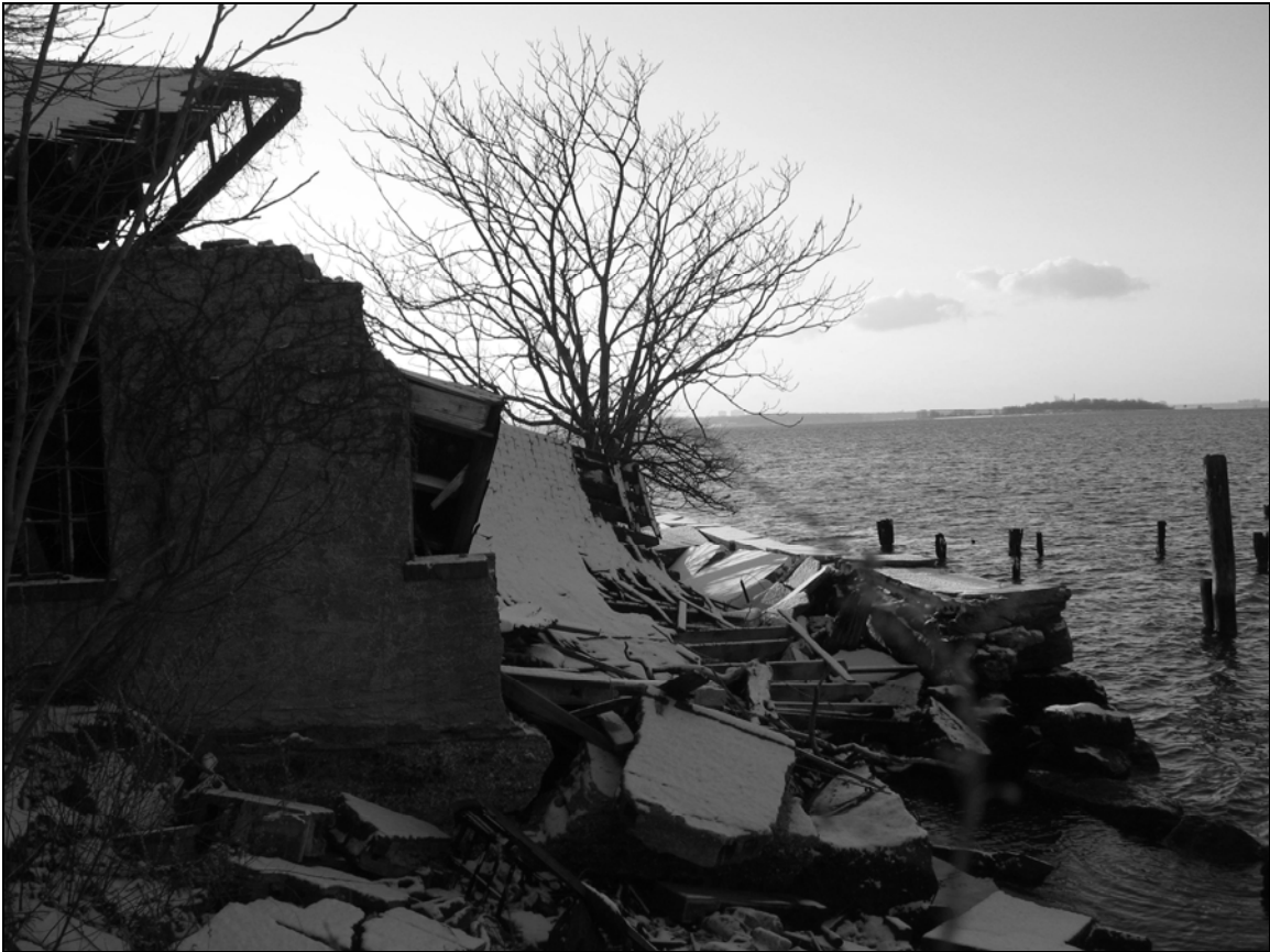
Photo 14. Northern façade, looking southwest.
