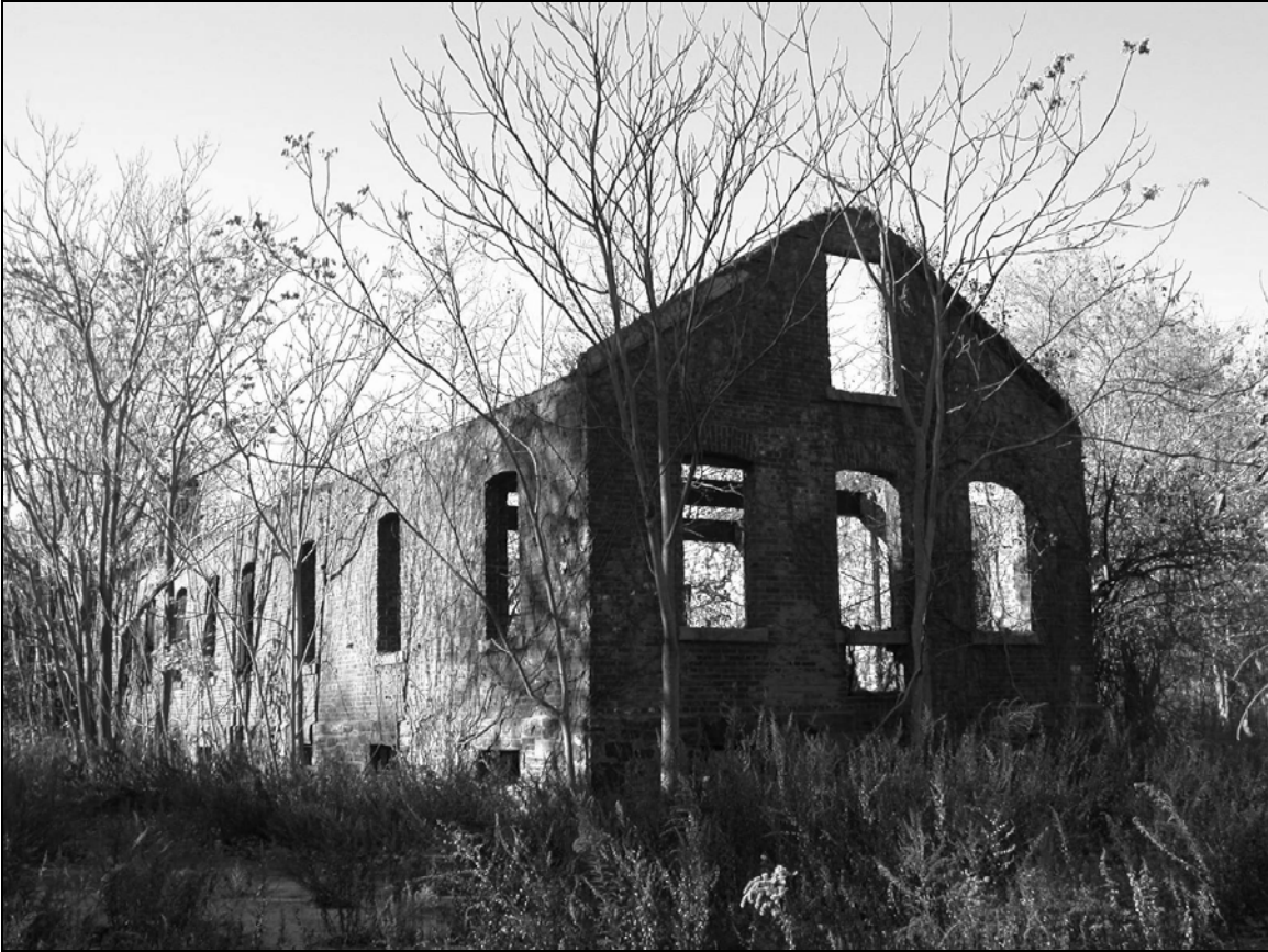
Photo 3. Southeast façade, facing northwest.
