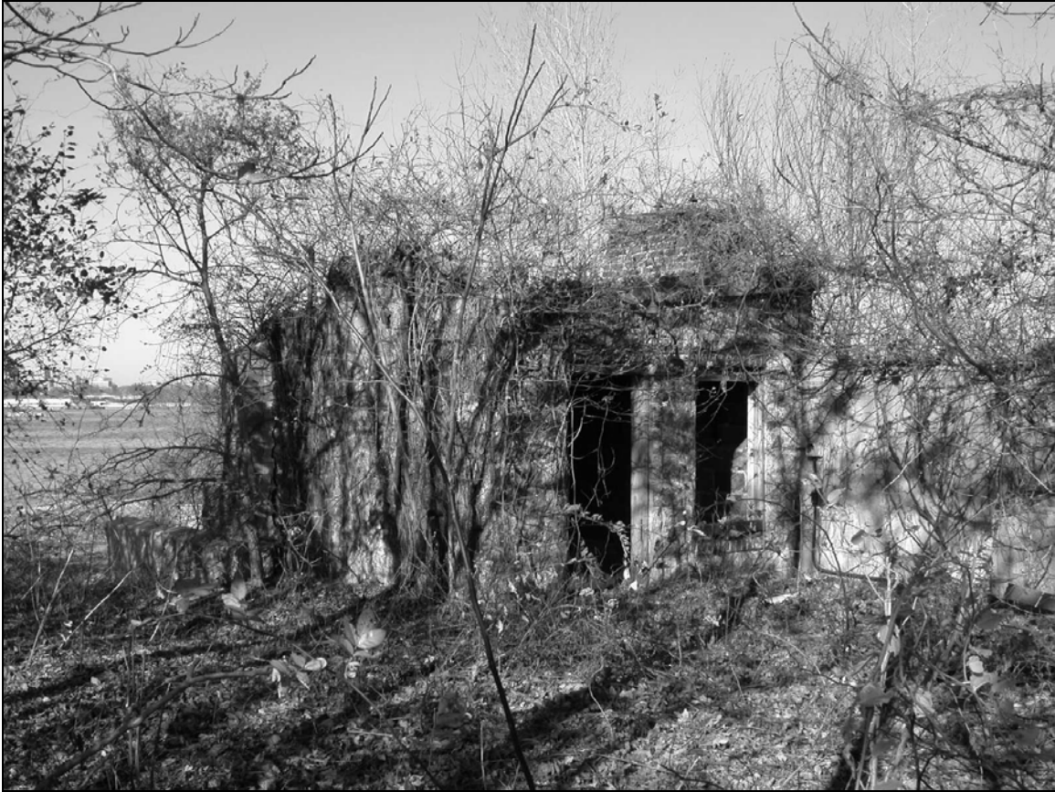
Photo 2. Southeastern façade, facing west.
