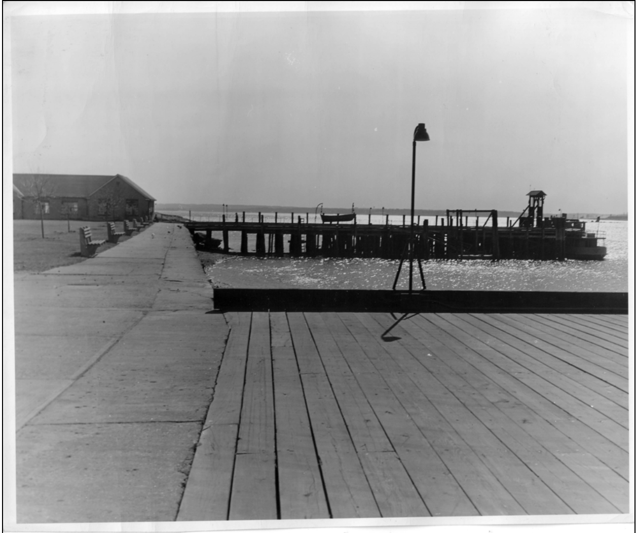
Figure 5. Circa Second World War photo. View southeast. Building 30 is located at far left. Fort Slocum Collection, New Rochelle Public Library, New Rochelle, New York.
