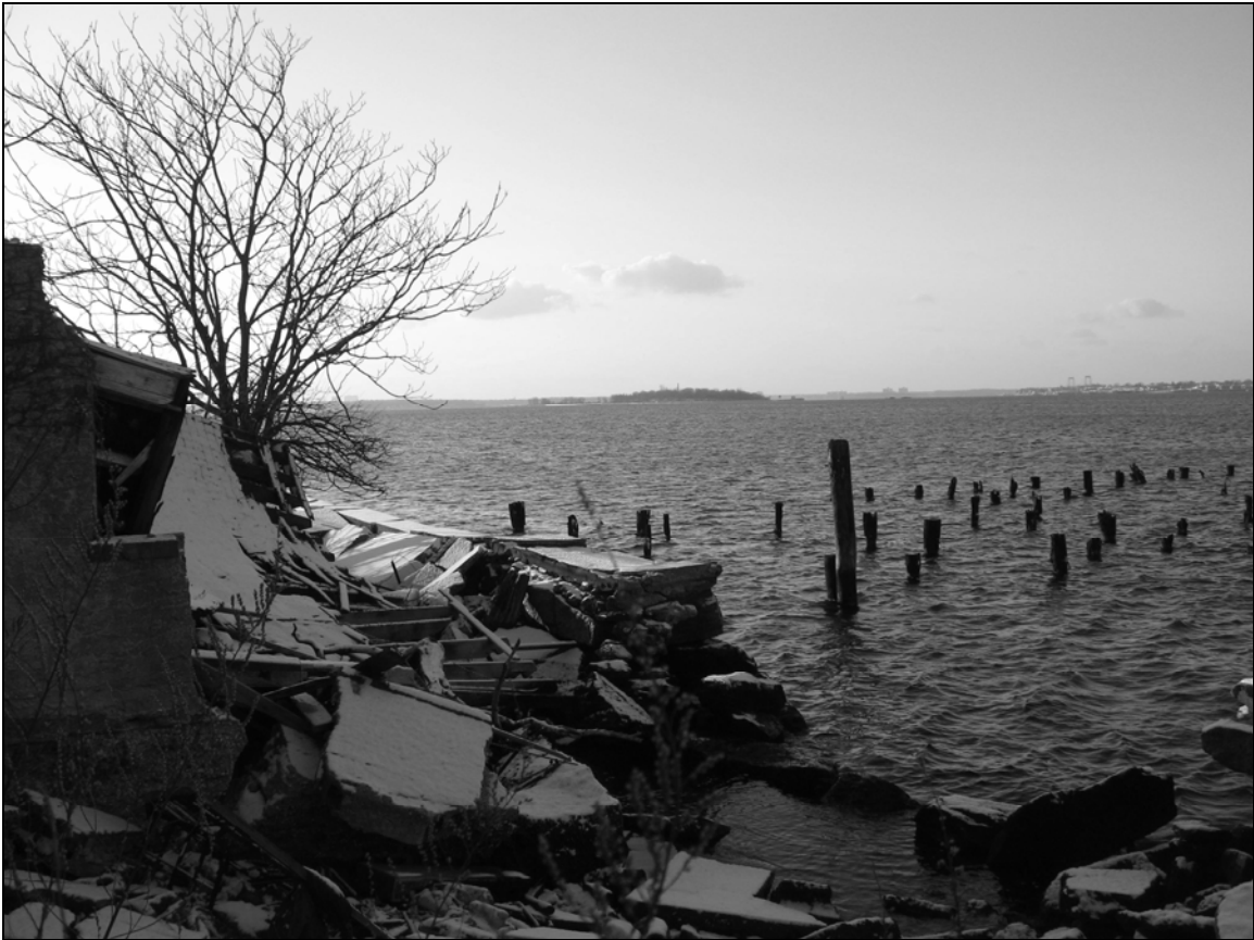
Photo 15. Northern façade, looking southwest.
