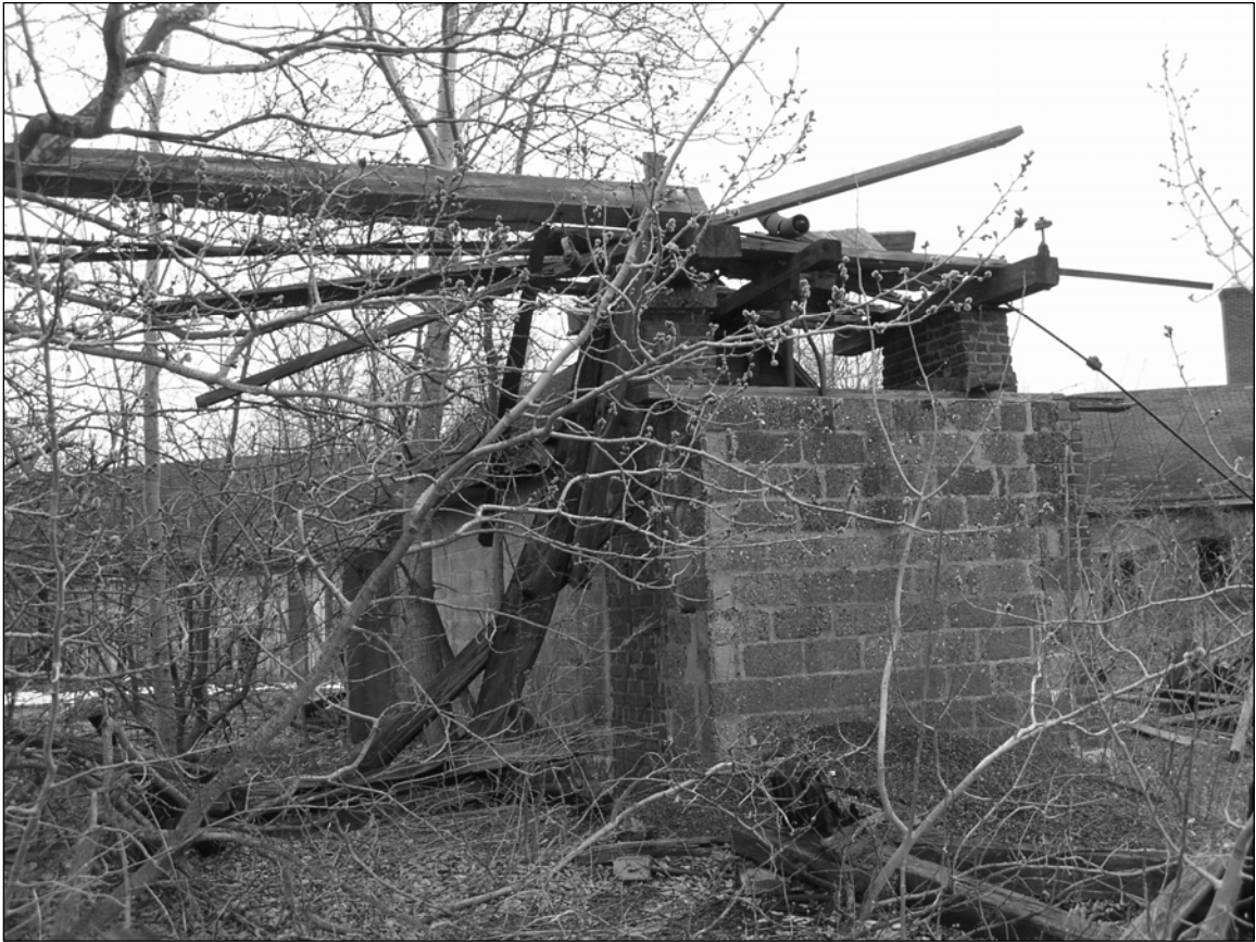
Photo 3. Northwestern end of building showing coal conveyor piers of brick built into the northeastern and southwestern walls, facing south.
