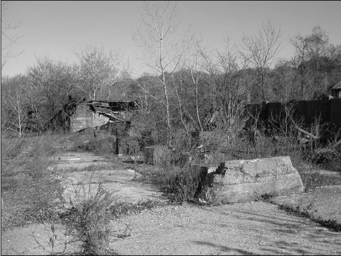
Photo 8. Coal yard and conveyor, facing east.
