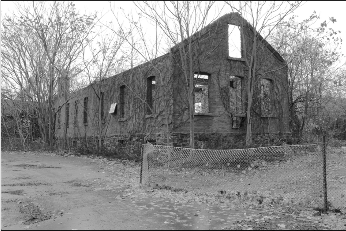
Photo 1. Southeast façade, facing northwest.
