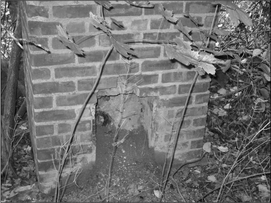
Photo 8. Chimney, facing south.
