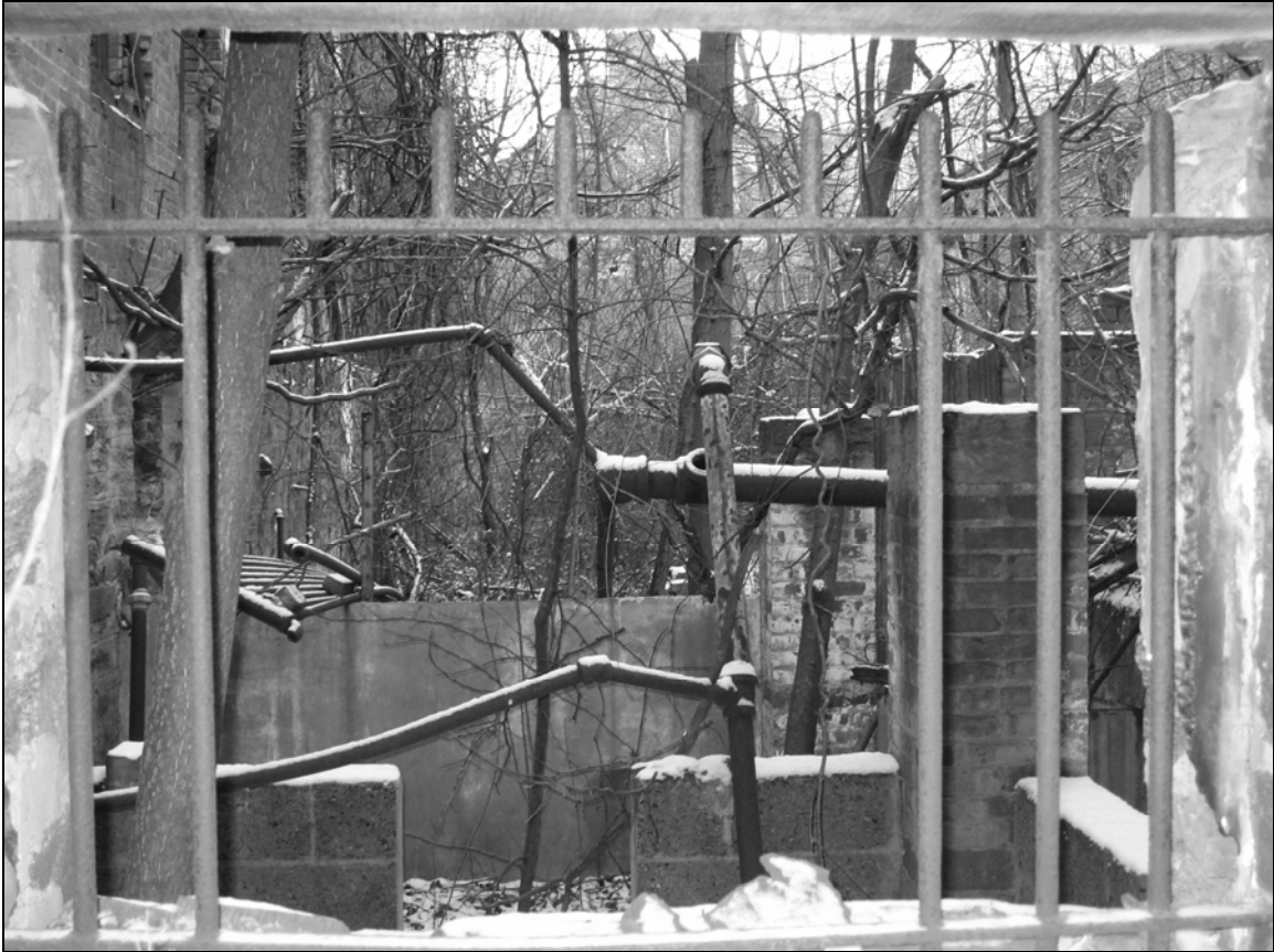
Photo 7. Interior, looking north.
