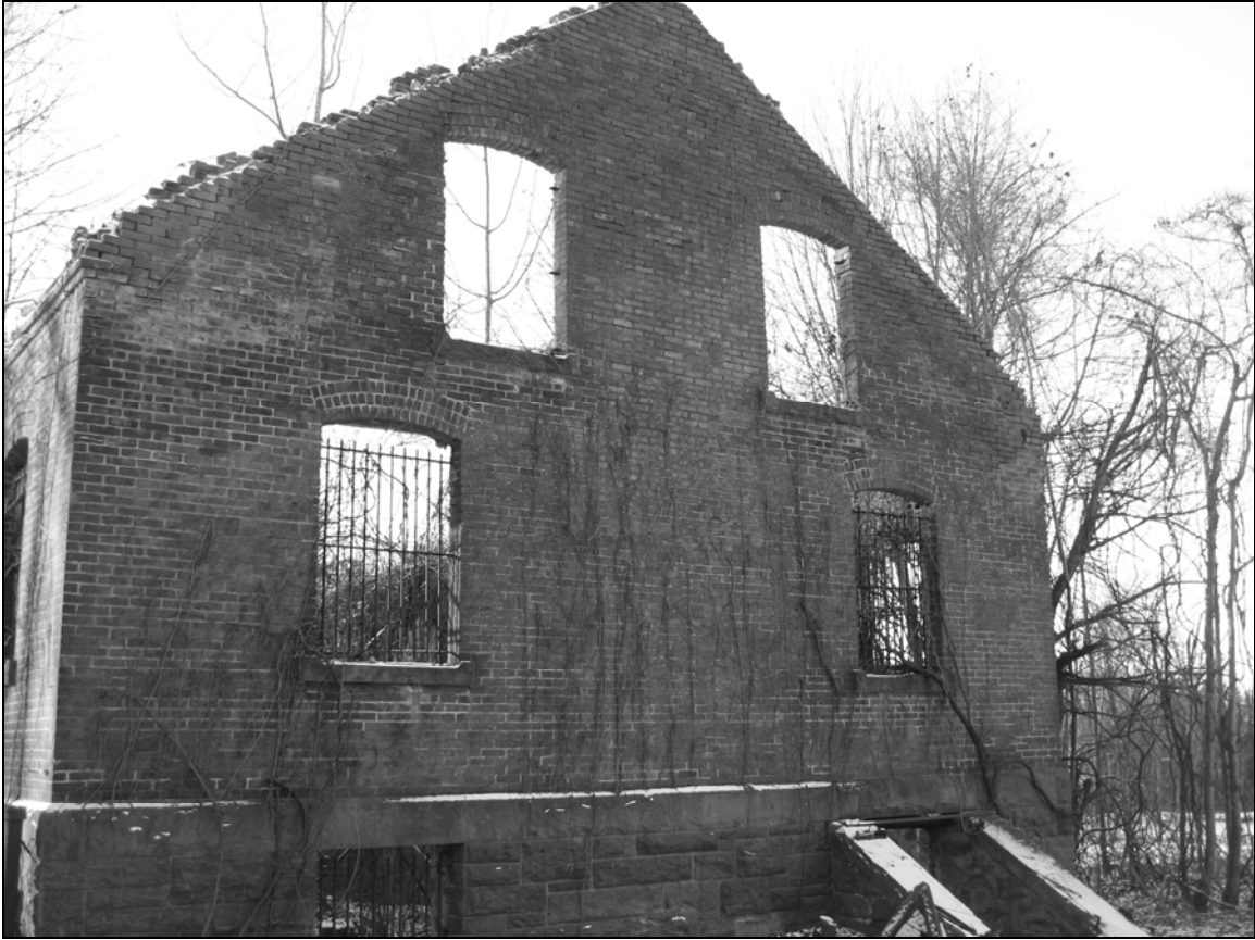
Photo 15. Northern façade, looking south.
