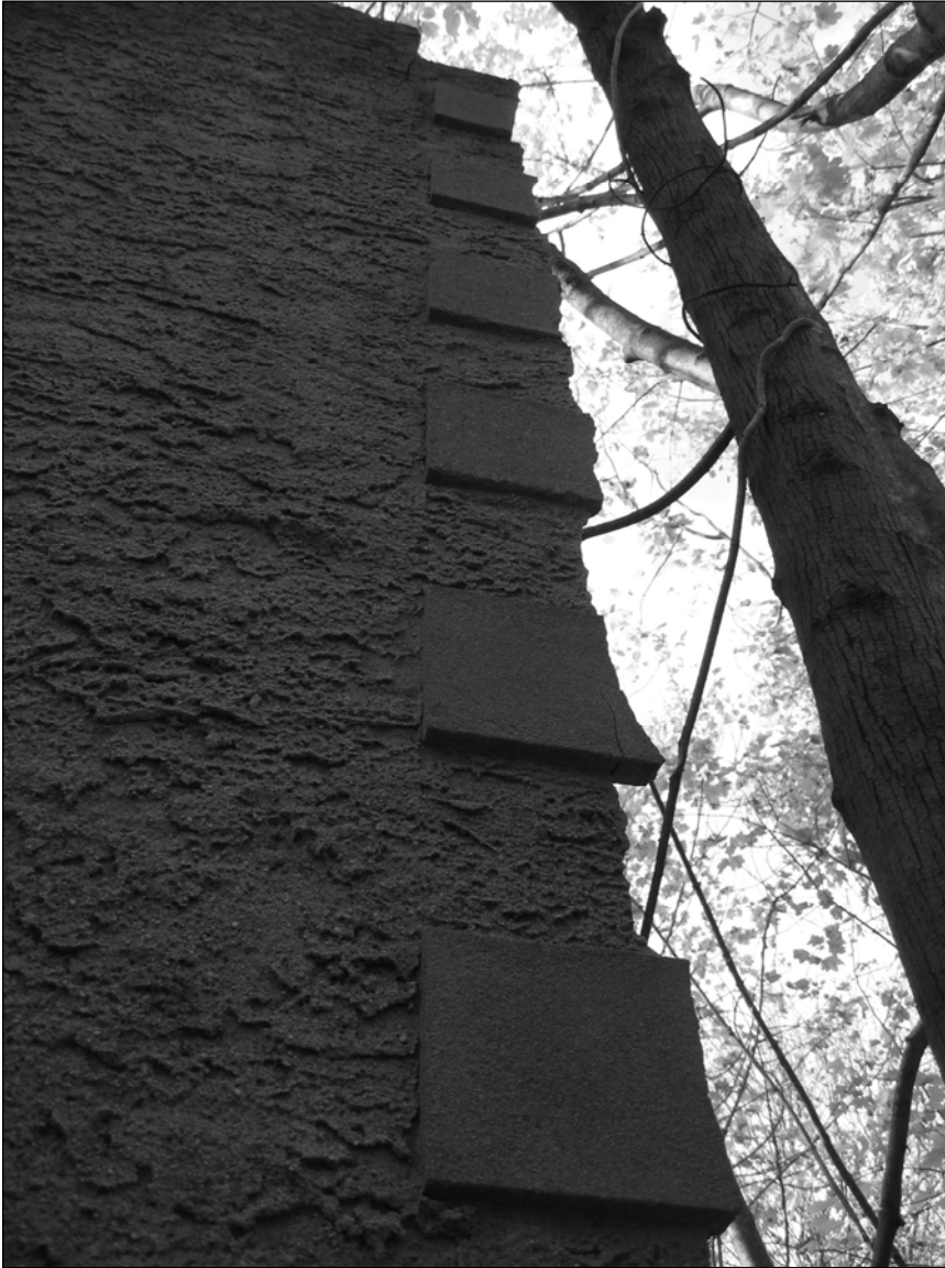
Photo 13. Northeastern corner detail.
