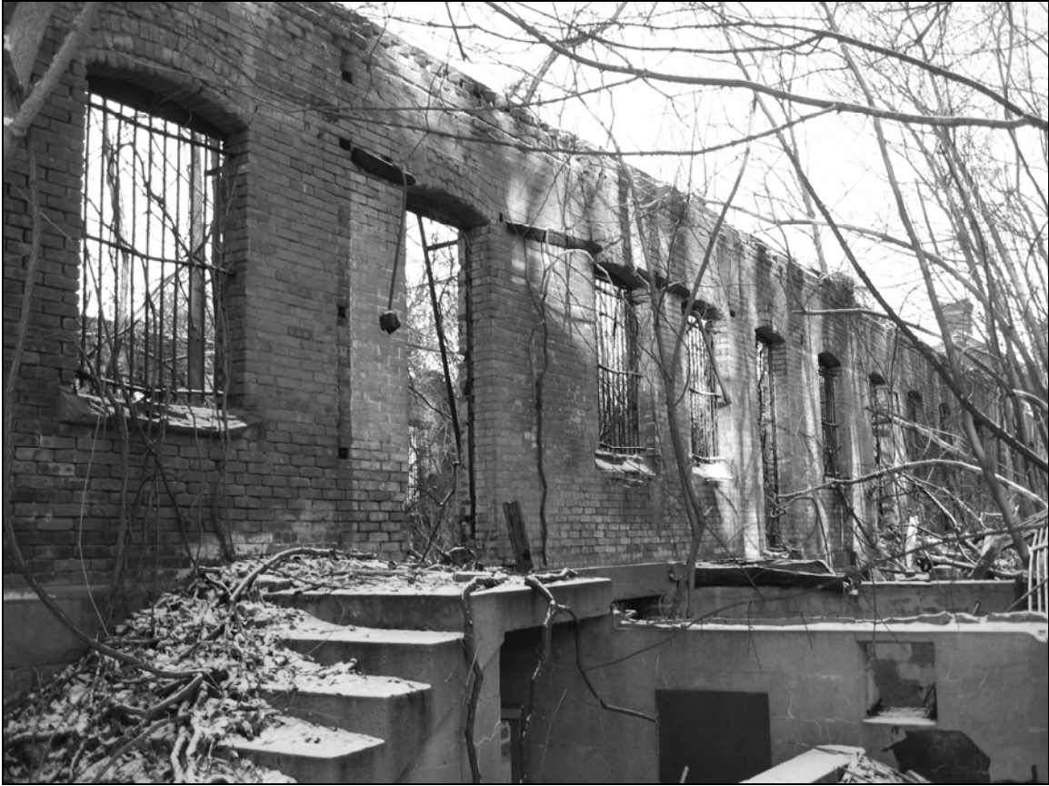
Photo 8. Eastern façade, looking northwest.
