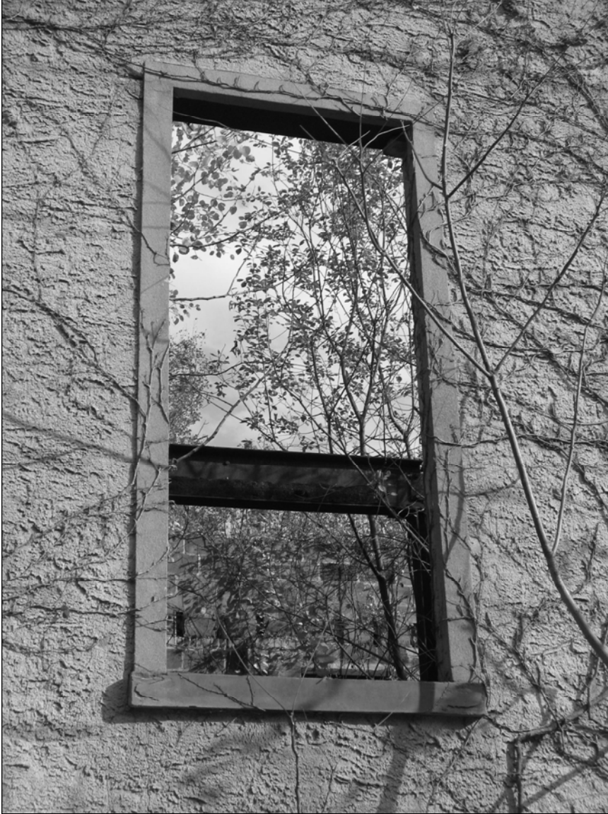
Photo 7. Western elevation facing east.
