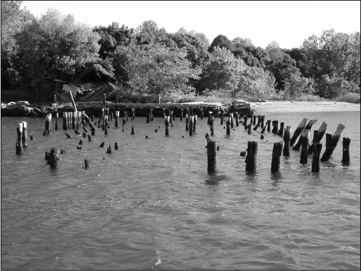
Photo 2. View of southwest end of Passenger Dock looking northeast.
