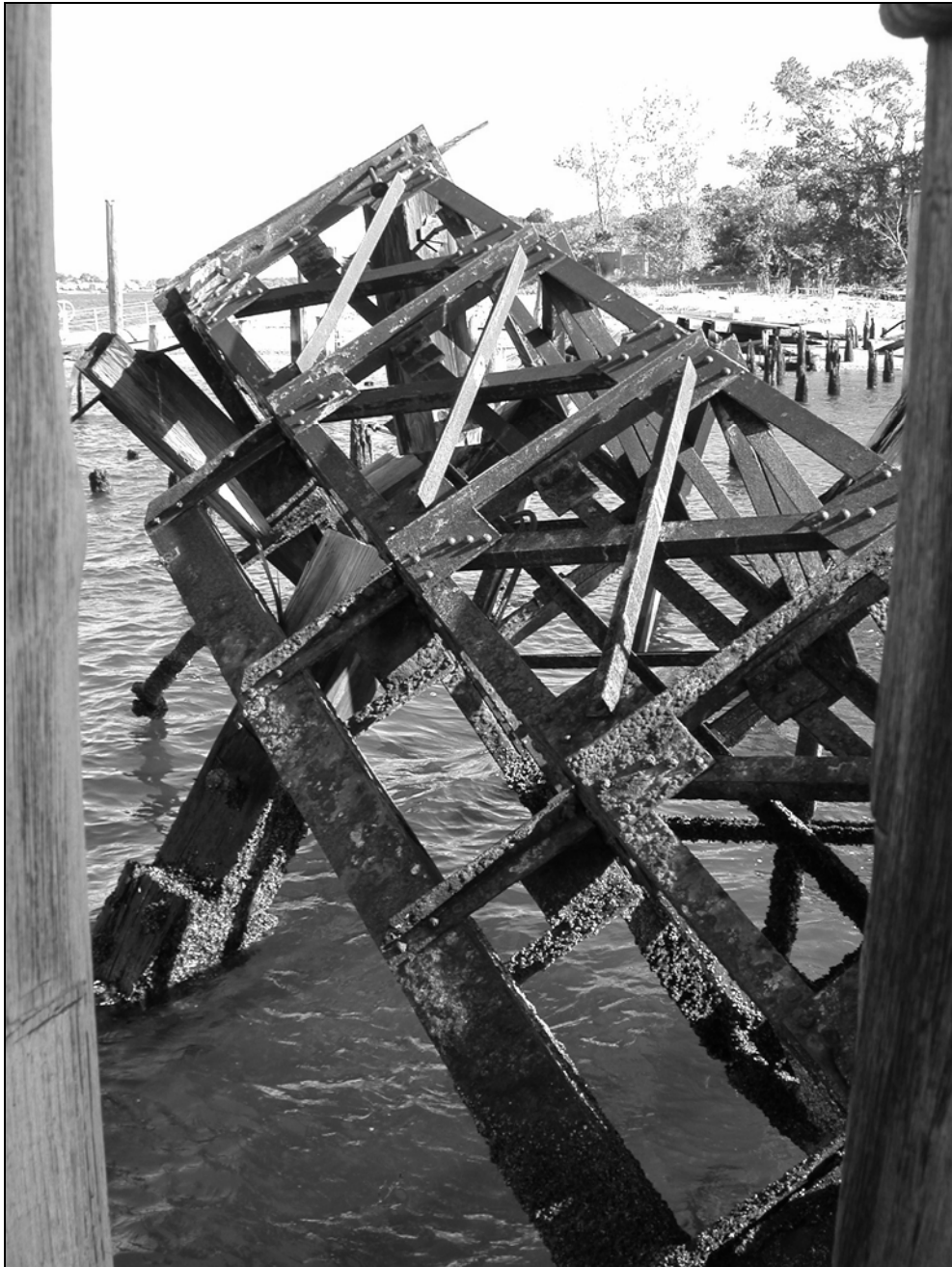
Photo 12. Detail view of vehicle gangplank hoist gantry tower looking north.
