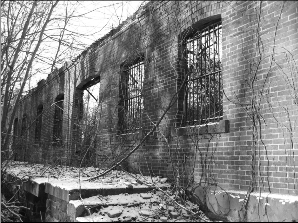
Photo 14. Eastern façade, looking southwest.
