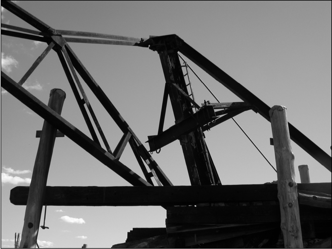
Photo 9. Detail view of Freight Crane backstays looking east.
