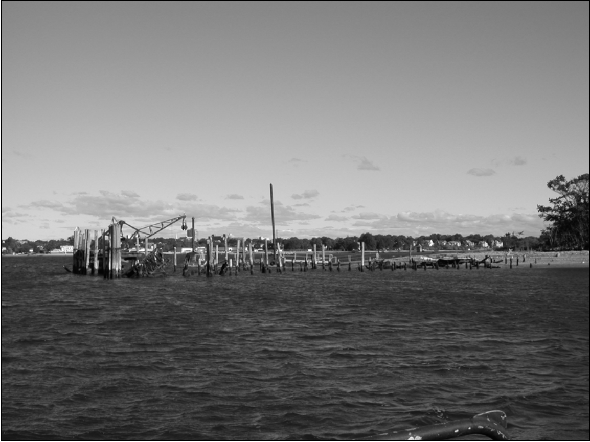
Photo 4. General view of southeast side of Fright Pier looking north.
