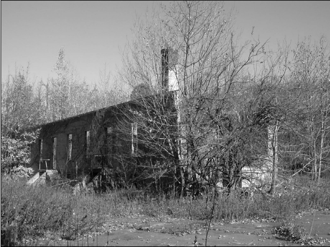
Photo 1. General view facing northeast.
