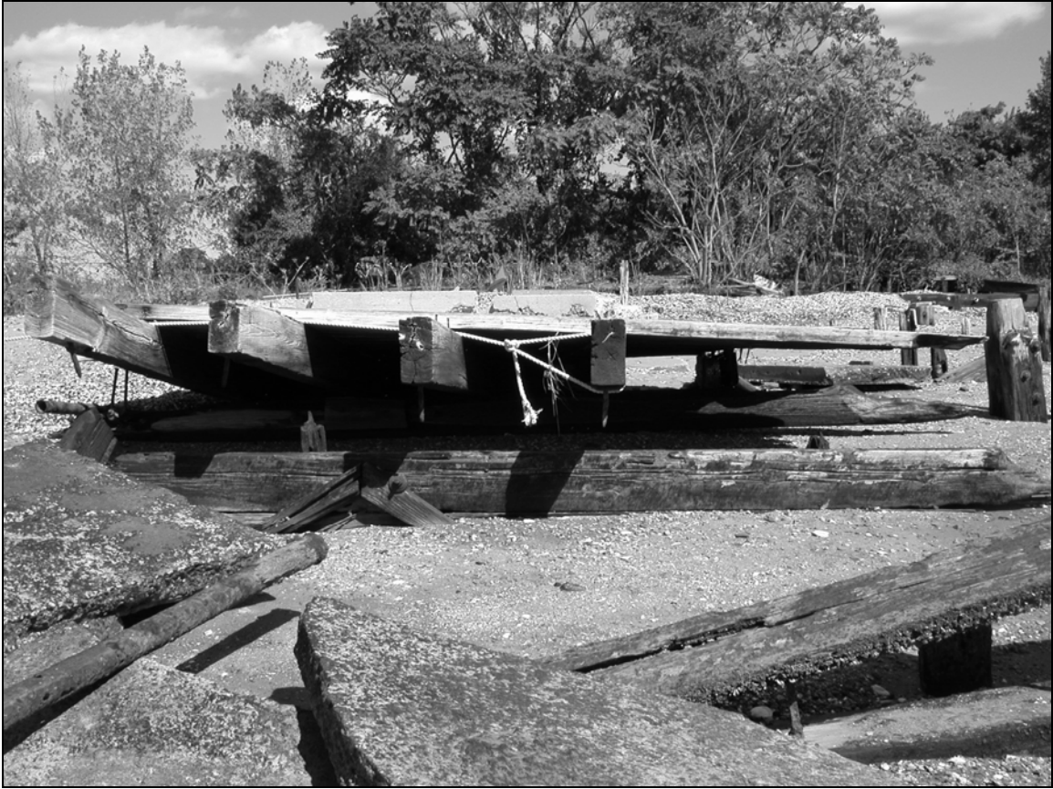
Photo 16. Detail view of Freight Pier deck structure looking northeast.
