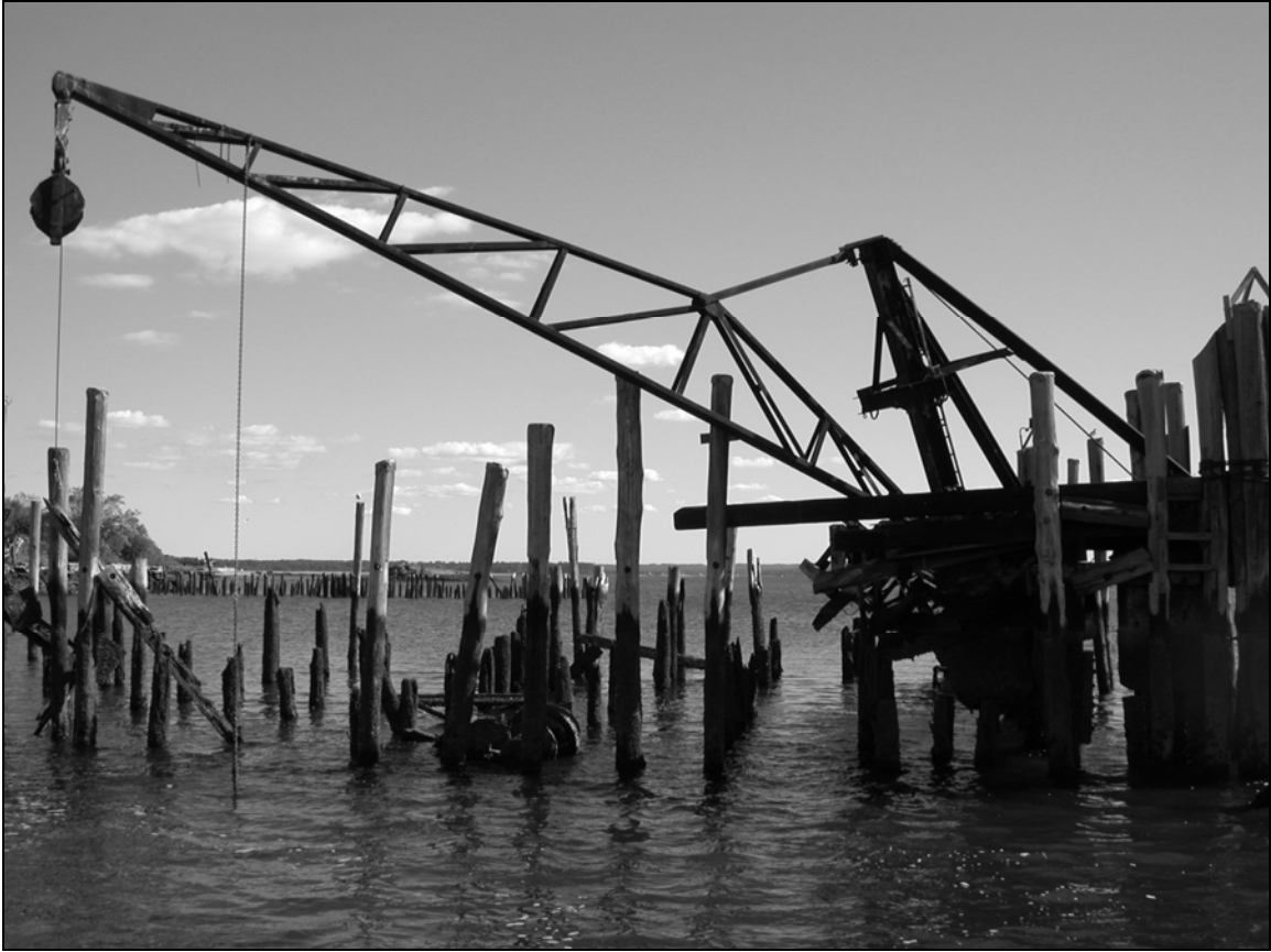
Photo 8. Detail view of Freight Crane boom looking southeast.
