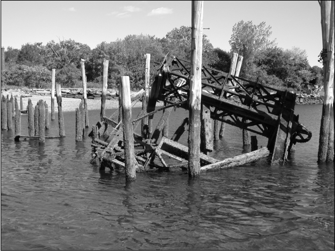
Photo 10. Detail view of vehicle gangplank hoist gantry tower looking northeast.
