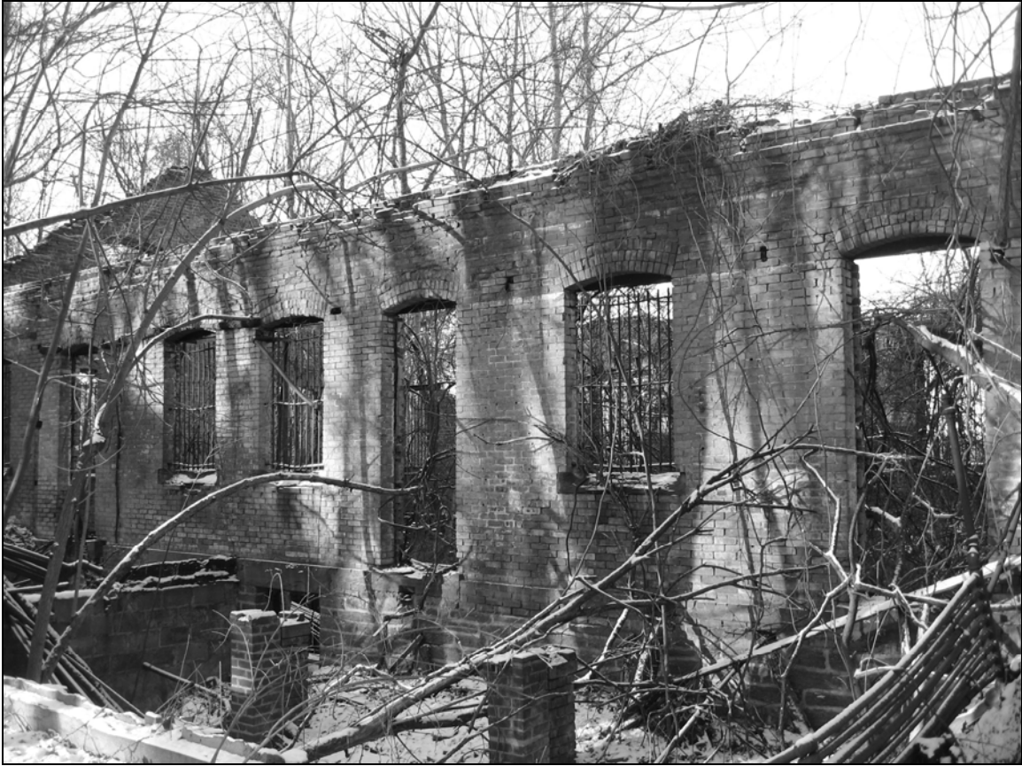
Photo 12. Eastern façade, looking west.
