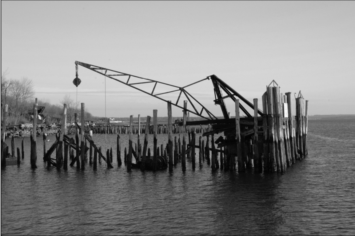
Photo 1. General view of northwest side of Freight Pier looking southeast.
