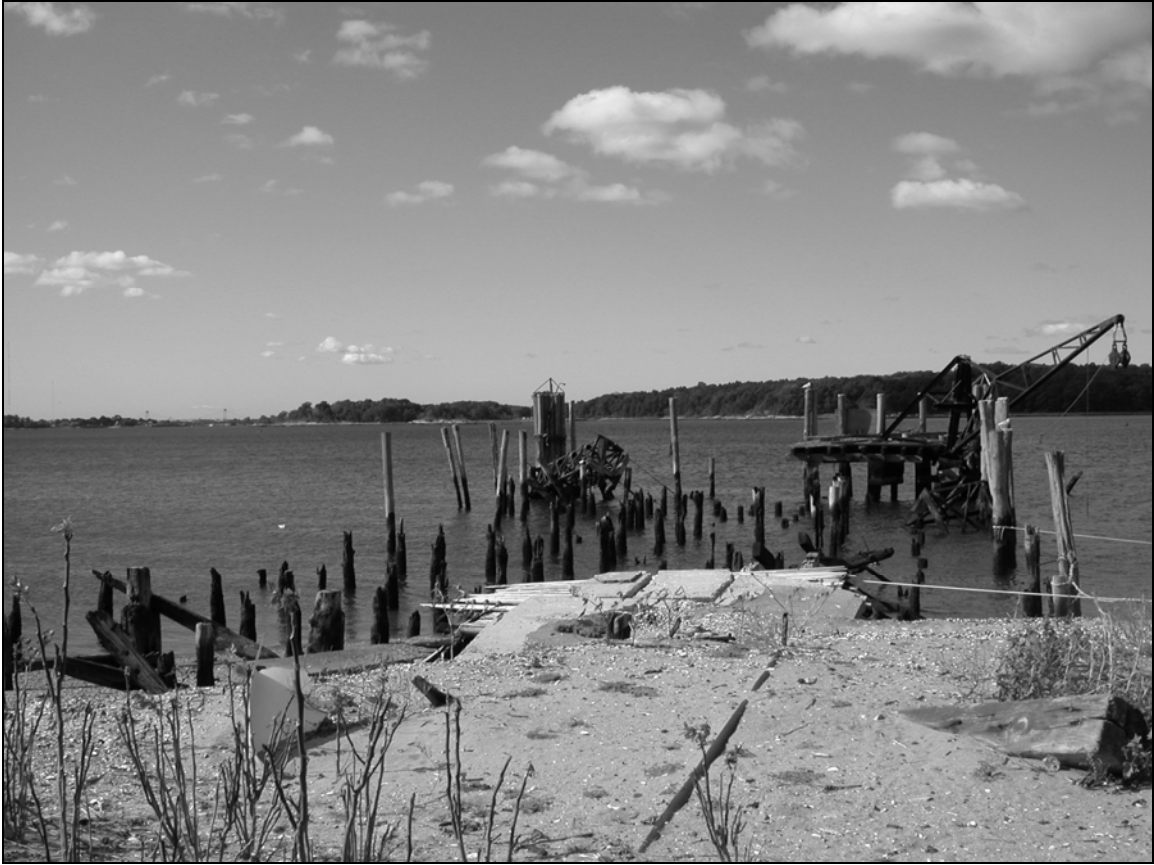
Photo 17. Detail view of Freight Pier deck structure looking southwest.
