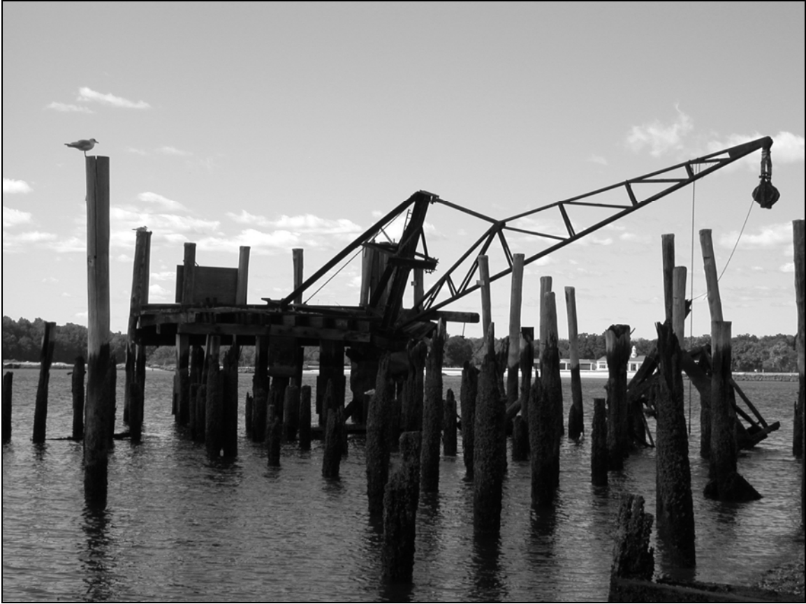
Photo 14. Detail view of Freight Crane looking northwest.
