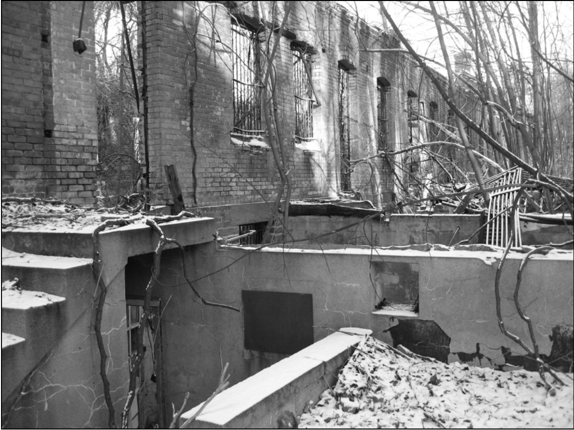
Photo 10. Eastern façade, looking northwest.
