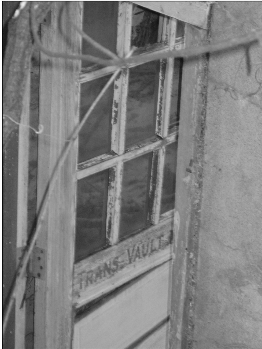
Photo 9. Eastern façade, detail.
