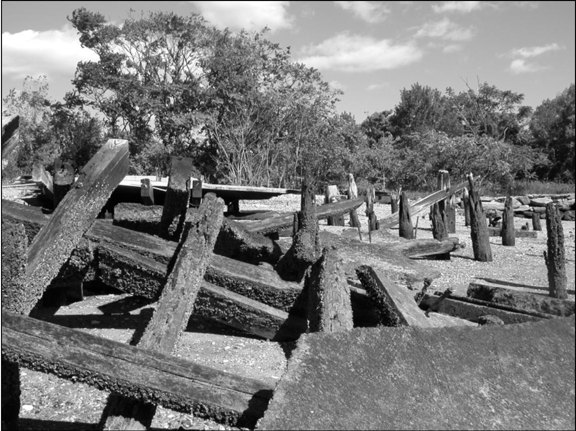
Photo 15. Detail view of Freight Pier deck structure looking northeast.
