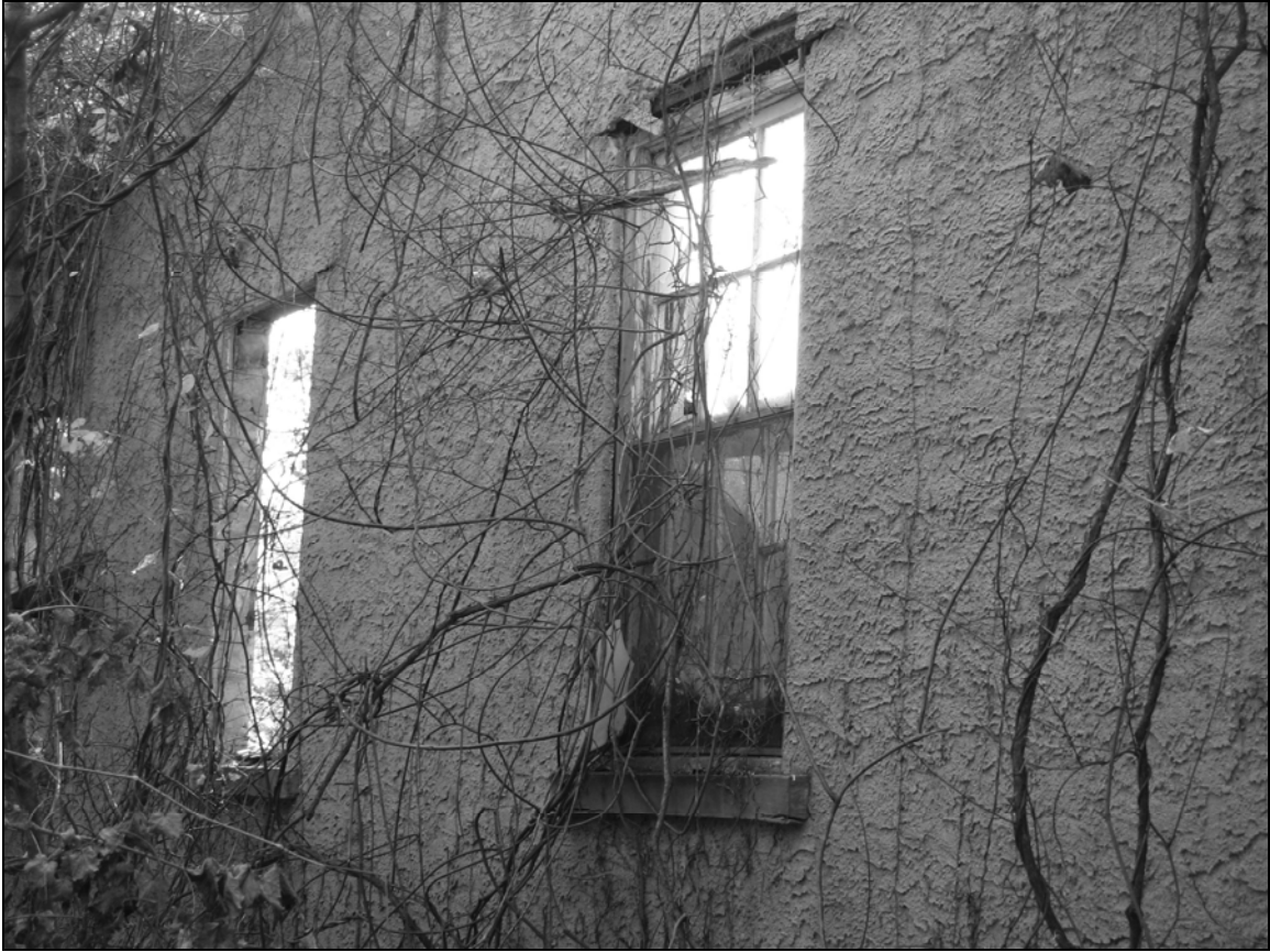
Photo 3. Eastern elevation facing southwest.
