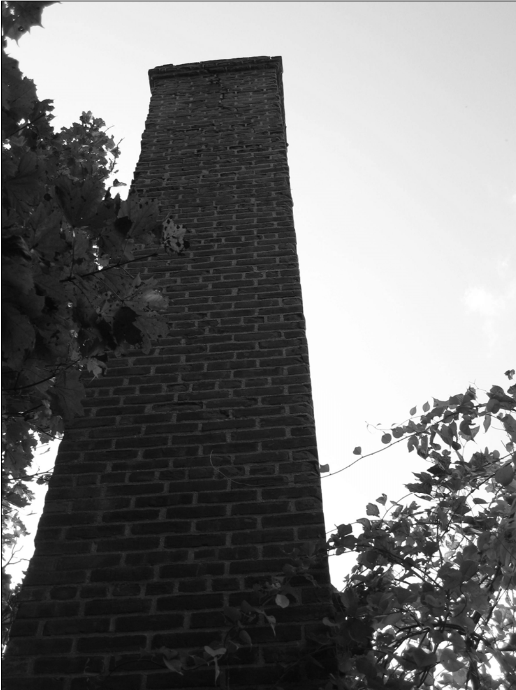
Photo 2. Chimney, facing north.
