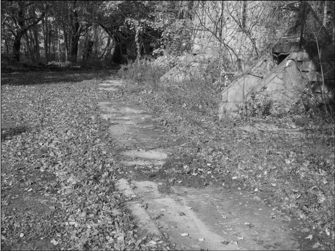
Photo 5. Perimeter sidewalk facing north.
