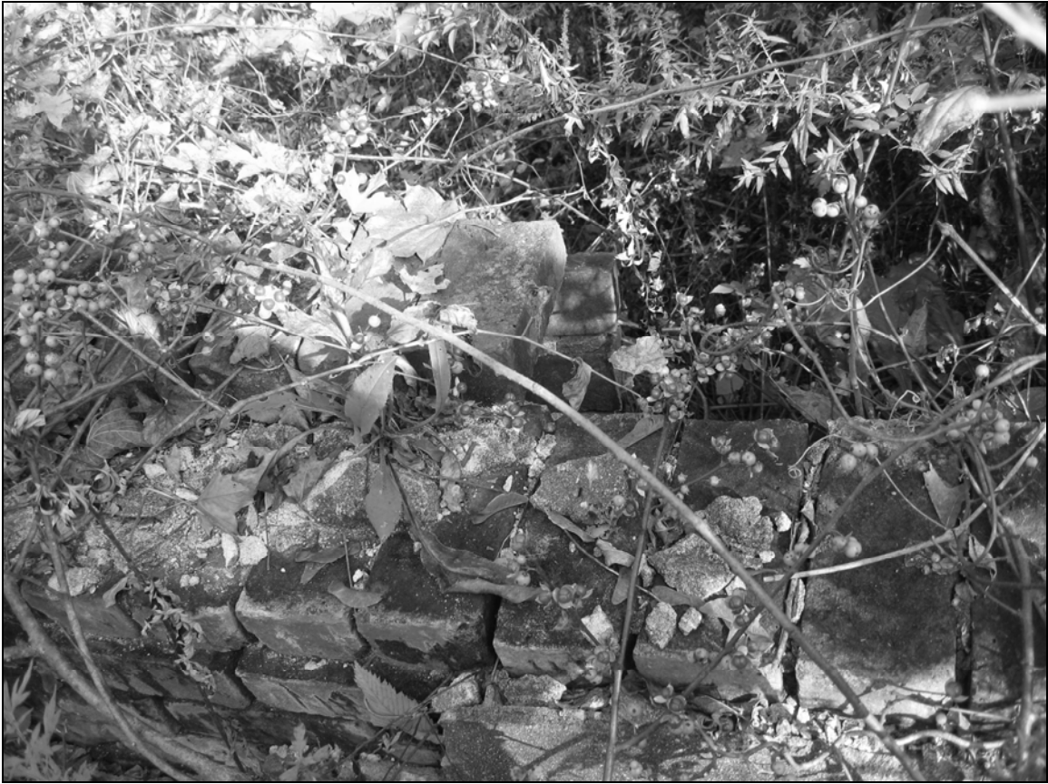
Photo 4. Western foundation detail.
