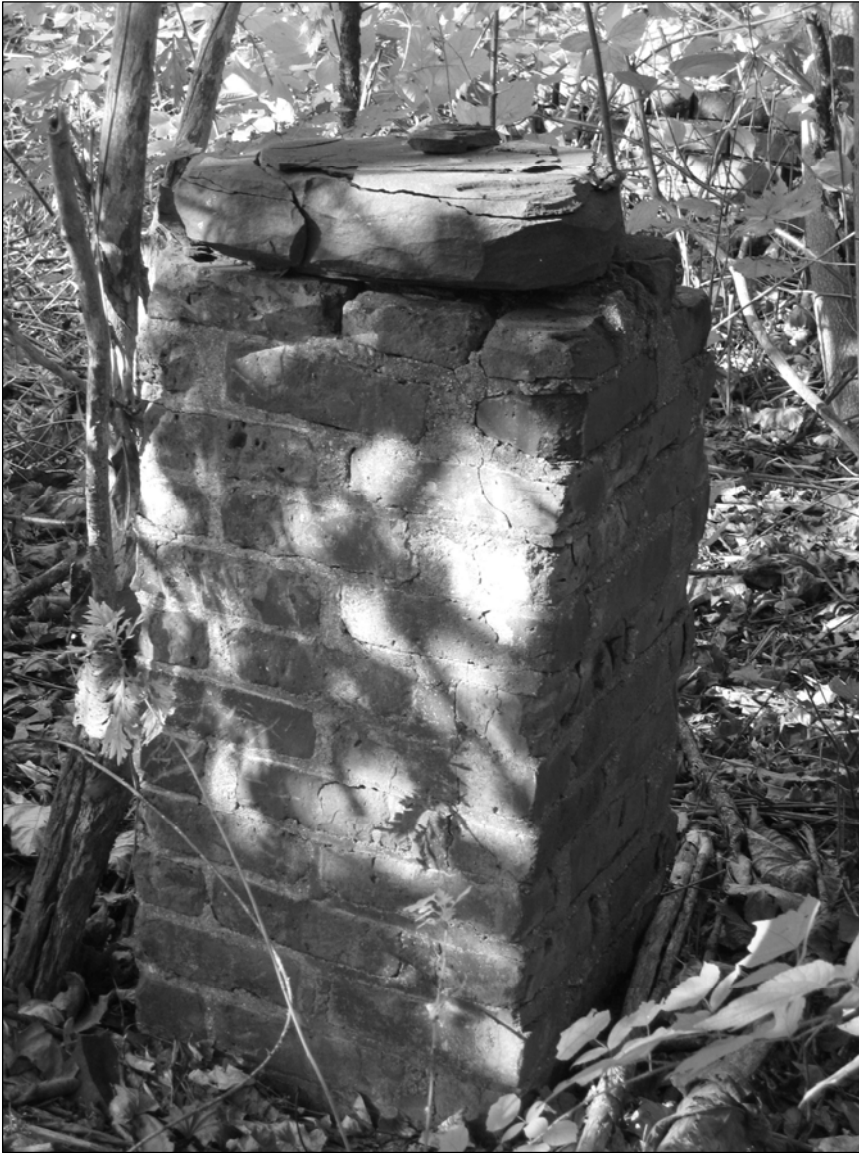
Photo 6. Porch pier, facing north.
