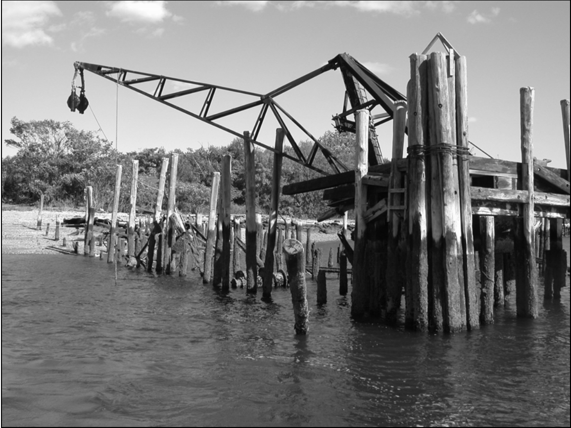
Photo 2. General view of west corner of Freight Pier looking east.
