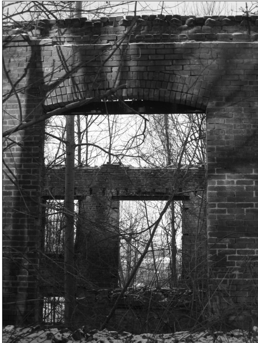
Photo 13. Eastern façade, detail.
