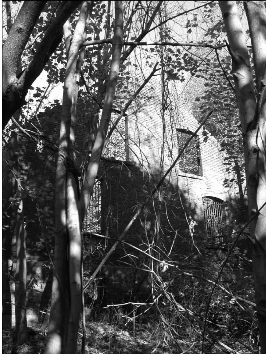
Photo 1. Southern façade, looking northwest.
