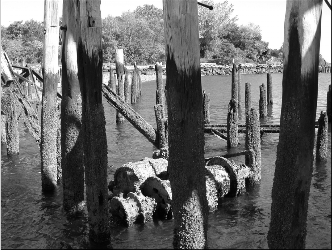
Photo 7. Detail view of electrical motor and cable hoist drum looking east.
