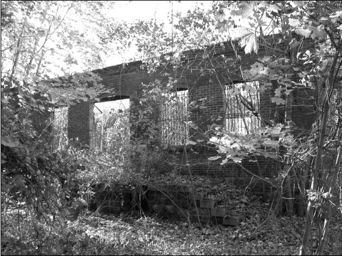
Photo 3. Eastern façade, looking west.
