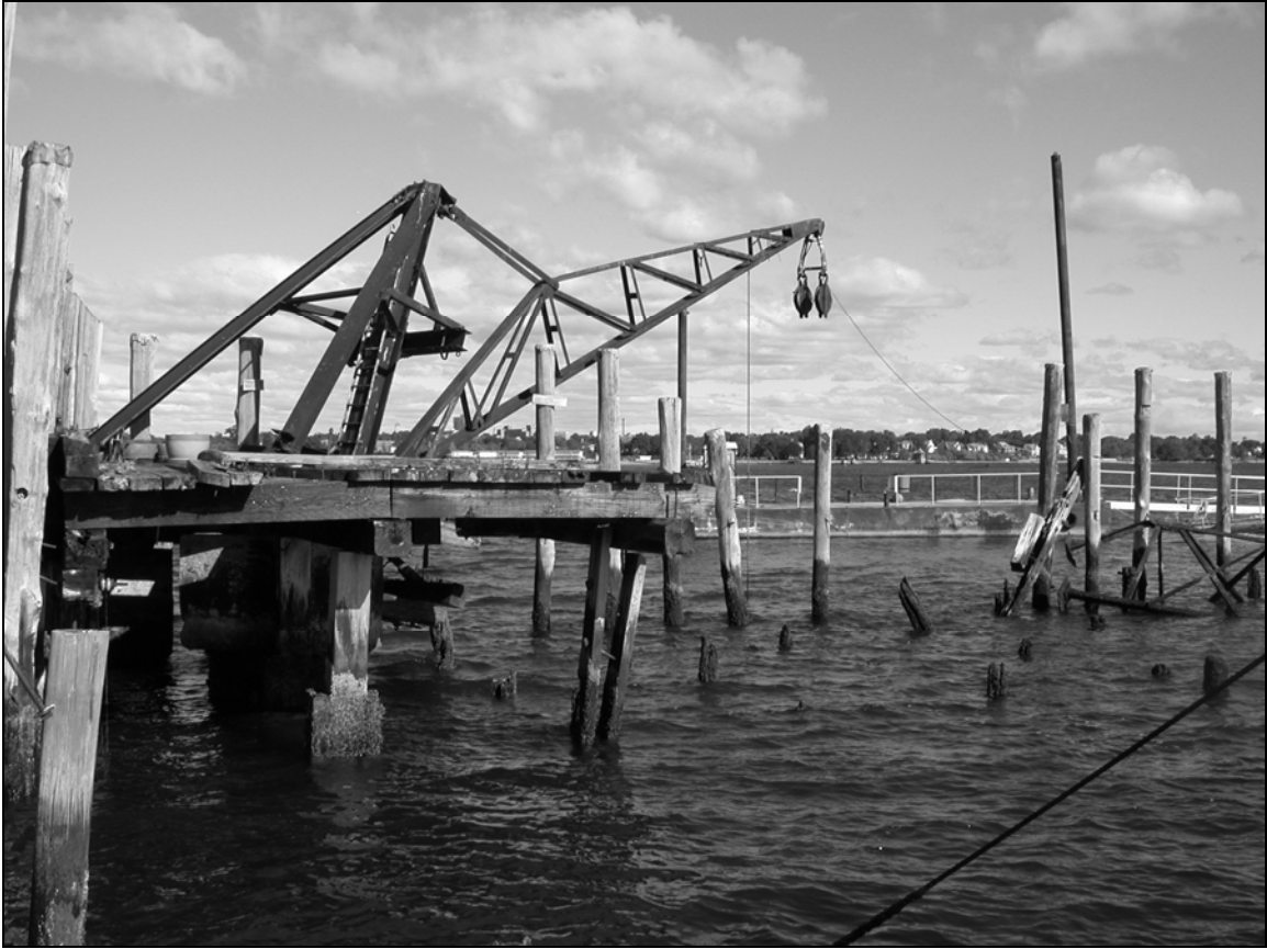
Photo 13. Detail view of Freight Crane looking north.
