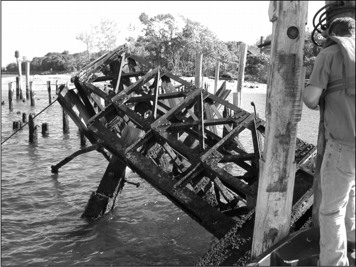
Photo 11. Detail view of vehicle gangplank hoist gantry tower looking northeast.
