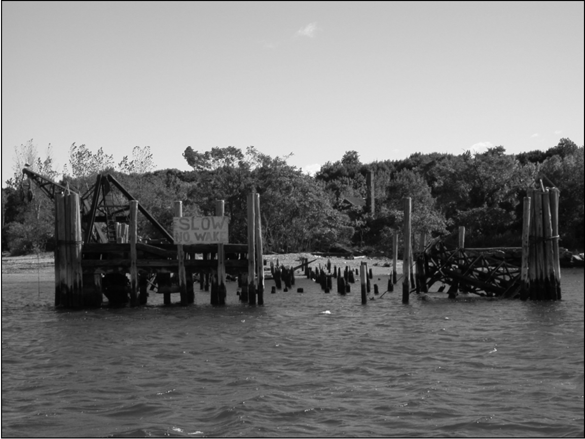
Photo 3. General view of southwest end of Freight Pier looking northeast.
