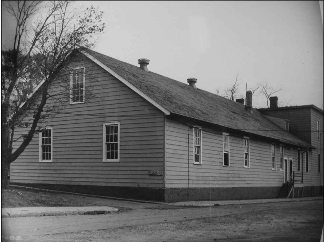
Figure 7. Inventory photo, probably mid-1930s. View southeast. Record Group 111, National Archives, College Park, MD.
