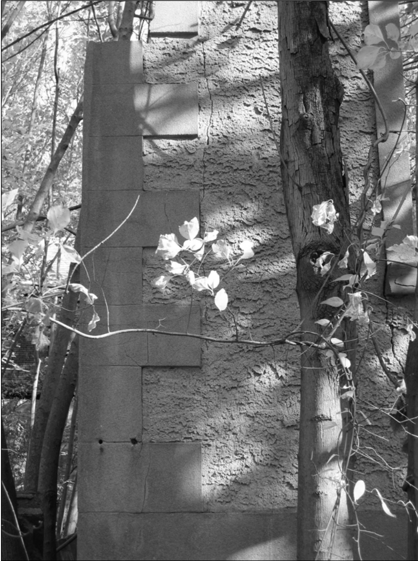
Photo 9. Northwestern corner, facing east.
