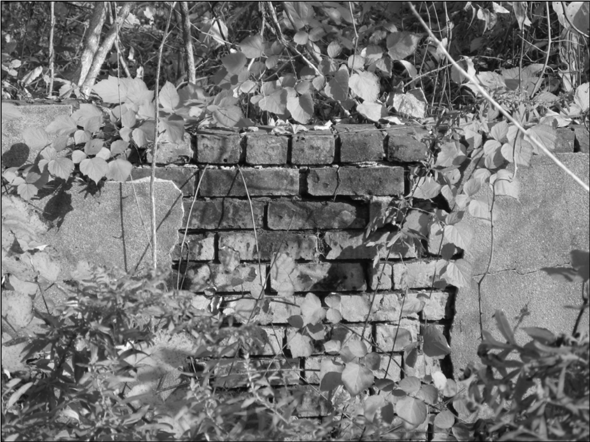
Photo 5. Western foundation detail.
