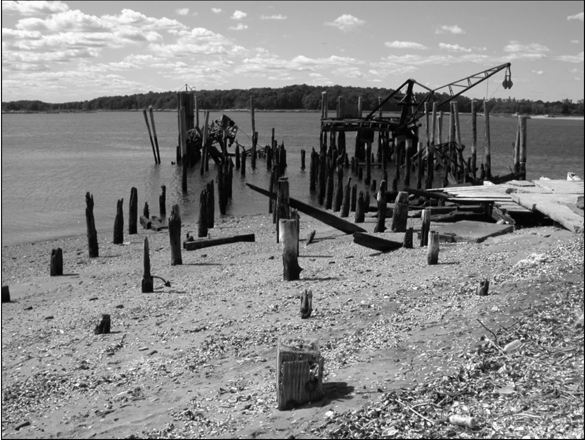
Photo 6. General view of Freight Pier looking southwest.
