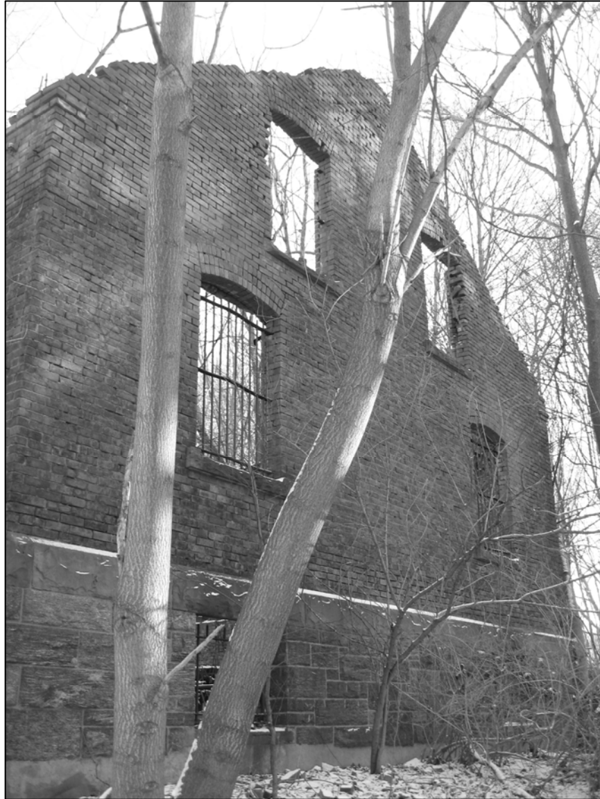
Photo 5. Southern façade, looking northeast.
