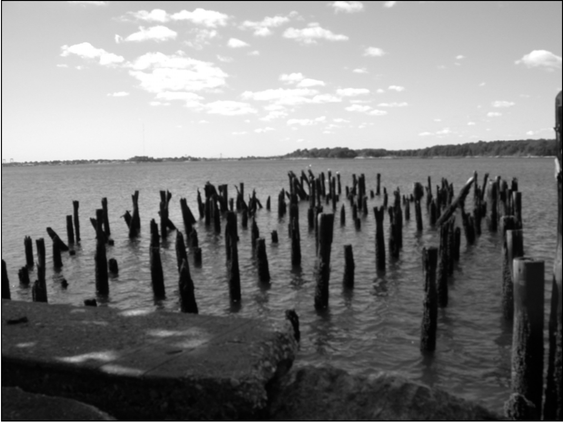
Photo 5. View of Passenger Dock looking southwest from seawall.
