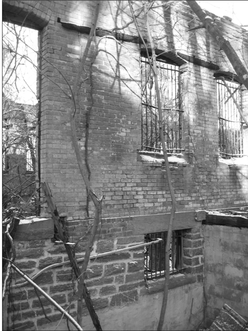
Photo 11. Eastern façade, detail.
