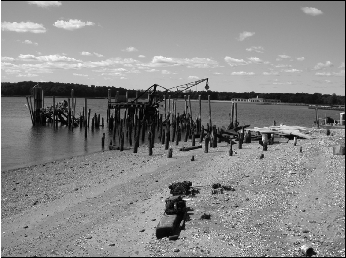
Photo 5. General view of southeast side of Freight Pier looking northwest.
