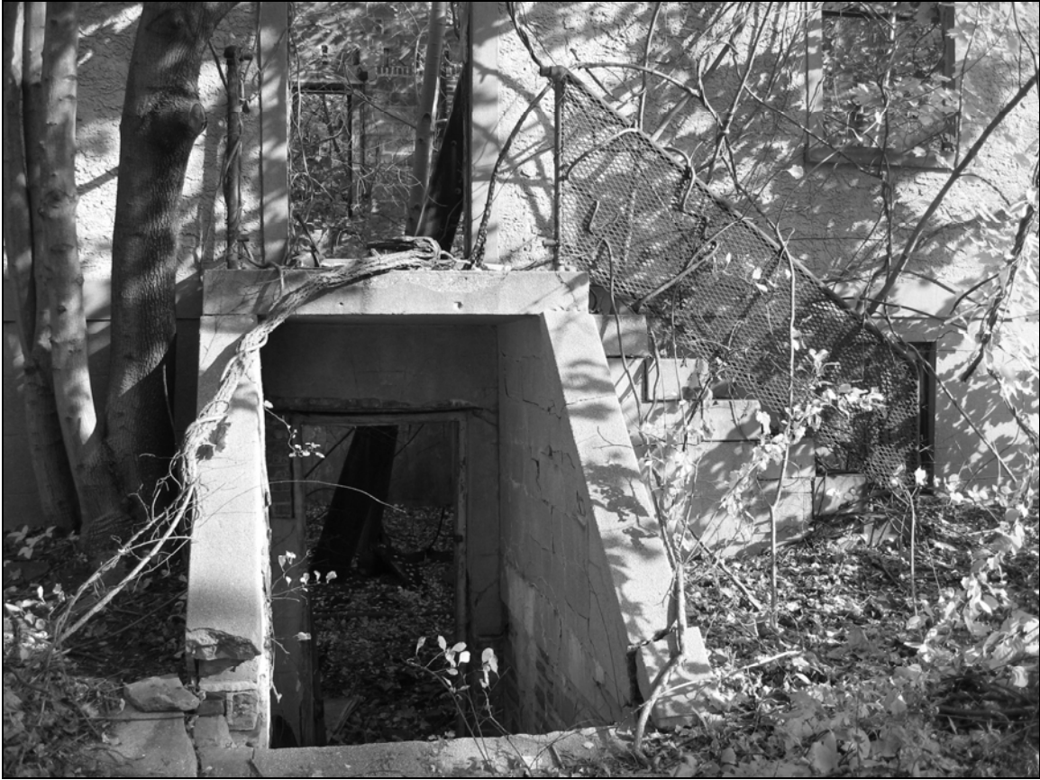
Photo 8. Western elevation facing east.
