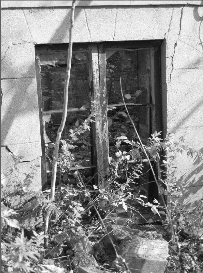
Photo 6. Foundation detail, western elevation facing east.
