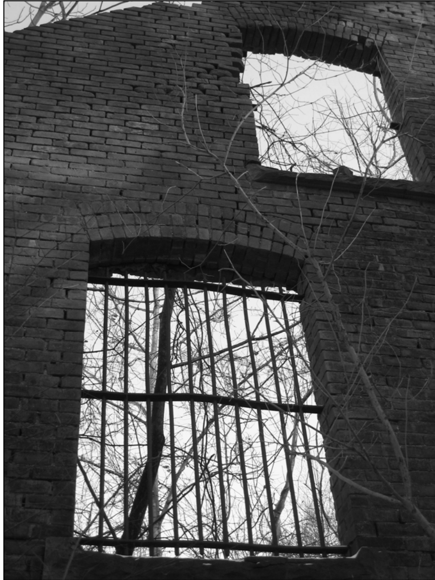
Photo 6. Southern façade, detail.
