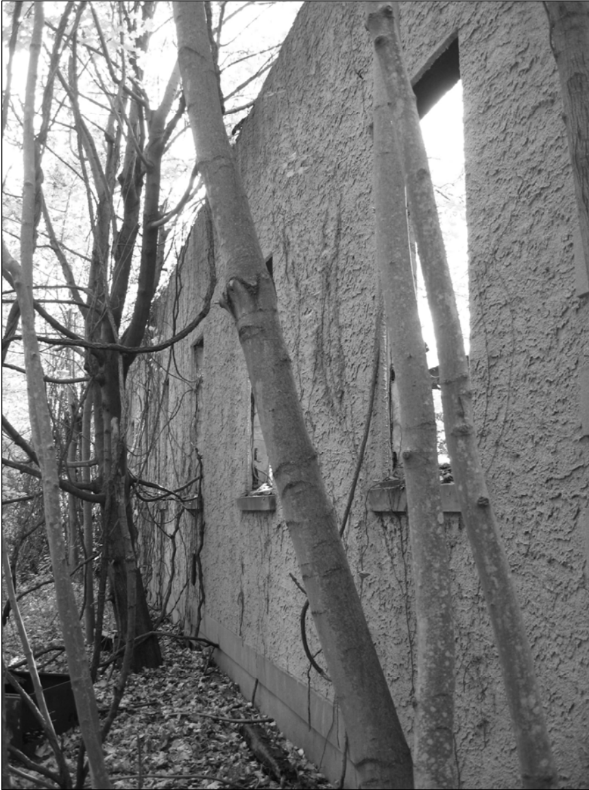
Photo 10. Eastern façade facing south.
