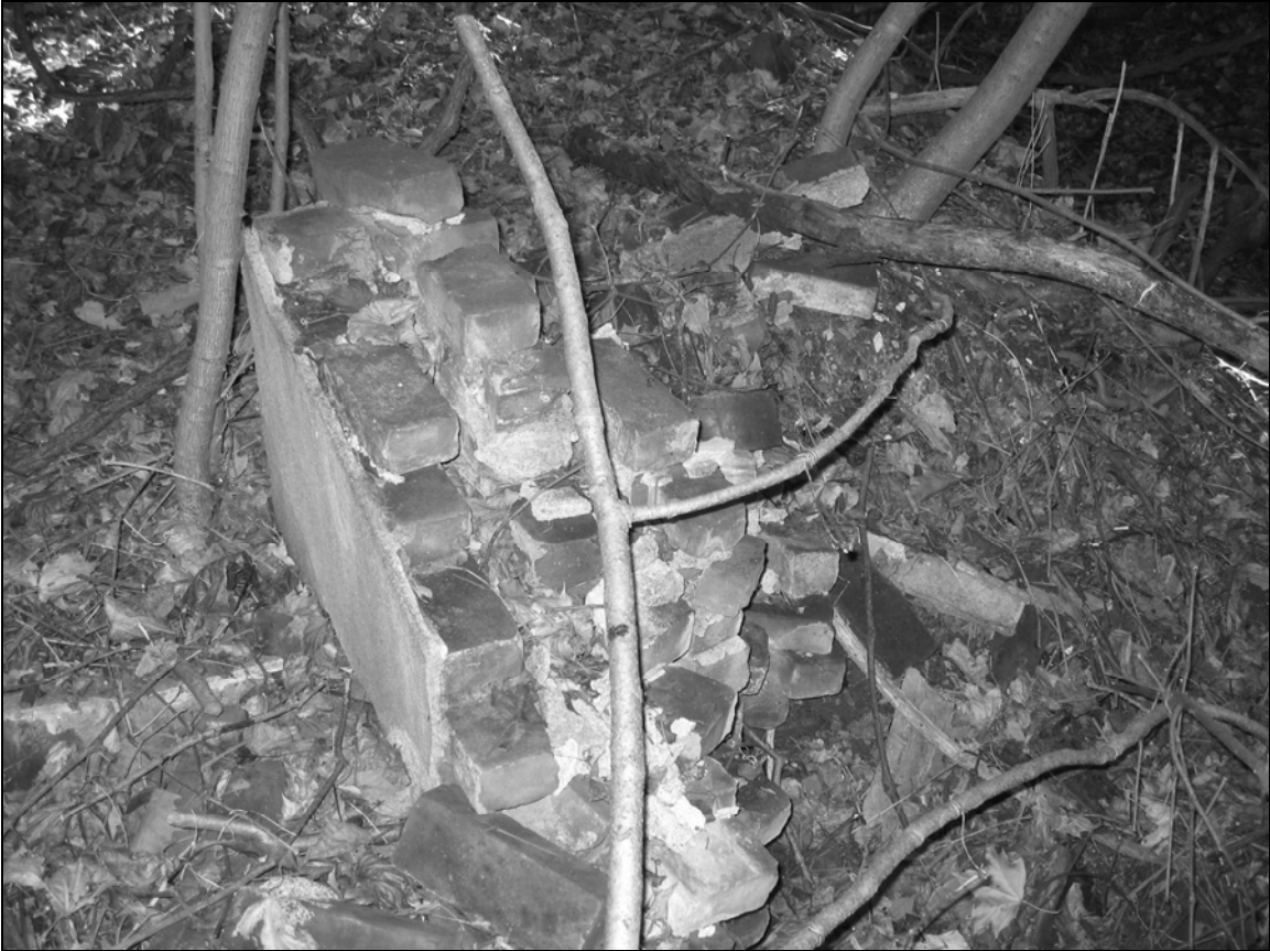
Photo 7. North wall detail.
