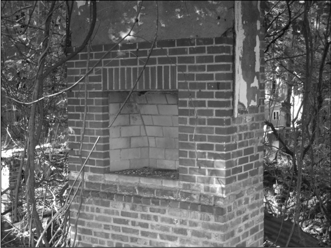
Photo 4. Fireplace looking west.
