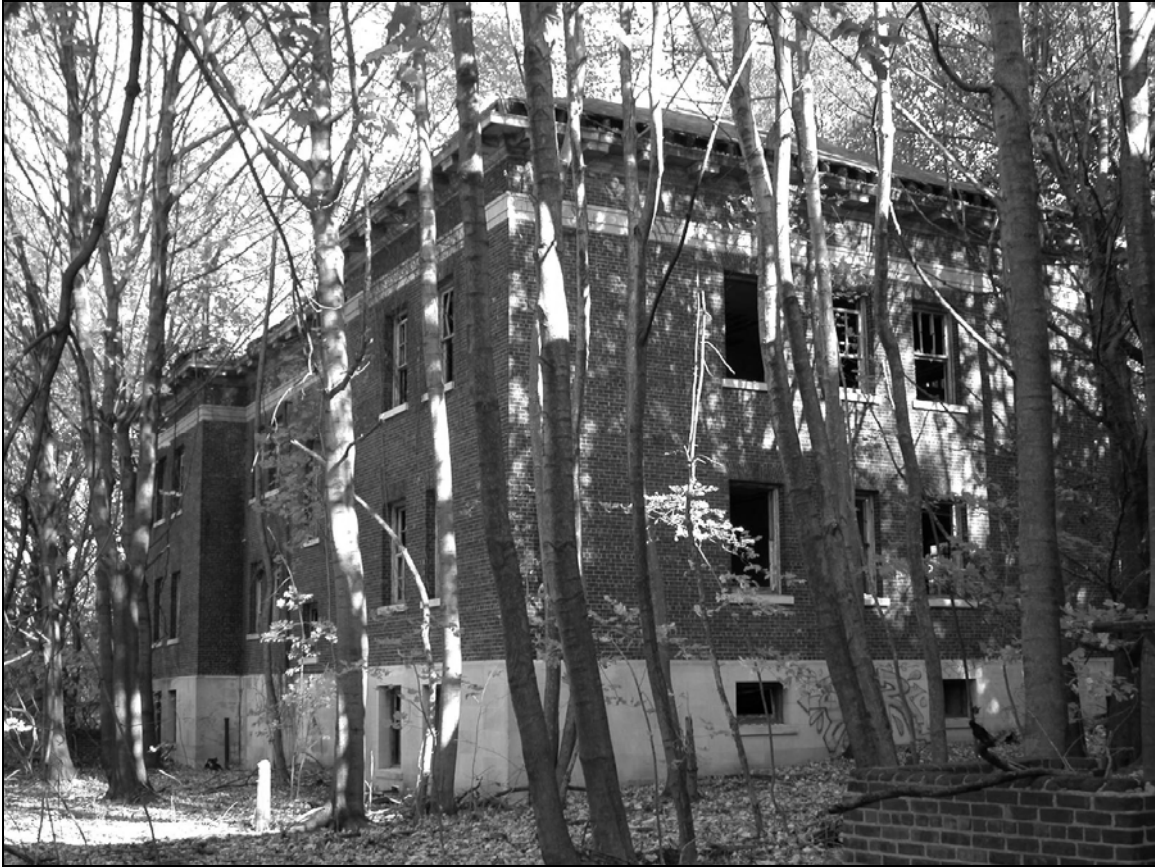
Photo 2. South and western façades, facing northeast.
