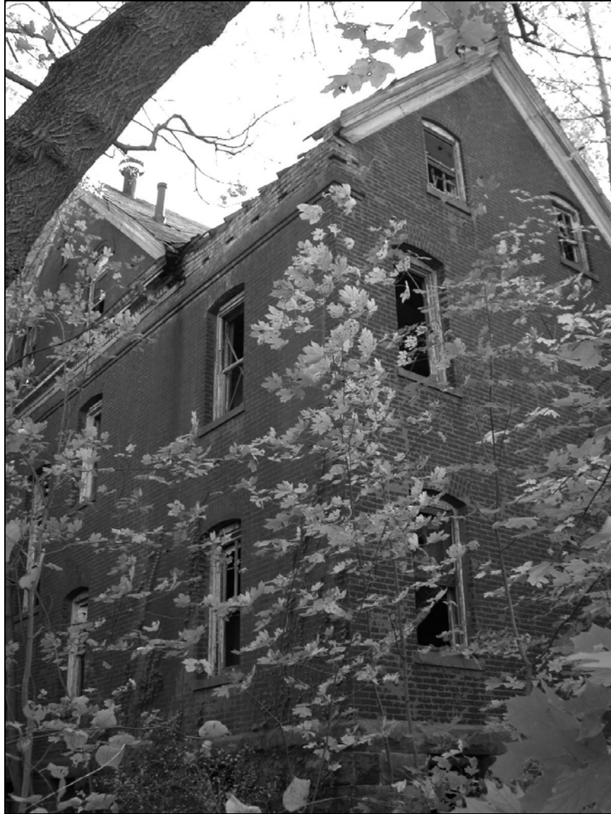
Photo 3. Northern and western façades, facing southeast.
