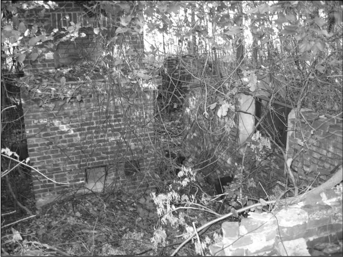
Photo 7. Foundation facing north.
