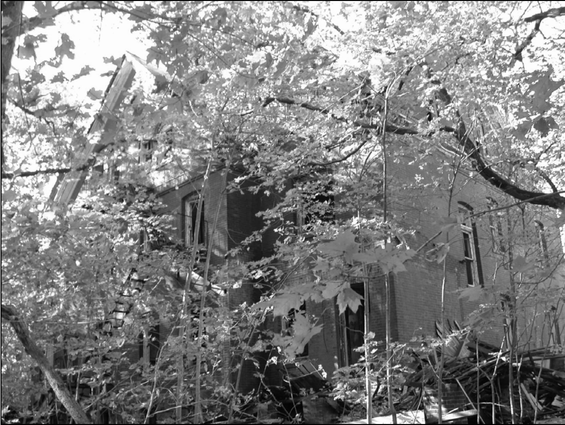
Photo 1. Northern and eastern façades, facing southwest.
