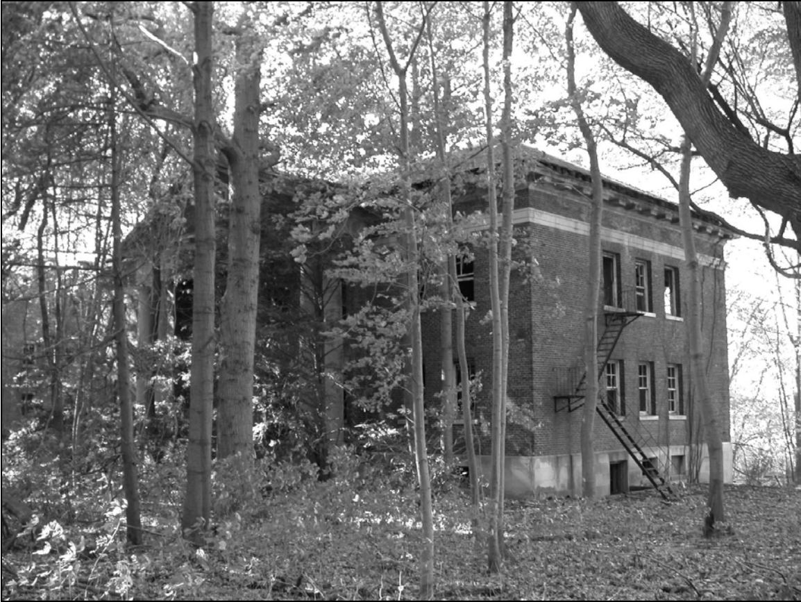
Photo 5. Northern and eastern façades, facing southwest.
