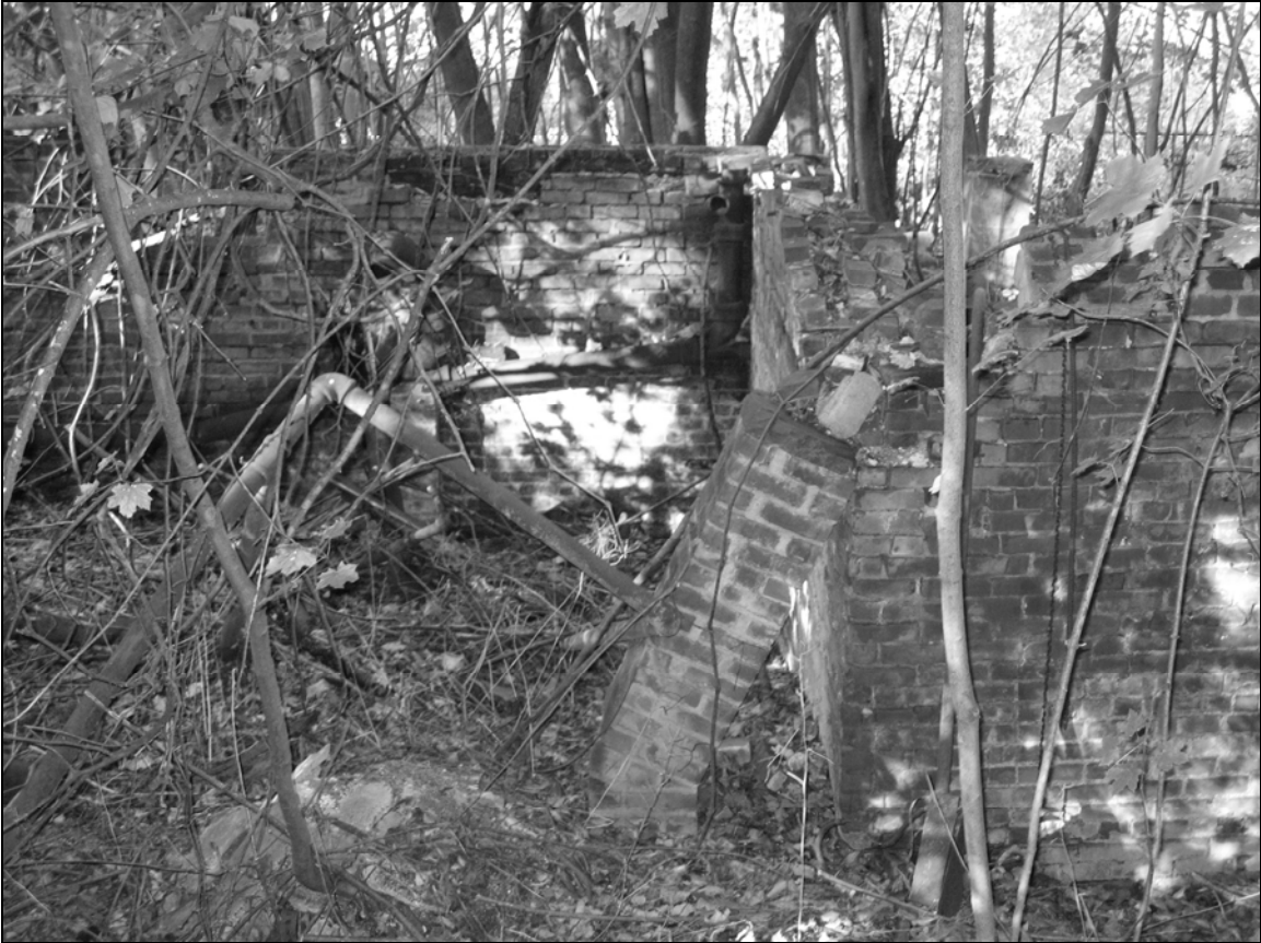
Photo 8. Foundation facing north.
