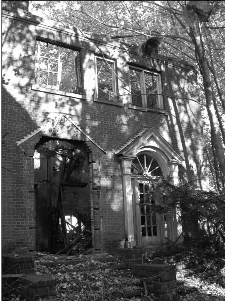
Photo 4. South façade of addition of circa 1939, showing entrance detail. Facing north.
