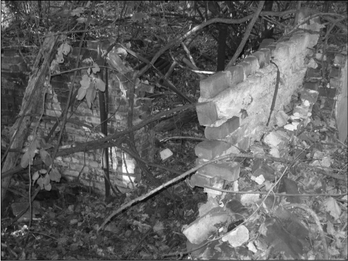
Photo 6. North wall detail.
