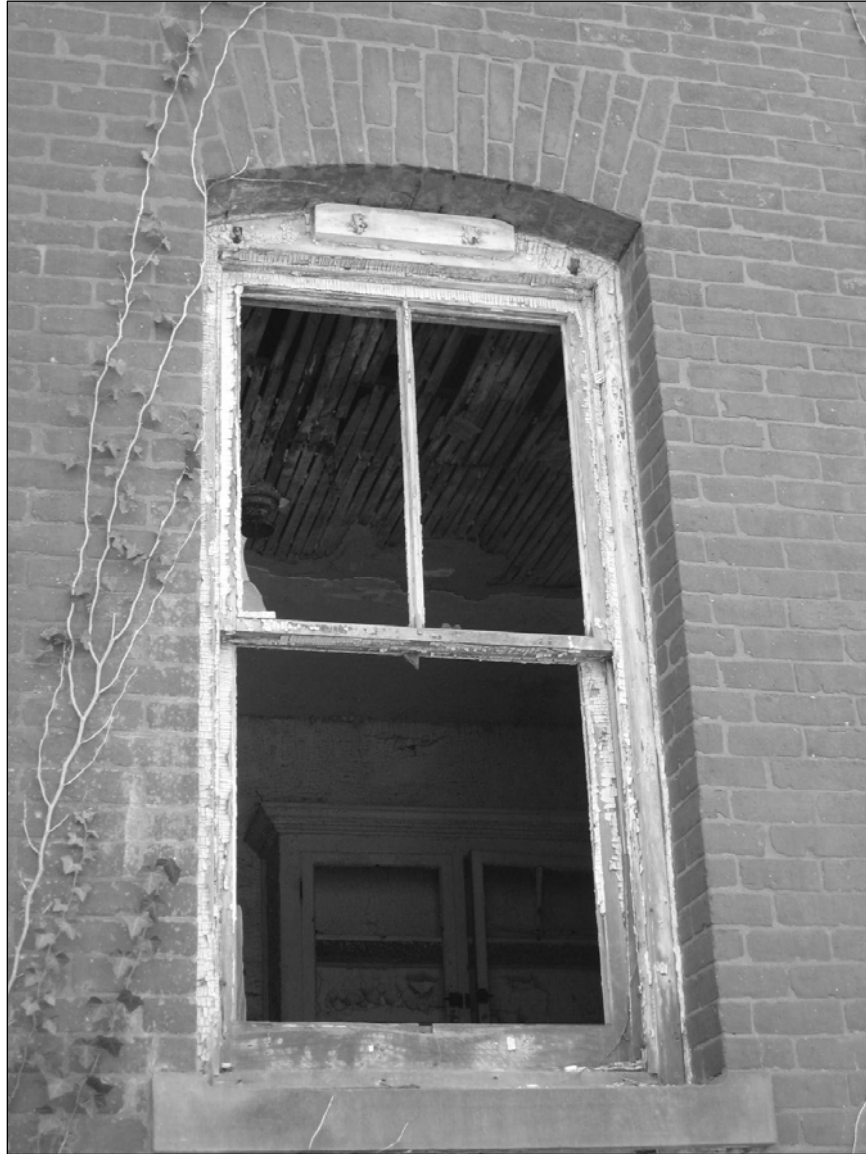
Photo 15. Northern facade, detail.
