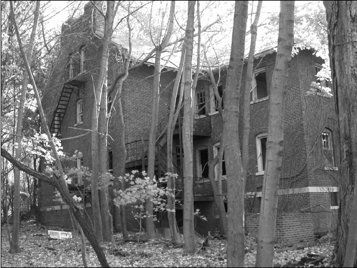
Photo 3. Northern façade, facing southeast.
