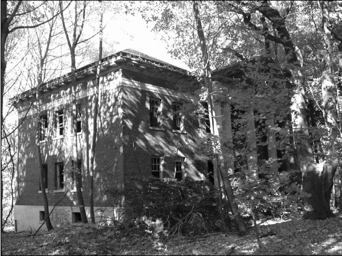
Photo 3. Southern and eastern façades, facing northwest.
