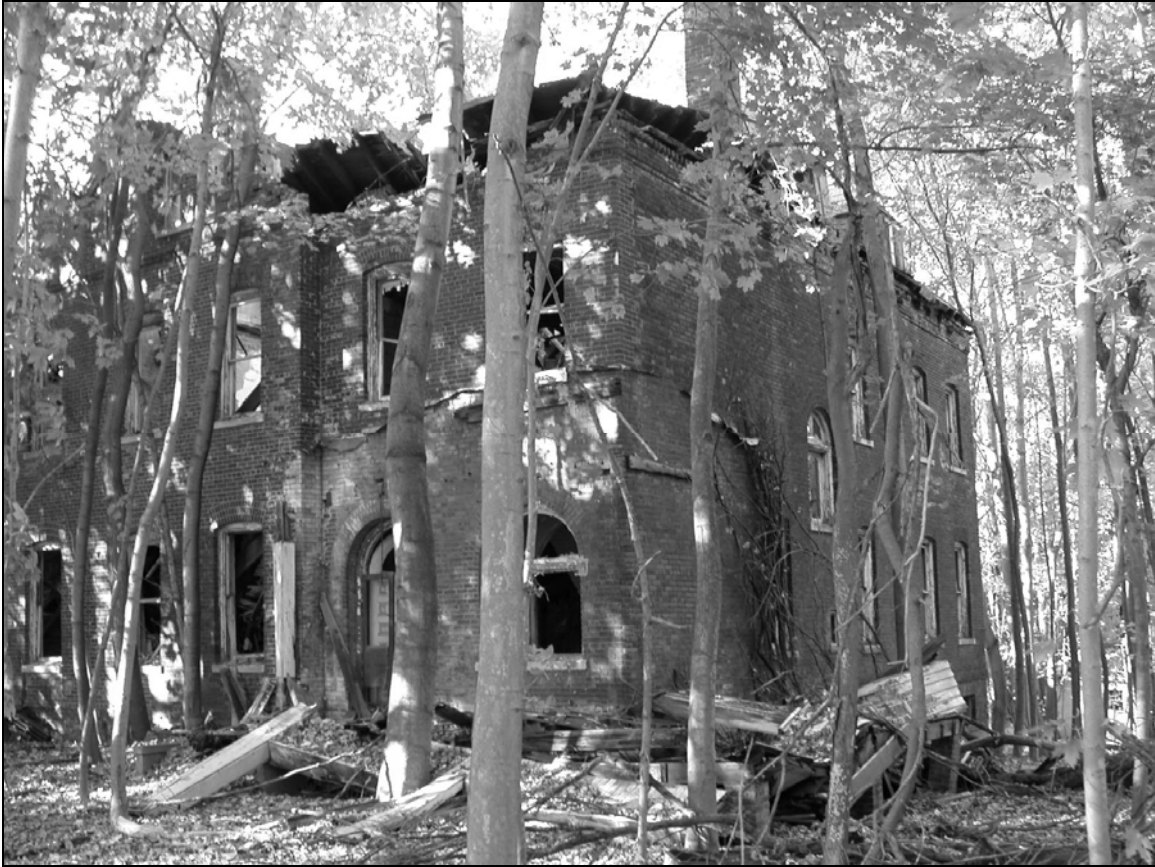
Photo 2. Eastern facade, facing southwest.
