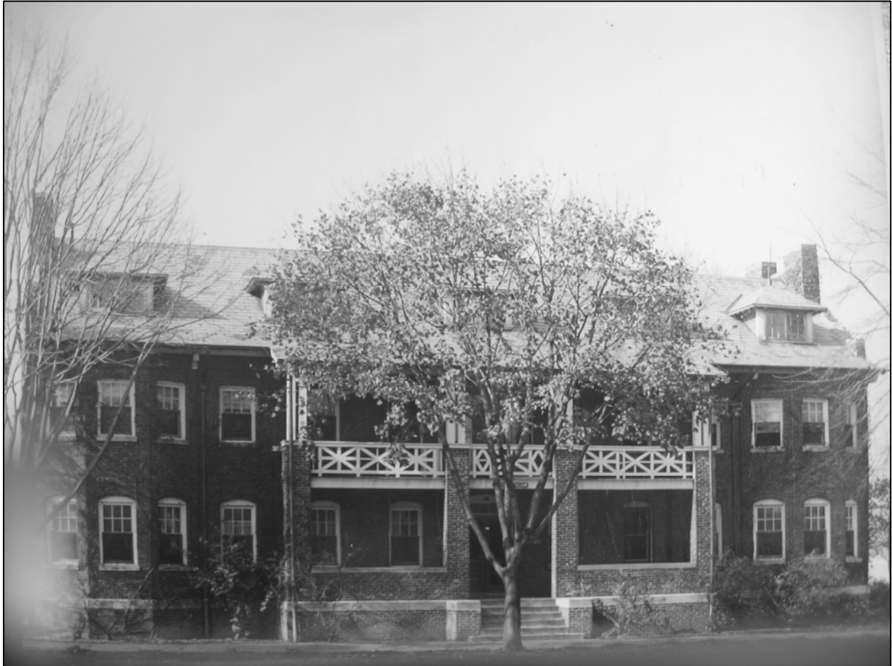
Figure 2. Inventory photo, circa 1920. View west. Record Group 111, National Archives, College Park, MD.
