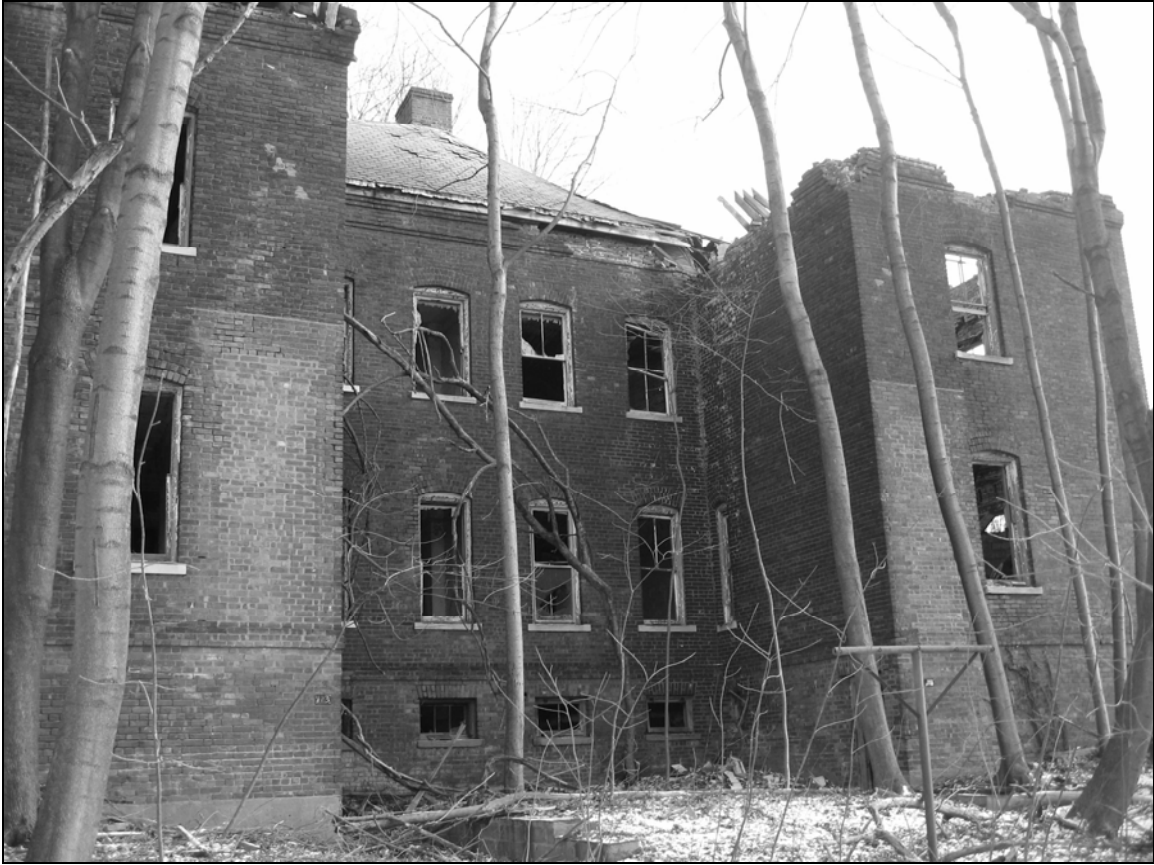
Photo 5. Western facade, facing southeast.
