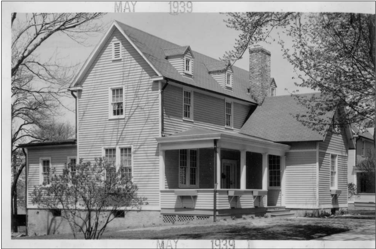
Figure 5. Property Record Photo, May 1939. View northwest. This image shows building after conversion to 2 ½-stories. Record Group 77, National Archives, College Park, MD.
