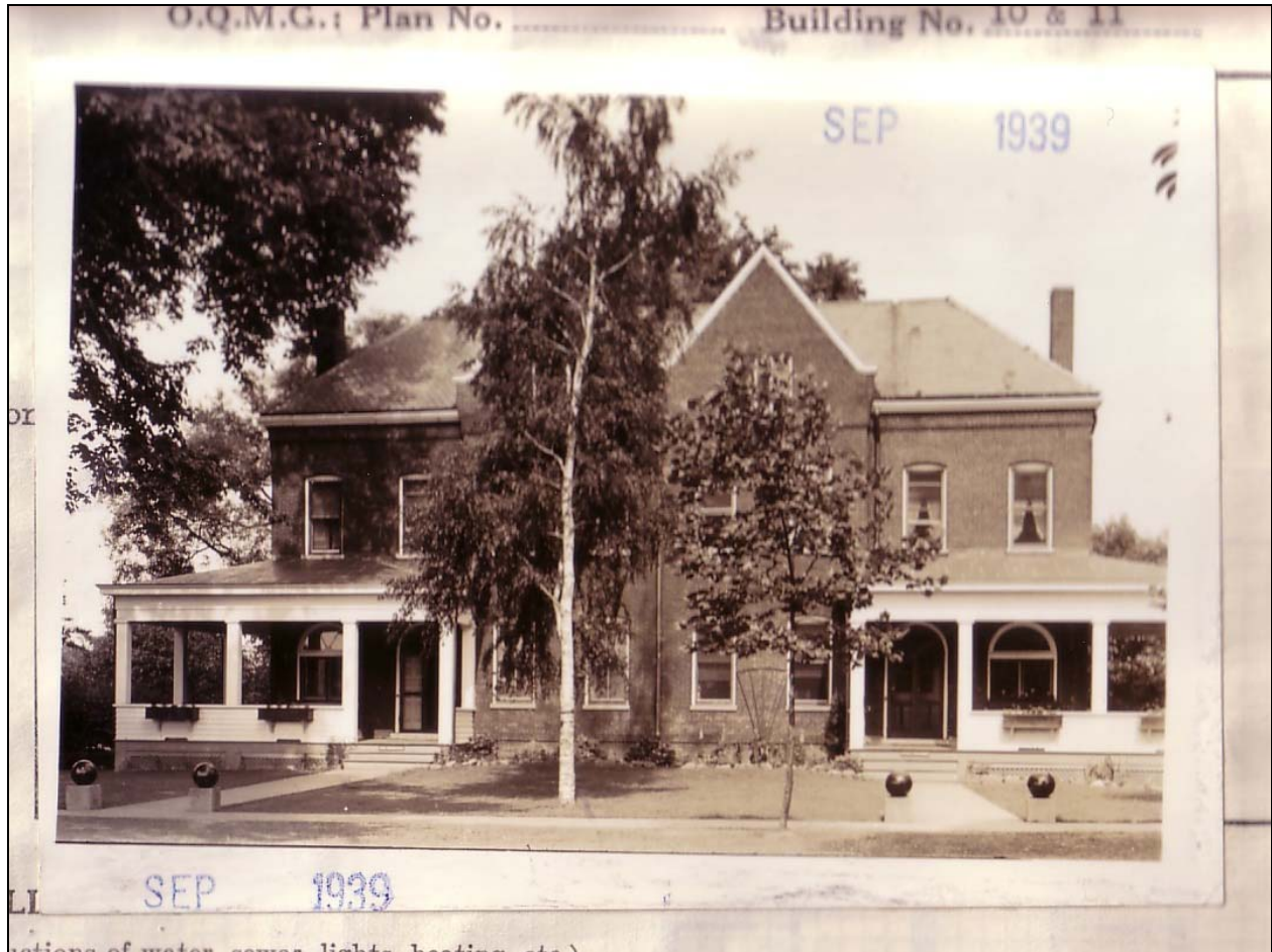
Figure 4. Property Record Photograph, September 1939. View west. Note the reconstructed and enlarged porches. Compare with Figure 5. Record Group 77, National Archives, College Park MD.
