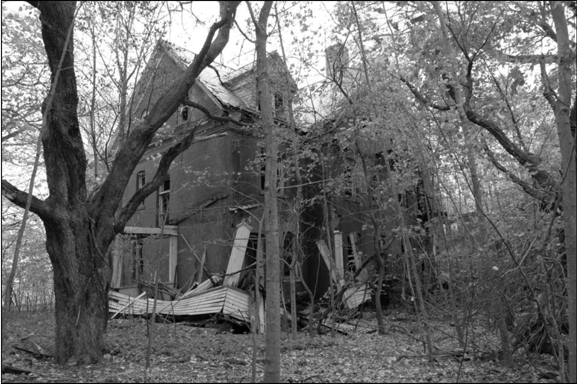
Photo 4. Southern and western façades, facing northwest.
