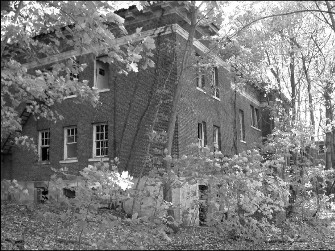
Photo 4. Northern and western façade, facing southeast.
