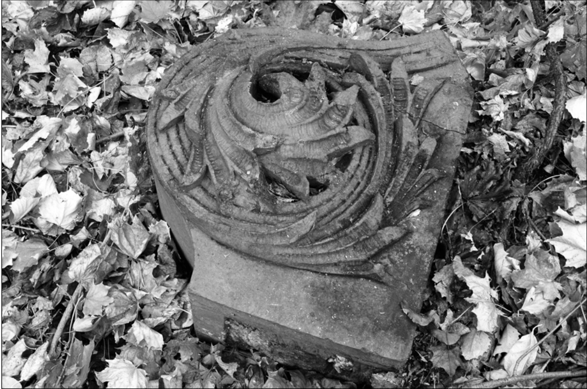
Photo 2. Terracotta parapet ornament from cross gable.
