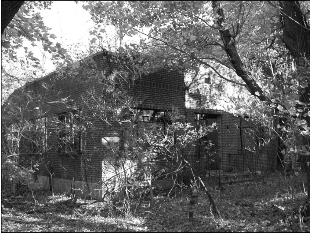
Photo 5. South and west façades of circa 1955 addition, facing northeast.
