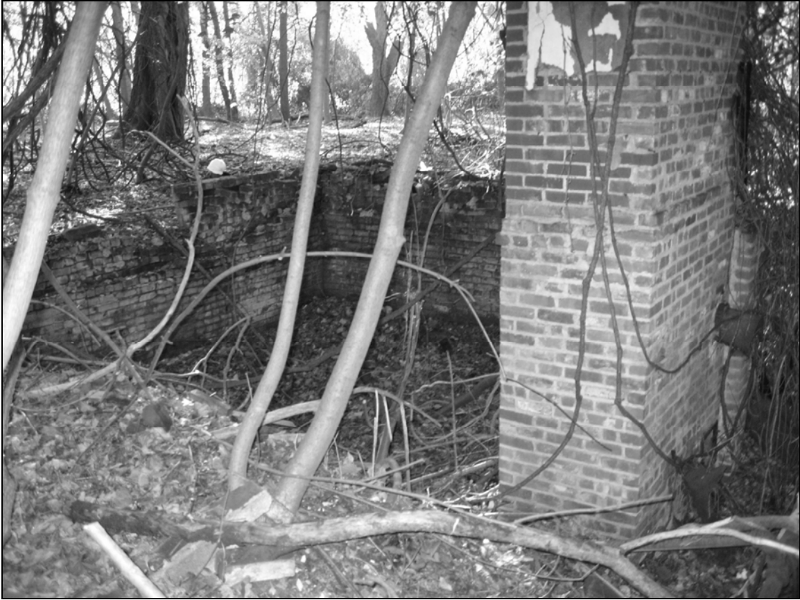
Photo 5. Foundation looking southwest.
