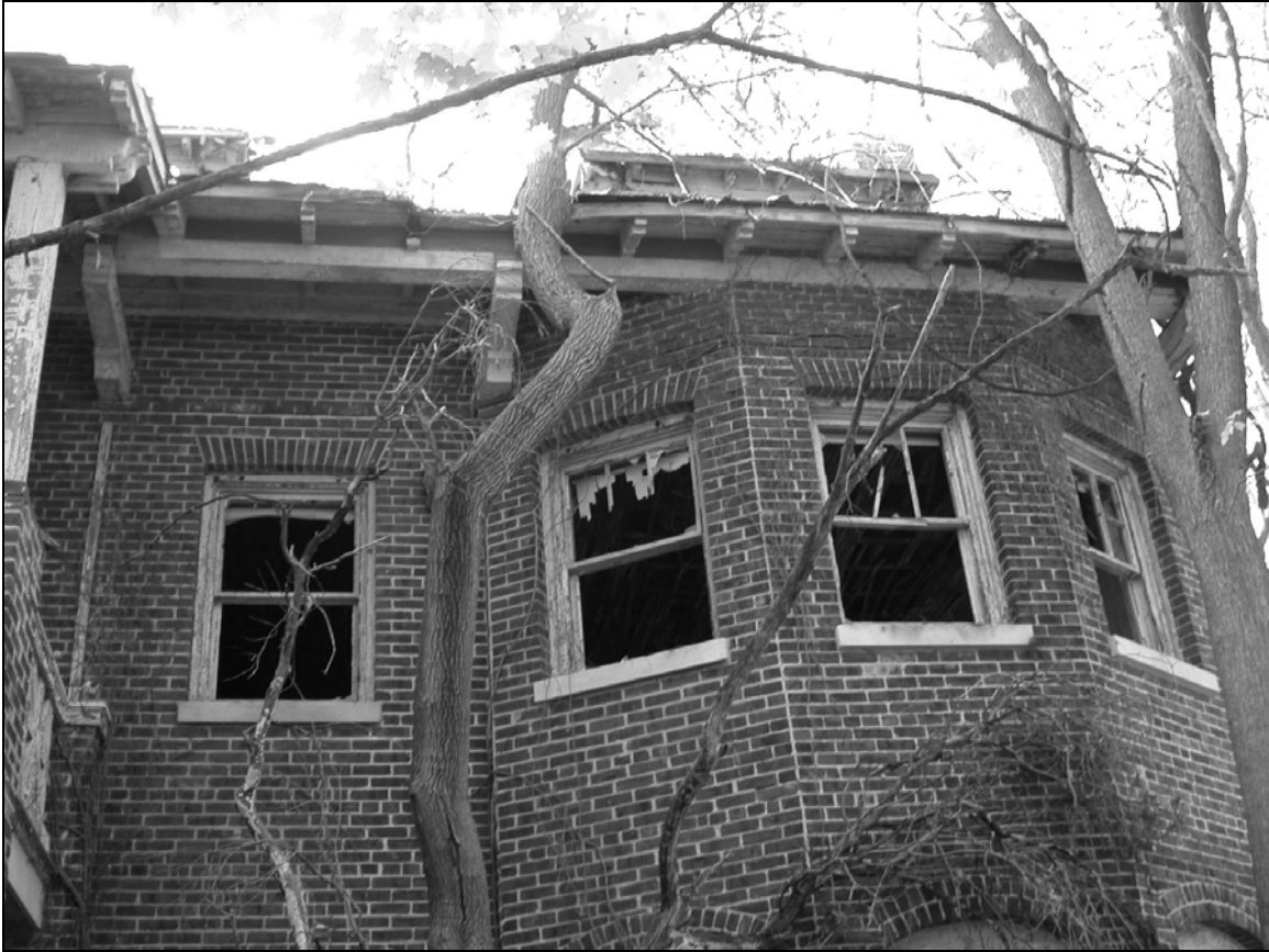
Photo 5. Eastern façade, detail.
