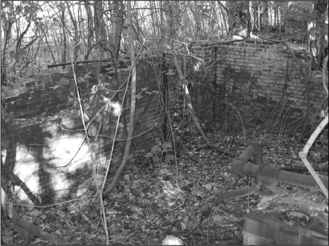
Photo 4. Cellar facing east.
