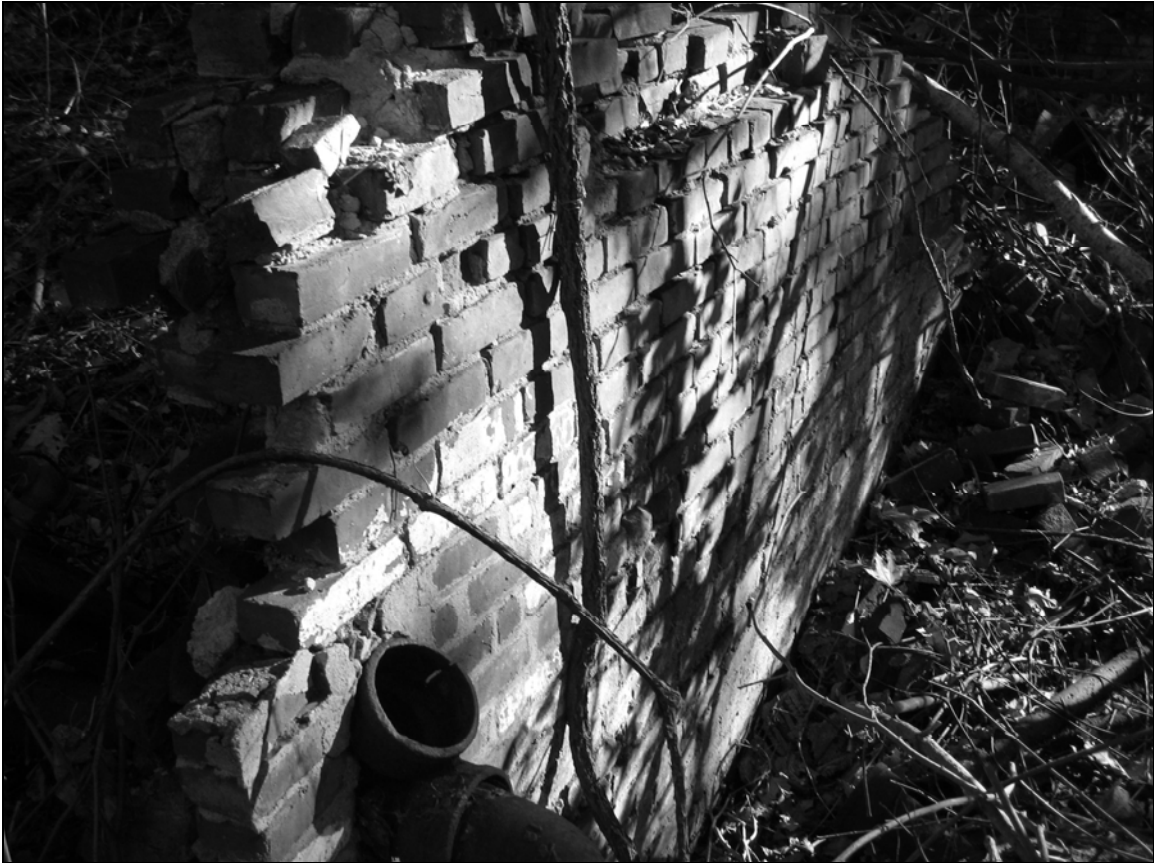
Photo 3. North wall looking south.
