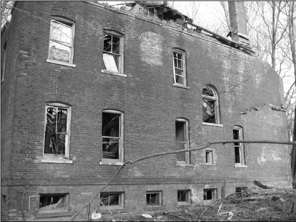
Photo 7. Southern facade, facing north.
