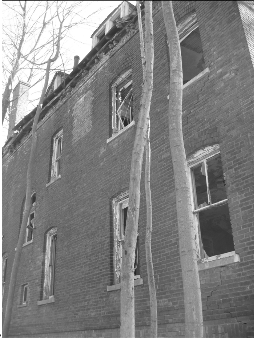
Photo 4. Eastern facade, facing southeast.
