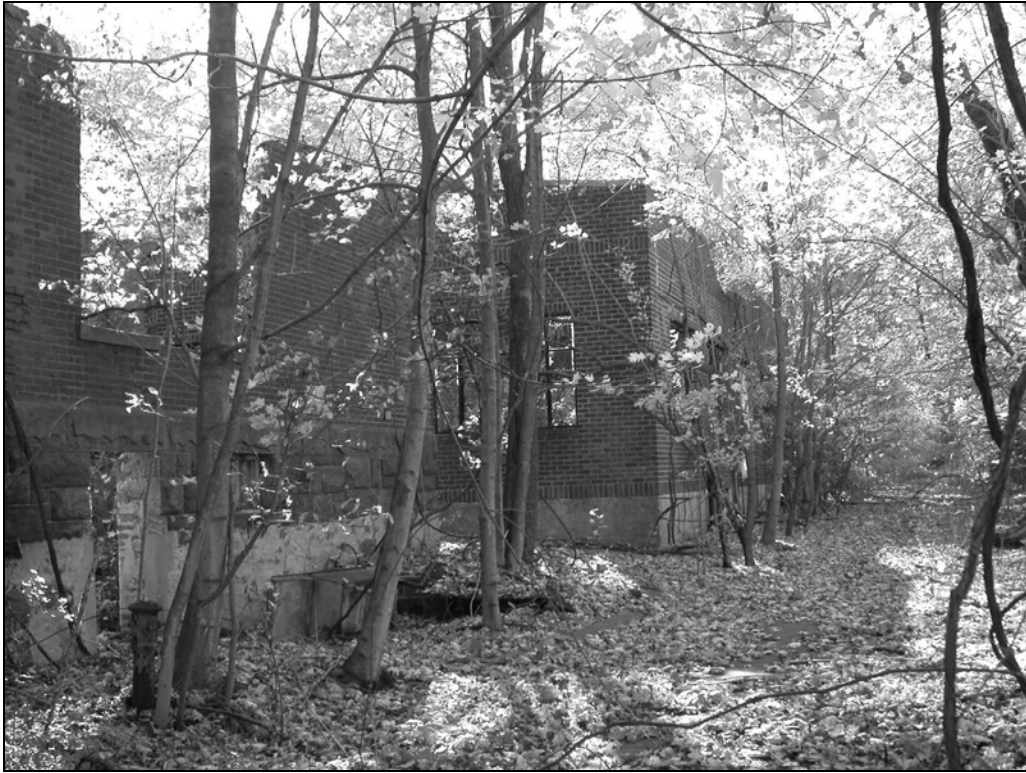
Photo 6. West façade facing southeast, showing original building at left and circa 1955 addition at center. Howard Road is at right.
