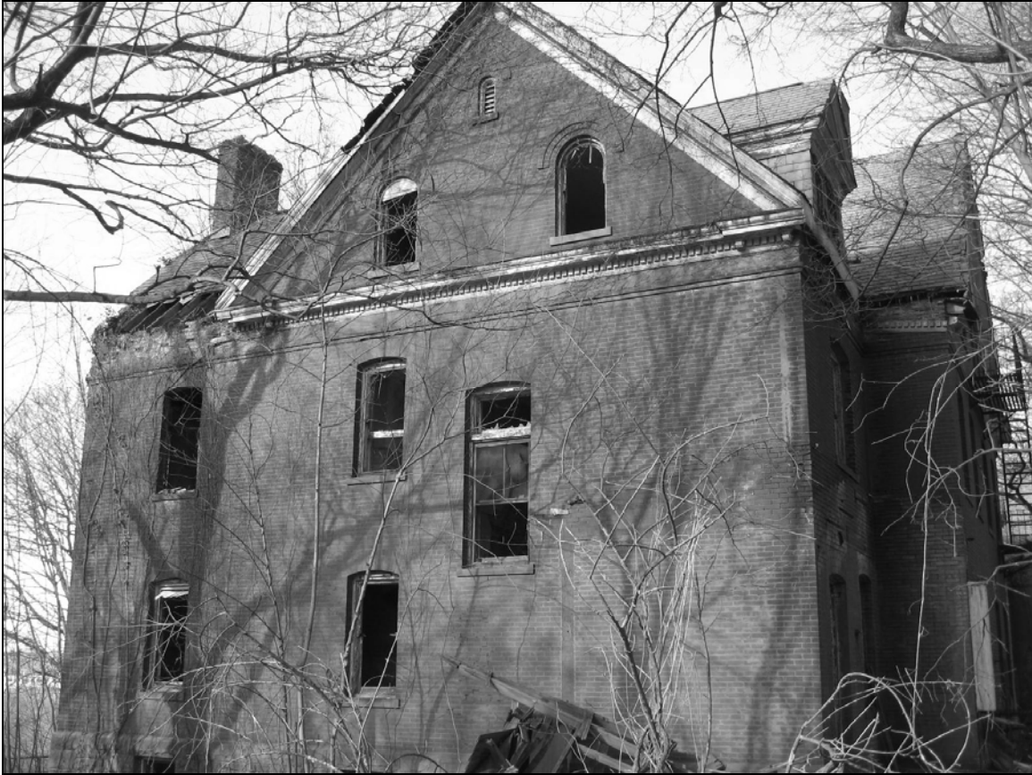
Photo 8. Southern facade, facing north.
