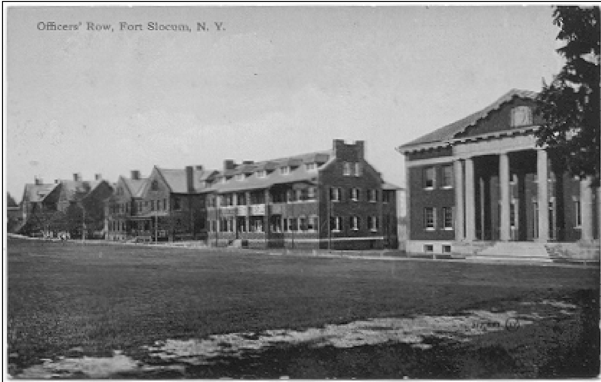
Figure 4. Undated postcard, "Officers' Row, Fort Slocum, N.Y." Building 13 is at far right. View to southwest. Fort Slocum Collection, New Rochelle Public Library, New Rochelle, NY.
