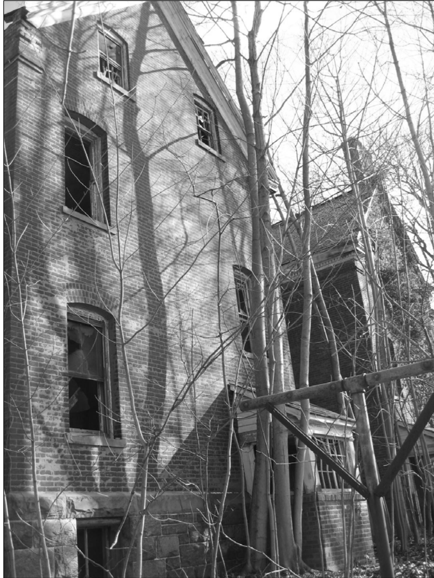
Photo 16. Western facade, facing southeast.
