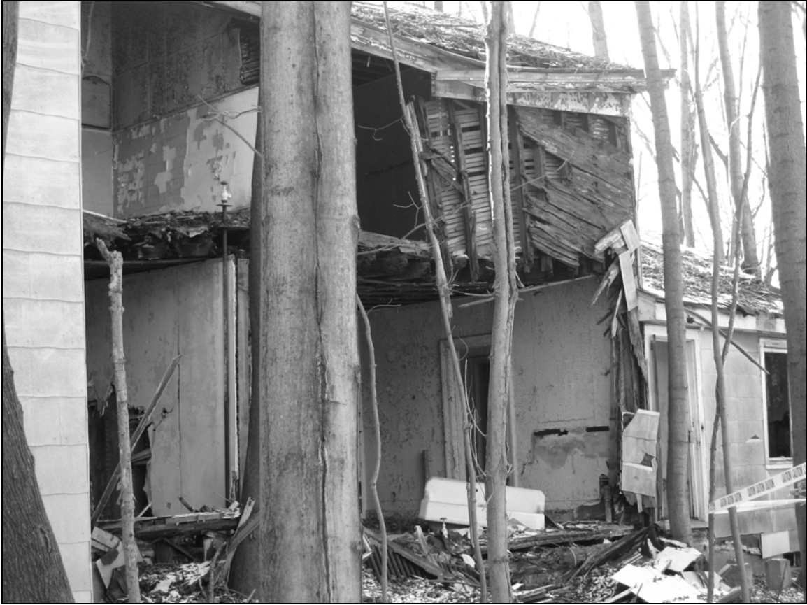
Photo 13. Northern façade, facing southwest.
