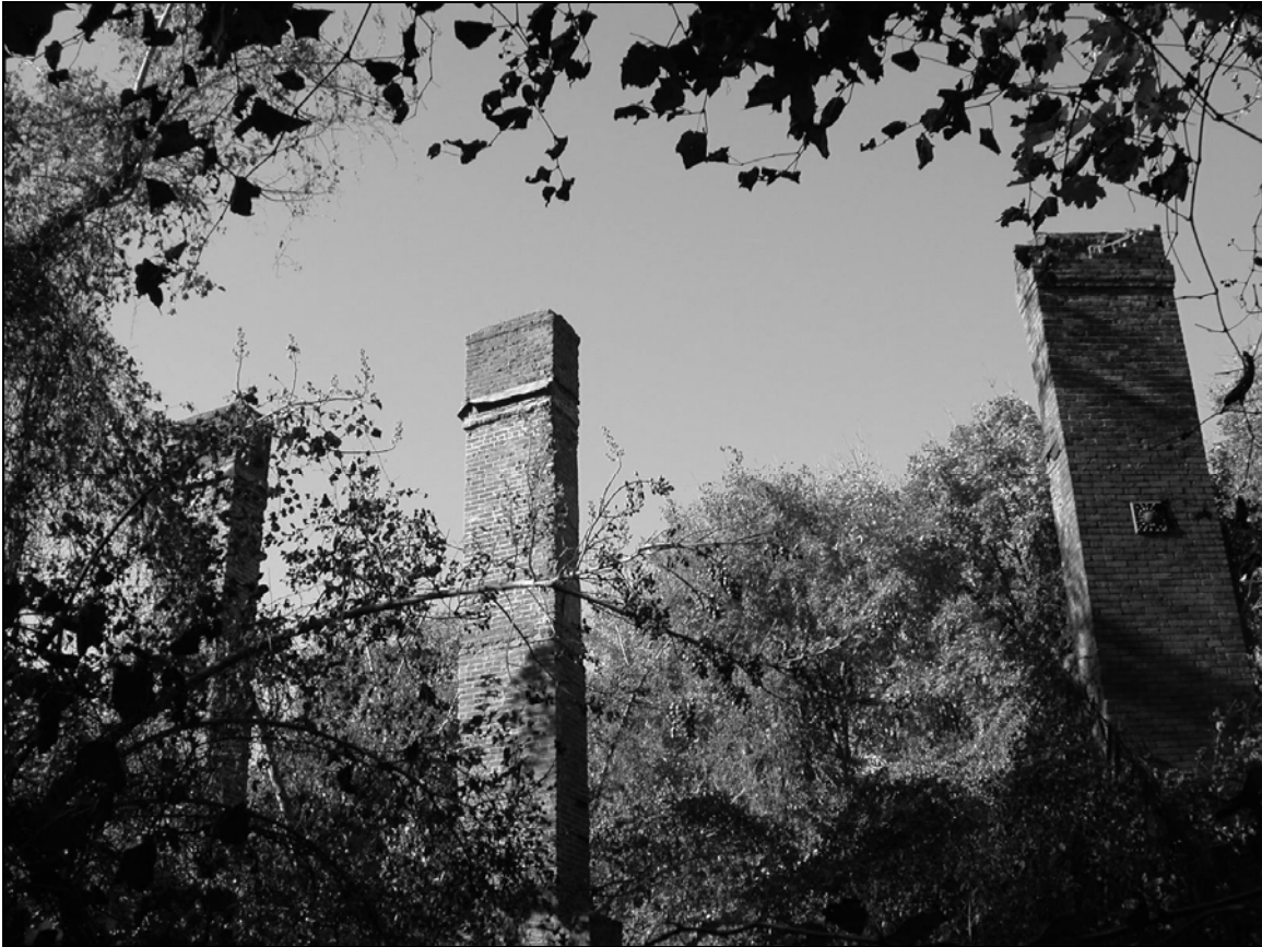
Photo 4. View facing west.
