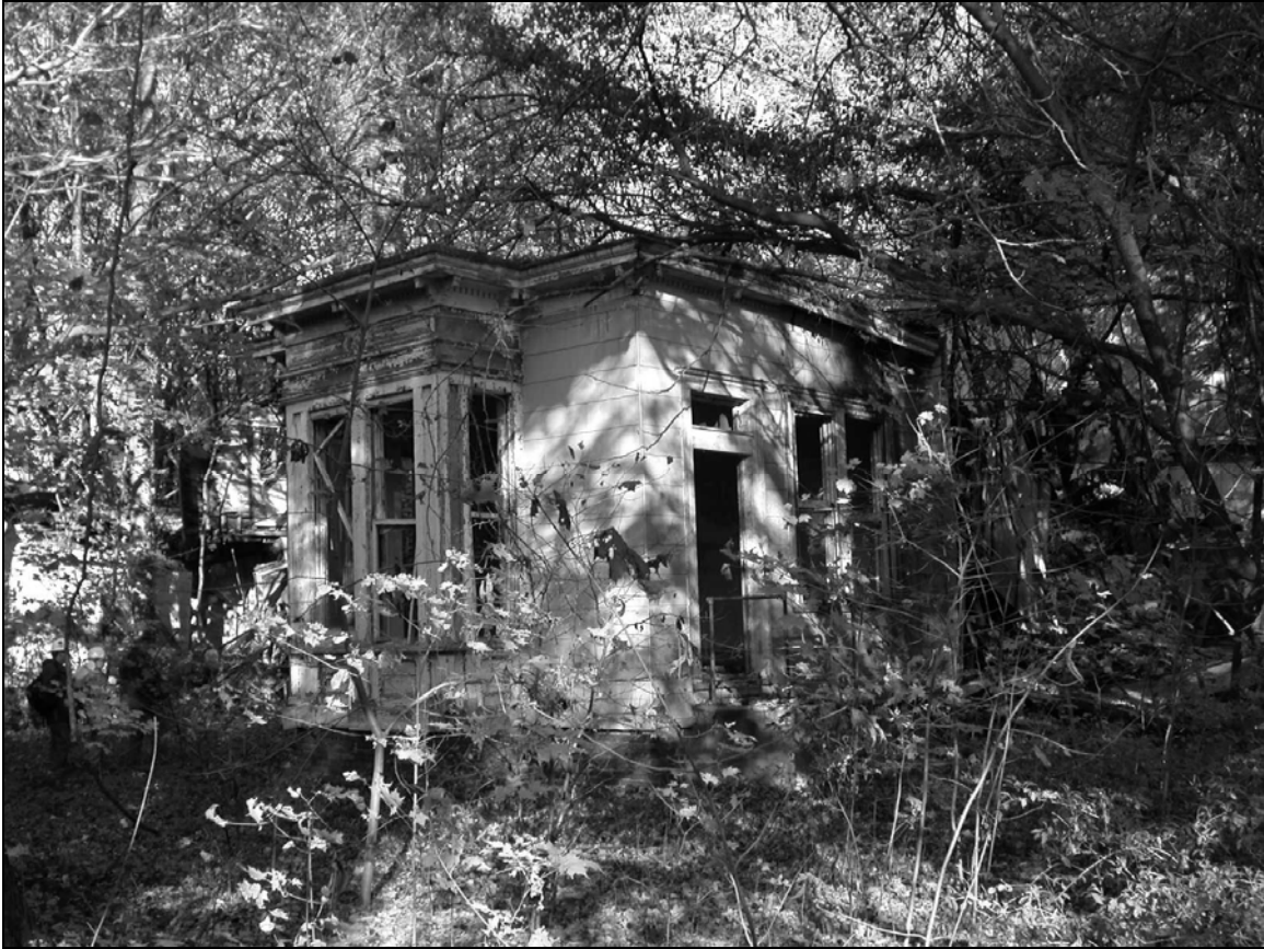
Photo 3. Southeast corner detail, facing northwest.
