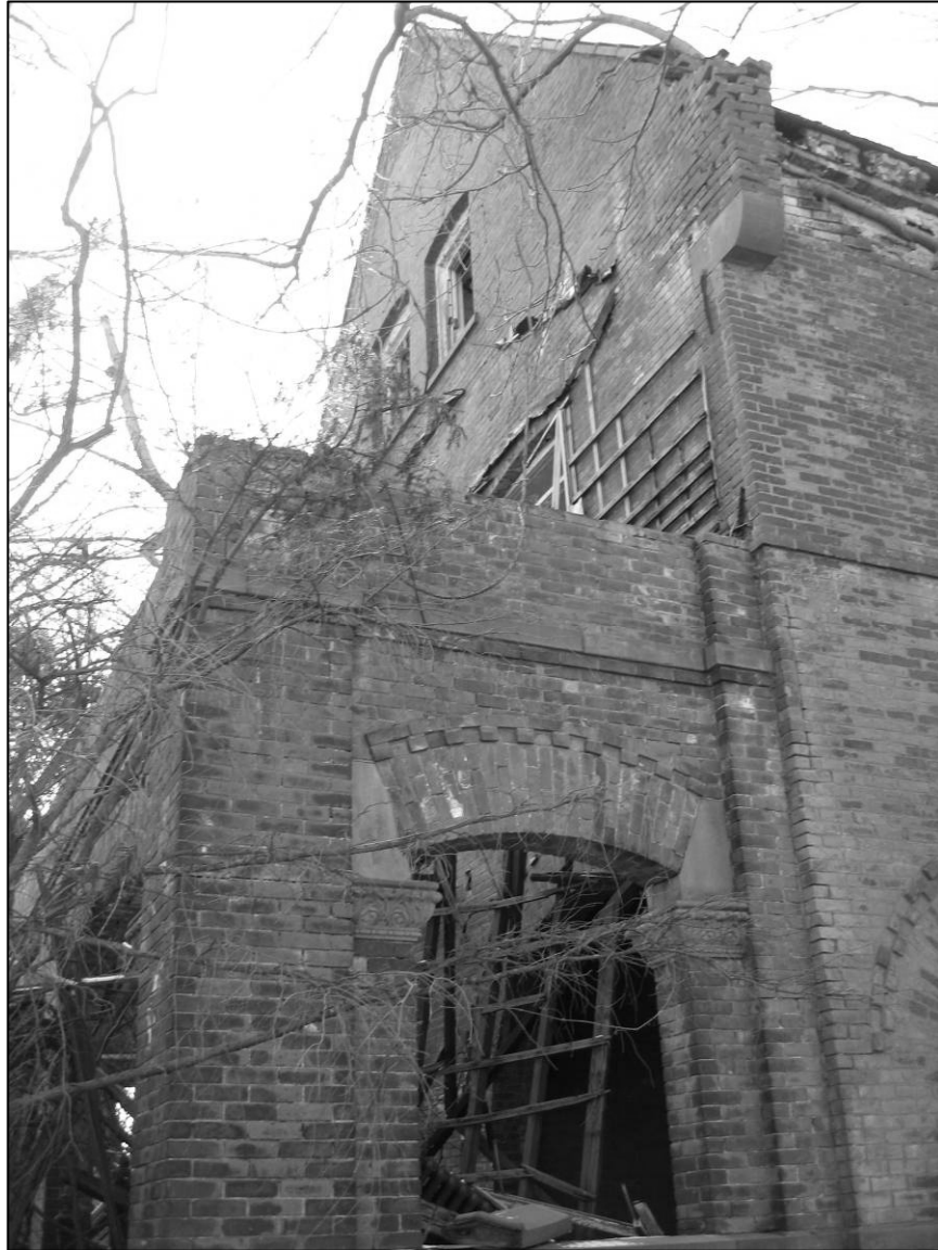
Photo 7. Eastern and northern façades, facing south.
