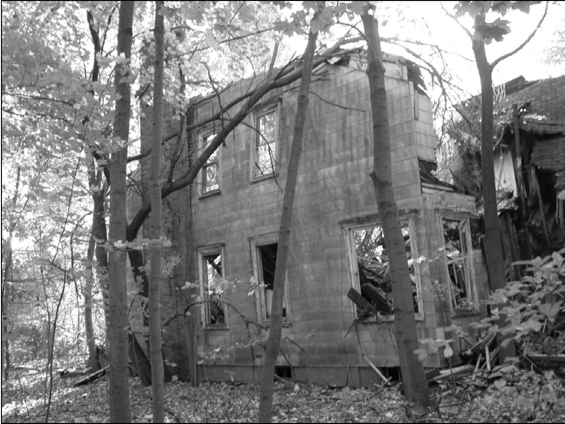
Photo 4. Northern facade, facing south.
