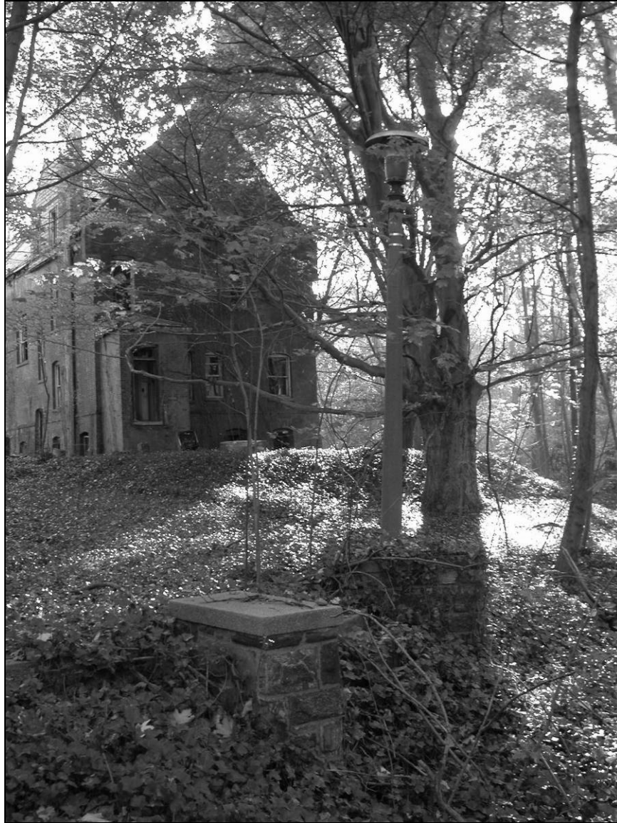
Photo 3. View of building and rear yard, facing southeast.
