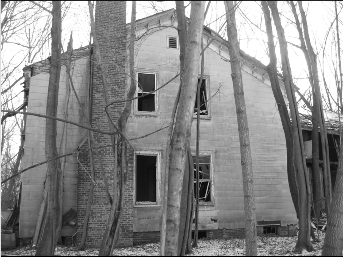
Photo 12. Northern façade, facing south.
