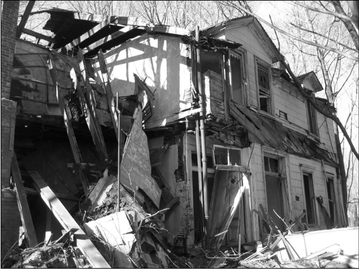
Photo 8. Eastern façade, facing northeast.
