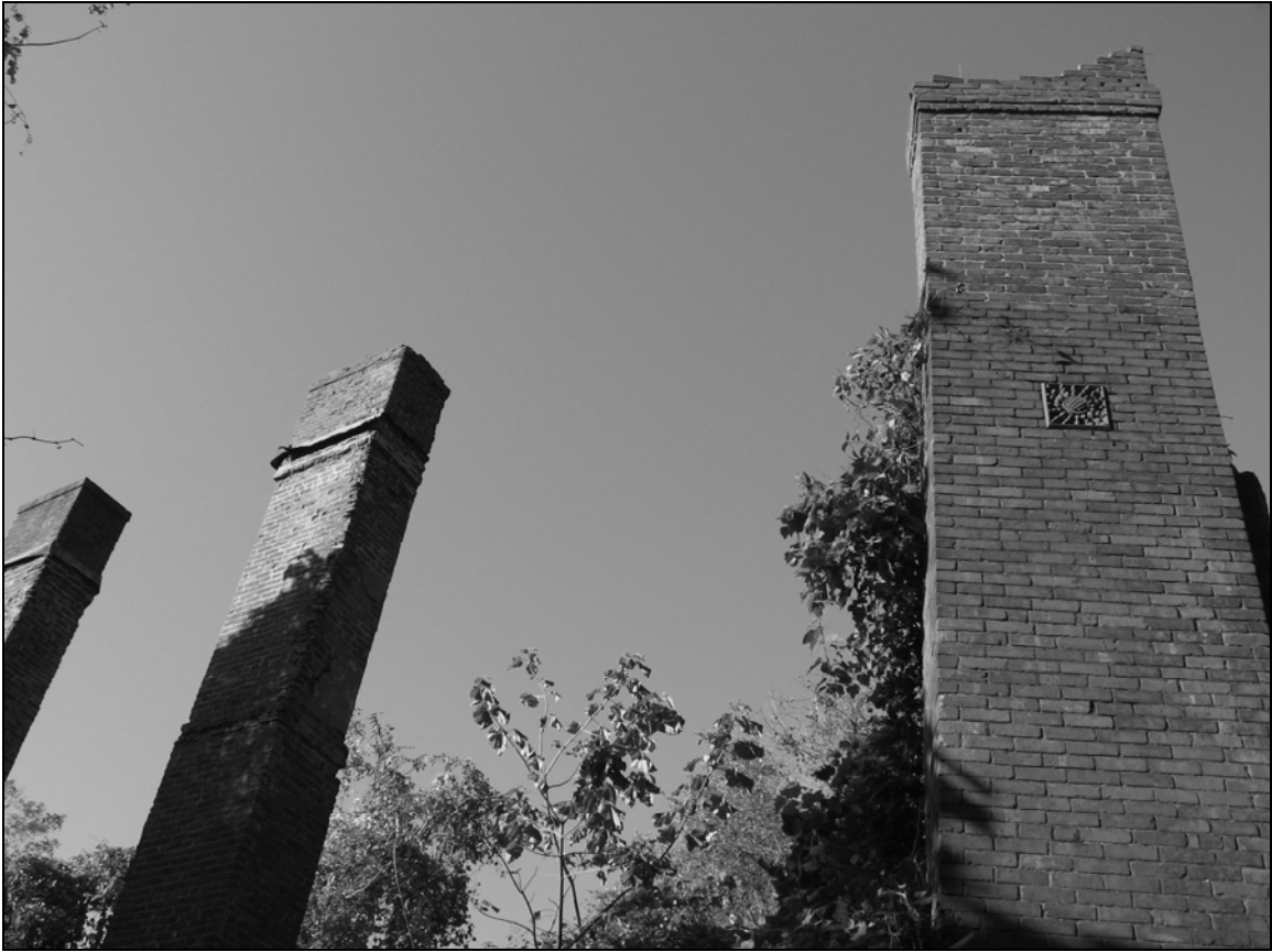
Photo 7. Chimneys facing southwest.
