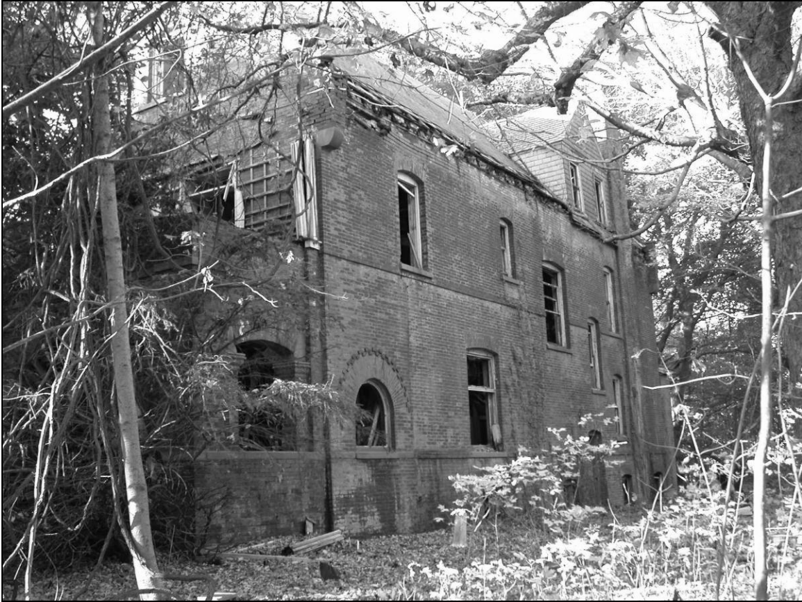
Photo 4. Northern façade, facing southwest.
