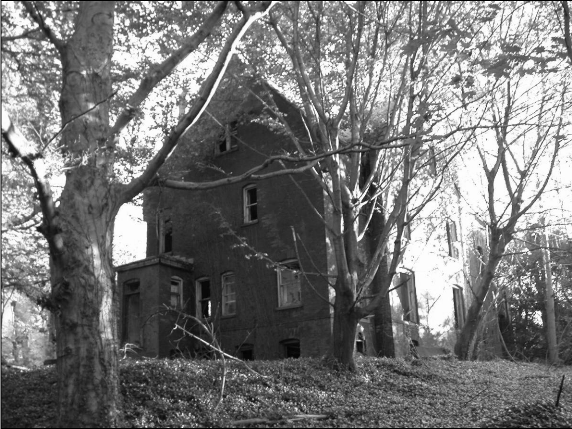
Photo 1. Western and southern façades, facing northeast.
