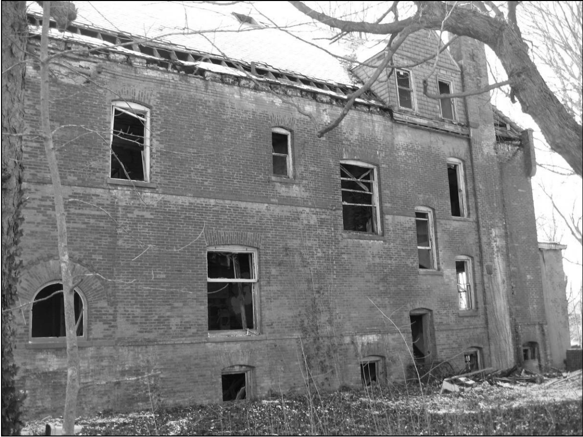
Photo 8. Northern façade, facing south.
