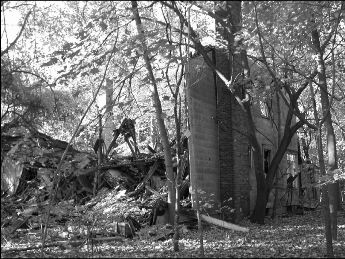
Photo 5. North facade, looking southwest.
