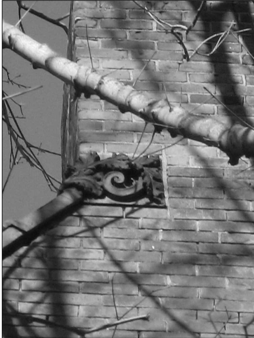
Photo 17. Terra cotta detail, southern façade.
