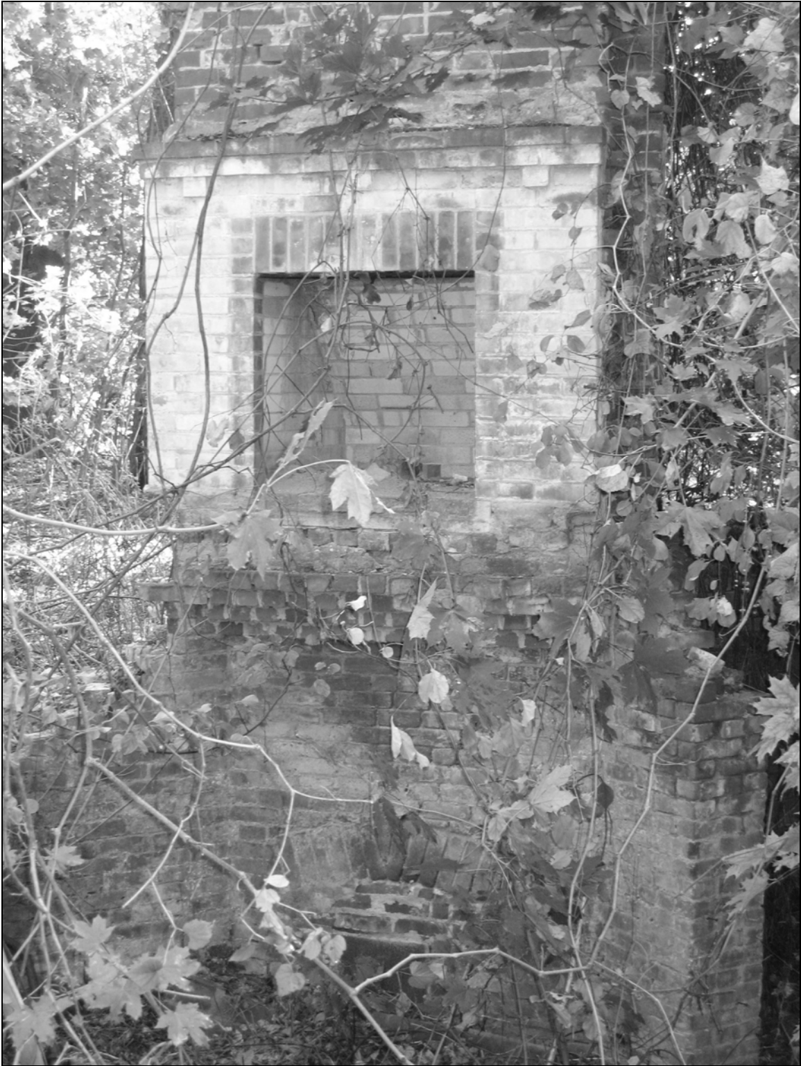
Photo 6. North chimney facing east.
