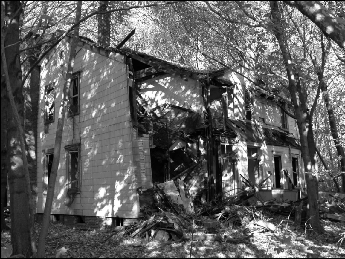
Photo 3. Southern and eastern façades, facing northwest.
