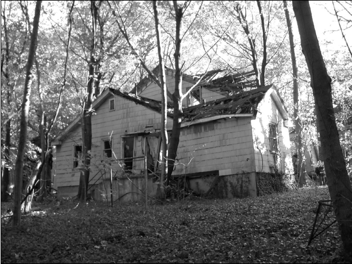
Photo 2. Western facade, facing northeast.
