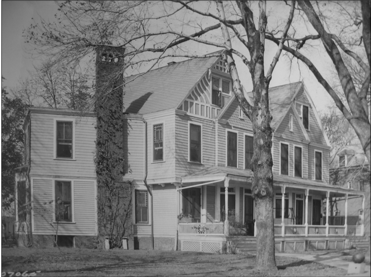
Figure 8. Circa 1920 inventory photo. View northwest. Note the angled orientation of the southern wing to the main section of the house. Record Group 111, National Archives, College Park, MD.
