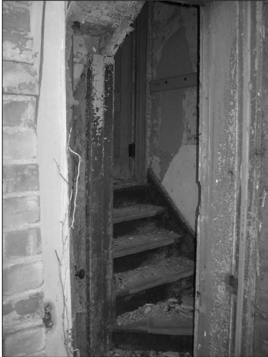
Photo 9. Interior, rear entry.
