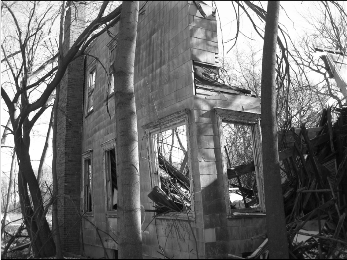
Photo 10. Northern facade, facing southeast.
