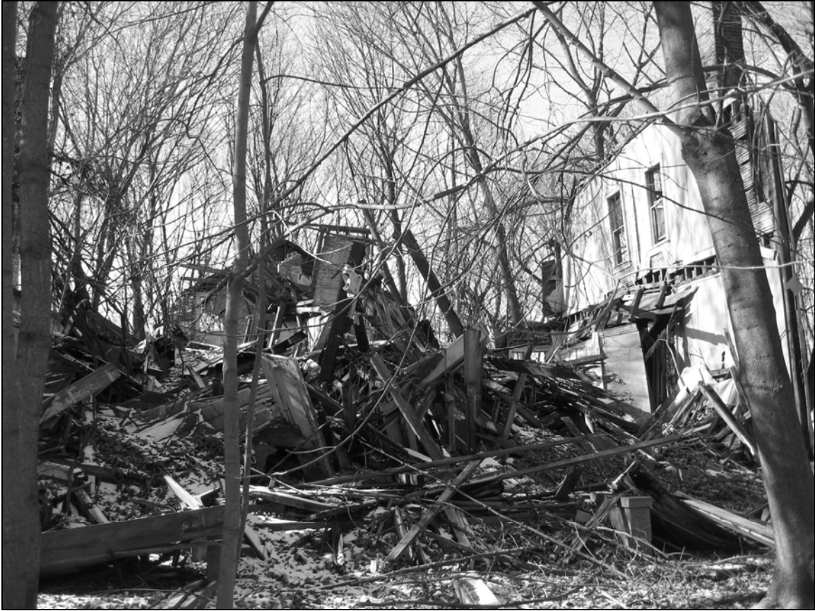
Photo 8. General site view, facing west.
