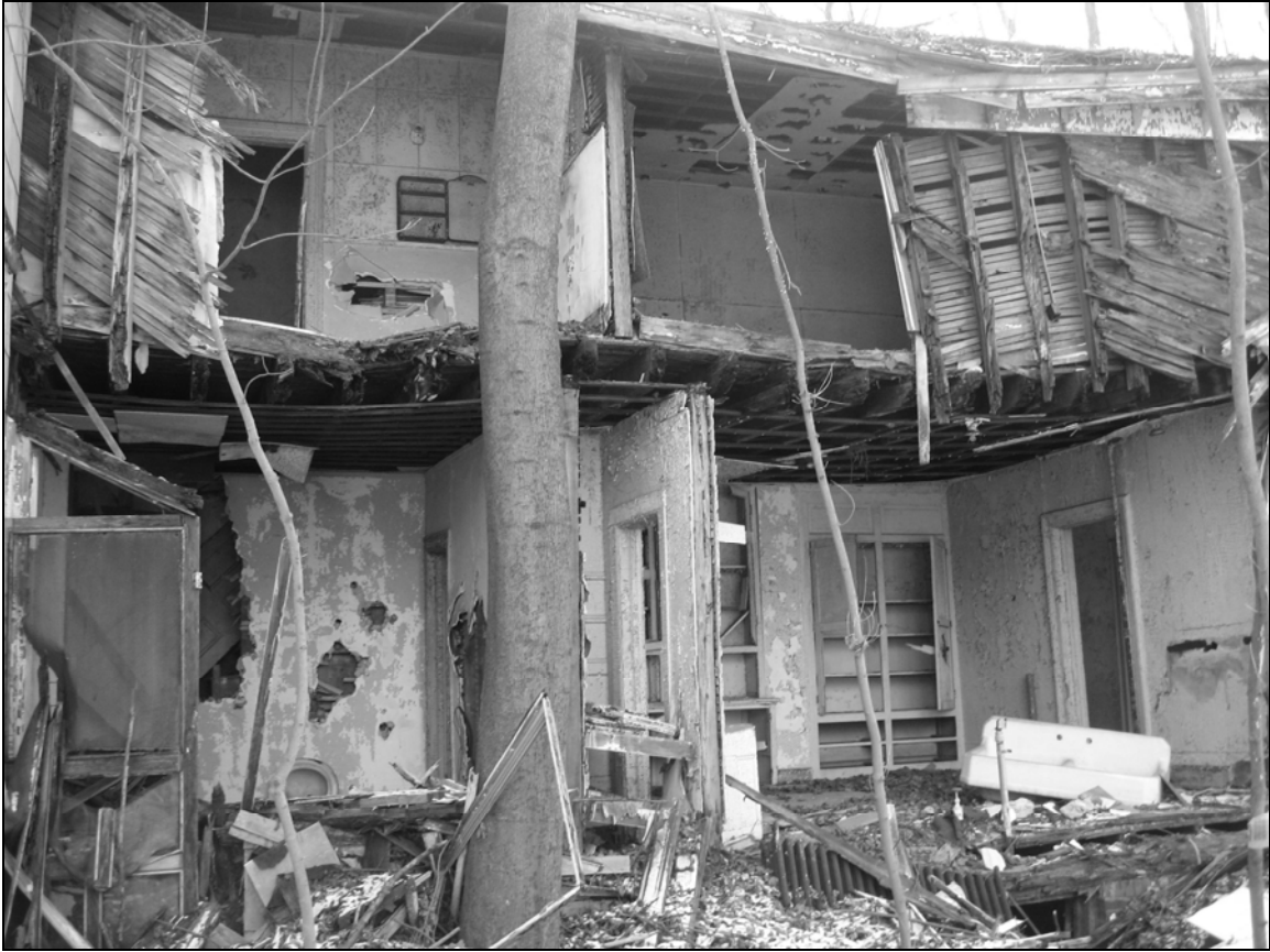
Photo 14. Northern façade, facing southwest.
