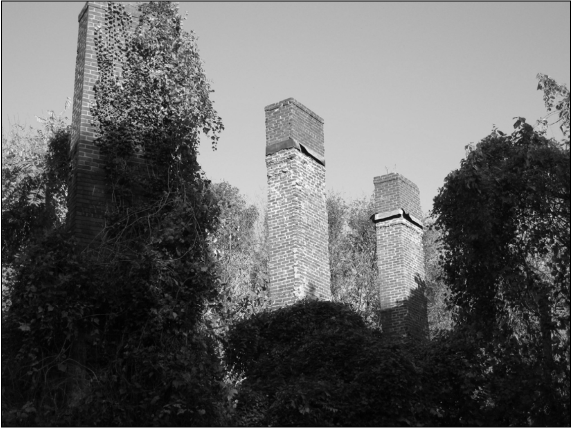
Photo 8. Chimneys facing northwest.
