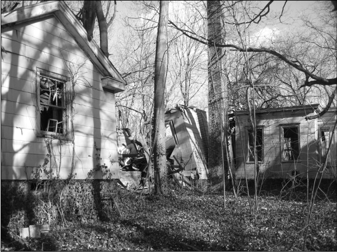
Photo 12. Southern facade, facing northeast.
