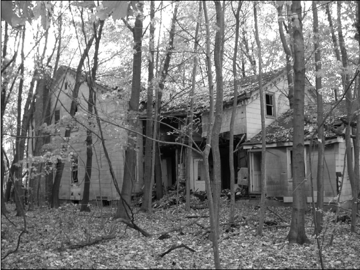
Photo 4. Northern façade, facing southeast.
