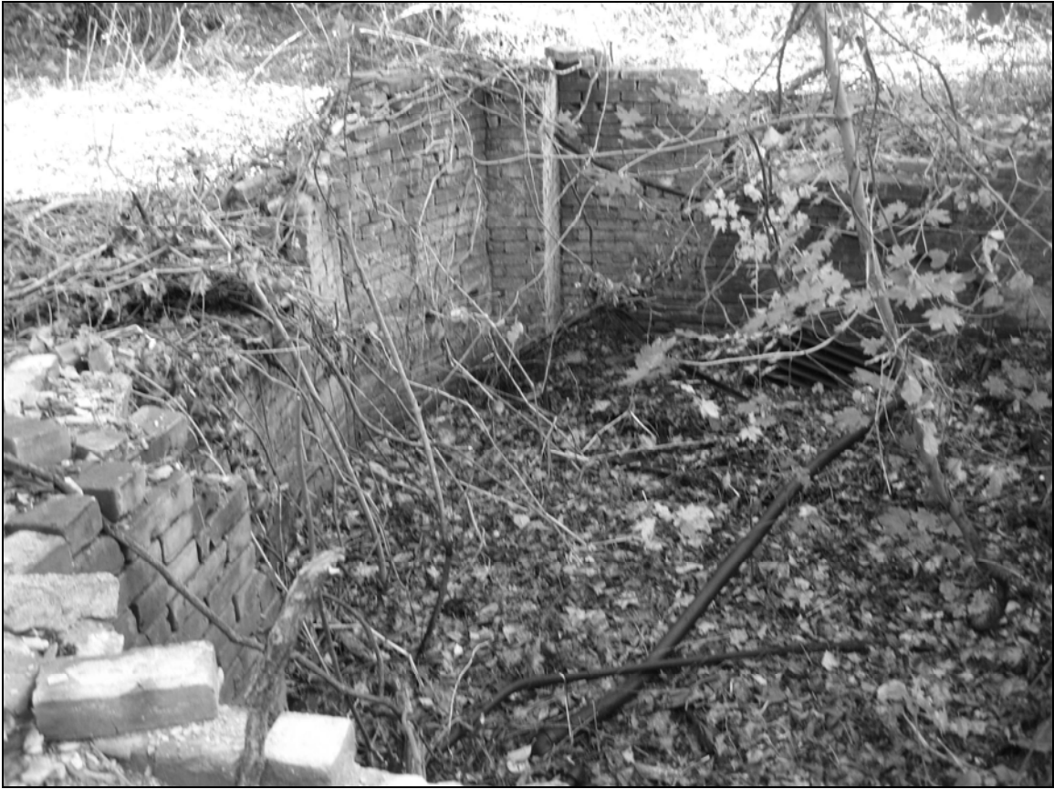
Photo 11. Foundation facing north.
