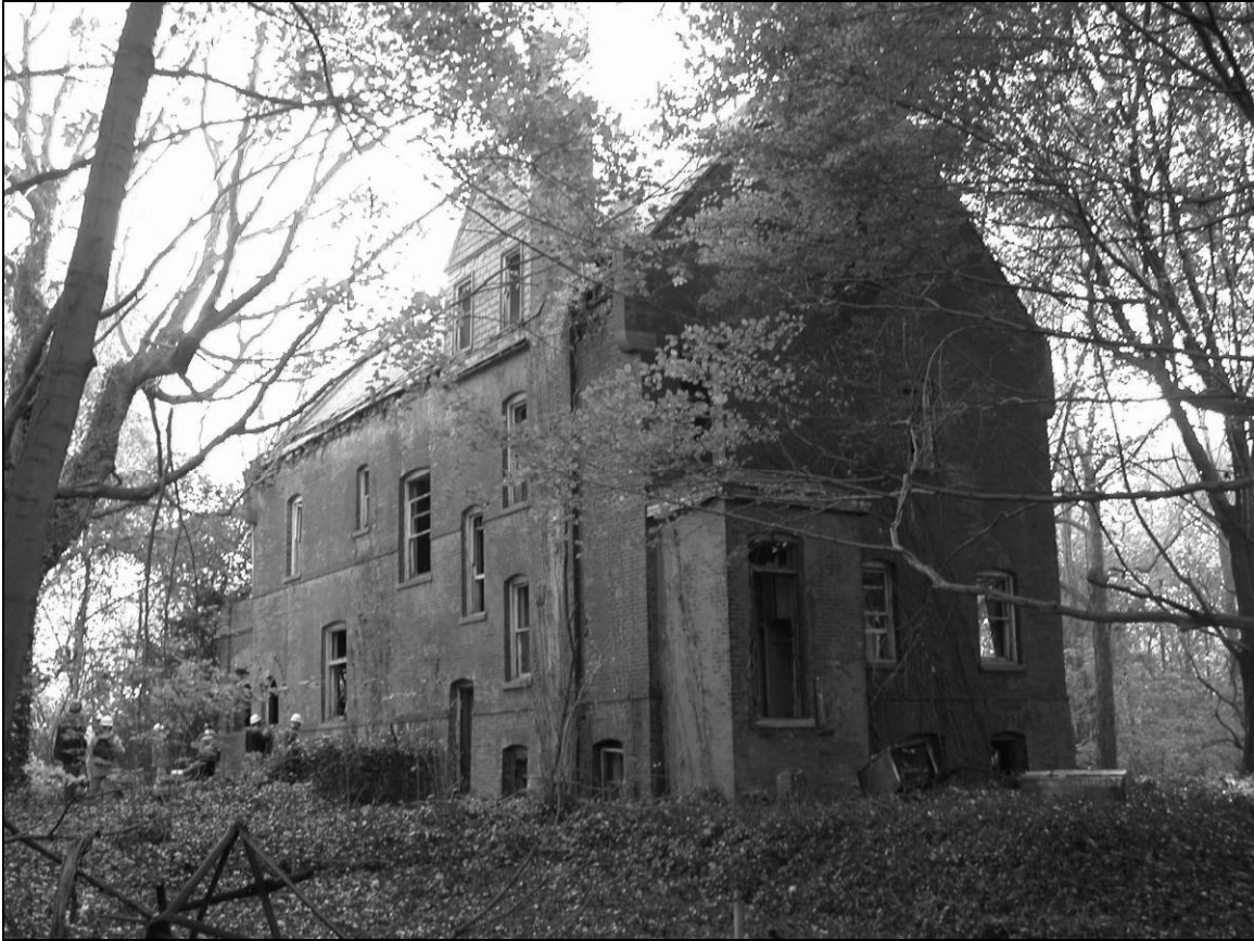
Photo 2. Northern and western façades, facing southeast.
