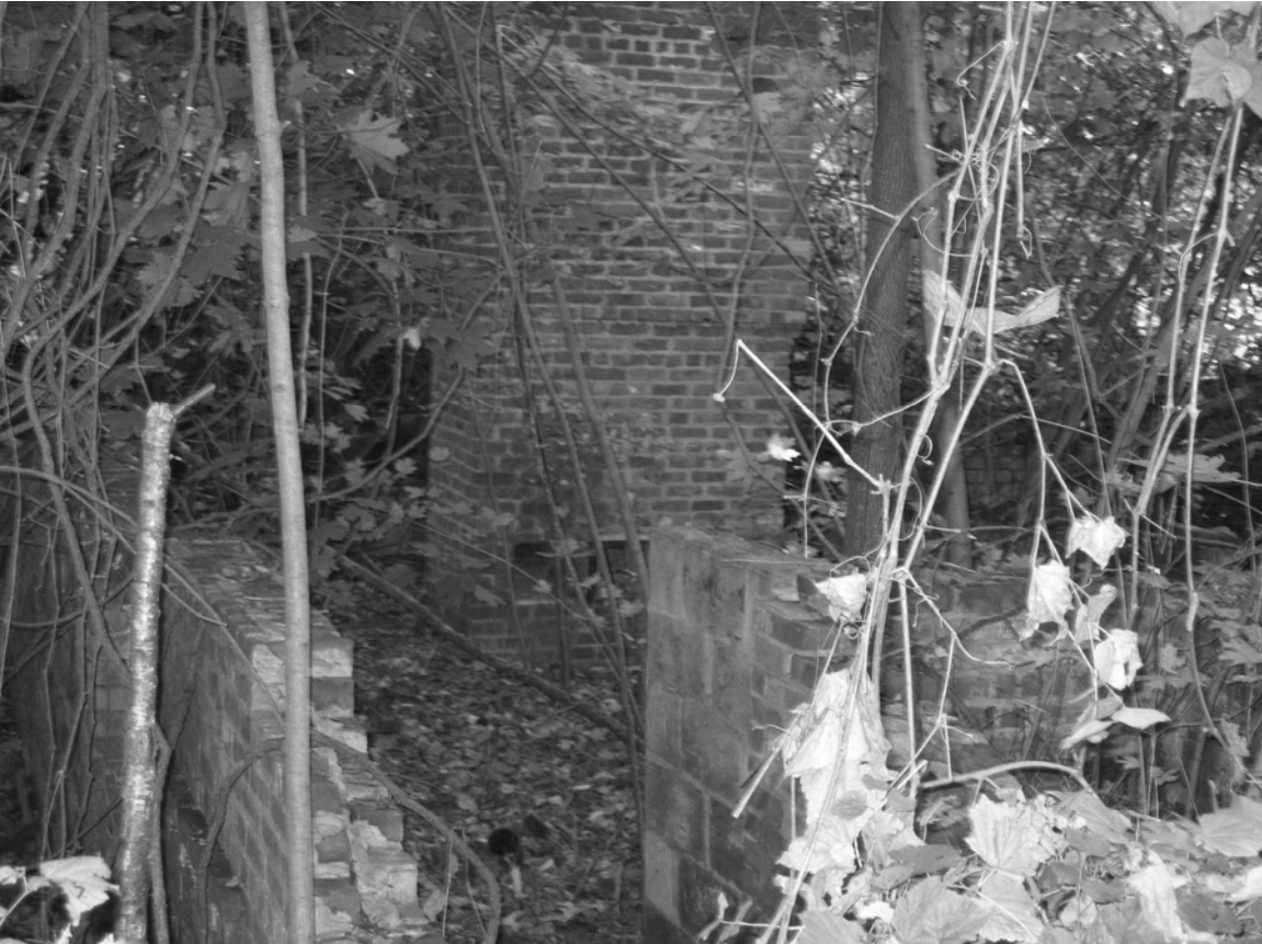
Photo 10. Foundation facing east.
