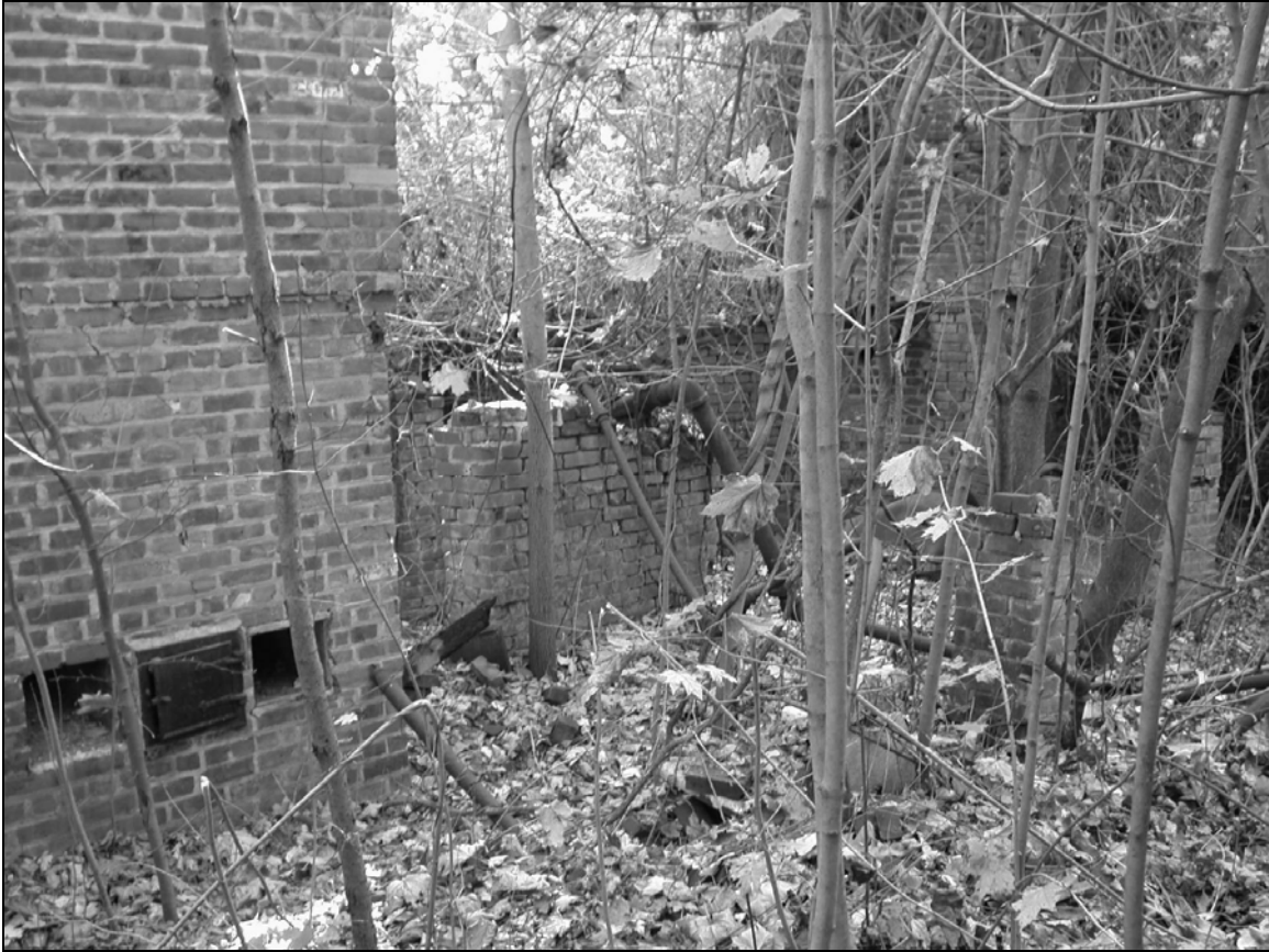
Photo 1. General view of site interior.
